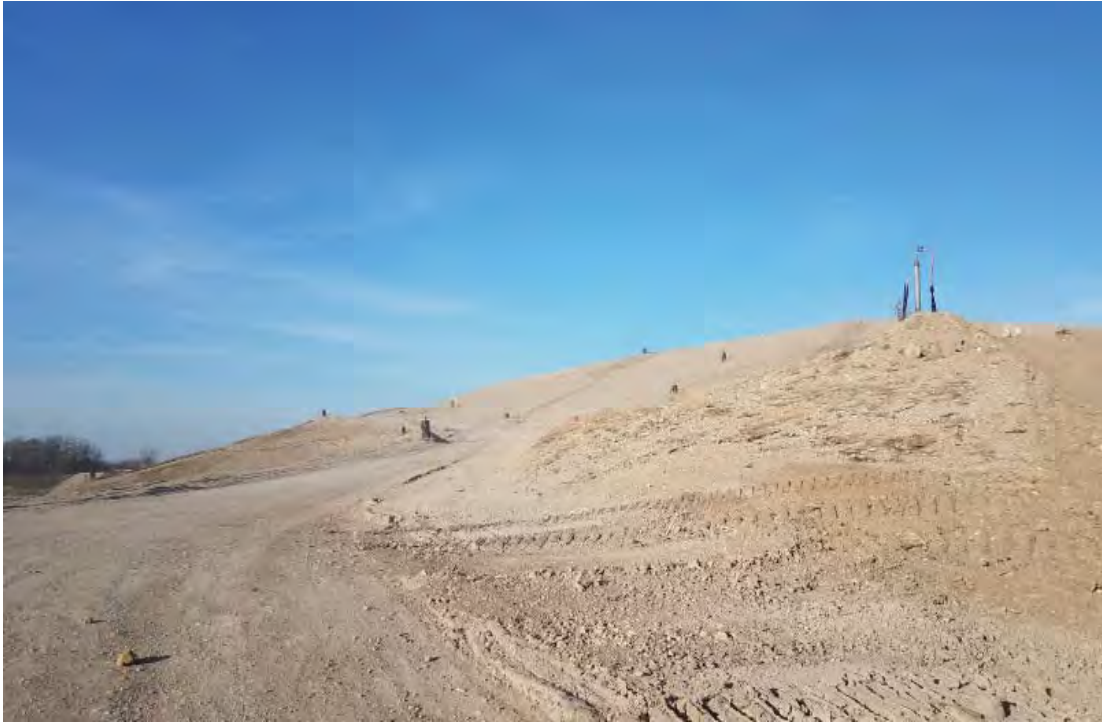
Access road with trench well on right hand side for gas collection
