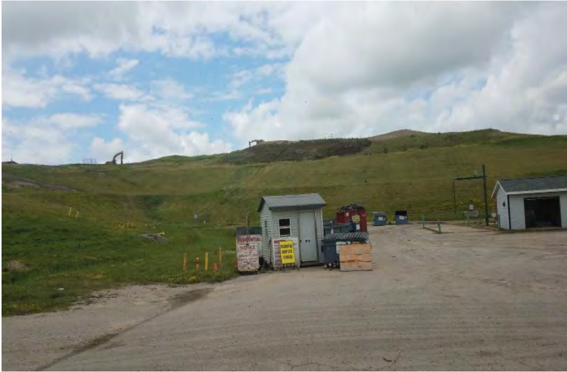
Phases 4 and 3, soil being excavated from on top of Phase 3 for cover
