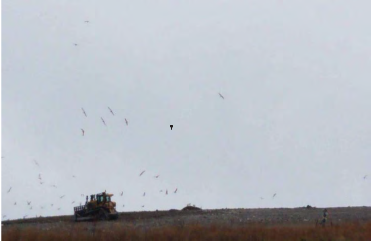
Dozer spreading cover on South top of slope of Phase 7 South
