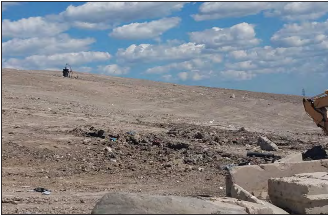
Excavation upslope of access road to address seeps and gas emissions. May not be capped by end of day, but will be by 6/26/2020
