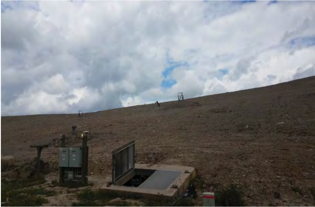
Vault at toe of Phase 7 South slope
