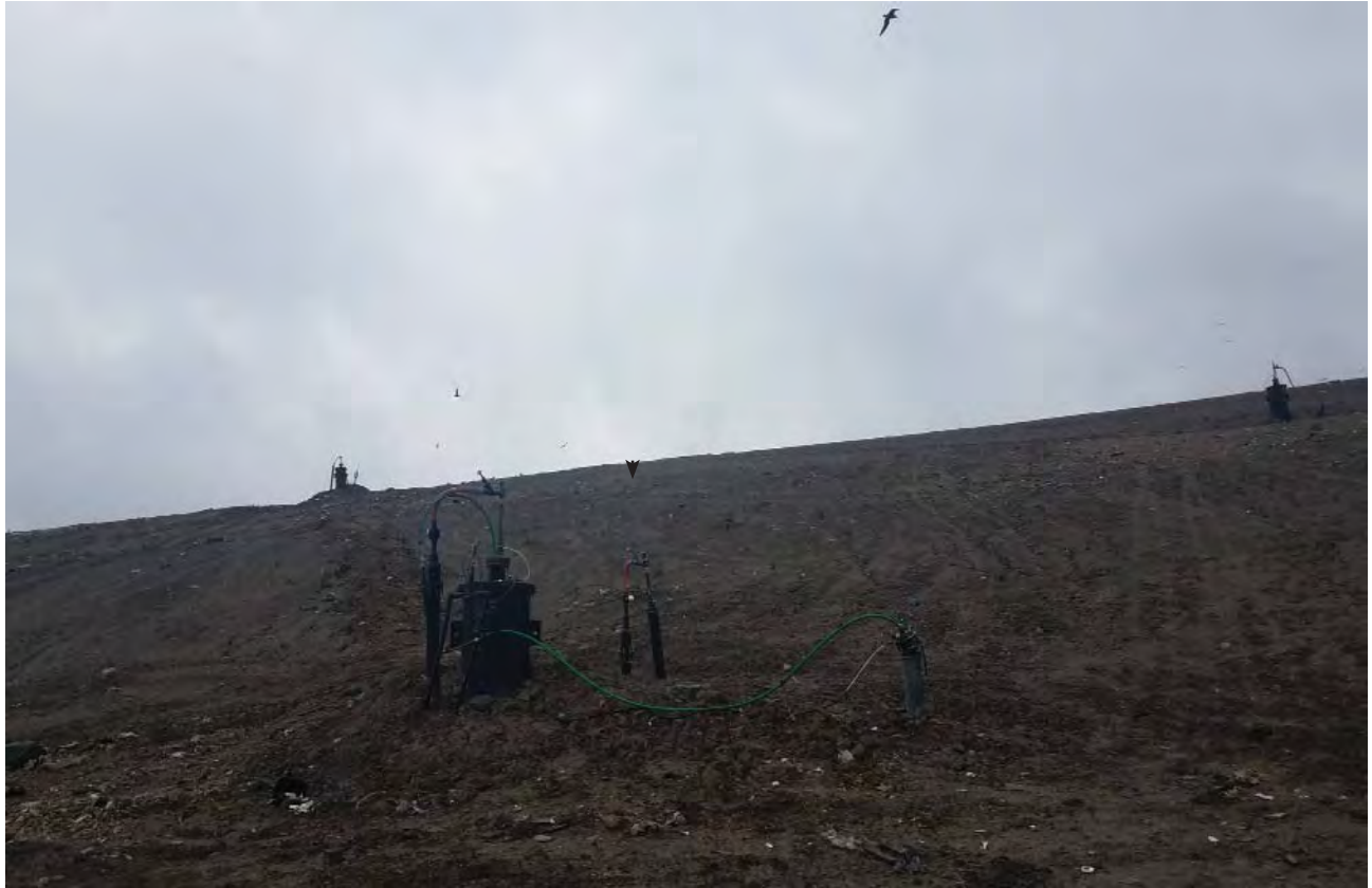
West slope of Phase 7 South, improved gas collection
