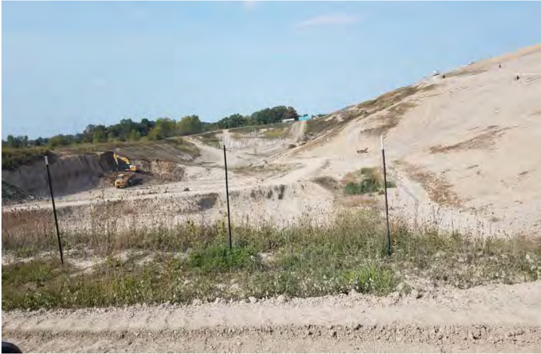
View North into Temp Sed Basin
