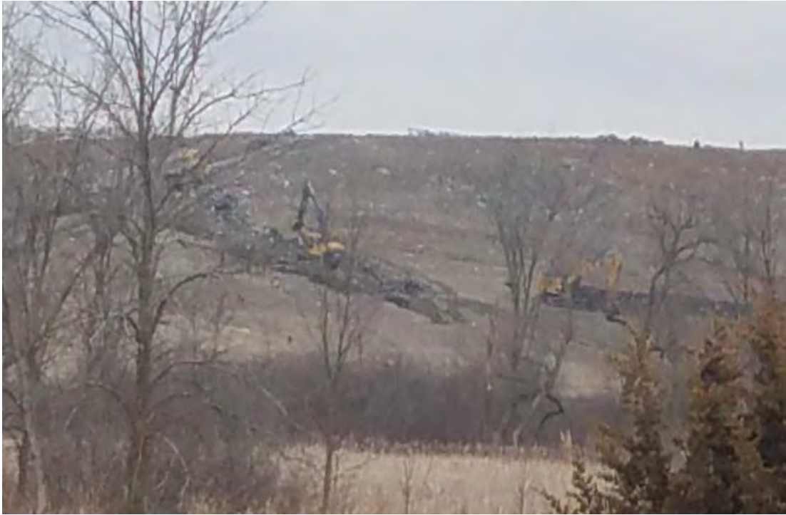
Trenching on Phase 7 slopes for the installation of air and force main lines
