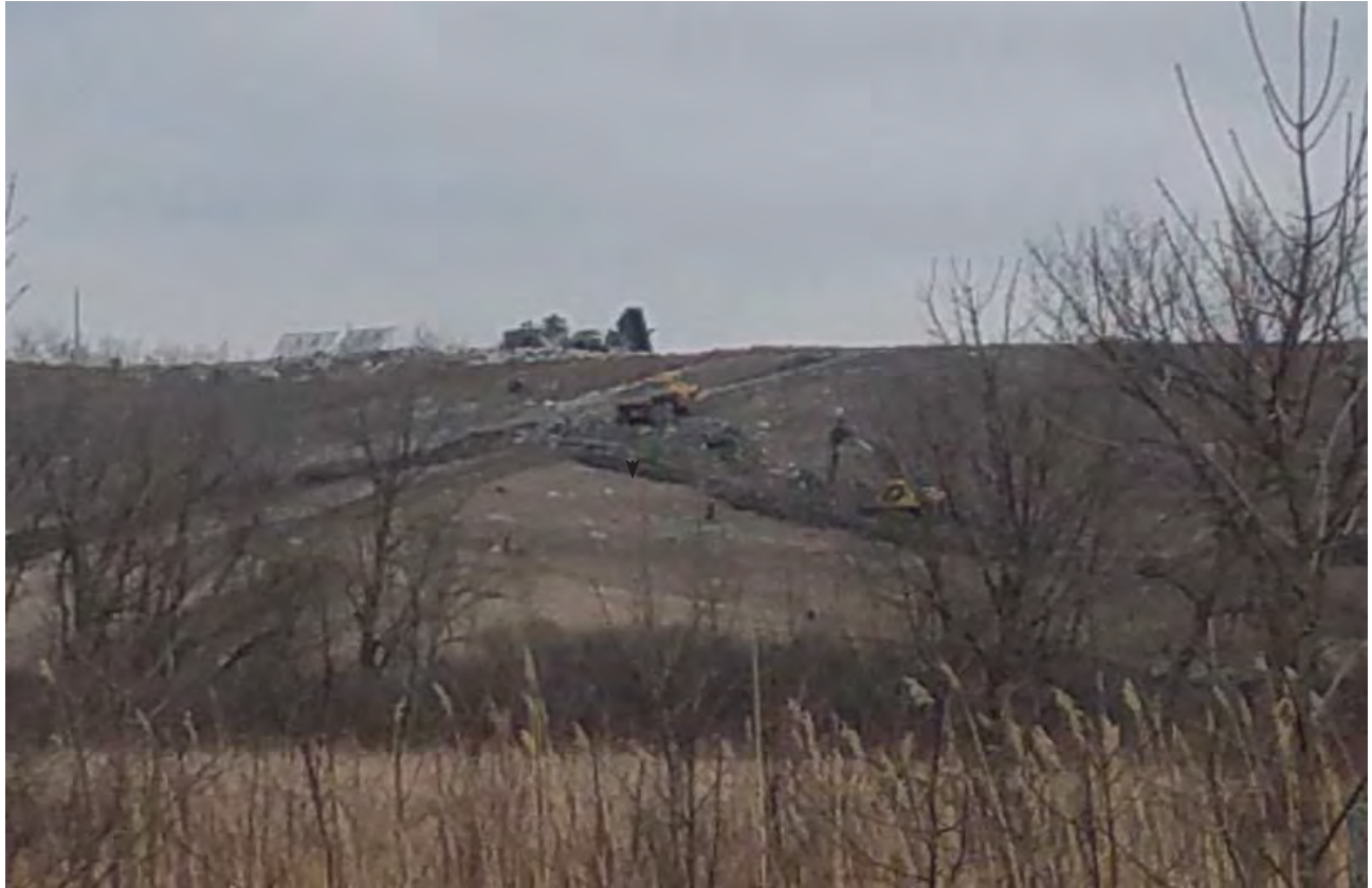
Trenching on Phase 7 slopes for the installation of air and force main lines
