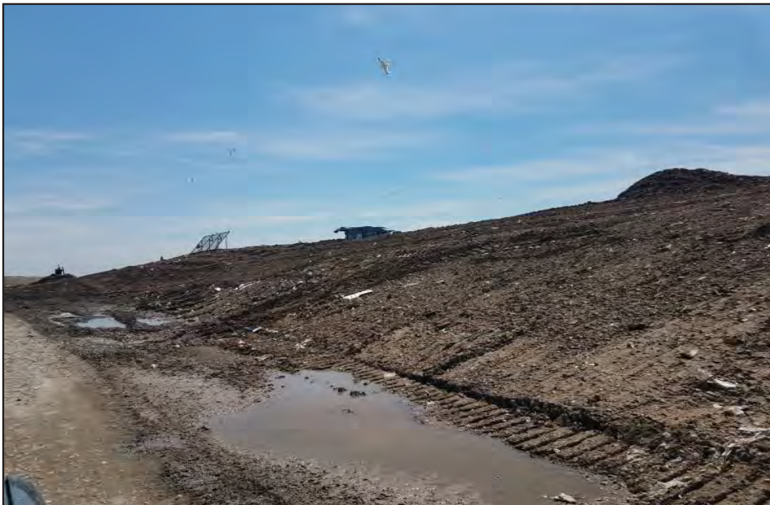
Wet area above previously repaired seeps along access road
