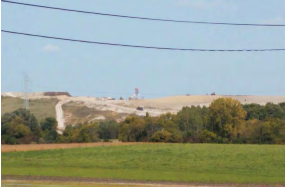
Phase 3 & 7 viewed from a distance and the West
