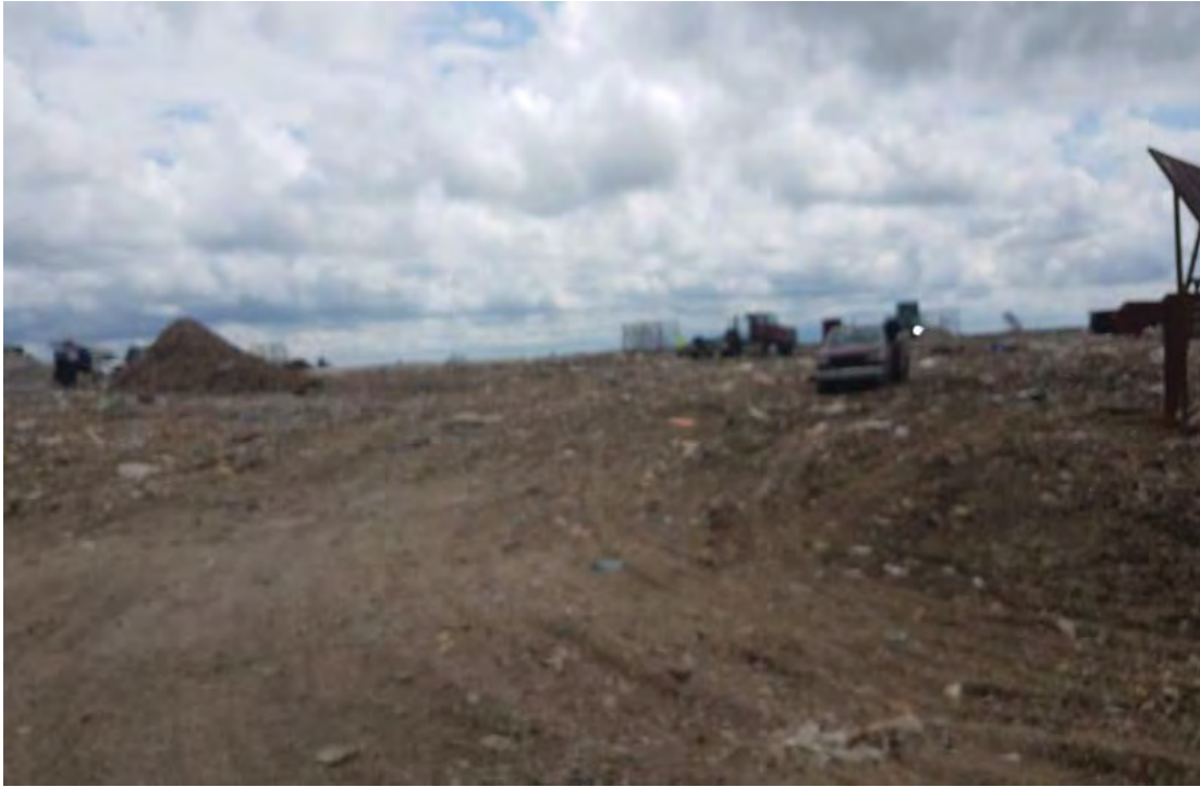
Phase 7 viewed from the North
