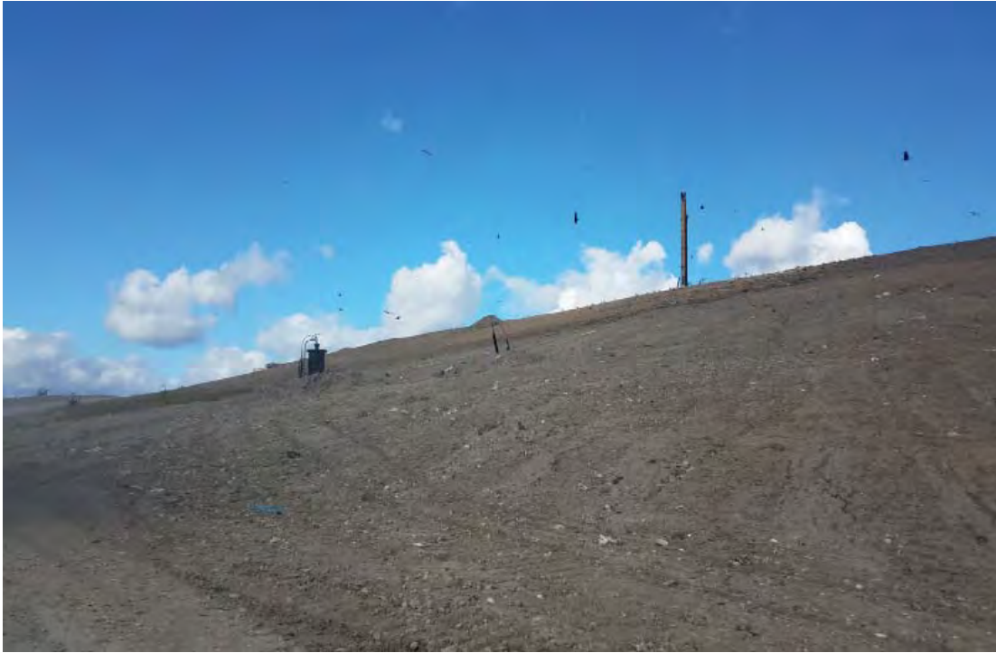
Phase 7 South West slope redressed.
