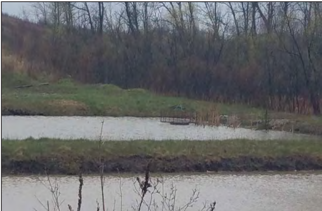
Control Structure of Basin 2
