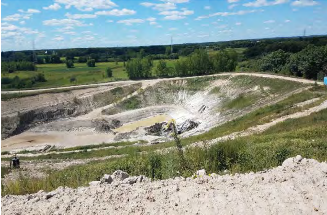
Temp sed basin viewed from Phase 7, not seep in sed basin in the South portion
