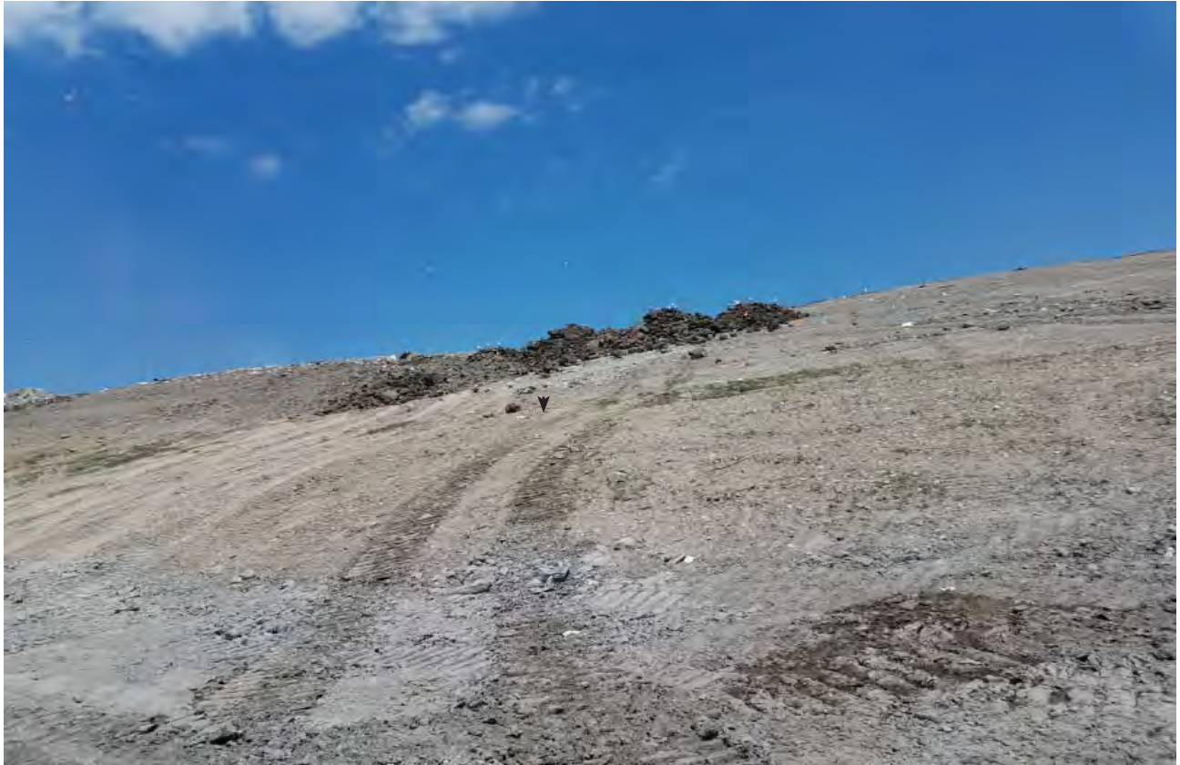
Working face at top of slope, soils stockpiled for daily cover
