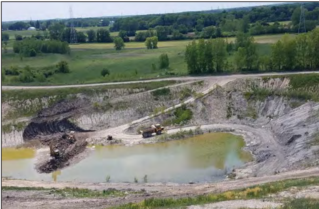
North end of temp sed basin, pumping from this area to tanker
