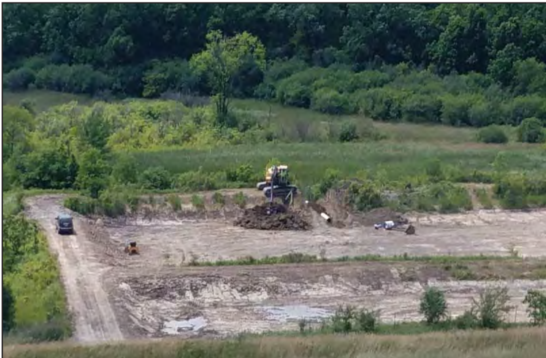
Basin #1 cleaned and restored, new control structure being installed
