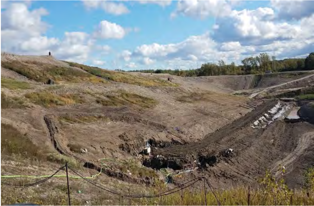
Excavation to sump adjacent to temp sed basin
