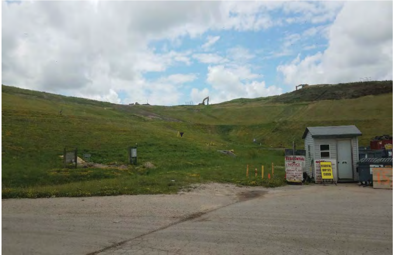
Slope repair on North slope of Phase 4, upper middle of Photo
