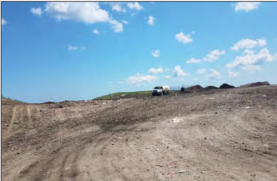
Working face in Phase 7 North/South boundary
