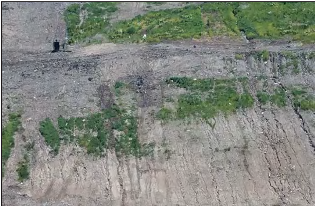
Seep repair on West slope of Phase 7 North, was a large seep
