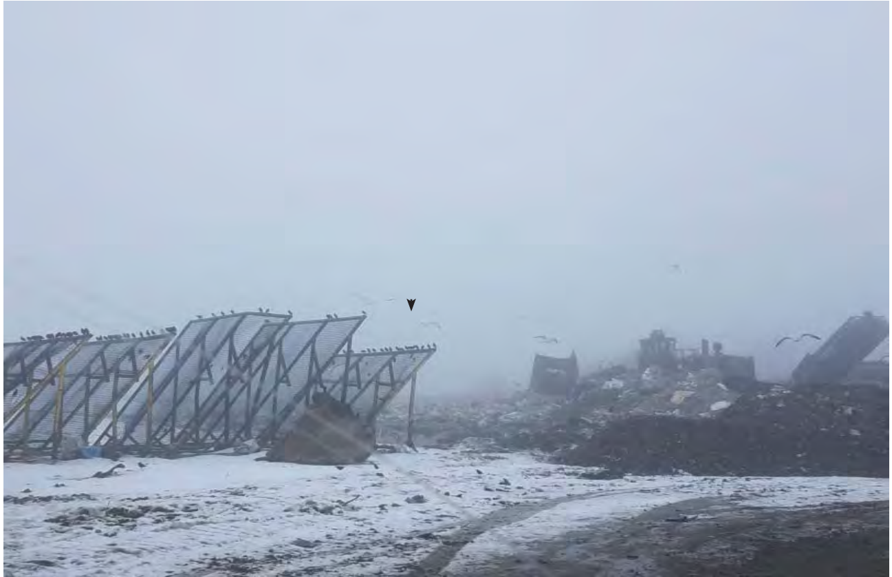
Working face viewed from the North. Cover stockpile to left
