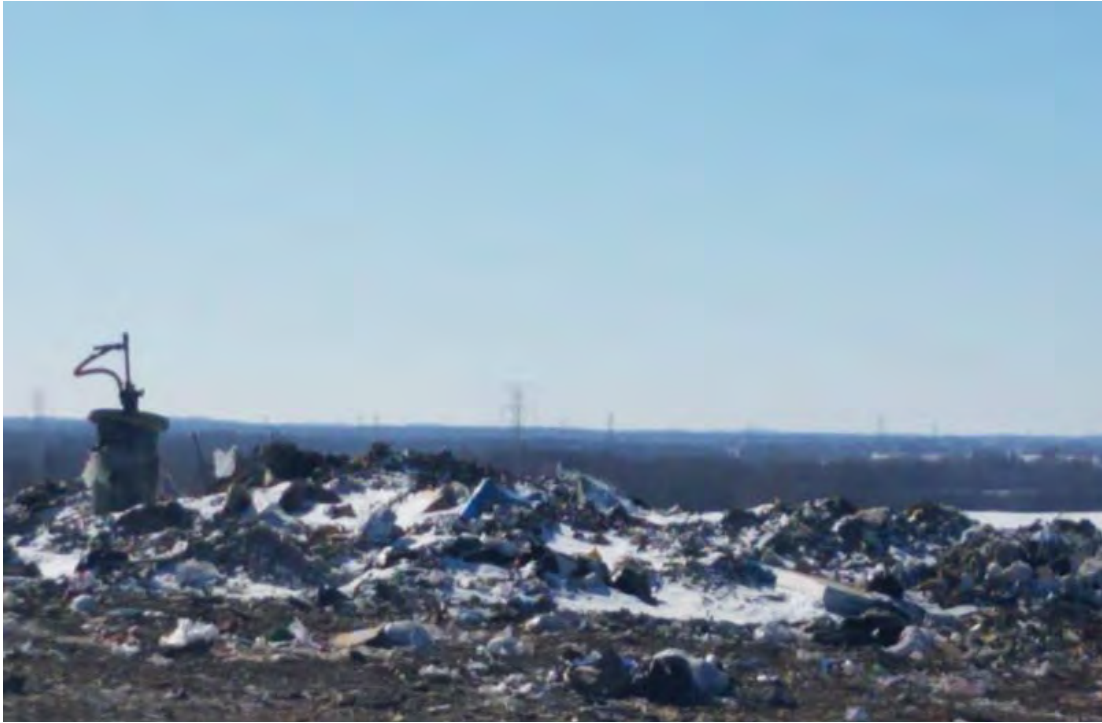
Previous covered waste and raised well
