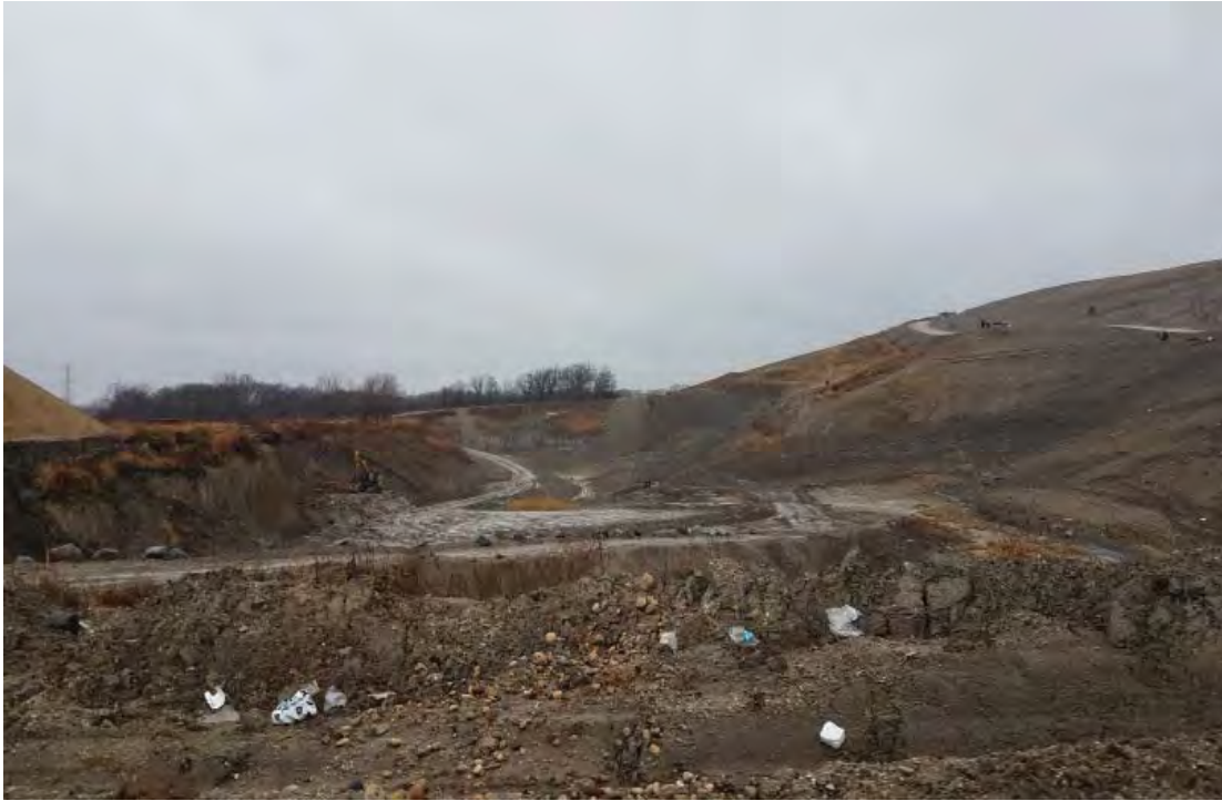
Temp sed basin viewed from access road to the South
