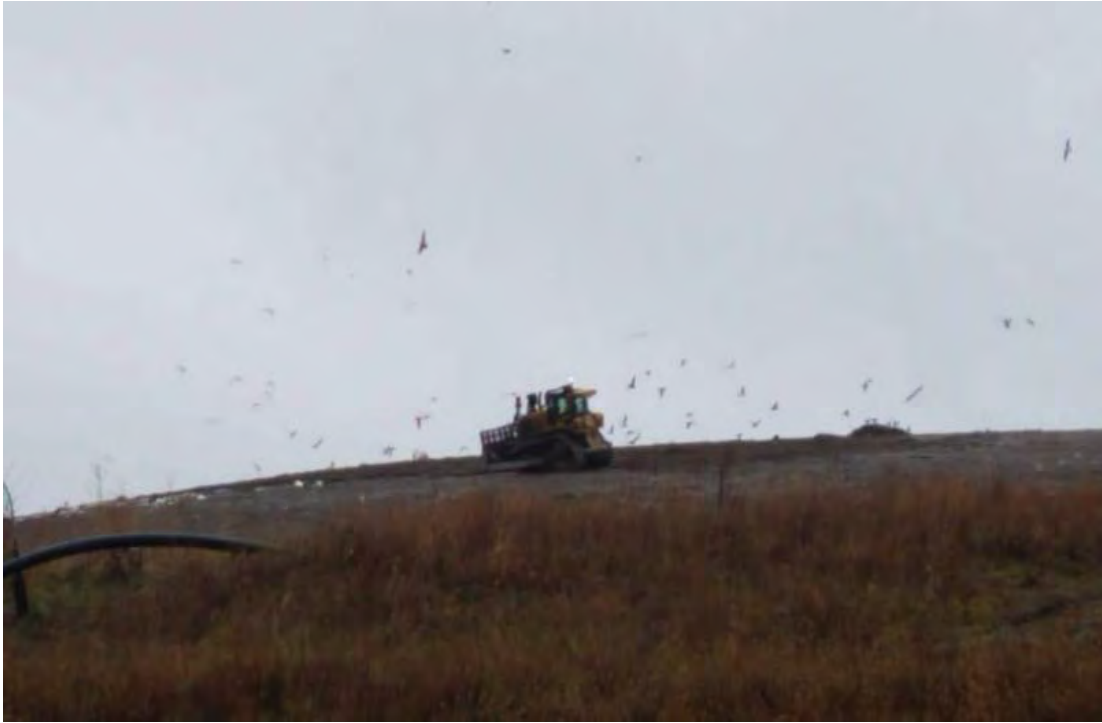
Dozer spreading cover on South top of slope of Phase 7 South
