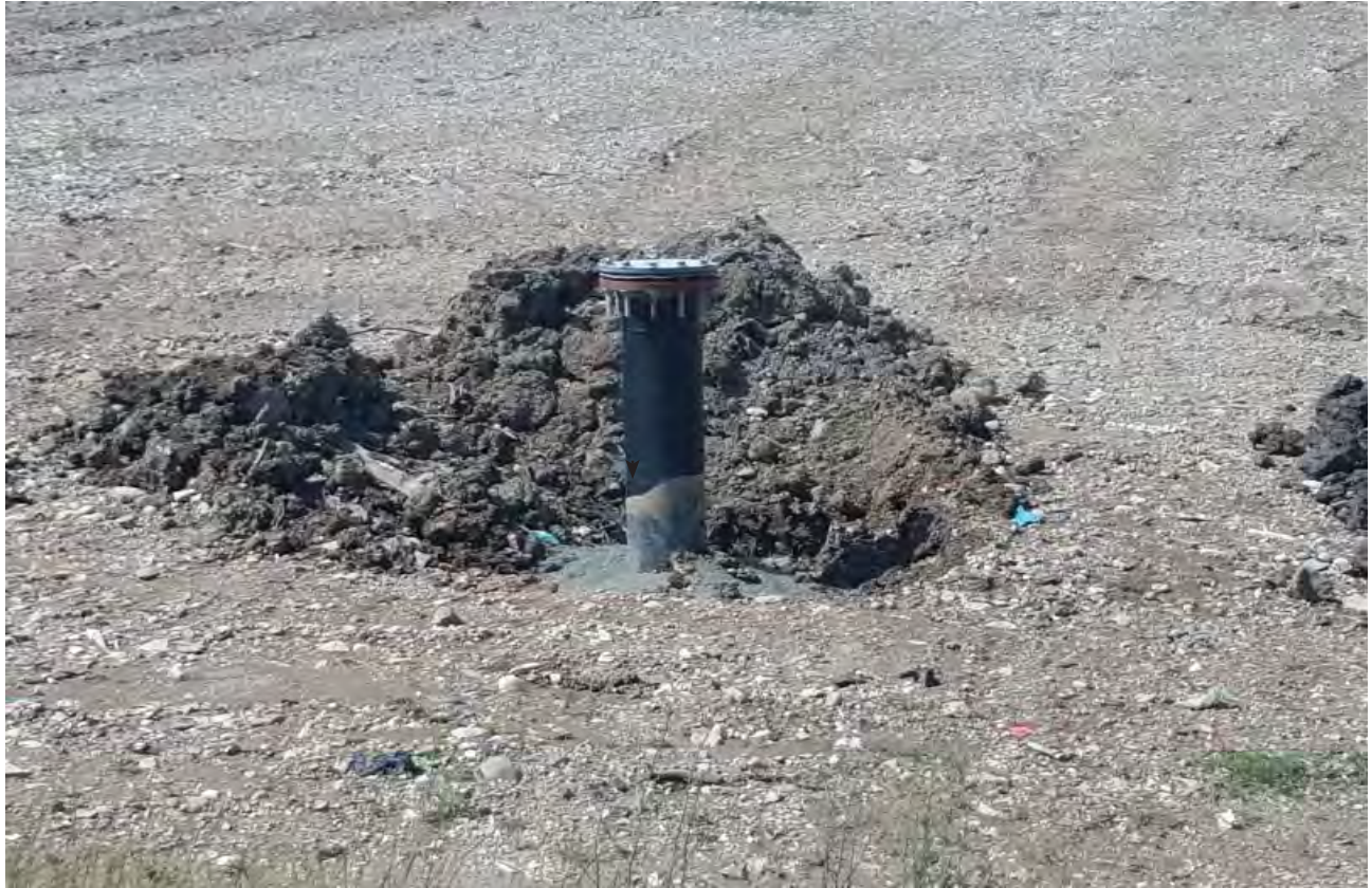
Bentonite and clay sealing about well heads
