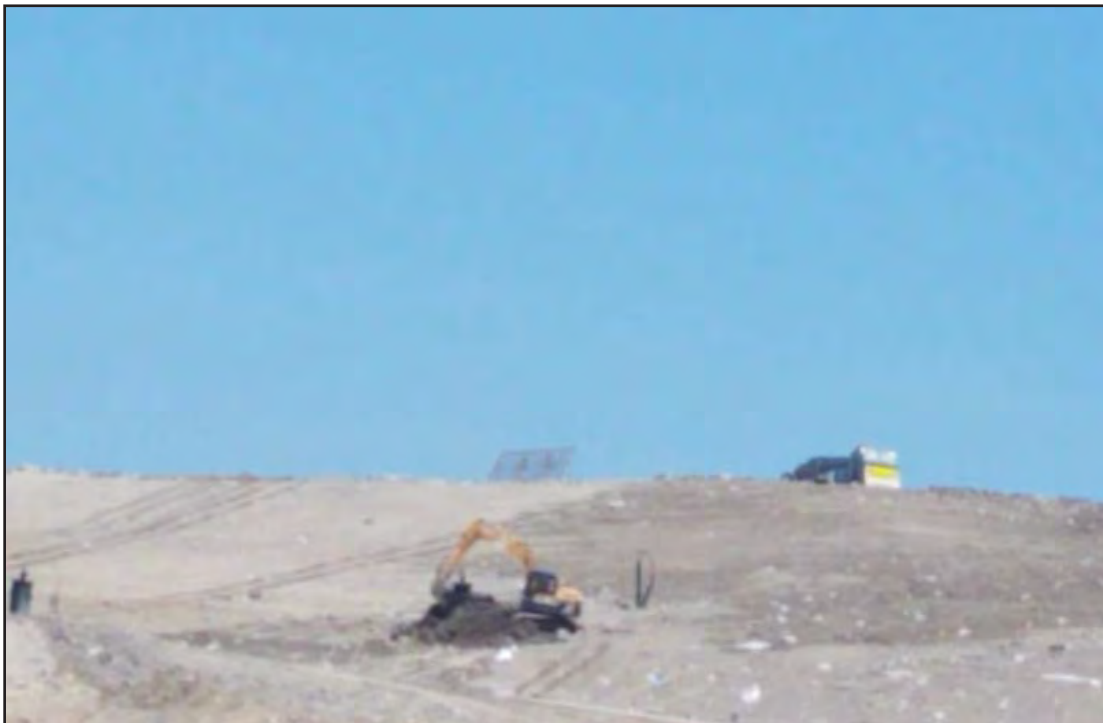
Slope repairs to improve gas collection
