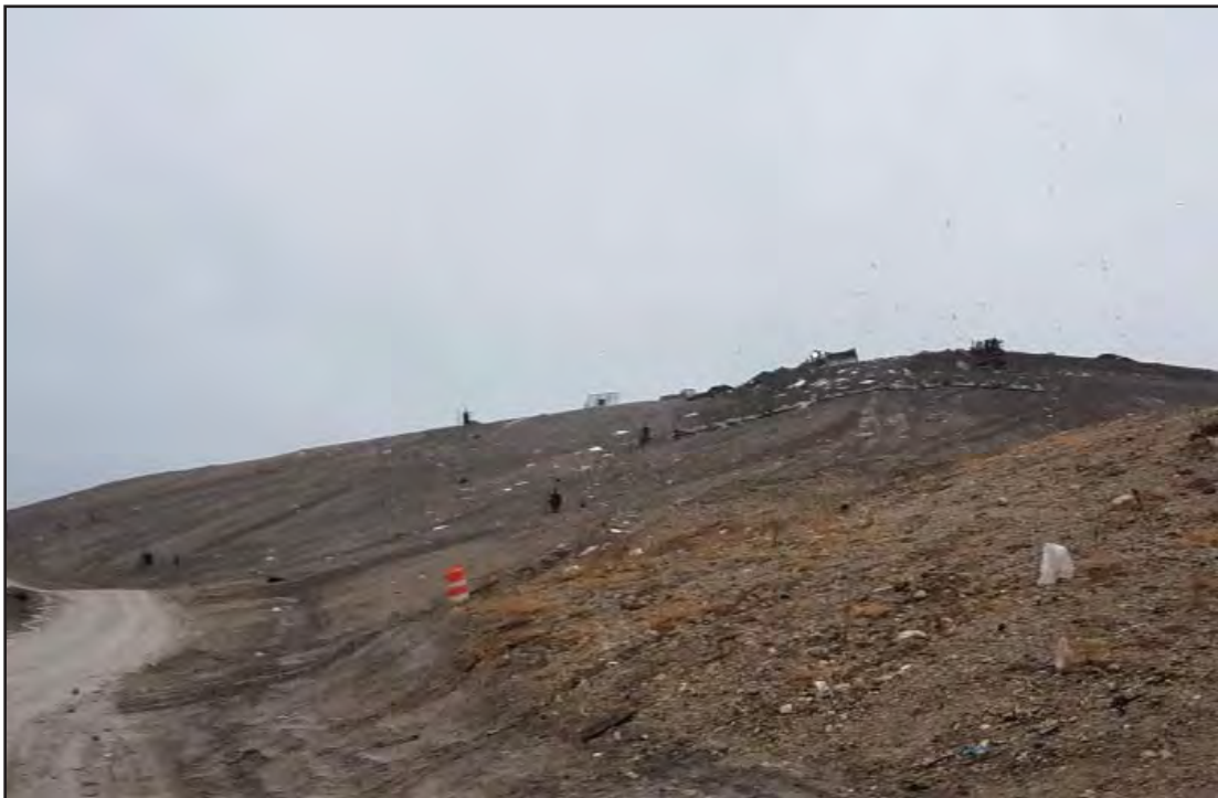
West slope of Phase 7, along access road, probable location of odors and placement of horizontal trench
