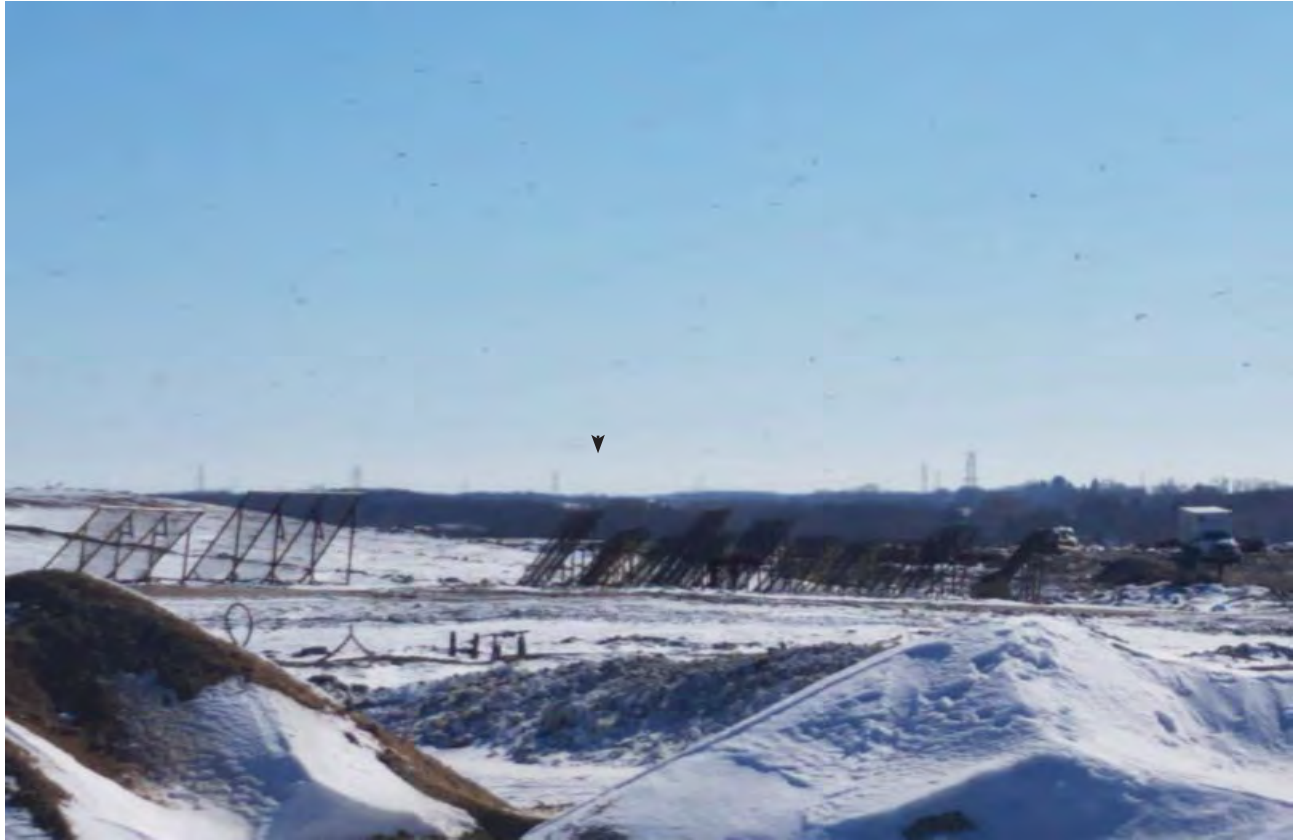
Fences placed to account for high winds
