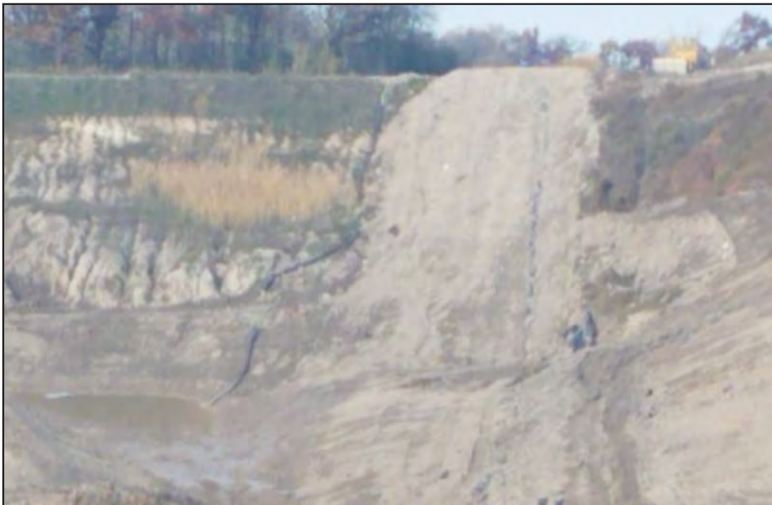
Rain flap and sump repair completed on West toe of slope, Phase 7
