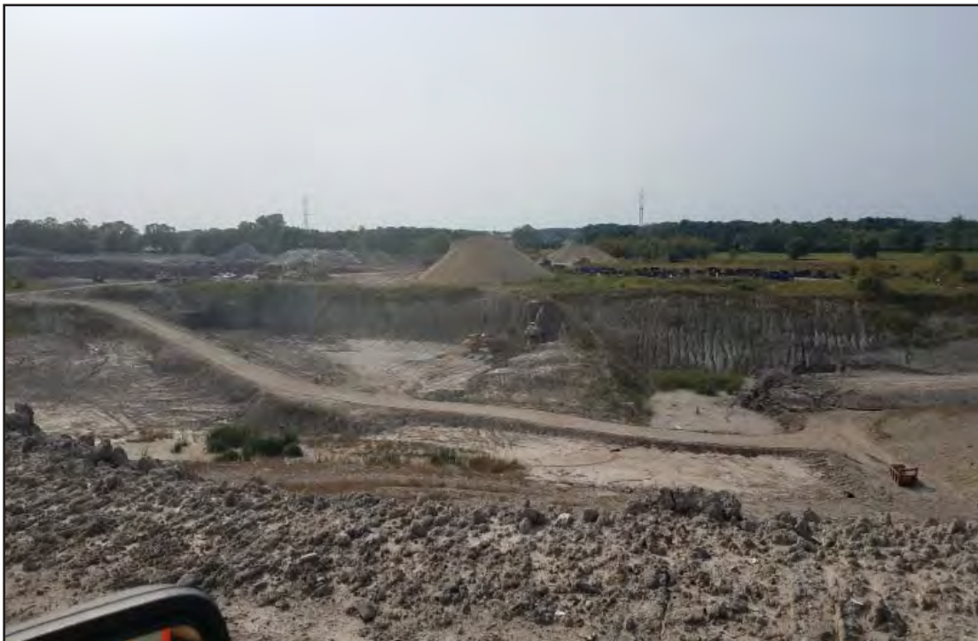
Temp sed basin, clean and dry
