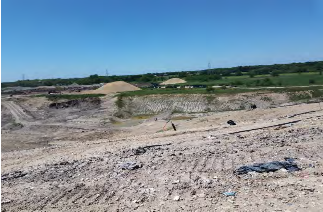
Previous cover and West slope of Phase 7 North viewed from East
