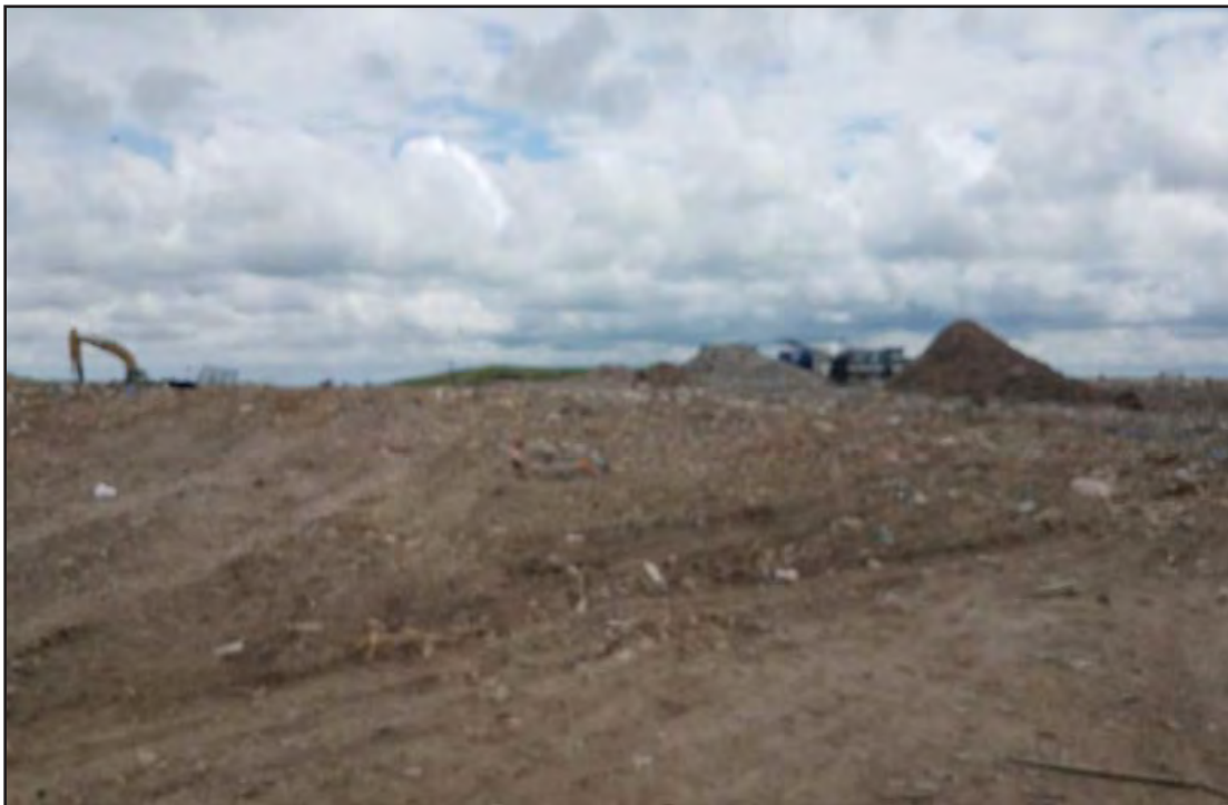
View across Phase 7
