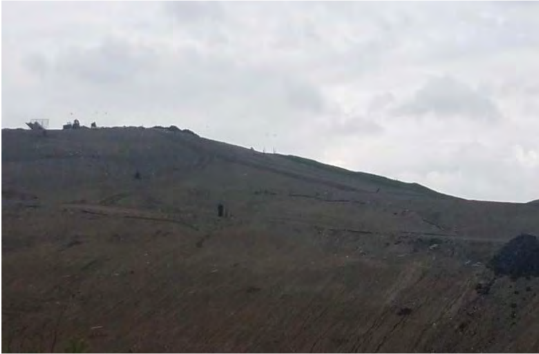
4. Southwest corner of Phase 7 South
