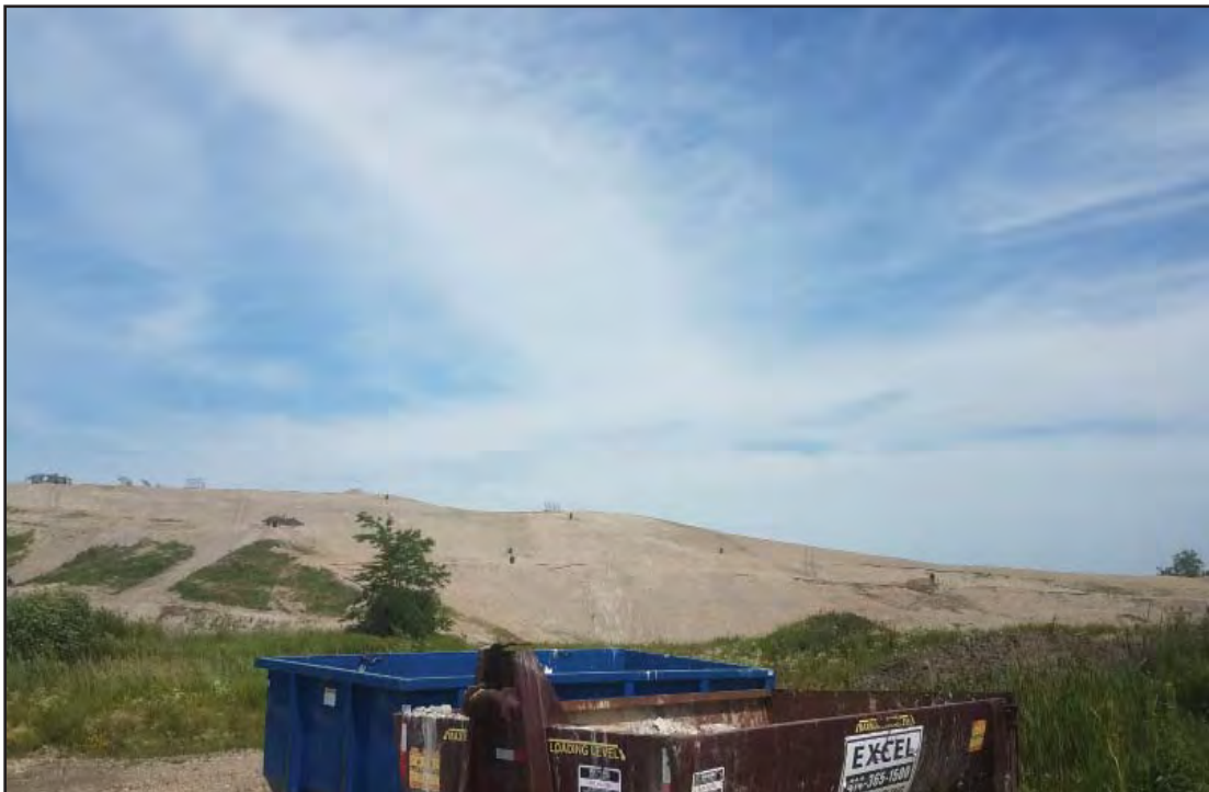
South end of Phase 7 viewed from the West
