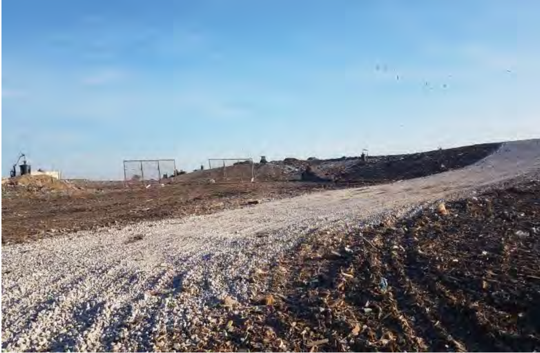
Travelway with stone to improve travel conditions across Phase 7
