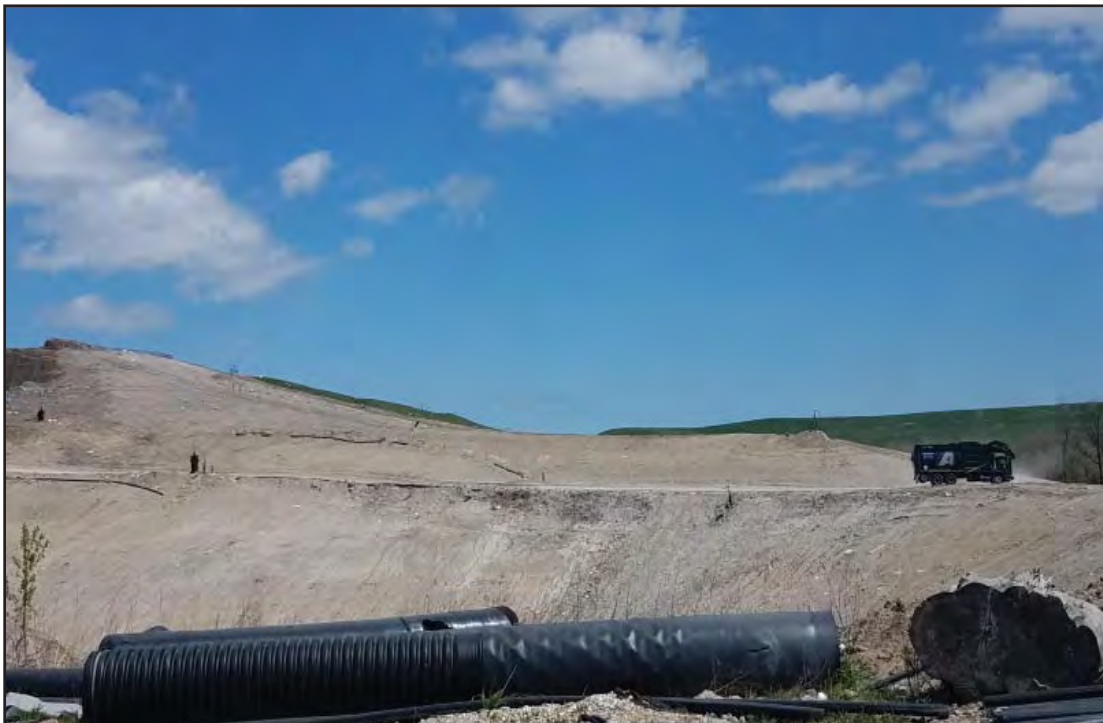
South edge of footprint viewed from West
