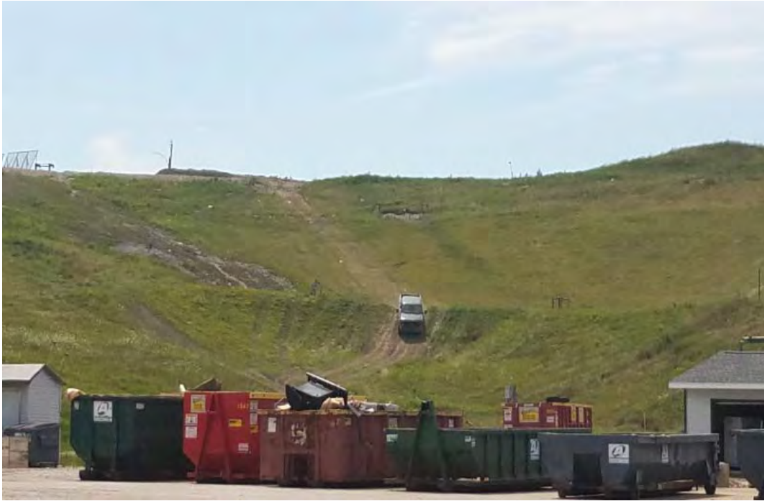
Travel over Phase 4 has started erosion locations
