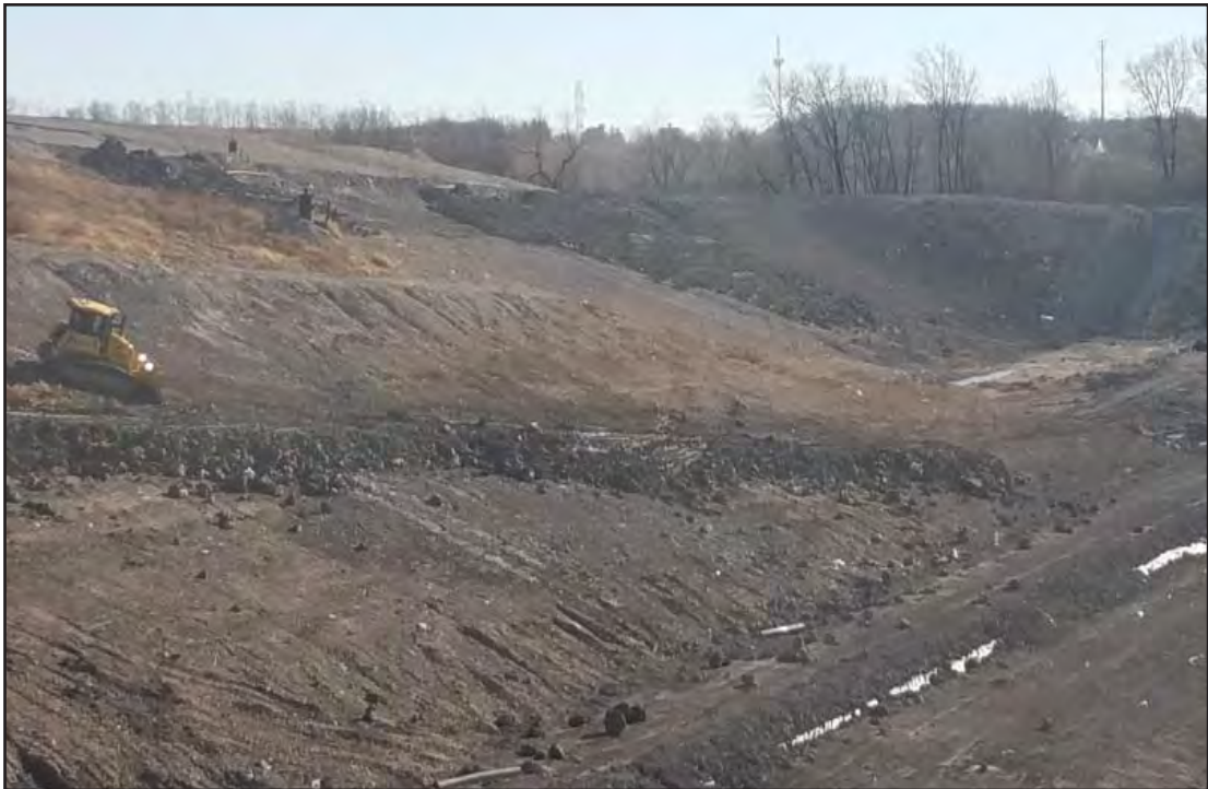
Berm development on West Slope of Phase 7
