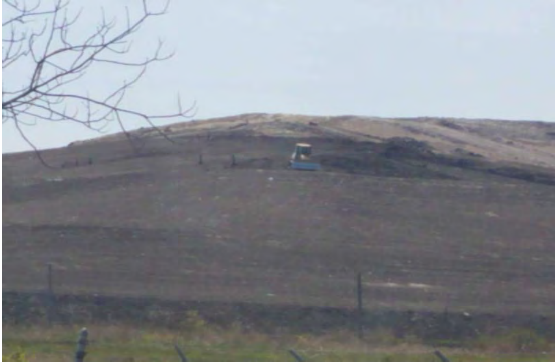
Cap development for Clearwater Pond Expansion
