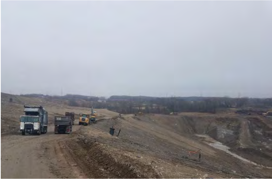
Installation of air line and force main by trenching and backfilling along West slope of Phase 7
