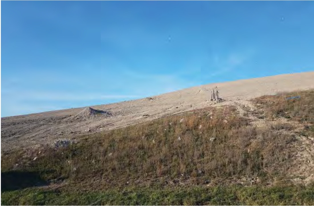
South slope of Phase 7 South and Phase 6, recently dressed with cover
