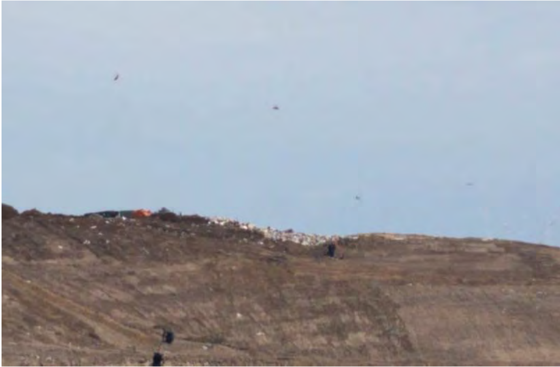
Edge of uncovered waste viewed from the West, in Phase 7 South
