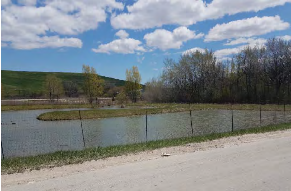
West slopes restored after trenching
