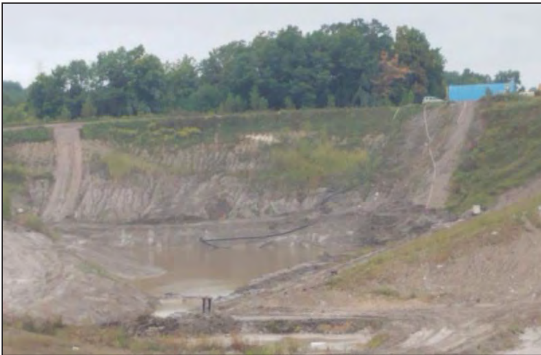
Temp sed basin viewed from South
