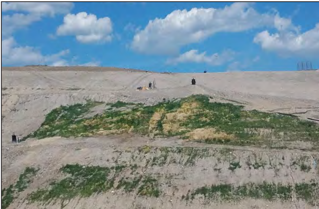
Vegetation slow to grow on West slope of Phase 7. Yellowing areas are potentially evidence of vegetative stress caused by LFG
