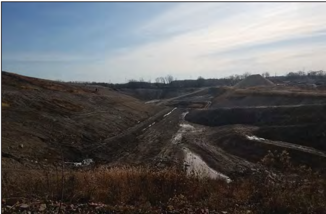
Temp sed basin and repaired rainflap with new access road
