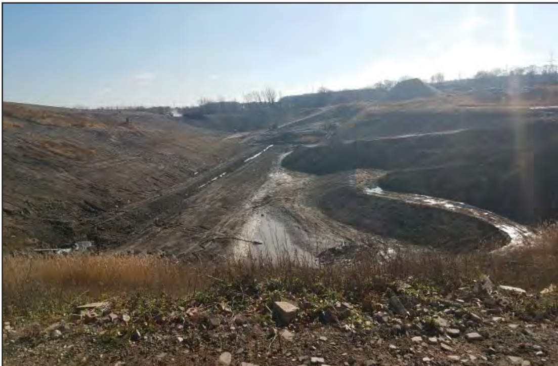
Temp sed basin viewed from the North, and repaired rain flap and berm
