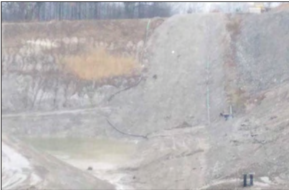
Temp sed basin and leachate header viewed from the South
