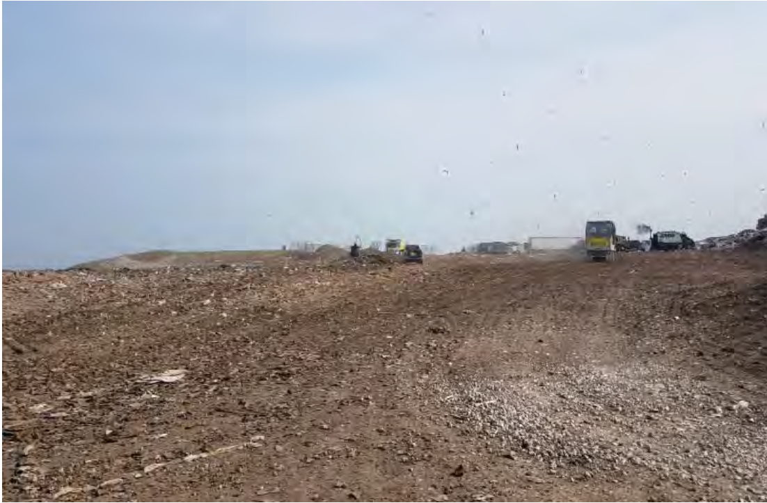
East portion of Phase 7, viewed from North, working face and new lift to the right of picture
