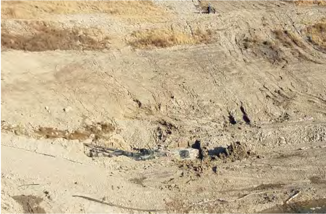
Repaired rainflap, base of Phase 7 South, to be covered
