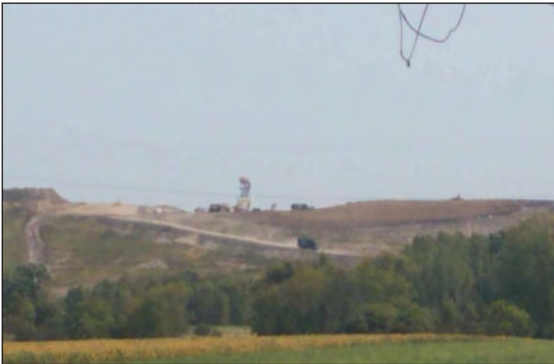
Overview of landfill from West
