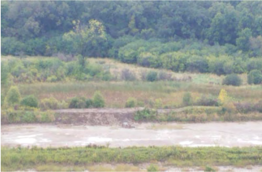
Basin #1, cleaned and control structure replaced
