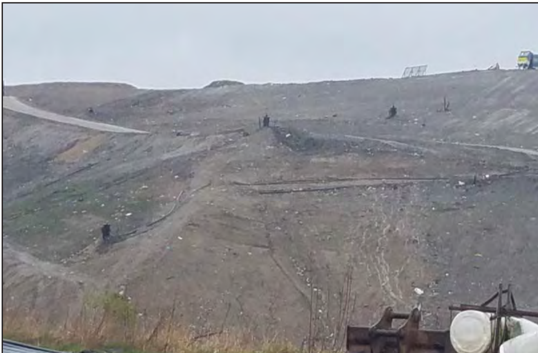
West slopes restored after trenching
