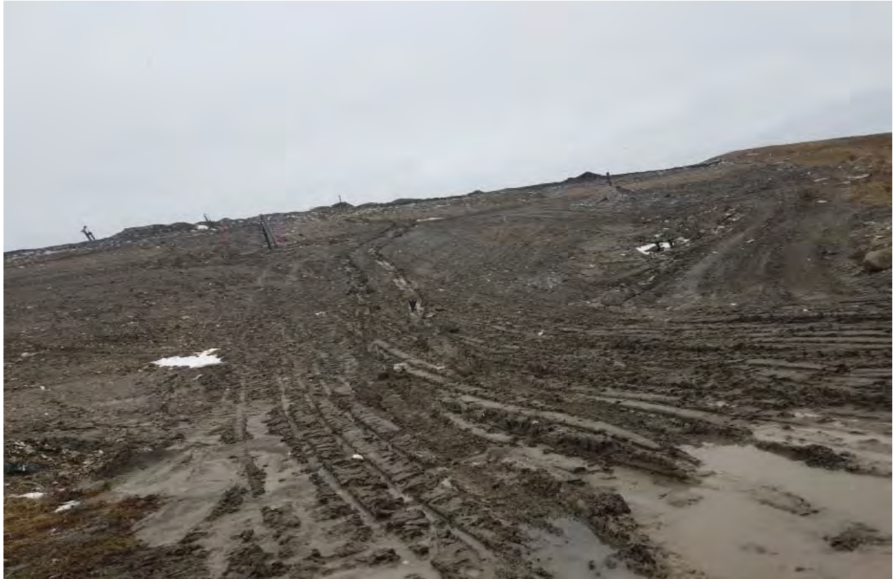
South slope of Phase 7 South, two new wells and well to be abandoned.
