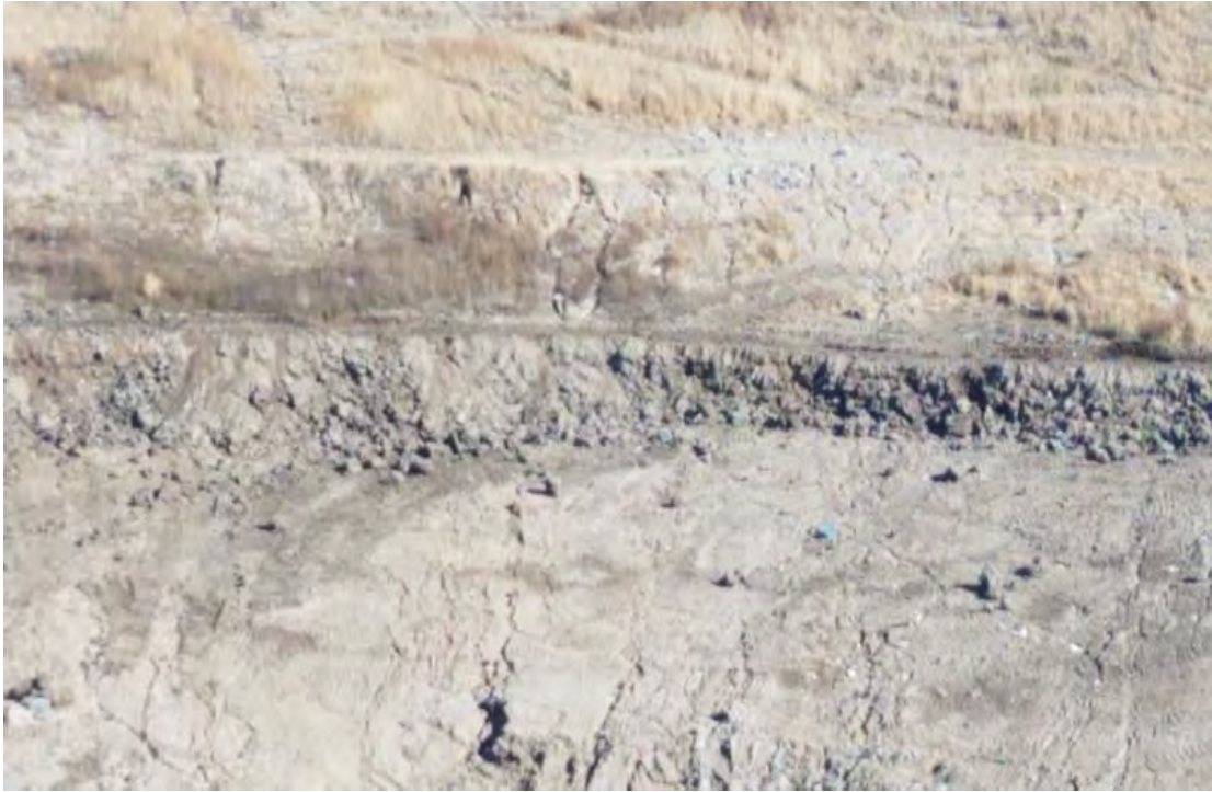
Berm development on West Slope of Phase 7
