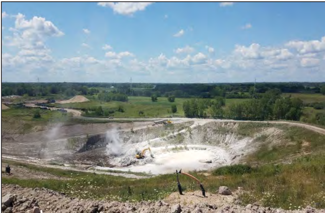
Overview of Temp Sed basin cleanup
