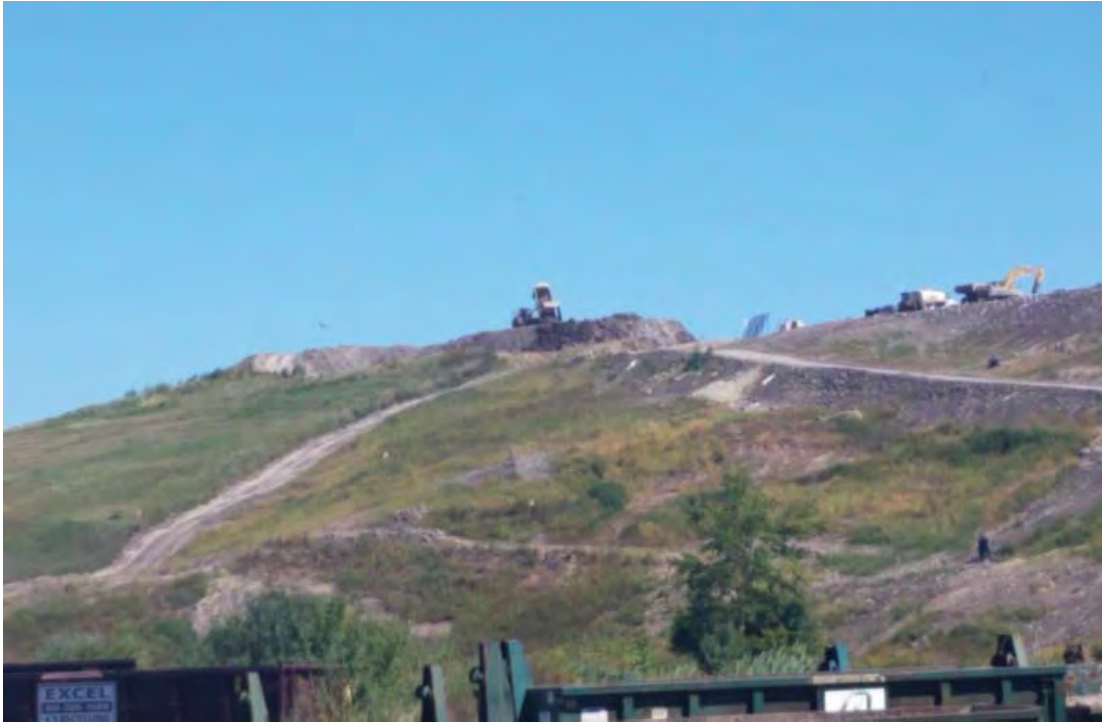
Stockpiling of soils from Temp Sed Basin on Phase 3
