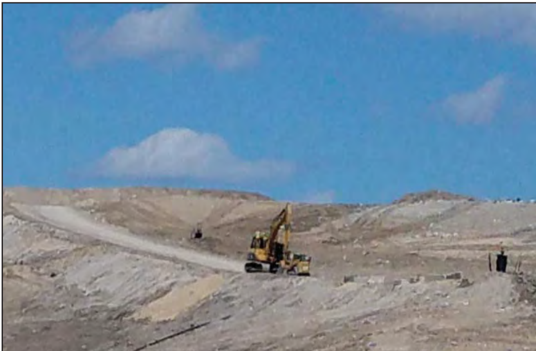
Trenching complete on West slopes and slope patched
