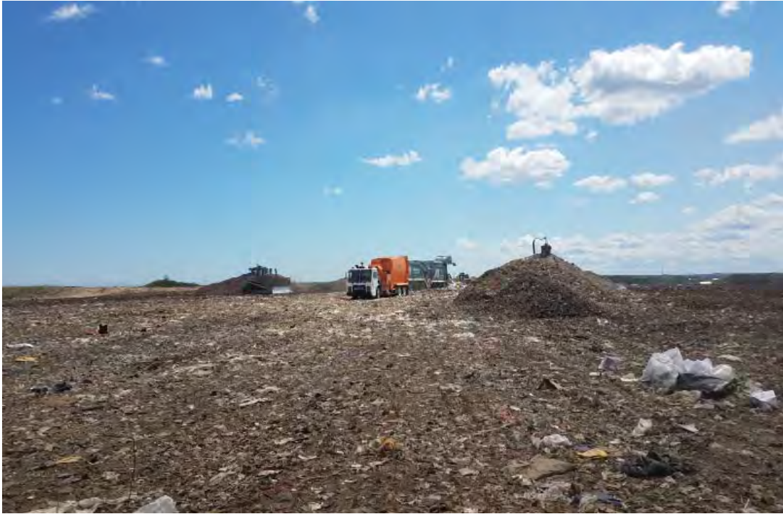
Working face in South end of Phase 7 South
