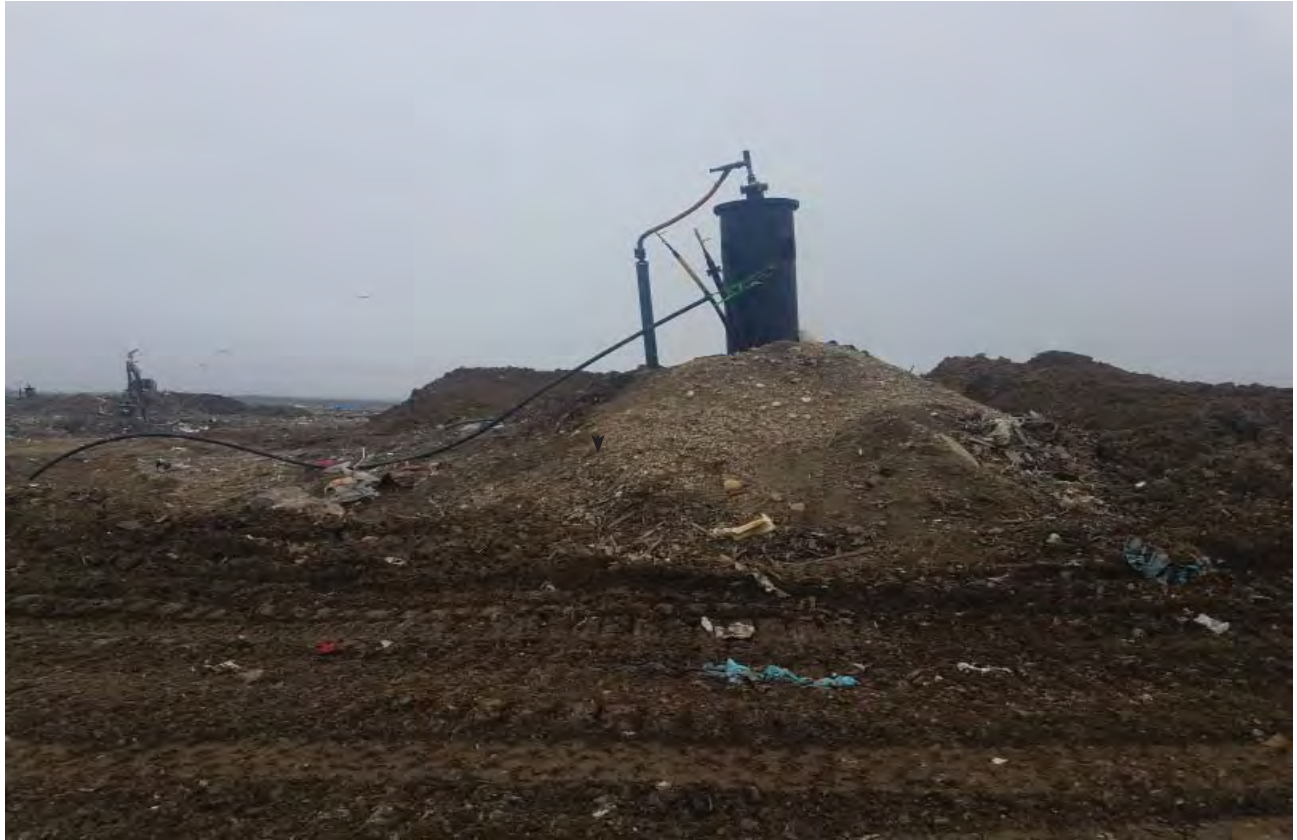
Raised well in Phase 7 North
