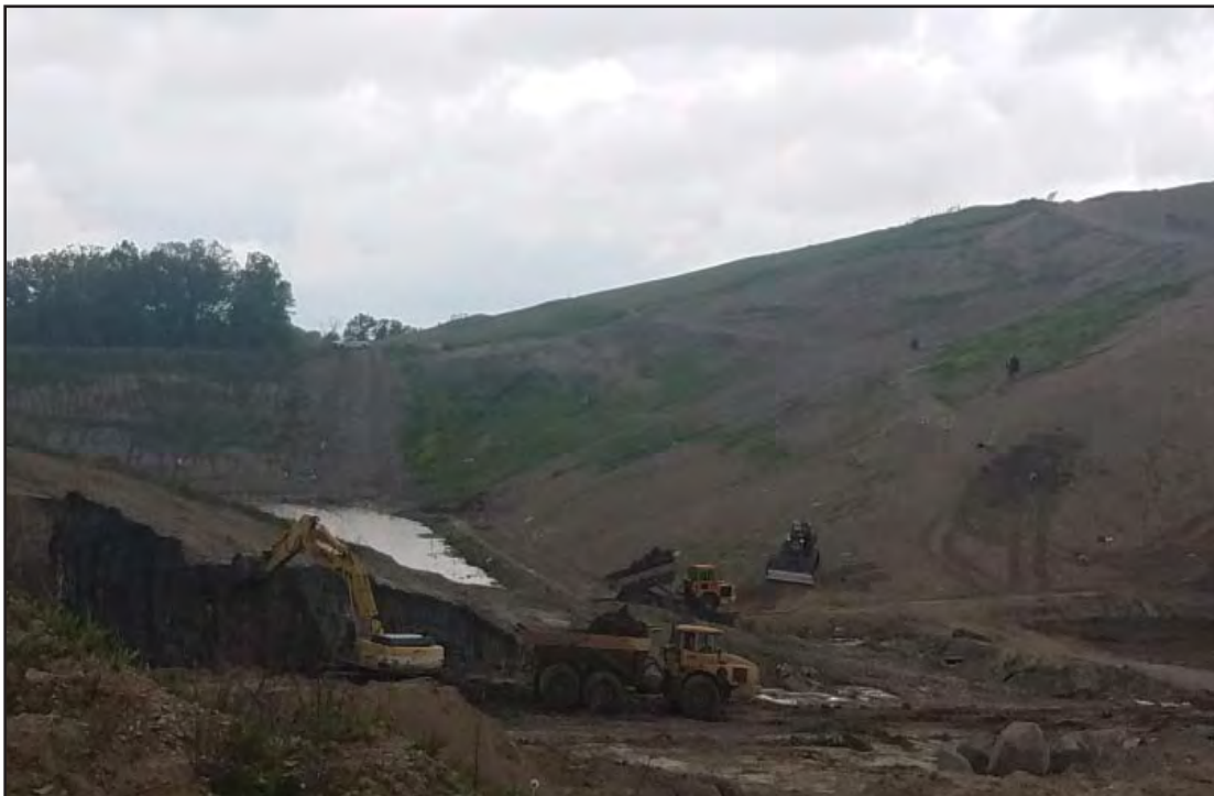
7. Excavation of future Phase 8, soil being used in the back ground at South end of Temp Sed Basin
