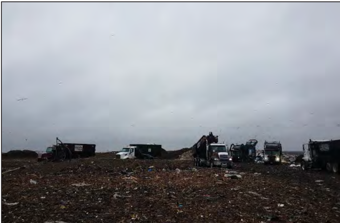
Working face very small and tucked up to create berm
