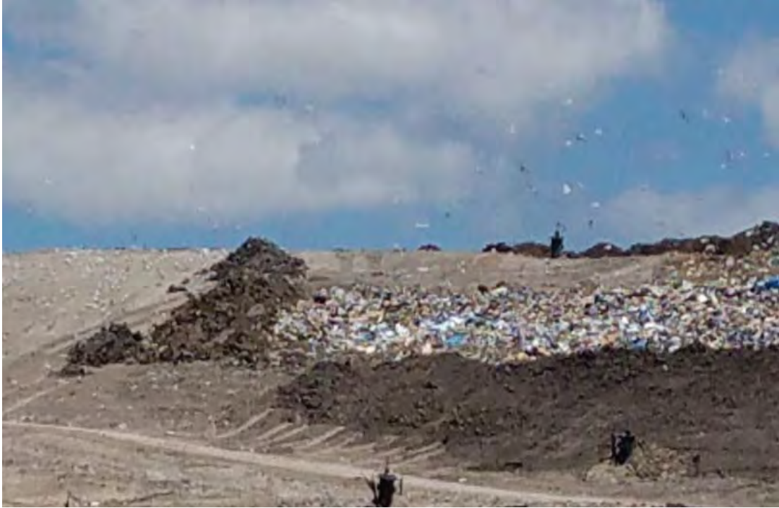
Phase 7 viewed from the West
