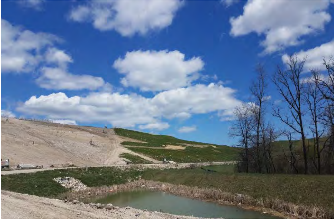
South slope, litter trapped in grasses on capped areas
