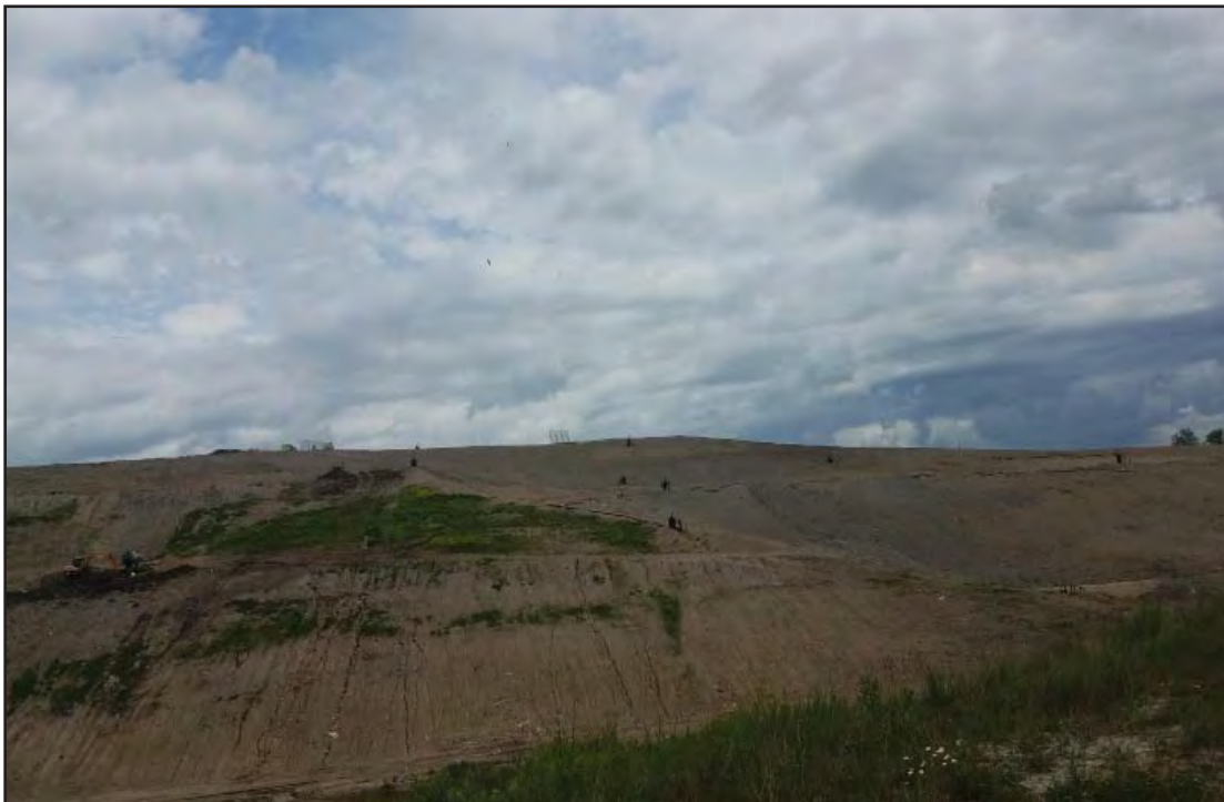
West slope of Phase 7 North
