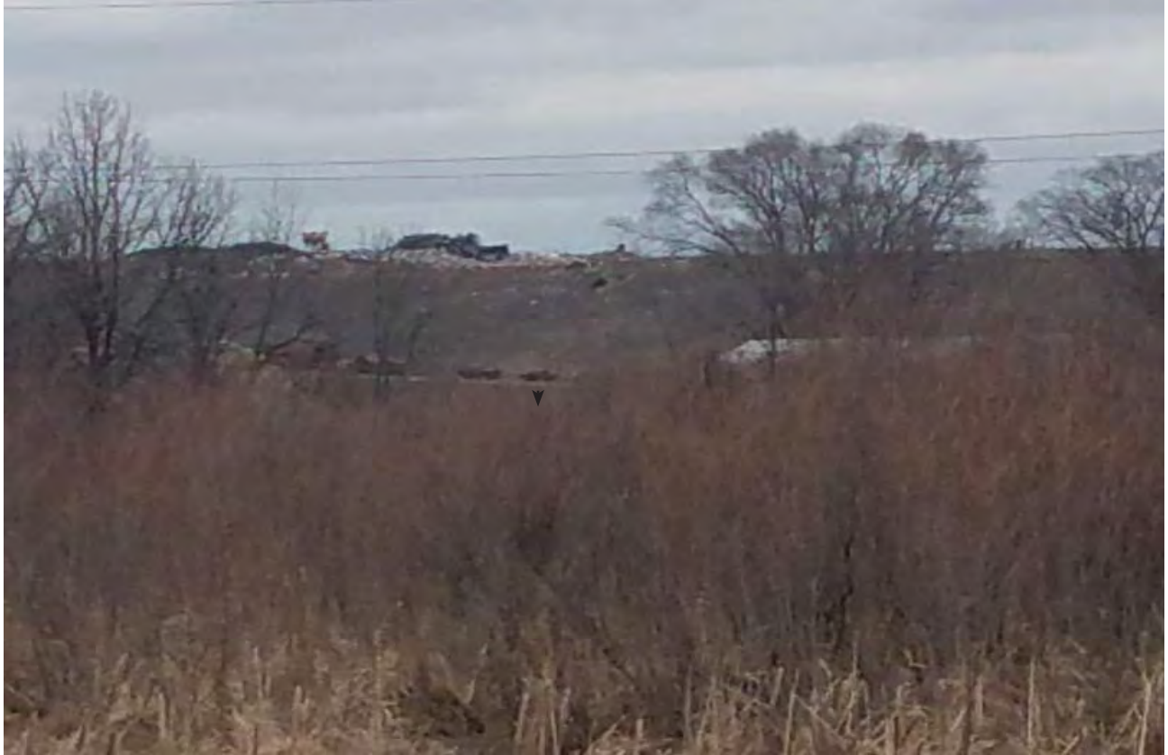
Working face and trenching project viewed from Union Church Road from the South
