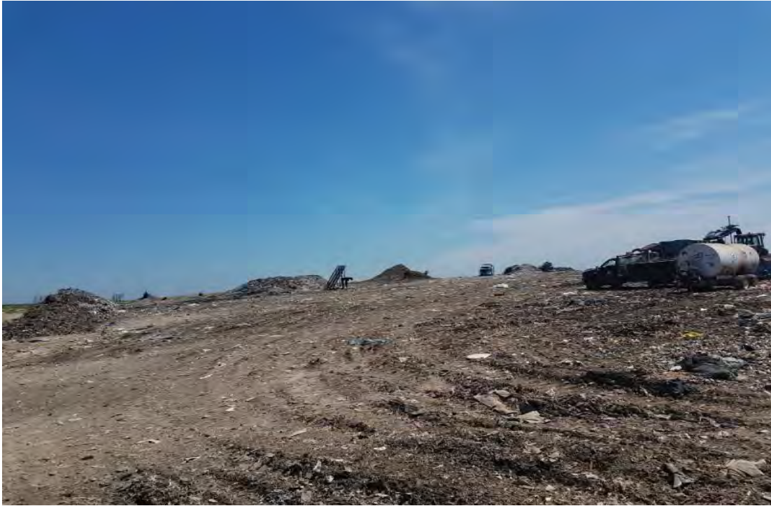
Current surface conditions about working face in Phase 7
