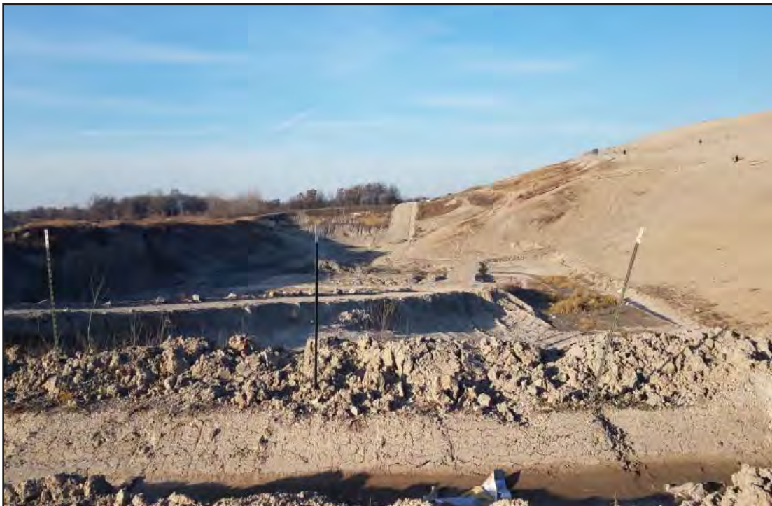
Temp sed basin viewed from the South
