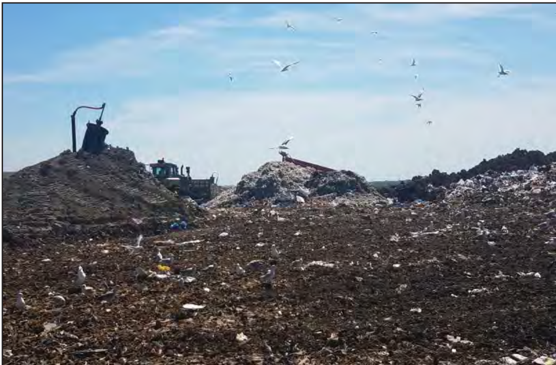
Protected wells and working face, well on left to be redrilled
