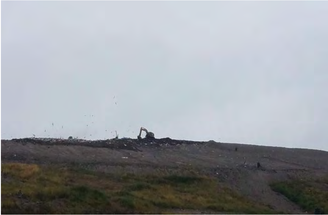
Well raising at top of West slope Phase 7
