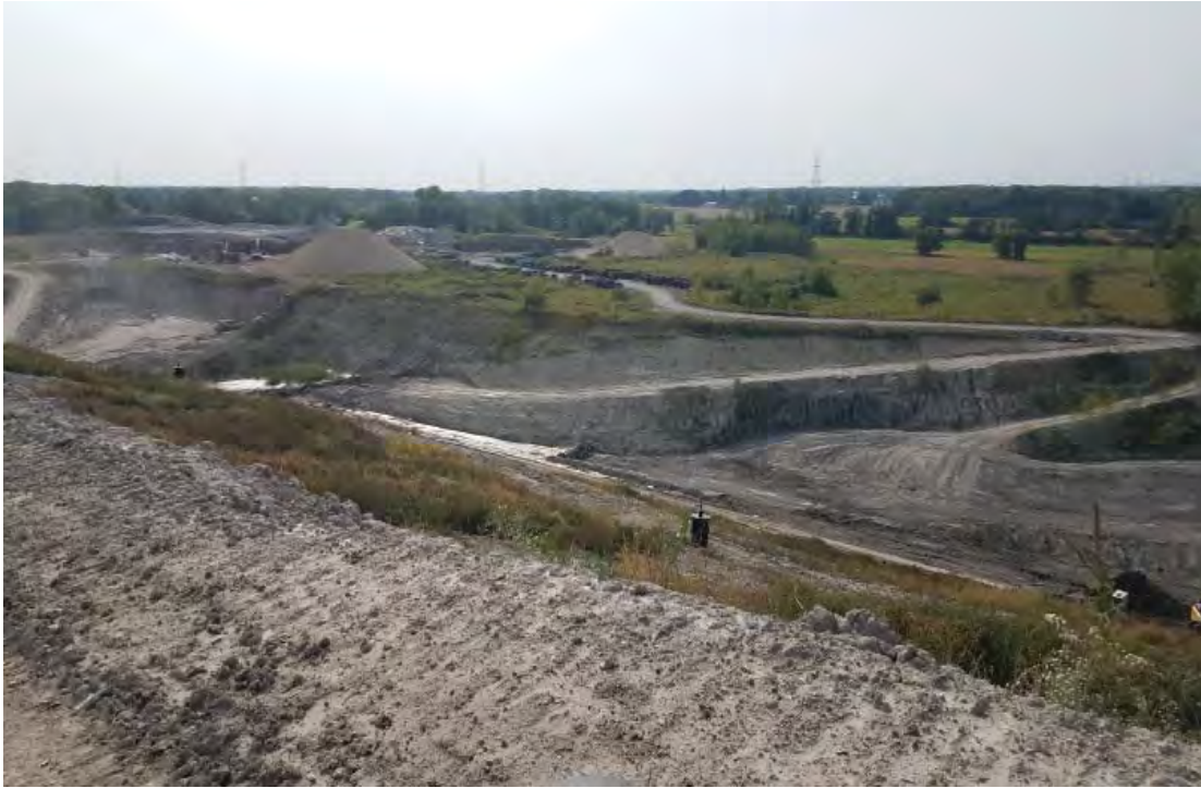
Temp sed basin, clean and dry
