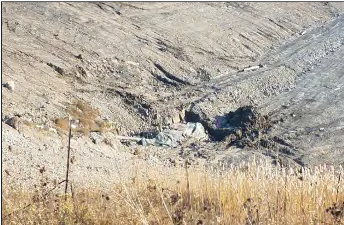
Restored sump at base of Phase 7 Slope
