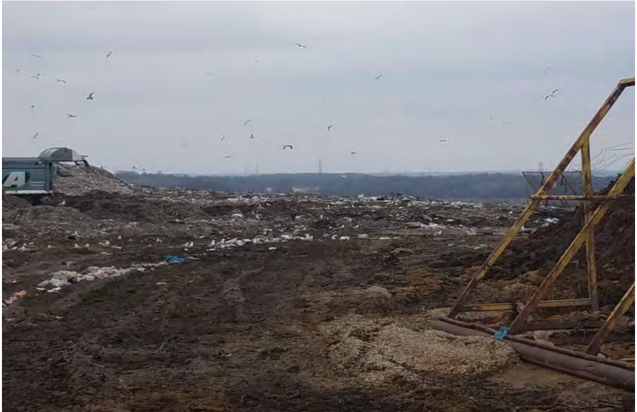
West edge of Phase 7 South viewed from the North
