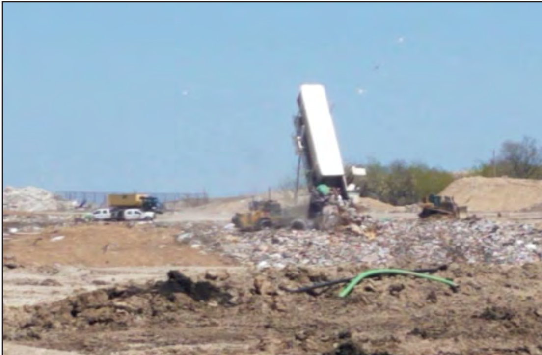
Tipper at South end of North Expansion West (NEW) over junction of Phase 1 & 2
