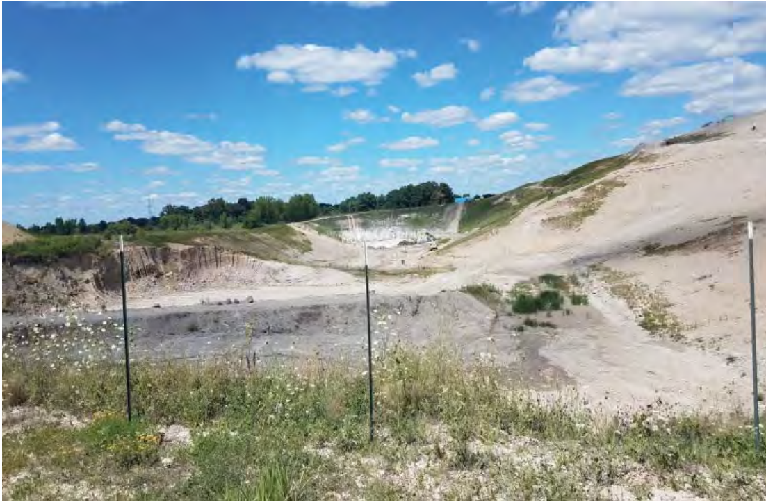
Temp Sed Basin viewed from South
