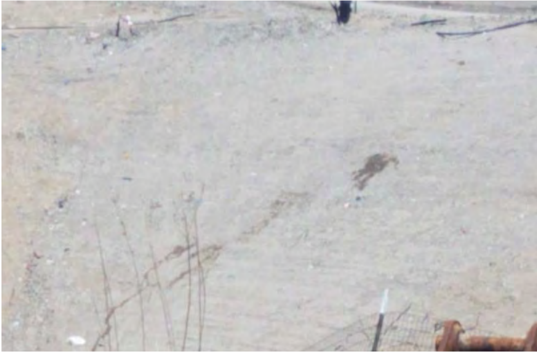
Small seeps on West slope of Phase 7
