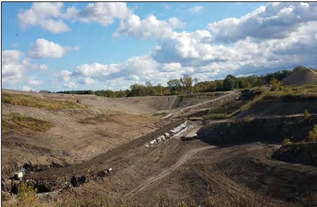
Temp sed basin, rain flap of Phase 7 exposed for repairs, awaiting scheduling of liner crew
