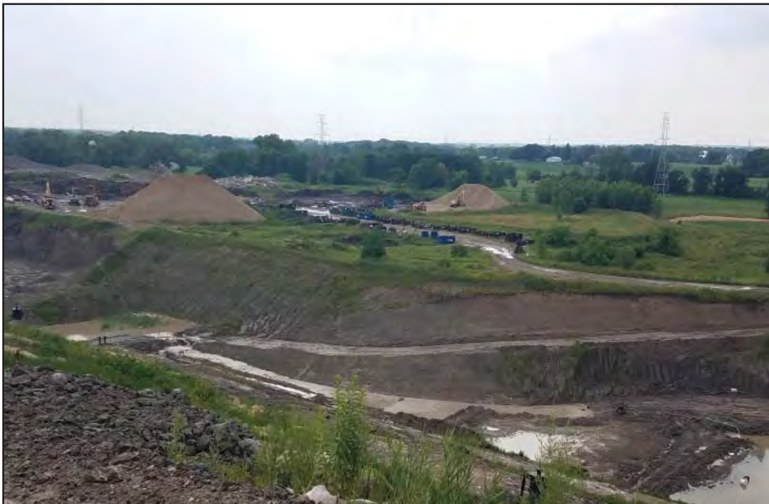
Temp sed basin laid out, prepped for leachate removal and dredging
