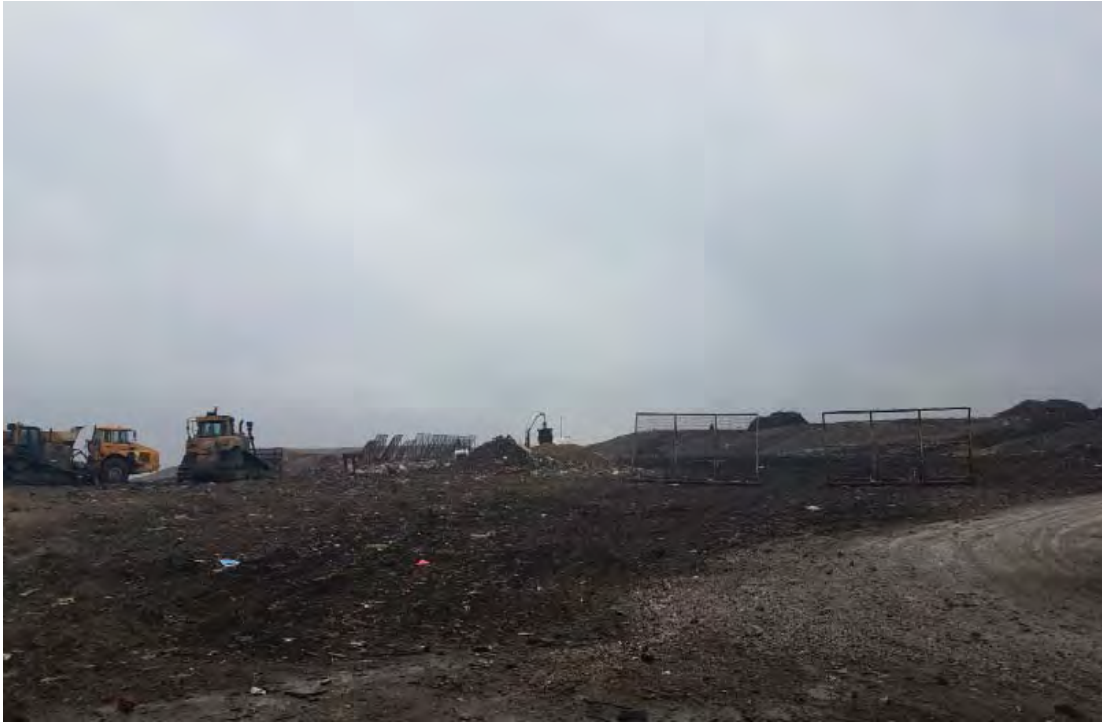
View across Phase 7
