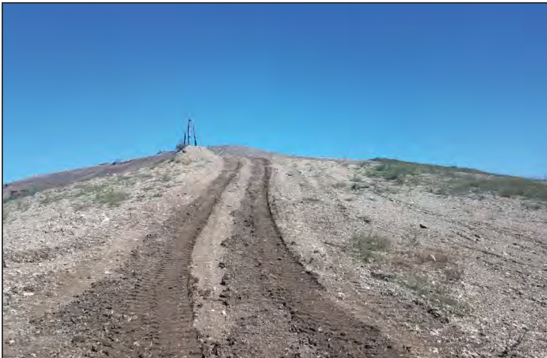
Damage to slope at Southwest corner of Phase 7 South by repeat travel of bull dozer
