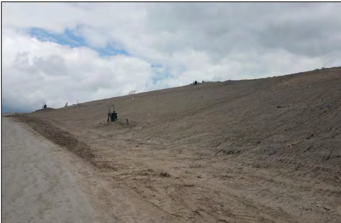
Access road headed North, potential area of odor release and where the most odors are encountered
