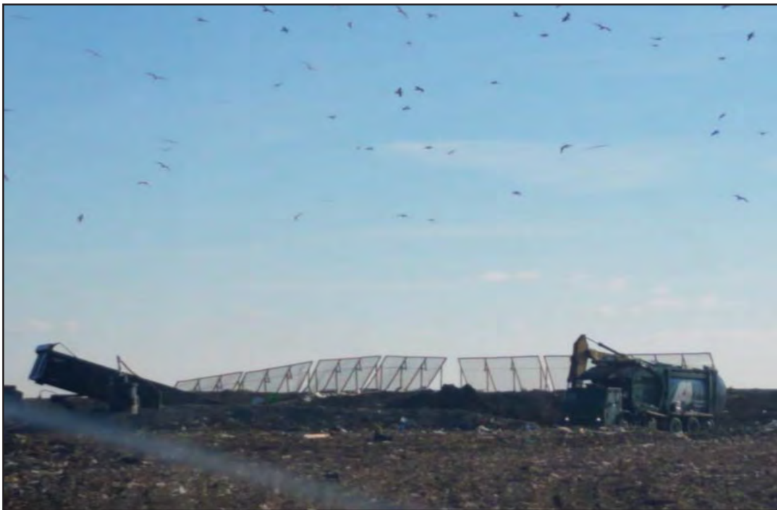
Mobile fences relocated to catch litter and prevent travel off the active area
