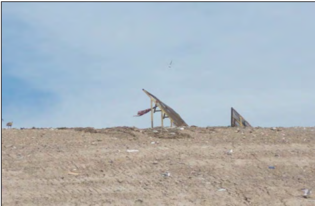
Top of slope, Phase 7, some stockpiling placed for cover
