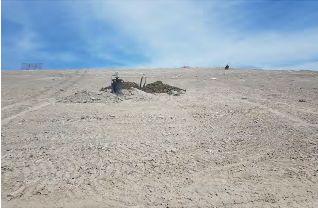
South slope of Phase 7 South, well being backfilled after placement of bentonite
