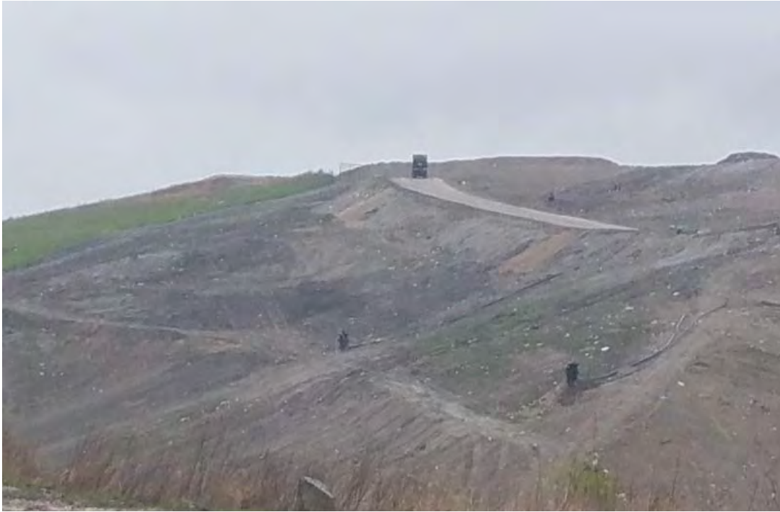
West slopes restored after trenching
