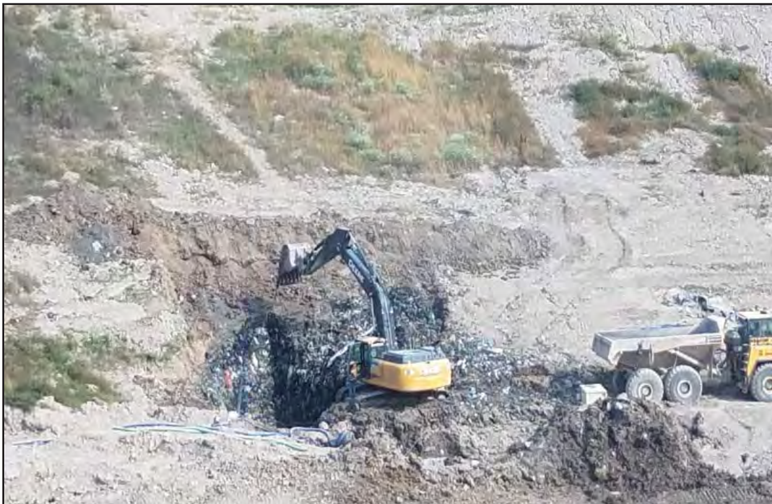
Excavation to sump, materials being placed in working face and covered
