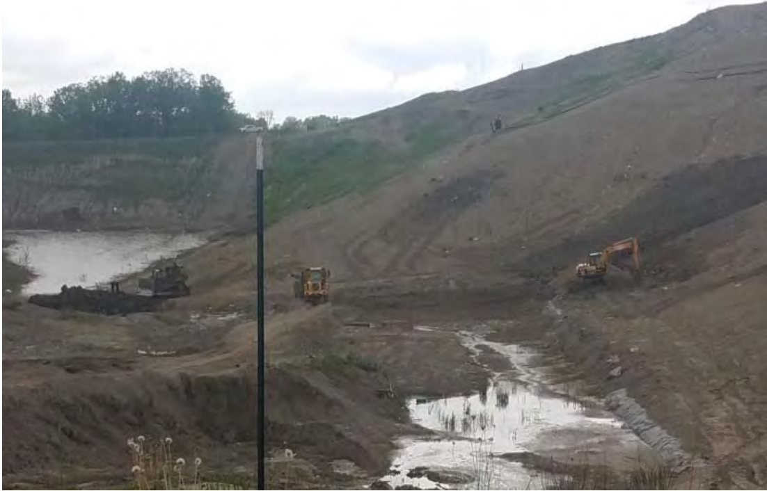
8. Temp Sed Basin Forebay, some cleaning appears to have been done for silt
