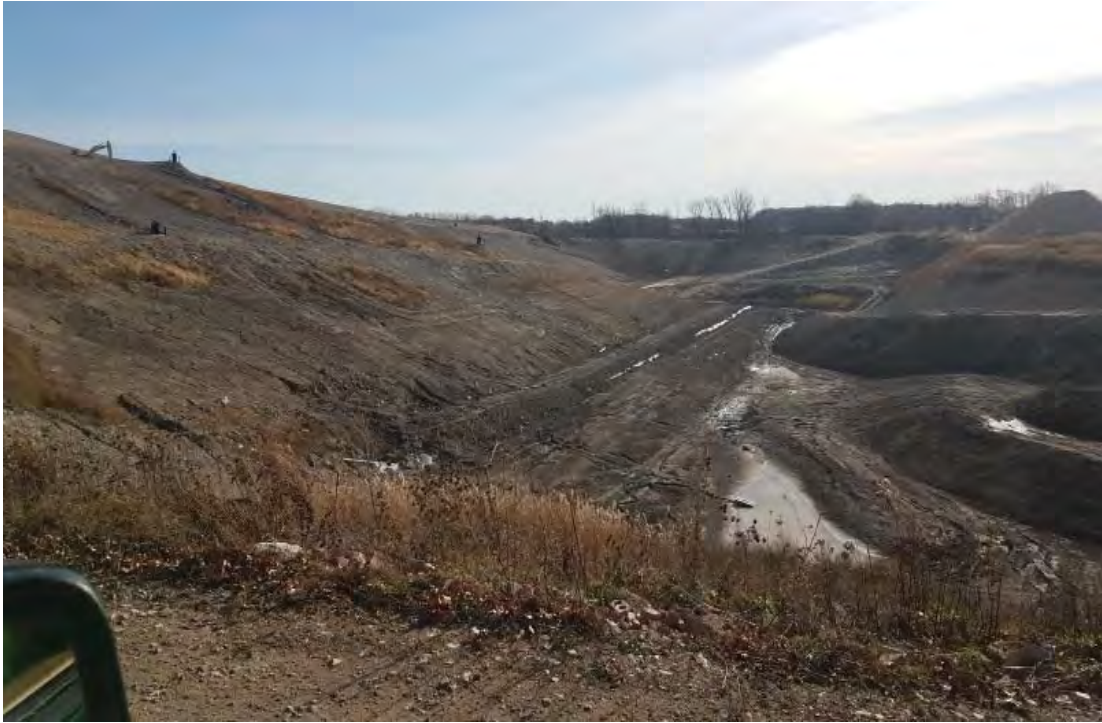
West slope of Phase 7, repaired rain flap and access road
