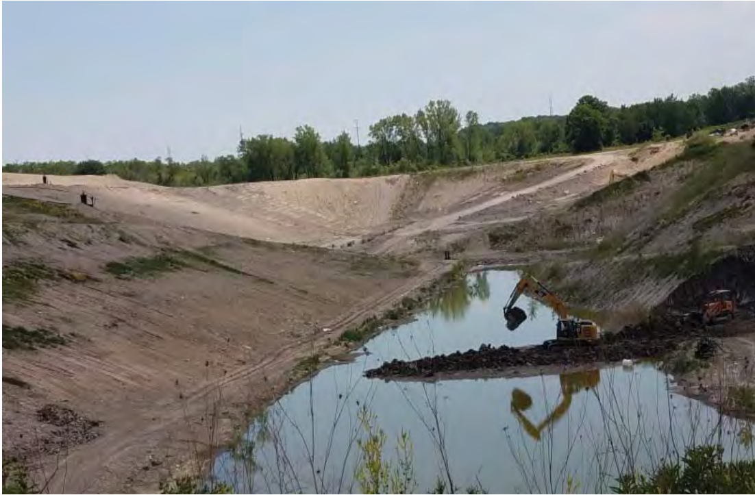
Contractor separating temp sed basin to aid in pumping and future flow control
