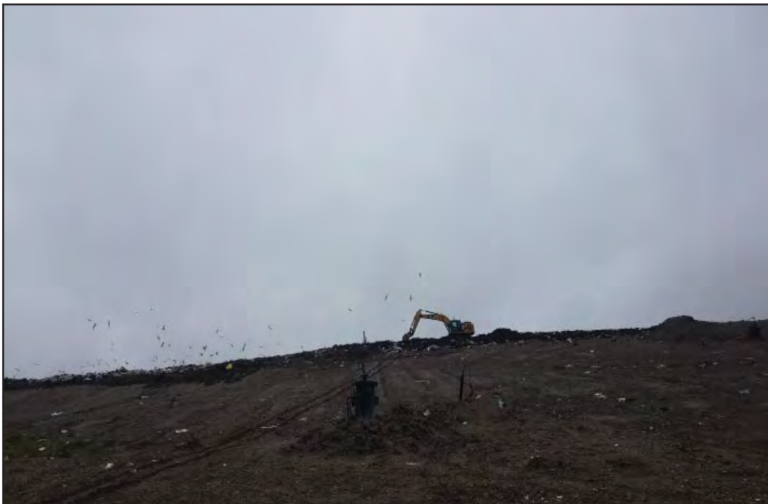
West slope of Phase 7 South, recently backdragged; area around access road where most odors are discovered
