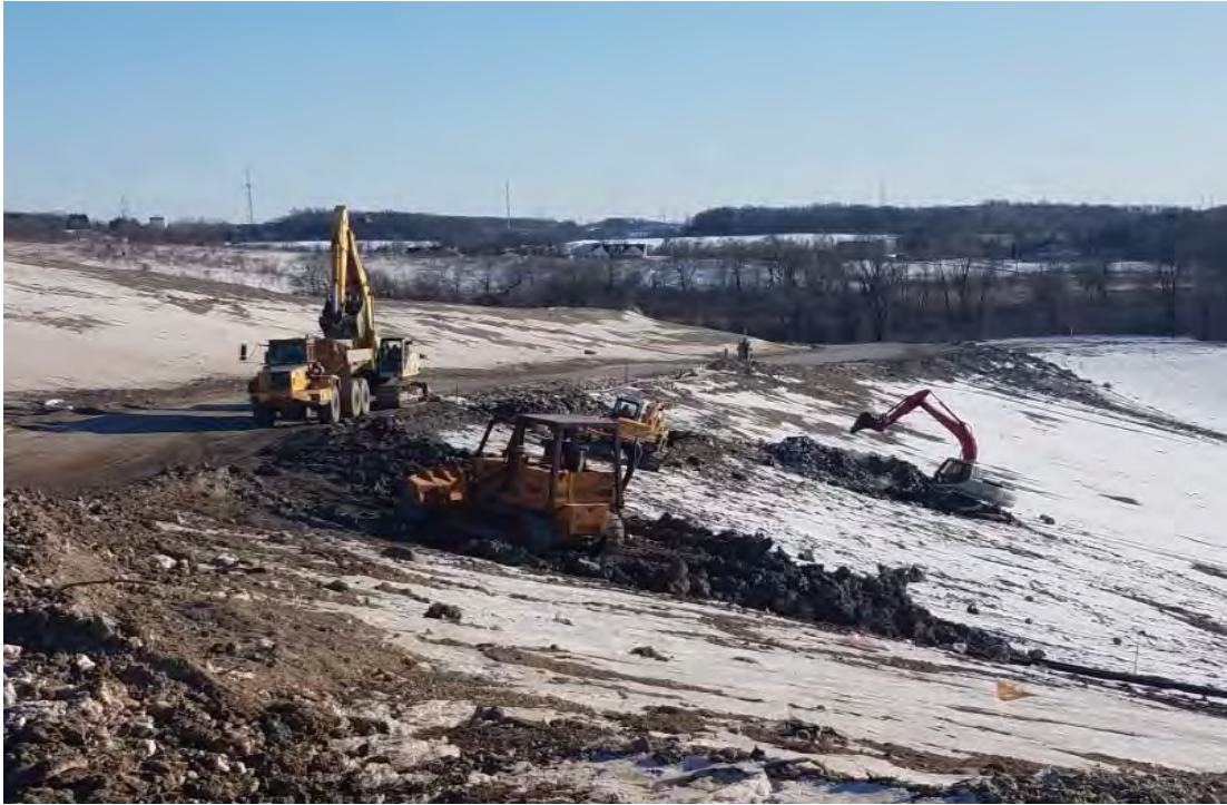
Seep repair and horizontal gas extraction trench construction on West slope of Phase 7; West of access road
