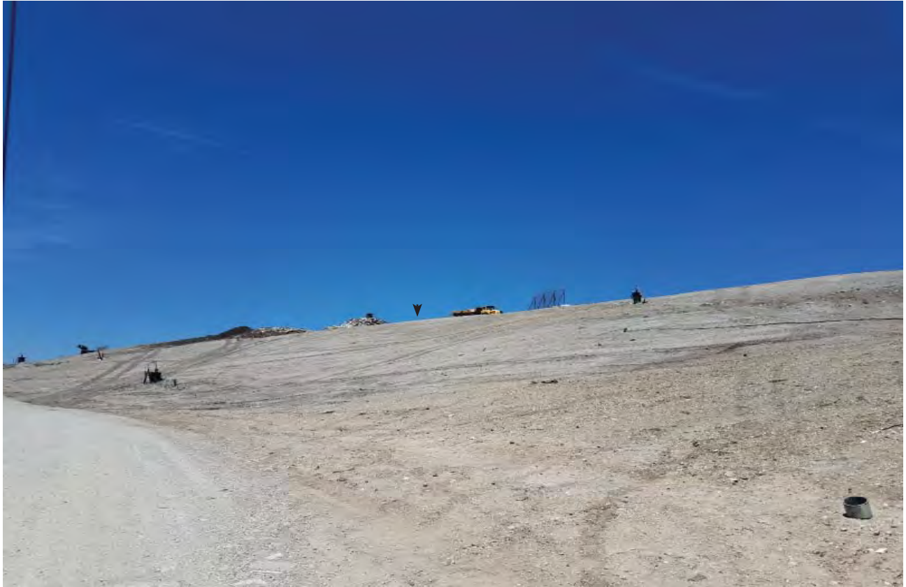
West slope on approach to working face in Phase 7
