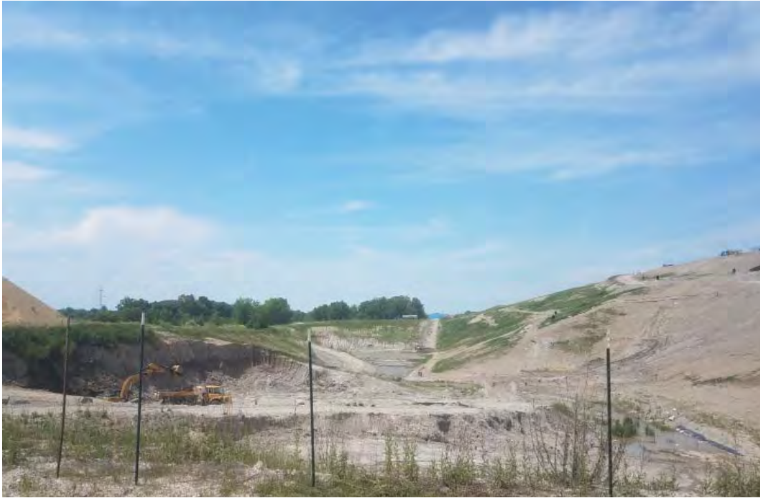
North end of Phase 7 viewed from West, East slopes in good repair
