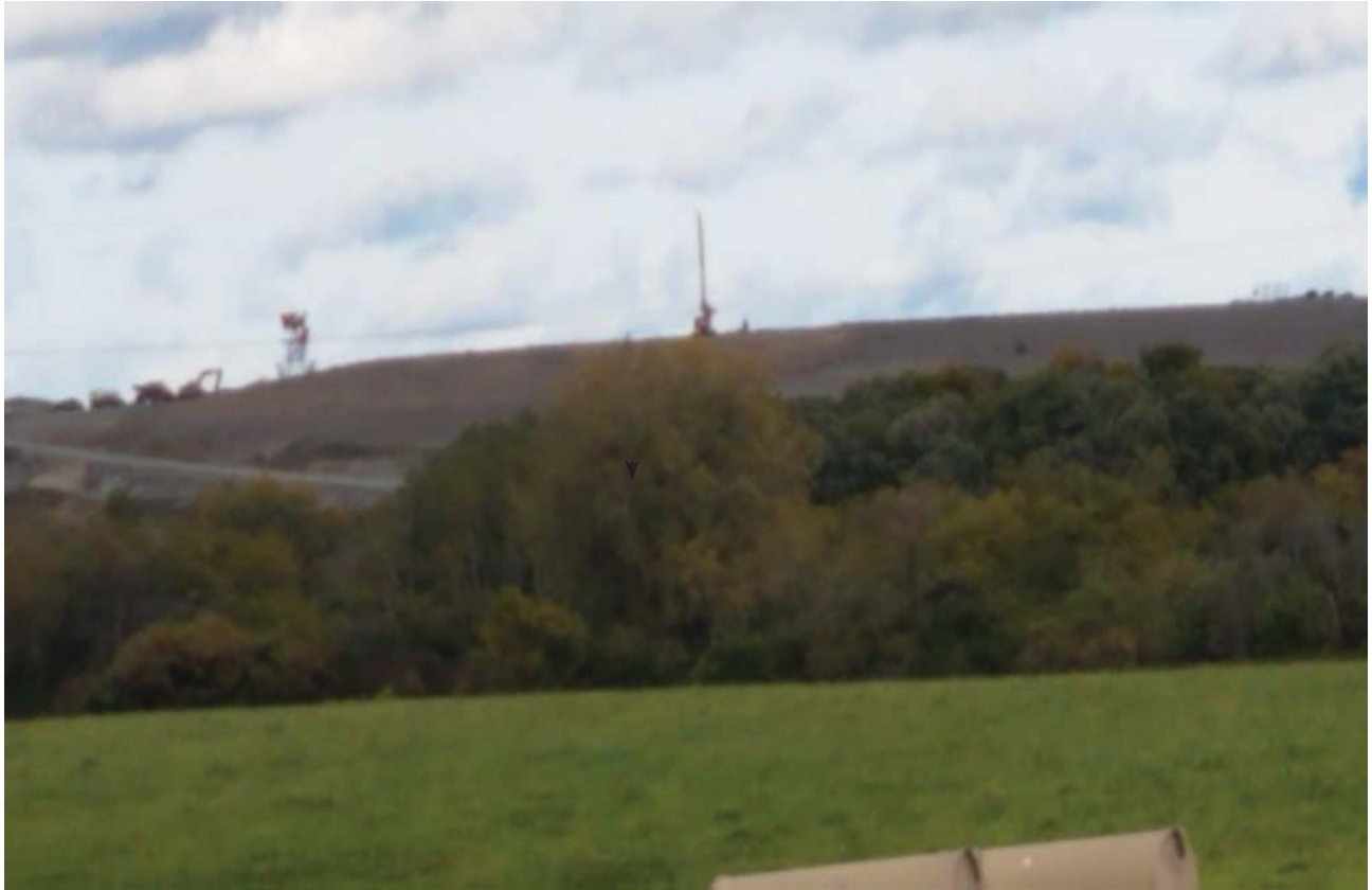
Rig in center of Phase 7 placing well.
