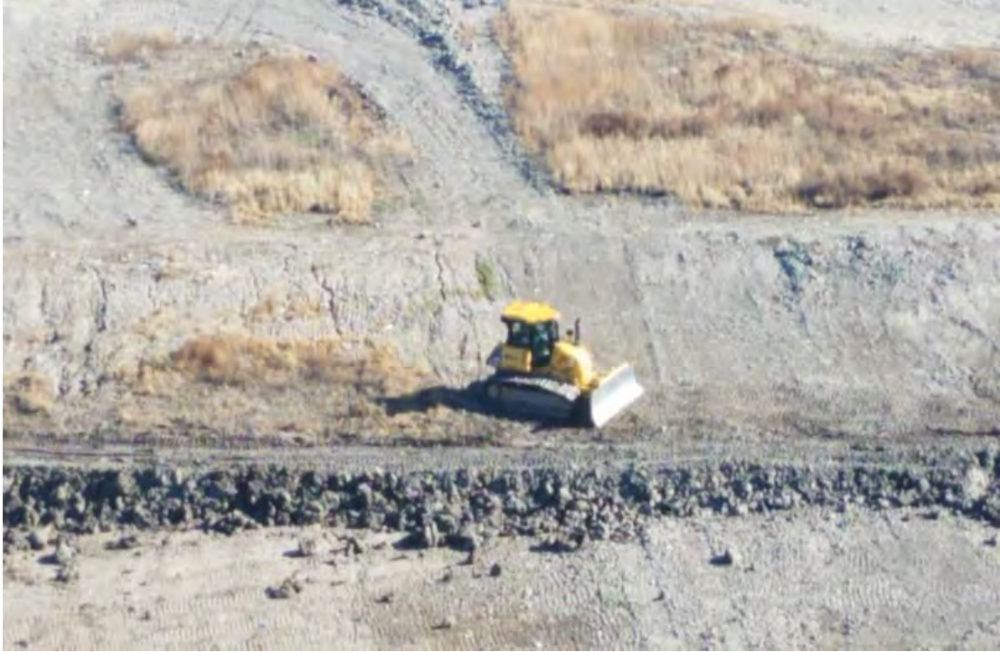
Berm development on West Slope of Phase 7
