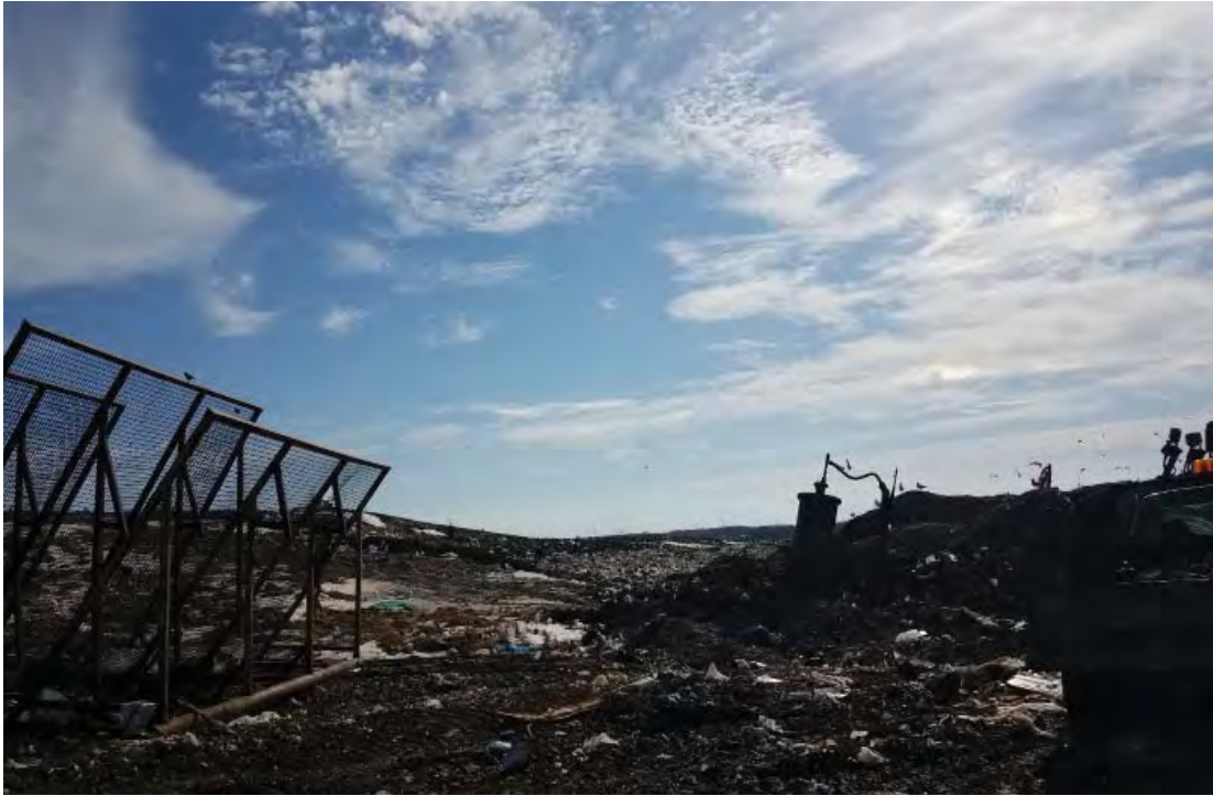
Eastern edge of Phase 7 South
