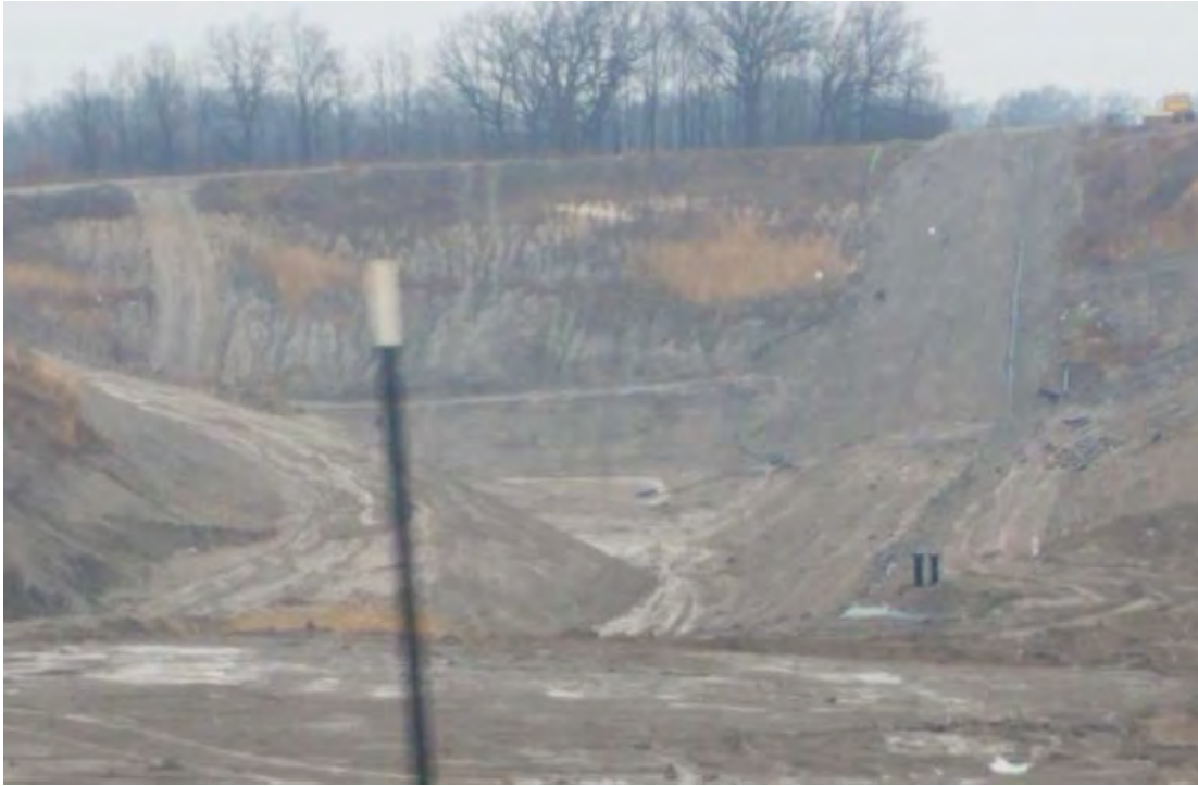
Temp Sed Basin viewed from the South
