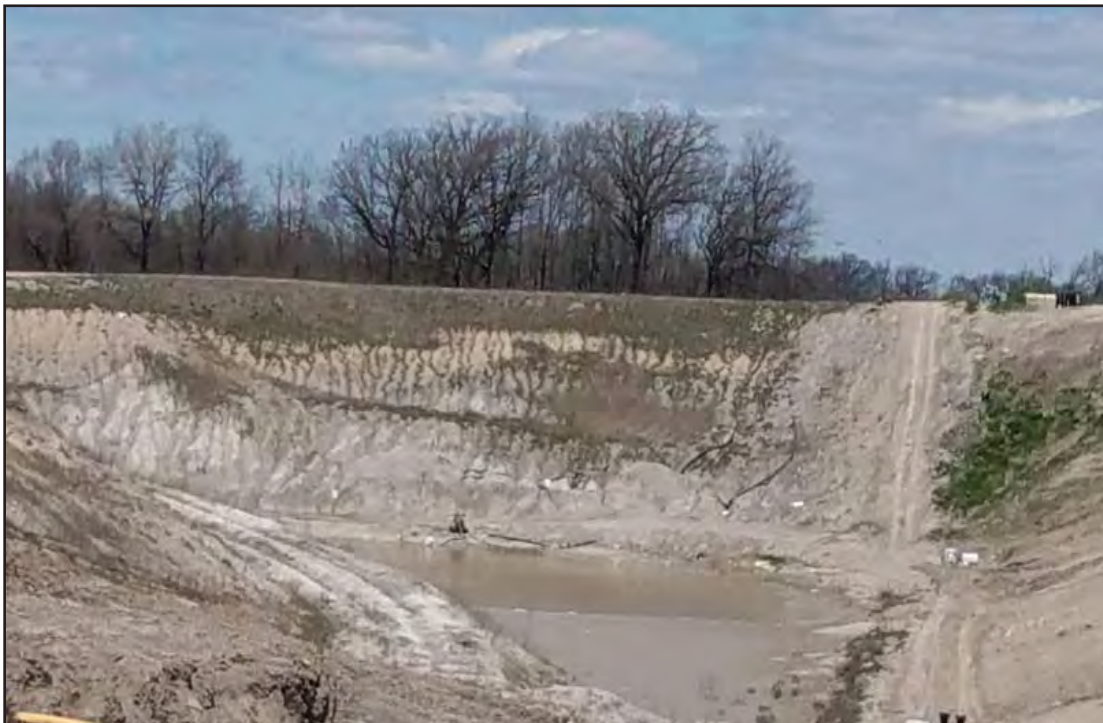
Temp. Sed Pond well pumped
