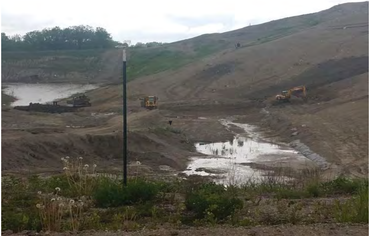
1. Temp sed basin forebay
