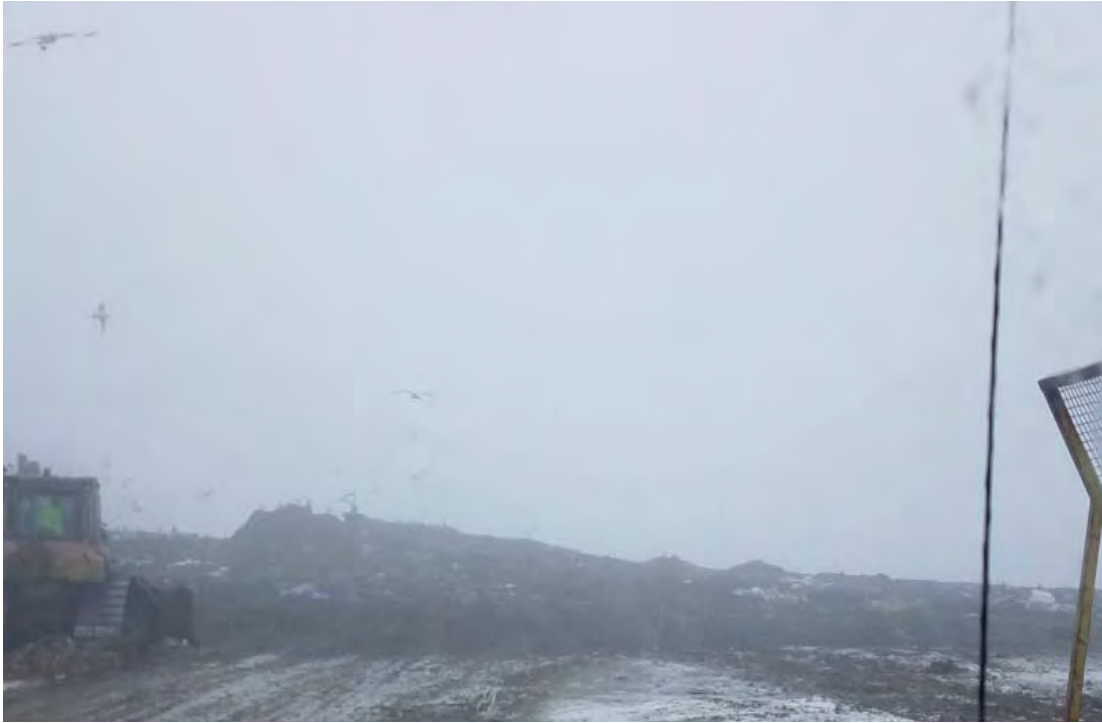
Mixed alternative daily cover (ADC) stockpiled for future cover
