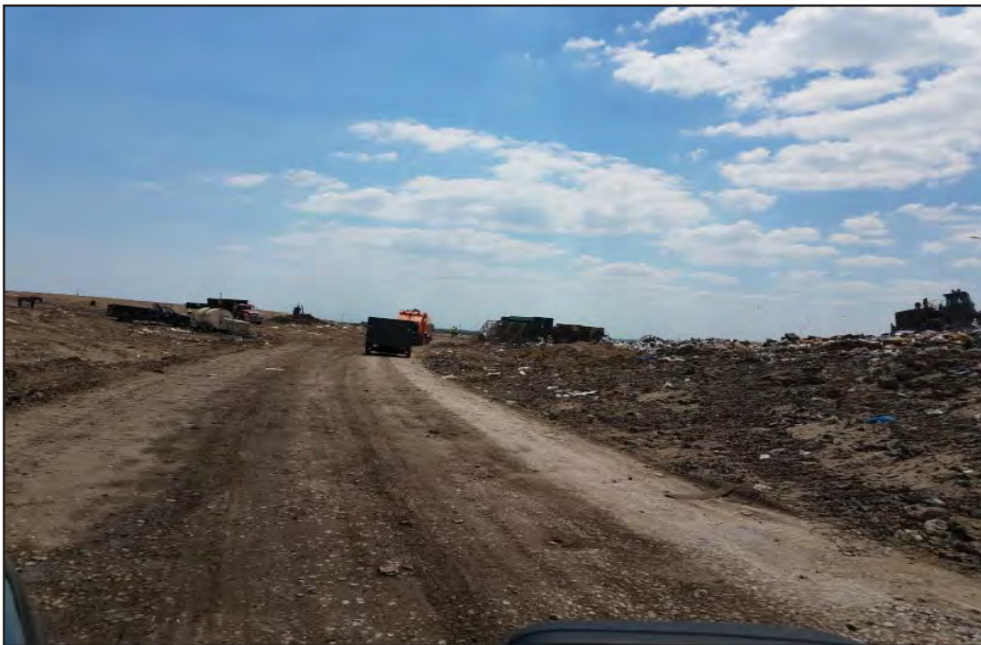
Access road from Phase 7 North to Phase 7 South, viewed from North
