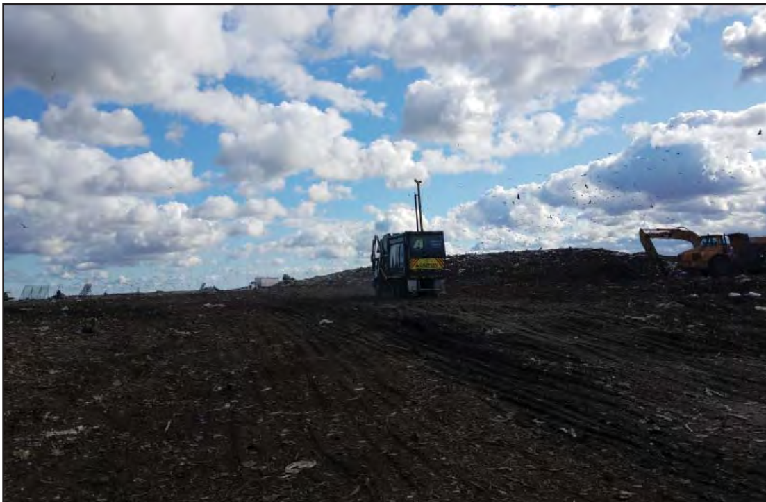
Phase 7 South, view from North, lift on West (right) side creating a windbreak
