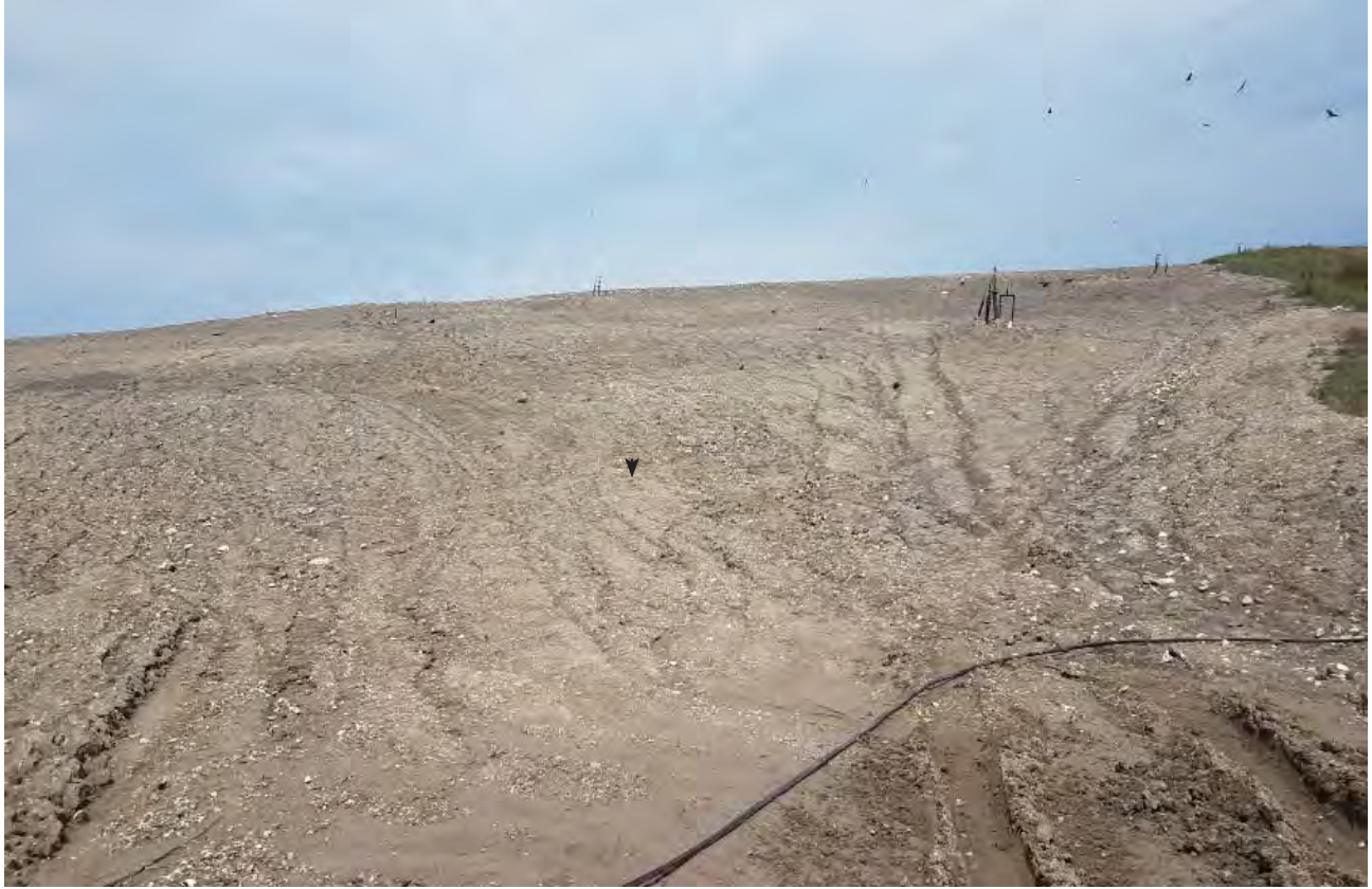
South slope of Phase 7 South, erosion developing
