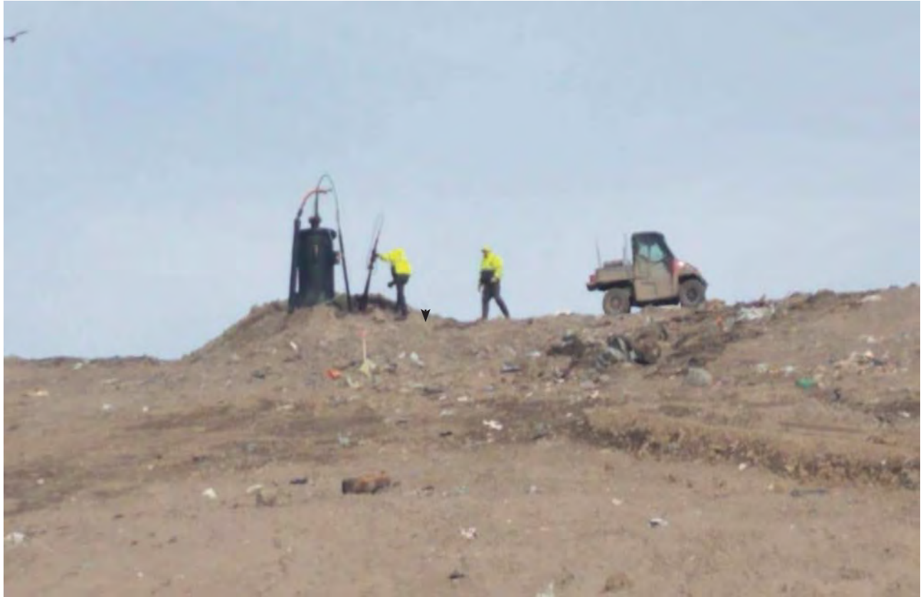
Gas techs adjusting connections at new well and trench well connections
