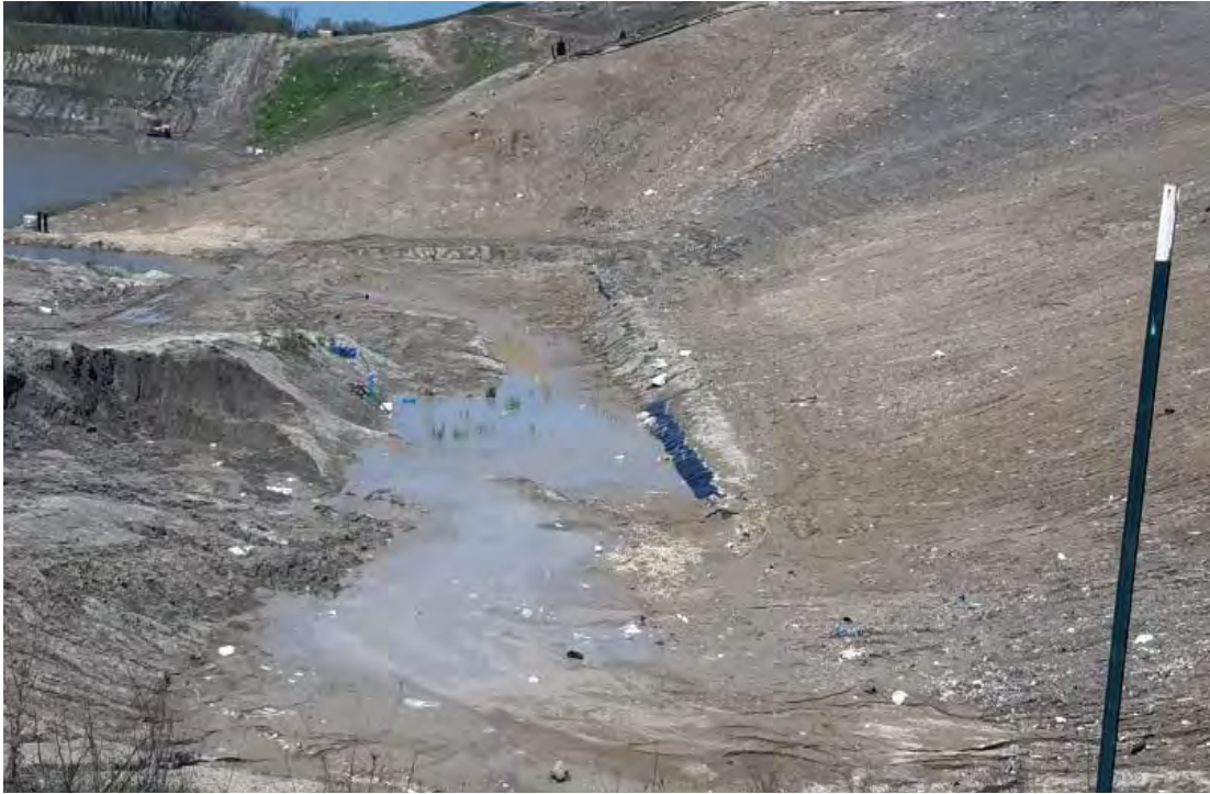
Siltation in South end of the Temp Sed basin, silt is higher than rain flap of Phase 7 South
