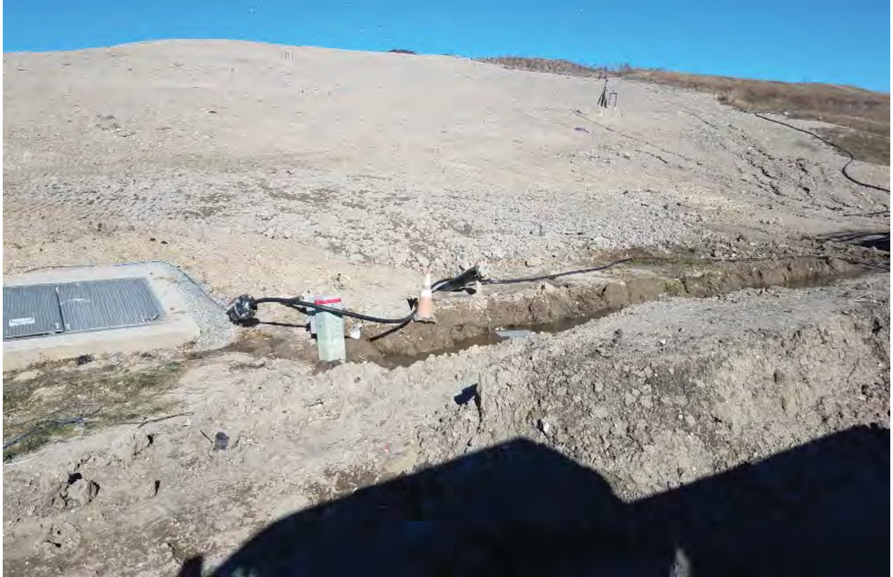
Leachate collection prior to filter tank and tanker hauling
