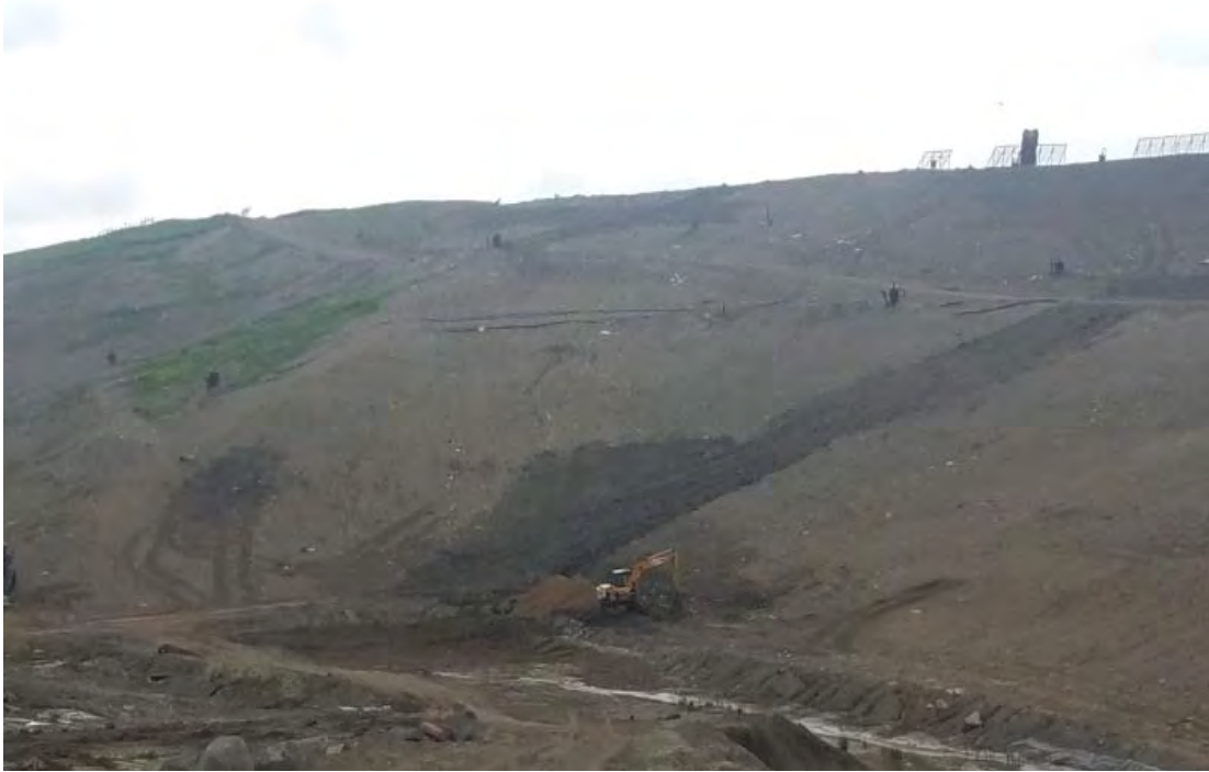
6. Excavator performing slope repairs for Emissions and/or seeps
