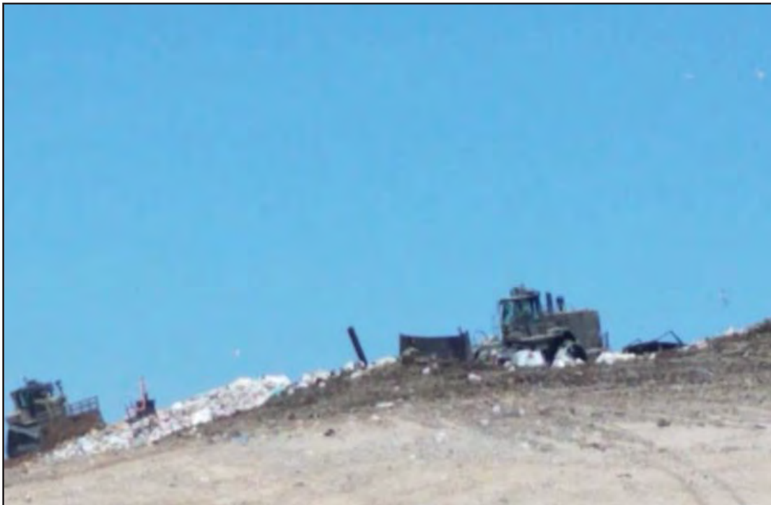
Compactor active at Working Face
