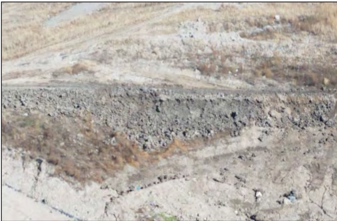
Berm development on West Slope of Phase 7
