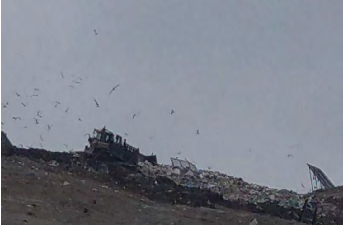
Dozer placing waste for compaction on outboard slope
