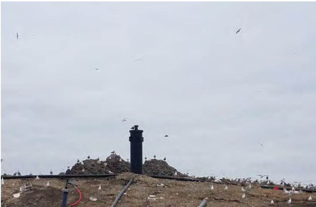
New gas well on top of Phase 5
