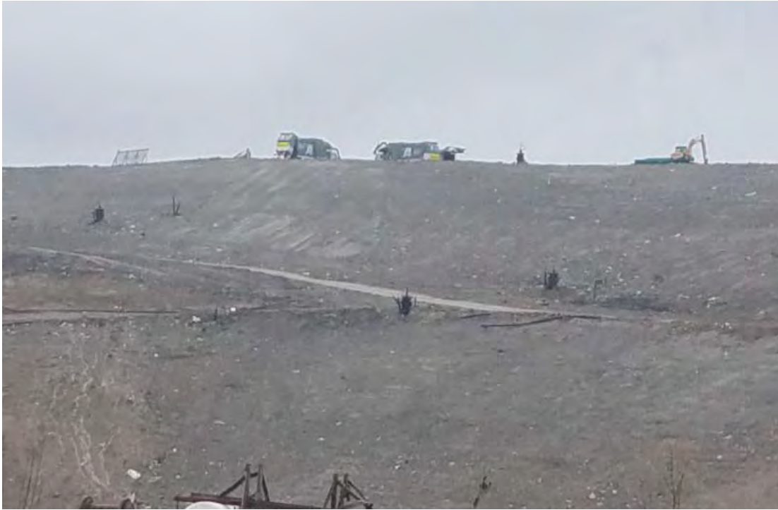
West slopes restored after trenching
