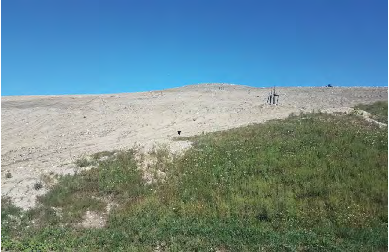
Top of Phase 7 South slope, at Phase 6 junction
