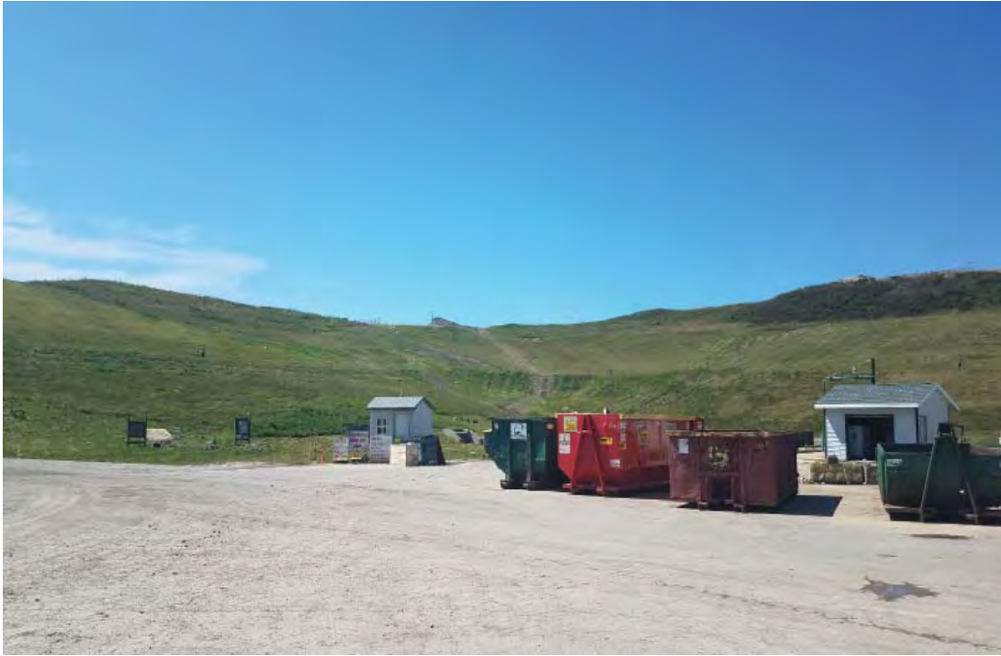
North slope of Phase 4, some wear and tear from vehicle traffic
