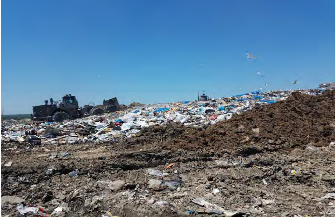
Working face with daily cover stockpiled about edges
