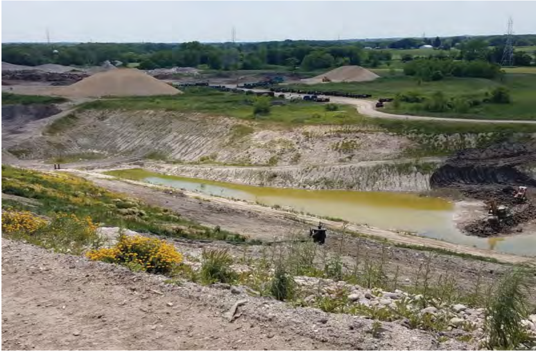
South end of temp sed basin
