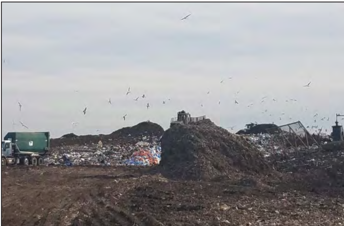
Working face at South end of Phase 7, viewed from the North. Abundance of autofluff ADC stockpiled
