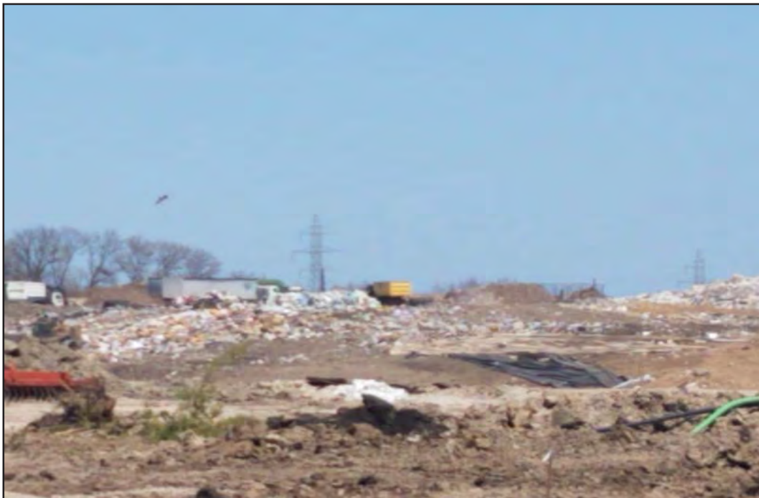
Waste being spread into Phase 2
