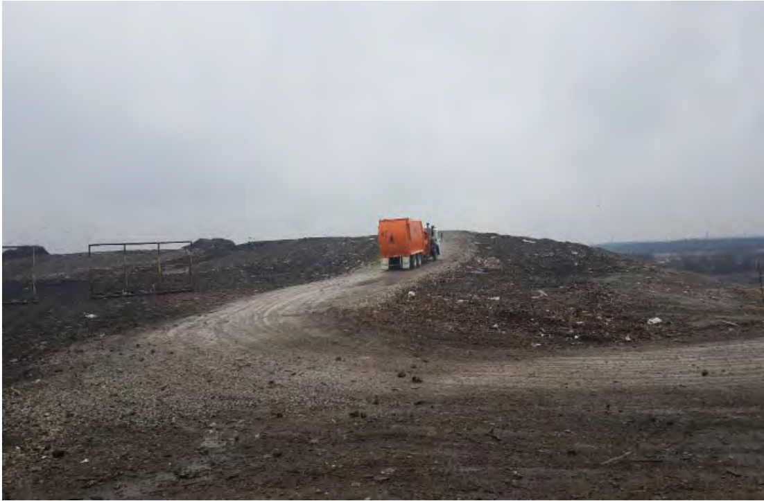
Access road extended another lift
