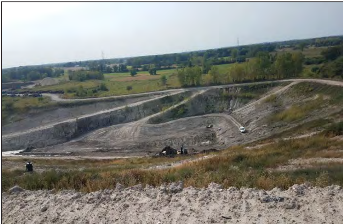
Temp sed basin, clean and dry
