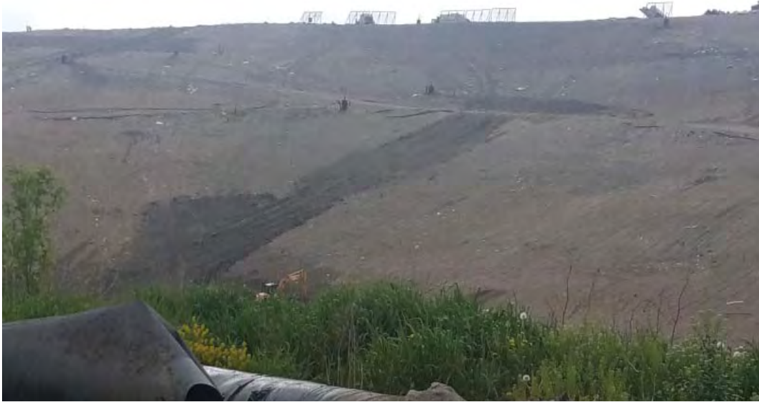
2. West slope of Phase 7 South, seep repairs by placement of soil cover
