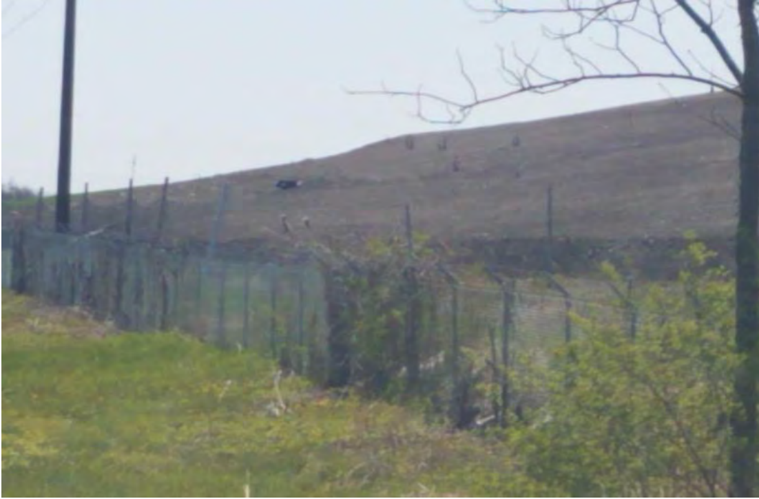
Cap development for Clearwater Pond Expansion
