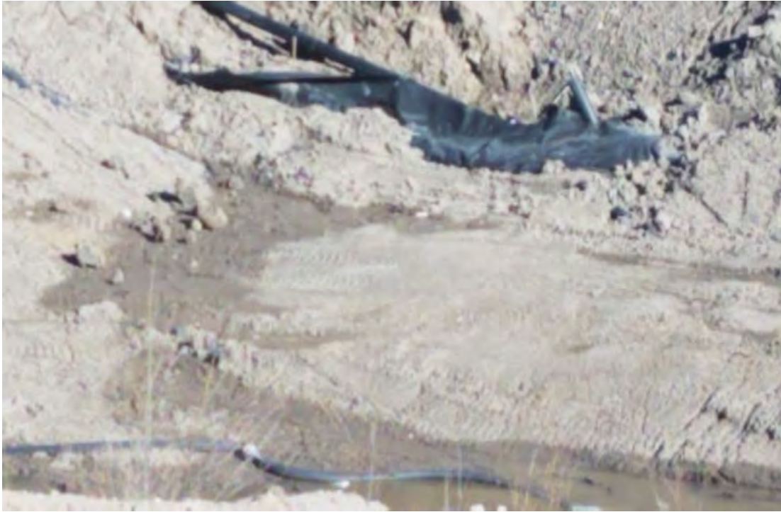
Header for leachate collection
