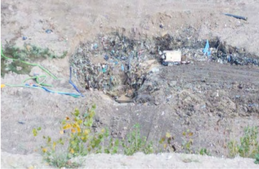
Phase 7 sump exposed by excavation
