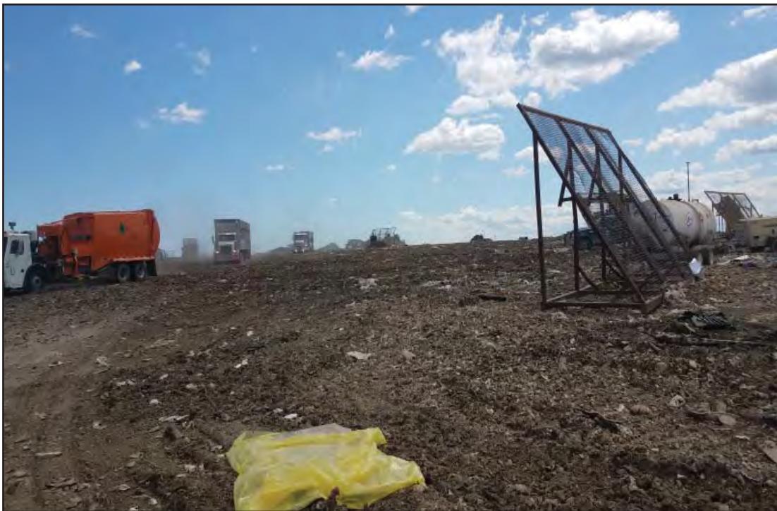
Active area viewed from North
