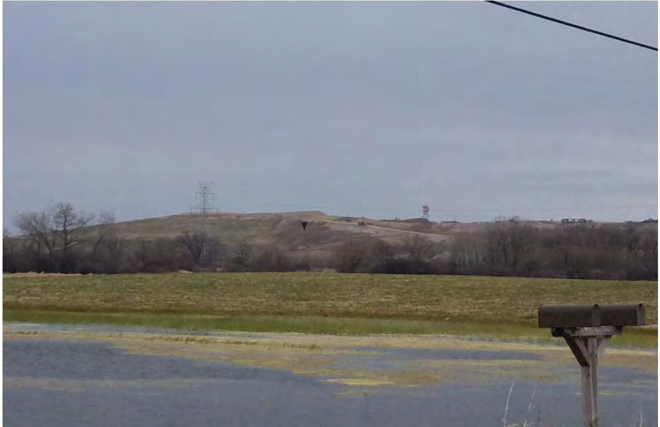
Working face viewed from Union Church Road from the South. Trenching project on South slopes blocked by trees
