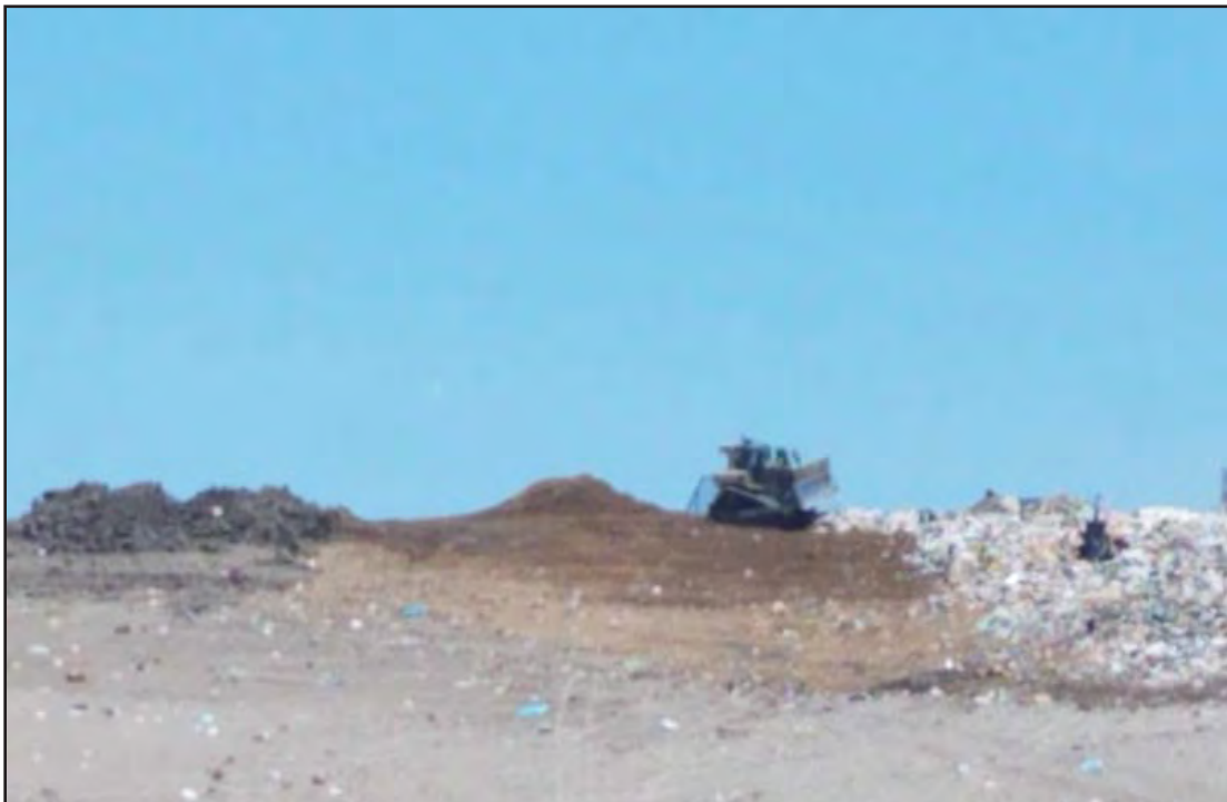
Dozer placing cover as slope elevations are reached
