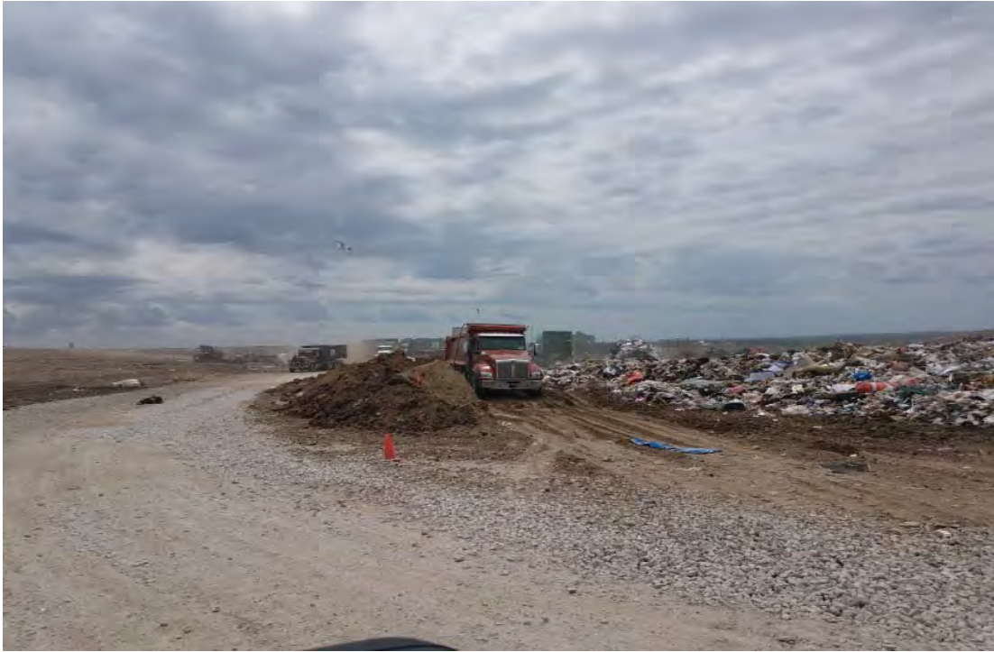
Working face in Northwest corner of Phase 7 South
