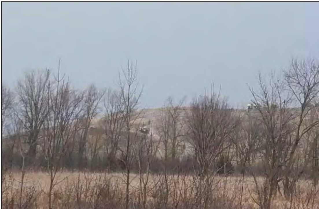
Trenching complete on West slopes
