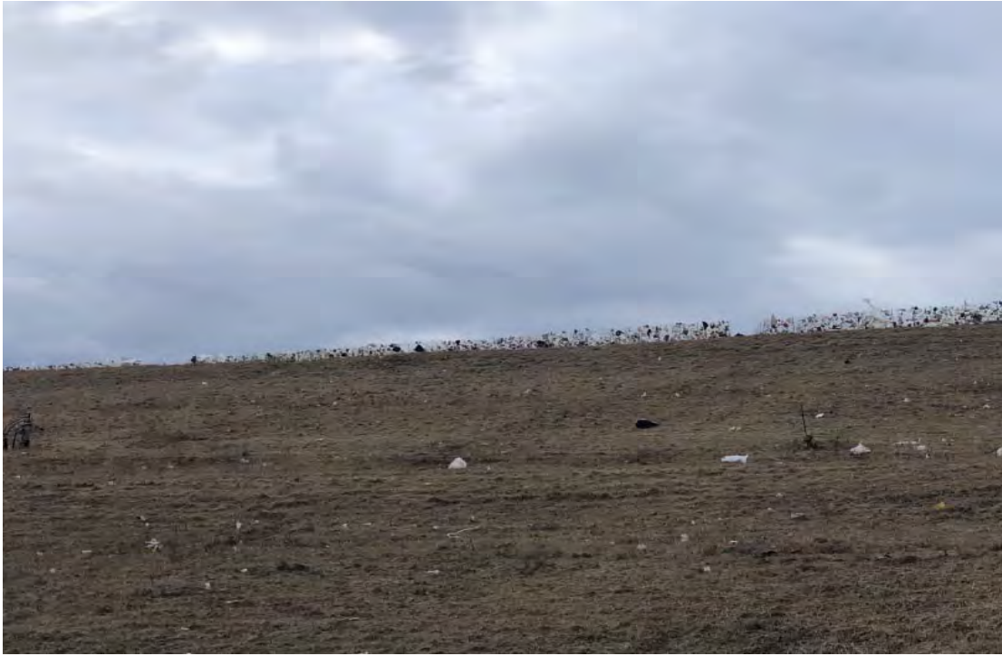
Capped slope with minor litter
