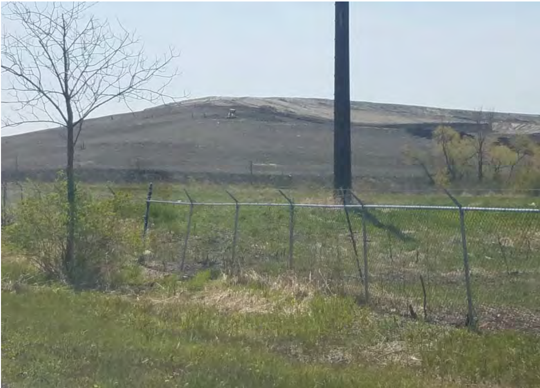
Cap development for Clearwater Pond Expansion
