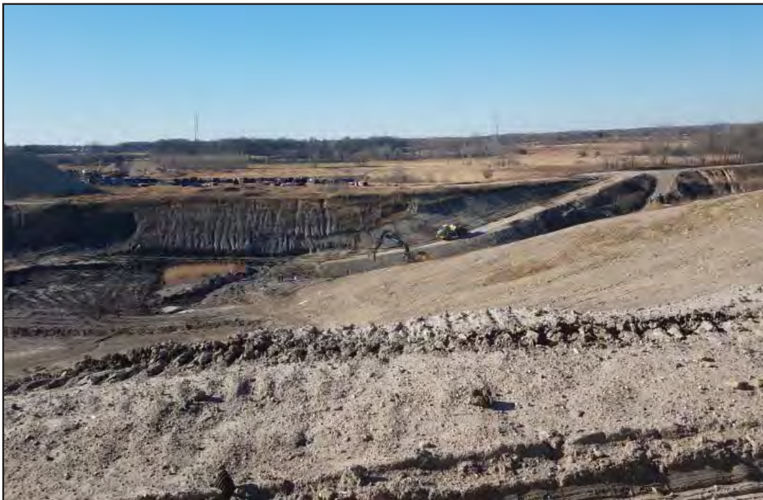
Contractor excavating future Phase 8 to provide material for construction of Phase 7 West slope berm
