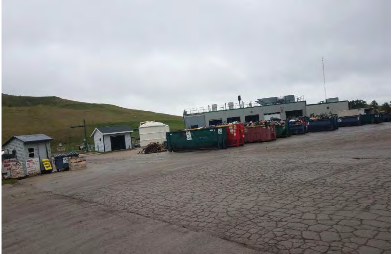
Residential Drop-off yard and gas plane
