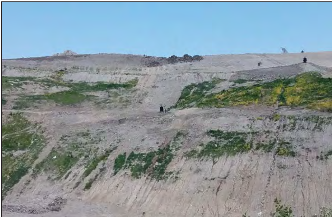
West slope of Phase 7, soils at top of slope for daily cover
