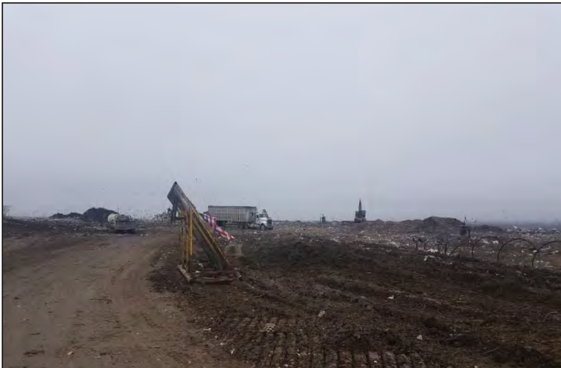
Overview of Phase 7 South
