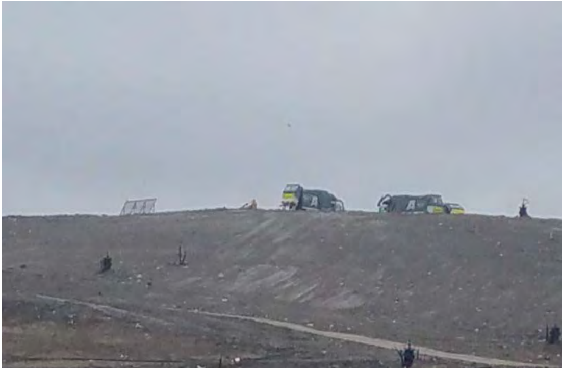
Phase 7 viewed from the West
