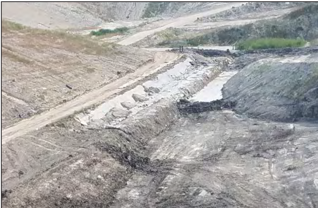
Exposed rainflap, awaiting liner crew for repairs.
