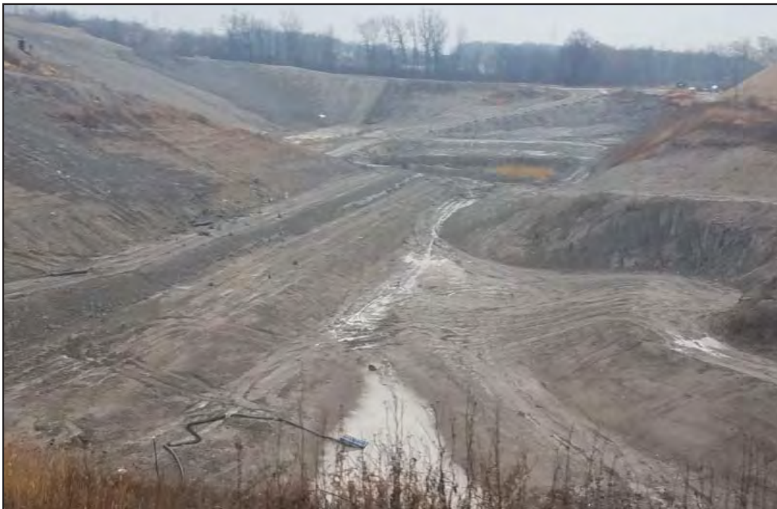
Temp sed basin viewed from the North
