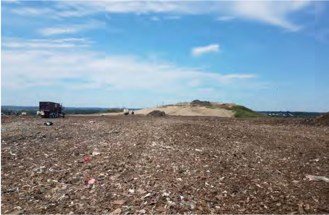
Phase 7 viewed from the North
