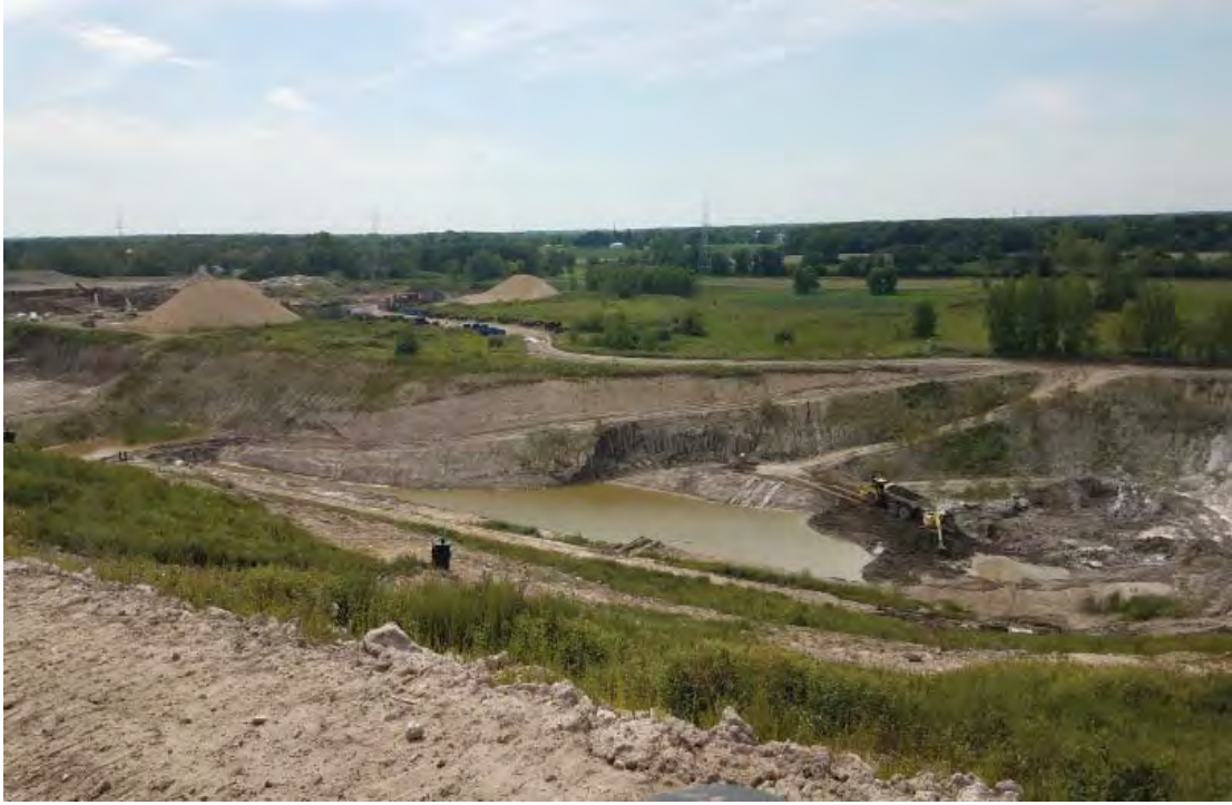
Overview of Temp Sed Basin, mostly cleared and cleaned
