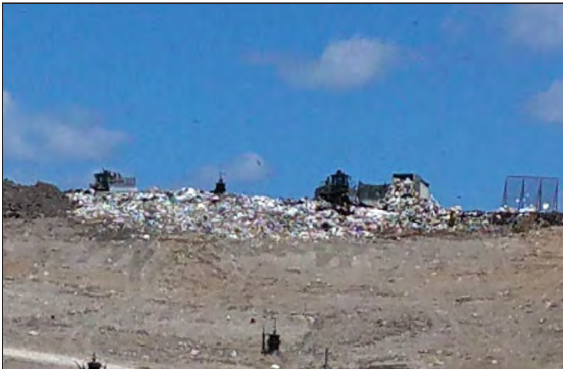
Working face at top of slope
