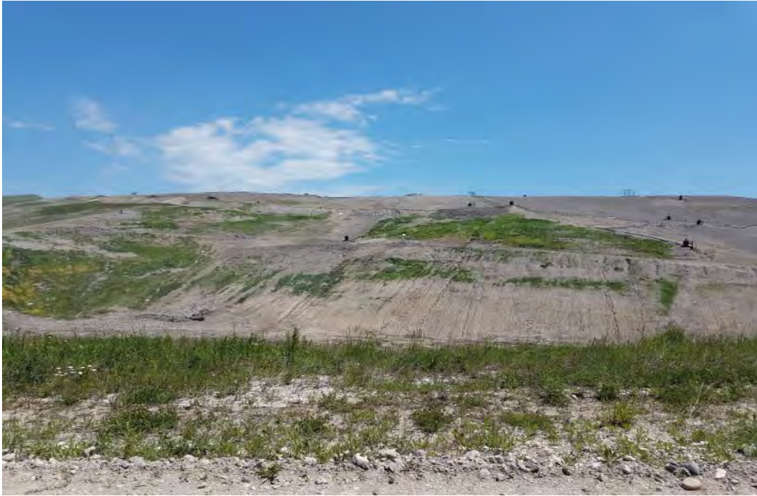
West slope of Phase 7 North, several seep repairs were done in last two weeks
