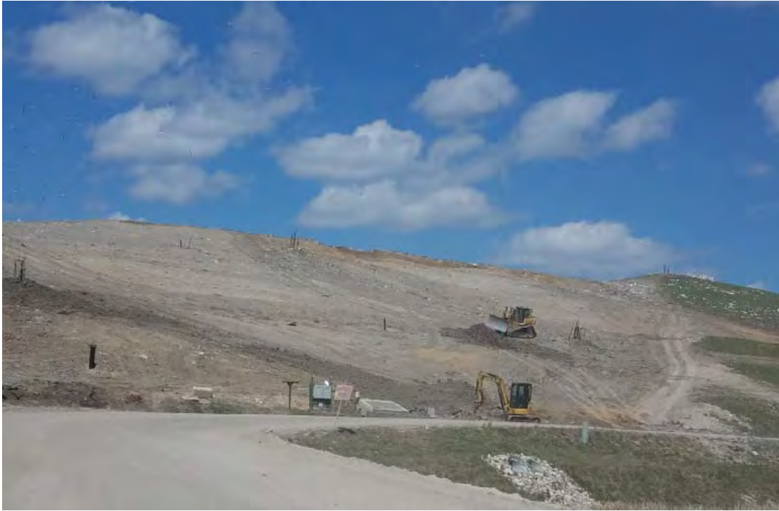
South slope of Phase 7 South, contractor repairing slope after trenching
