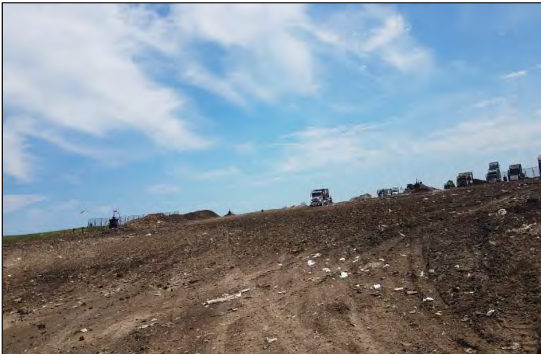
Phase 7 viewed from the North
