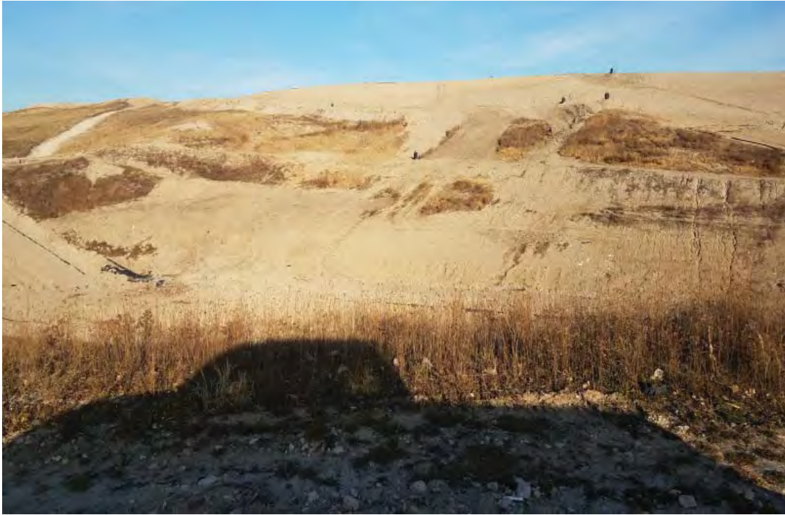
Rainflap exposed and repair at Northwest corner of Phase 7
