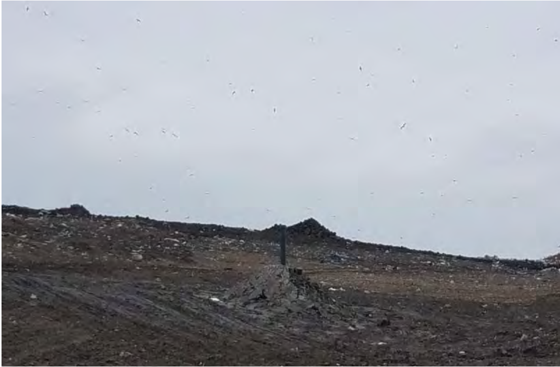
New well installed on Phase 7 South, South slope
