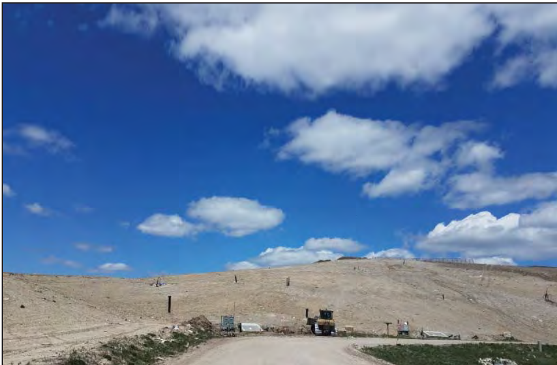
Dozer grading soils excavated for pipe repairs
