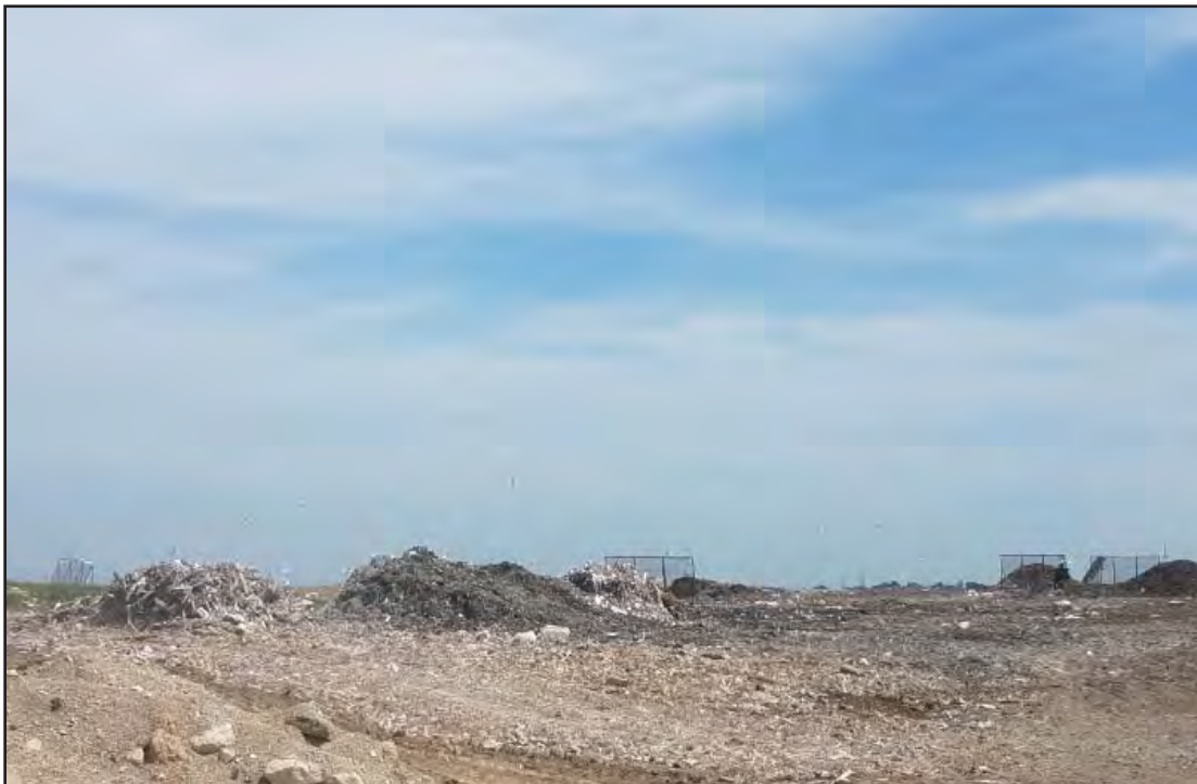
Phase 7 view to the South
