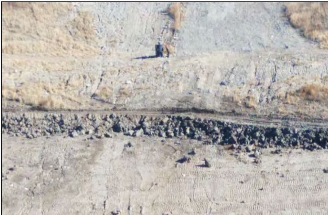
Berm development on West Slope of Phase 7
