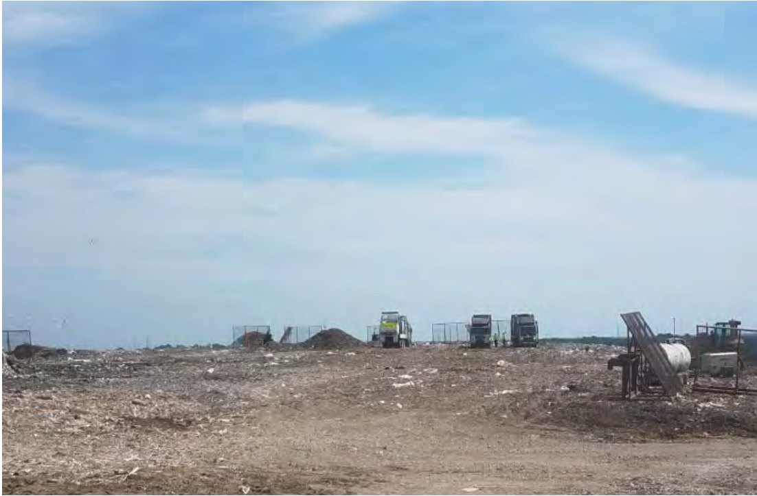
New lift moving West across Phase 7
