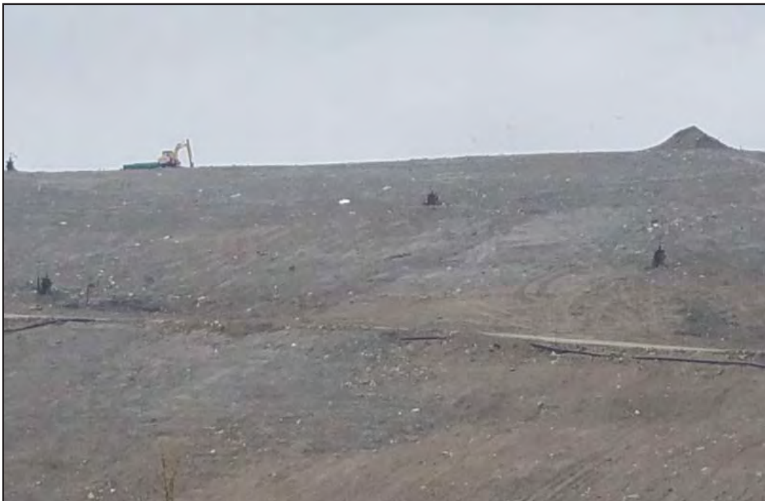
No evidence of seeps on West slope
