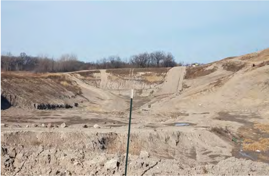
Temp Sed Basin viewed from the South
