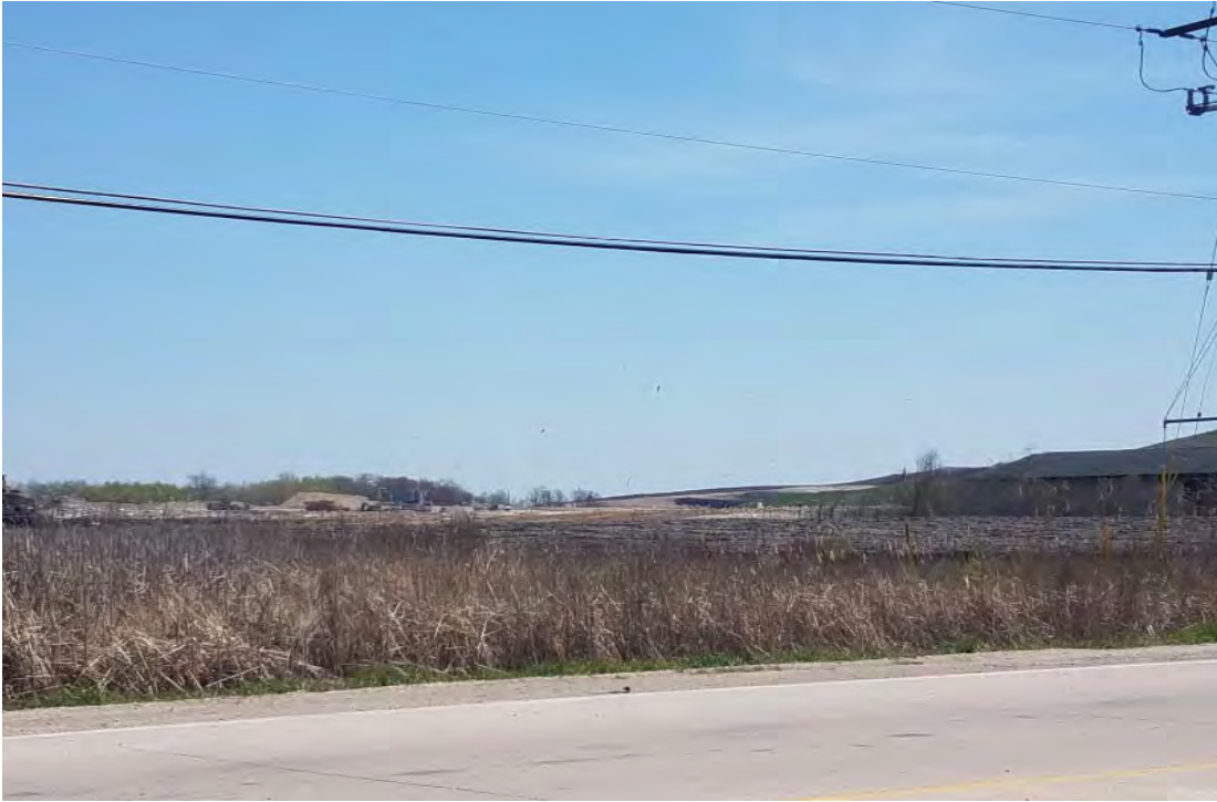
Berm construction with excavated soils from North Expansion West (NEW), Phase 2B
