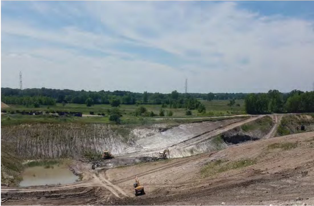
View across temp sed basin, East to West
