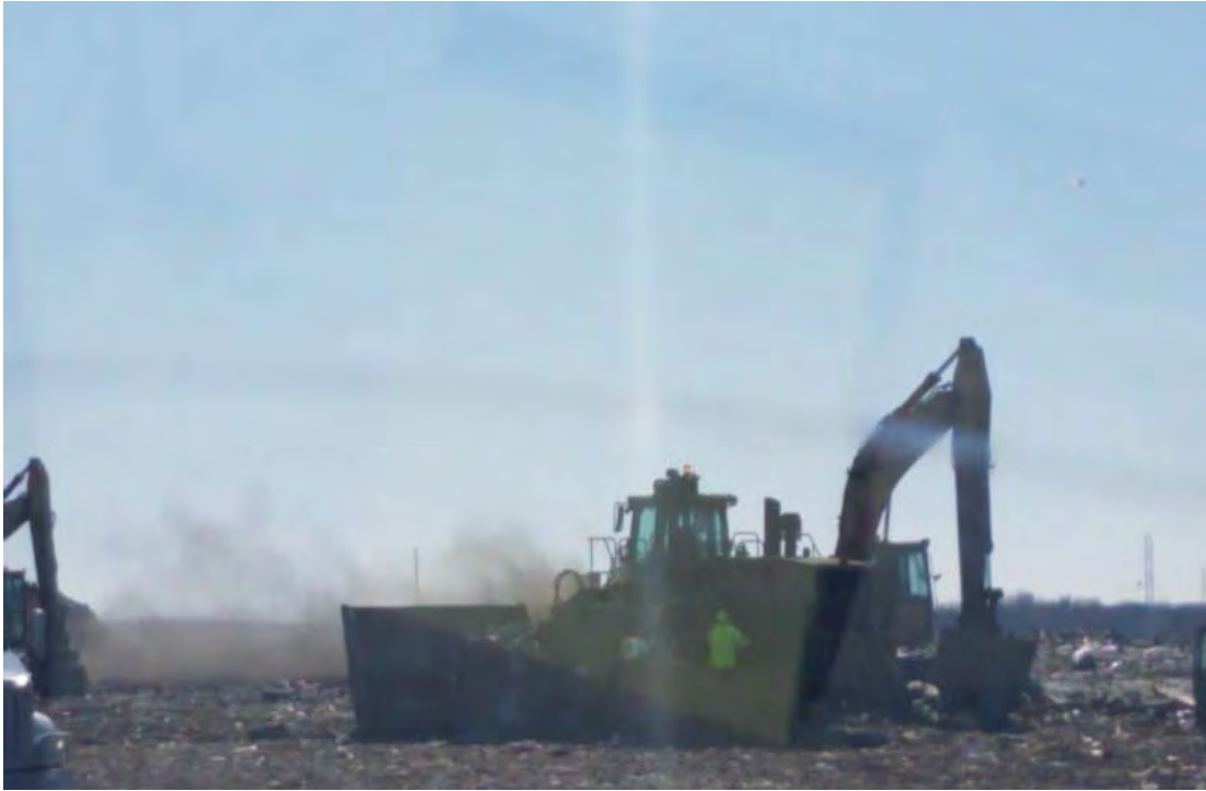
Compactor being cleaned out after dusty loads
