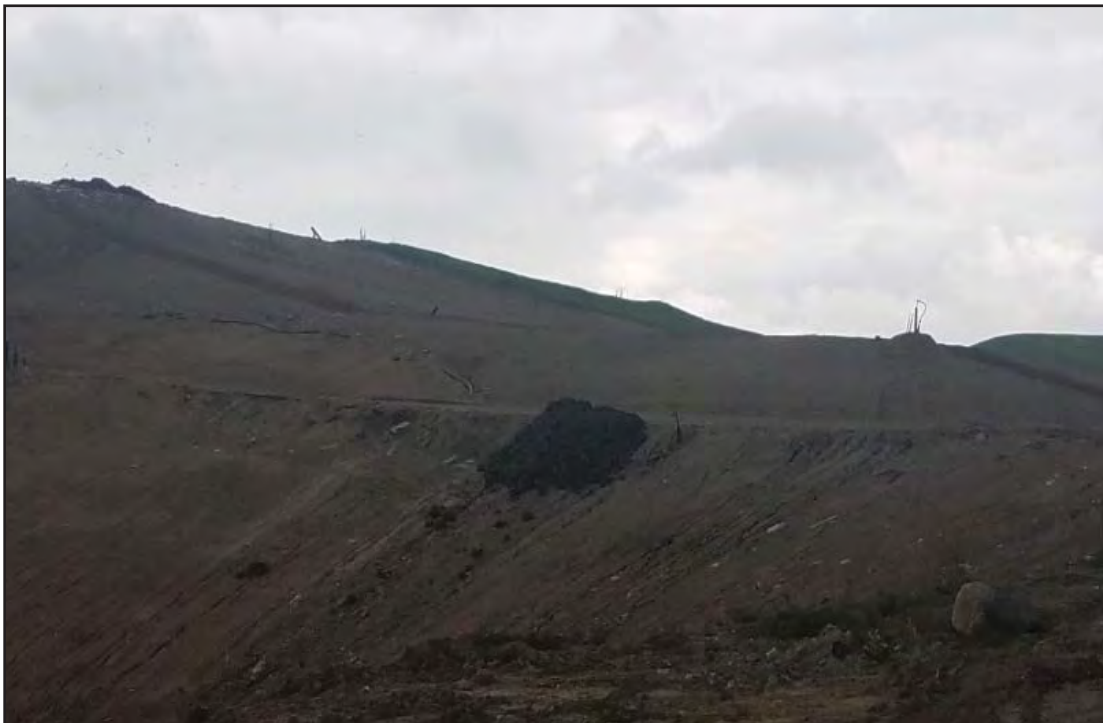
5. Soil stockpile to add to cover for seeps or emissions
