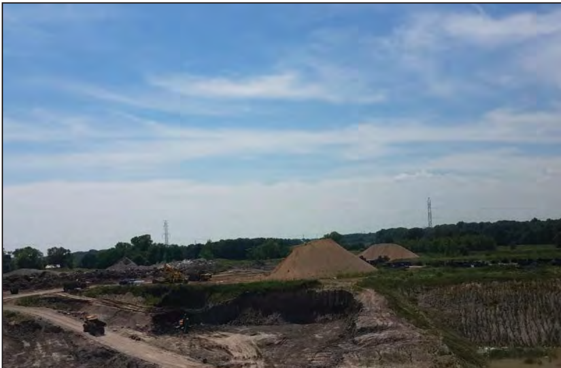
View into future Phase 8 excavation from the East
