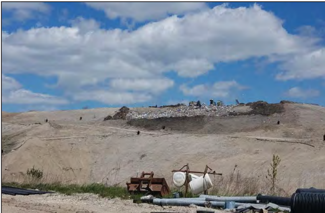
Phase 7 South, West slope, small seeps evident
