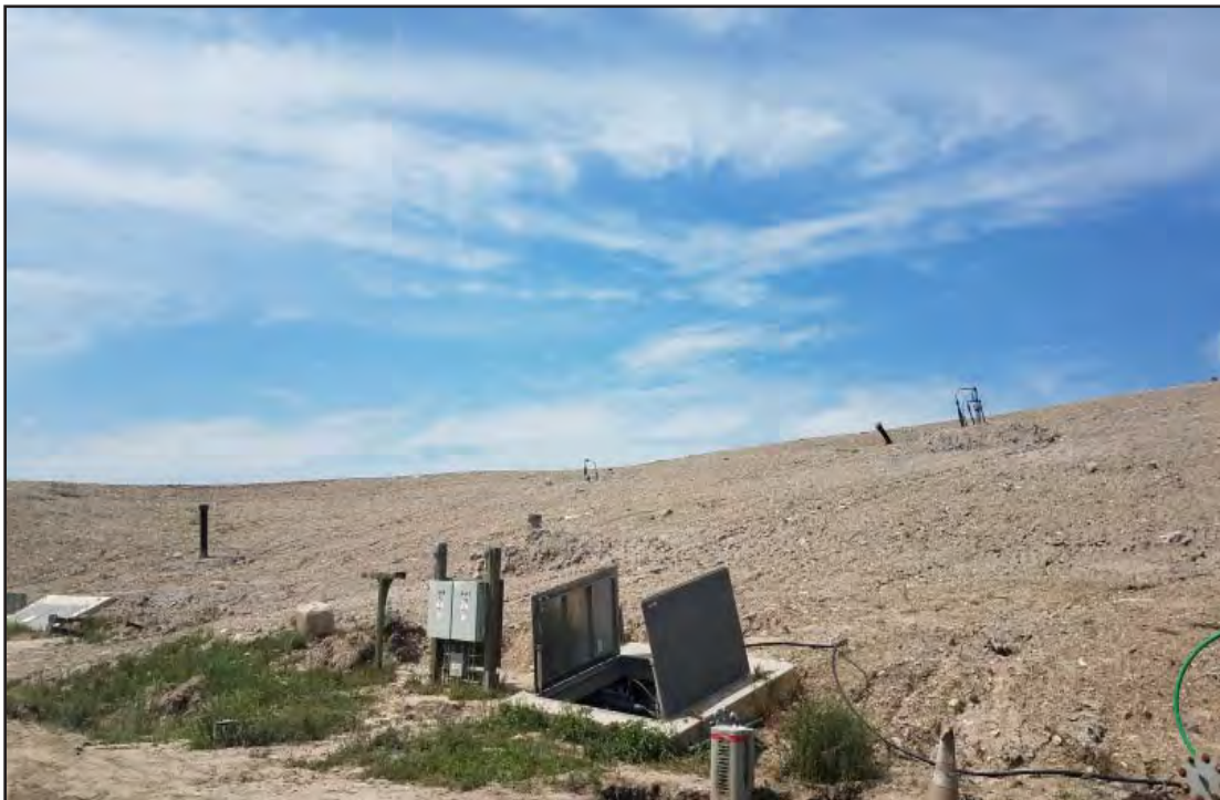
Work in leachate cleanout and system
