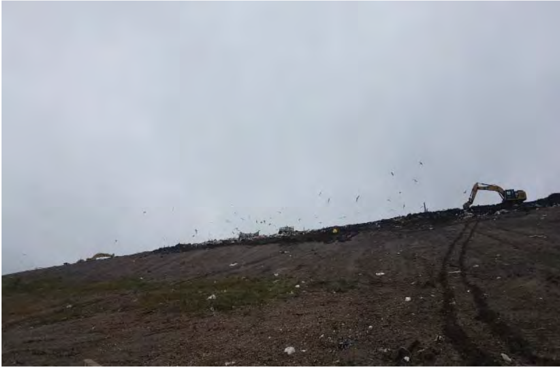
West slope of Phase 7 South, recently backdragged
