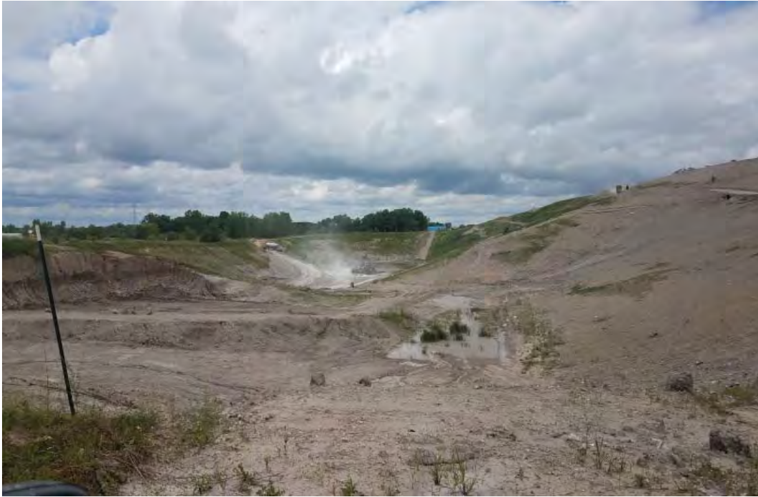
View across temp sed basin, South to North
