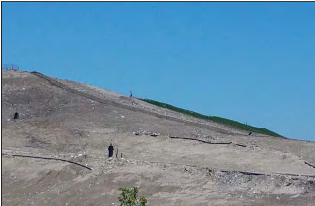
South slope of Phase 7 South, viewed from West
