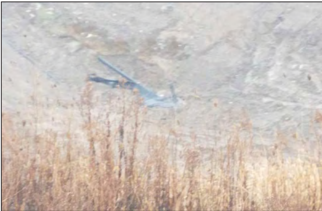
West slope of Phase 7, leachate sideslope riser exposed
