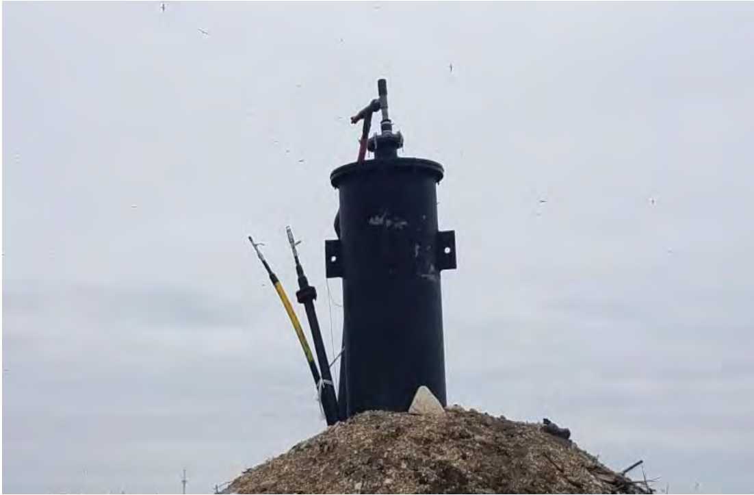
Existing cason well in Phase 7 North
