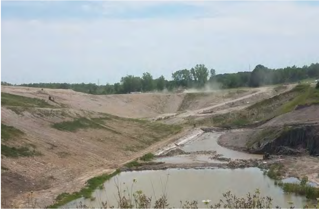
Temp sed basin broken into bays to aid in cleanup and restoration after leach-ate contamination
