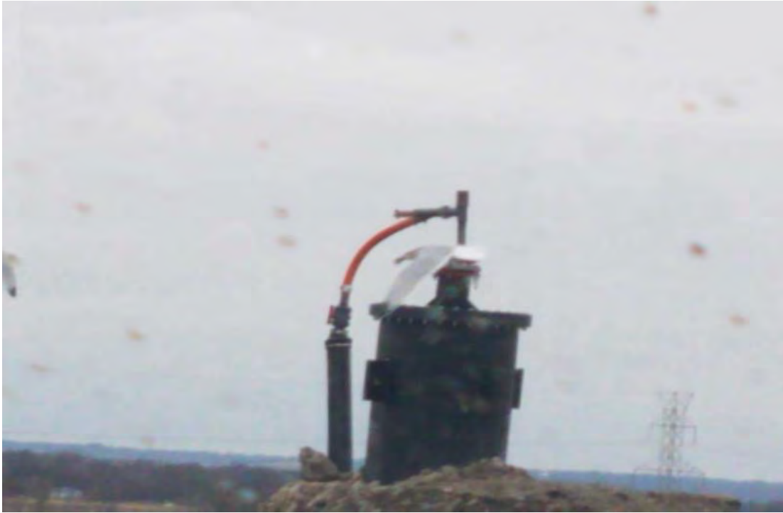
Cason well attached to gas collection system
