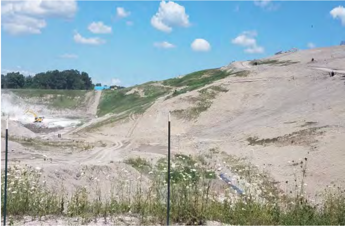
West, outboard slope, of Phase 7 South
