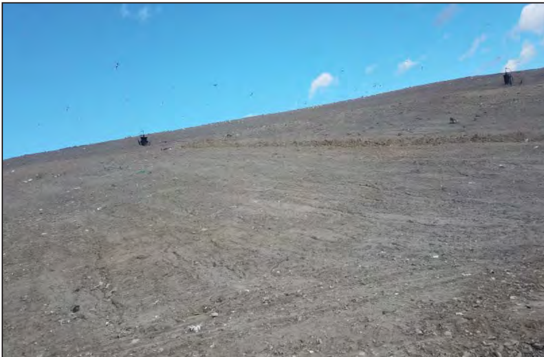
Phase 7 South West slope redressed.
