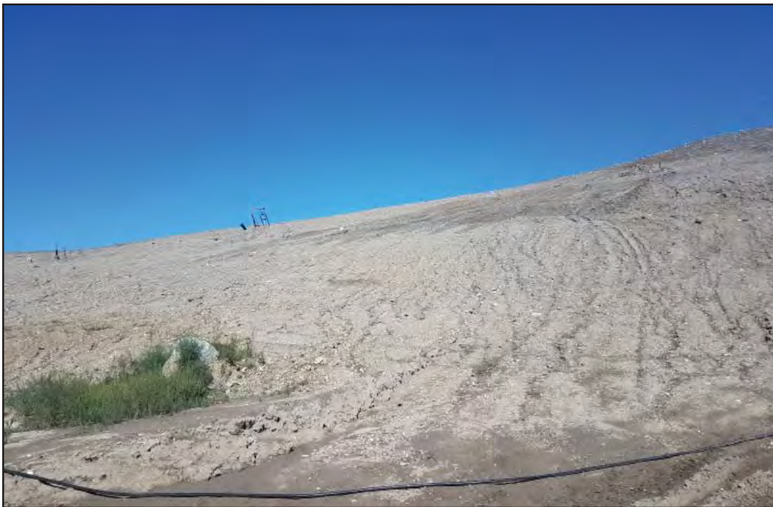
South slope of Phase 7 South showing some erosion
