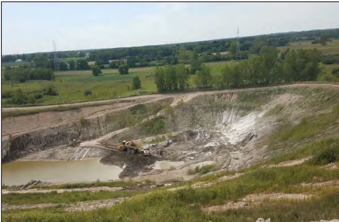
Lost portion of Temp Sed Basin being cleaned of sil, contaminated by leach- ate
