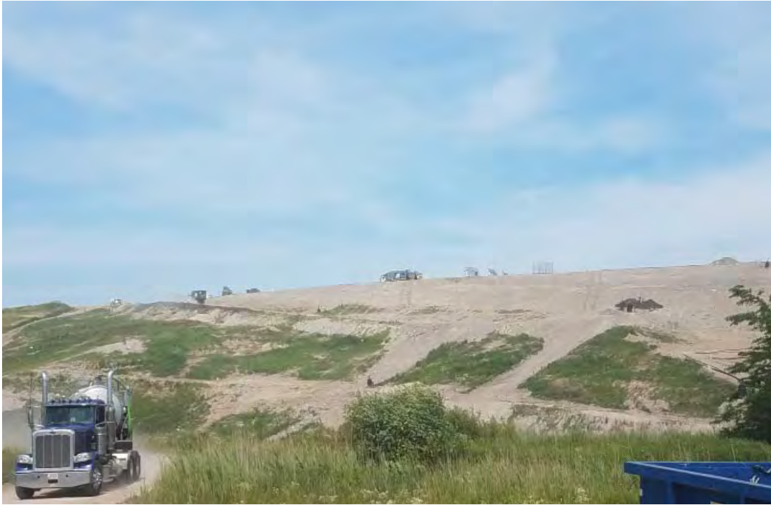
West slope of Phase 7, tanker truck leaving with a load from temp sed basin
