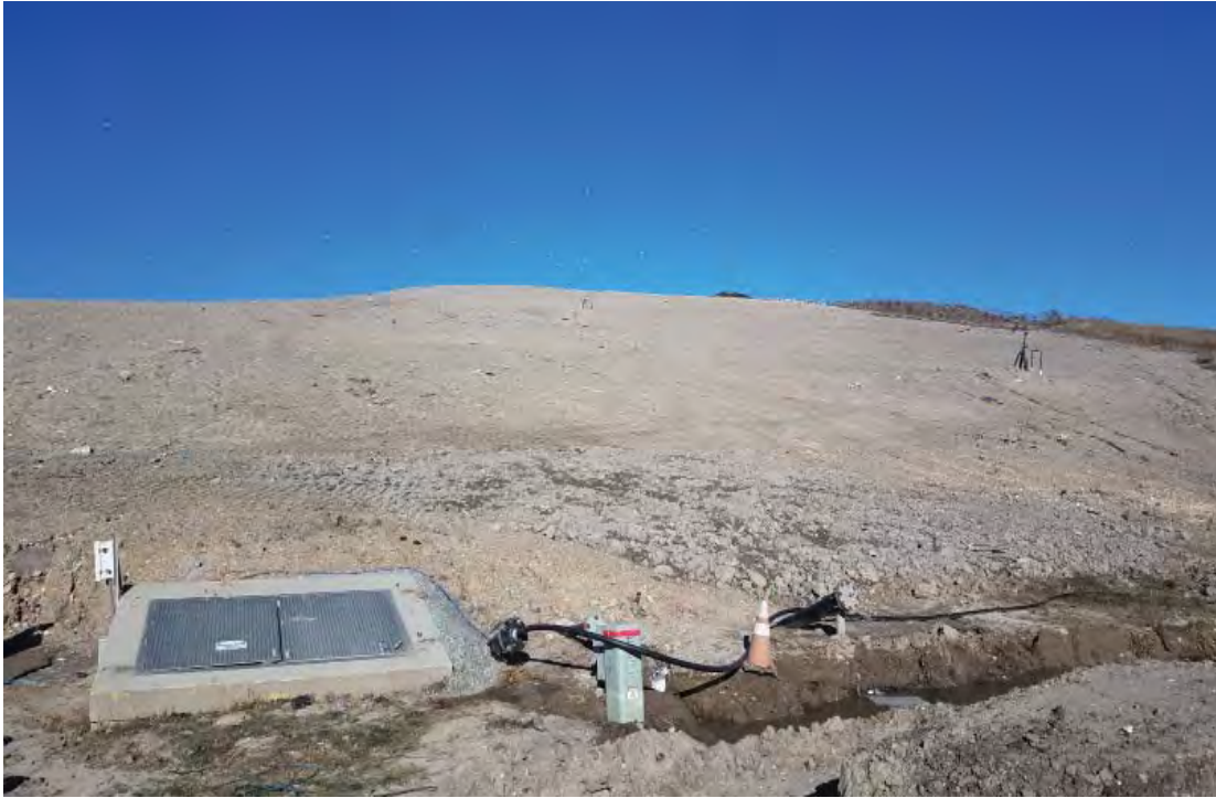
Leachate collection prior to filter tank
