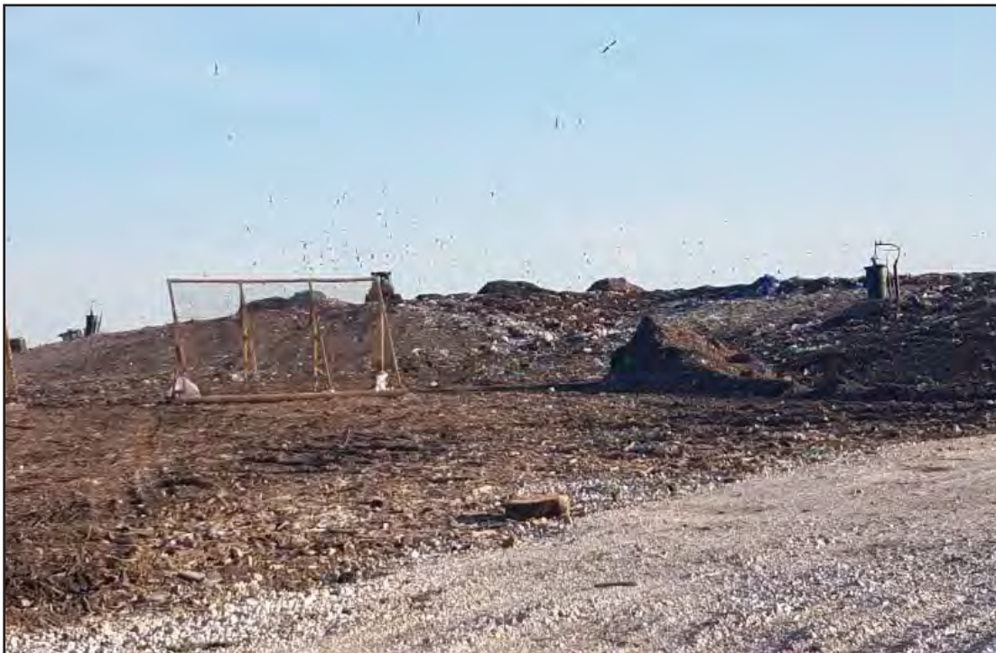
Active area viewed from the North
