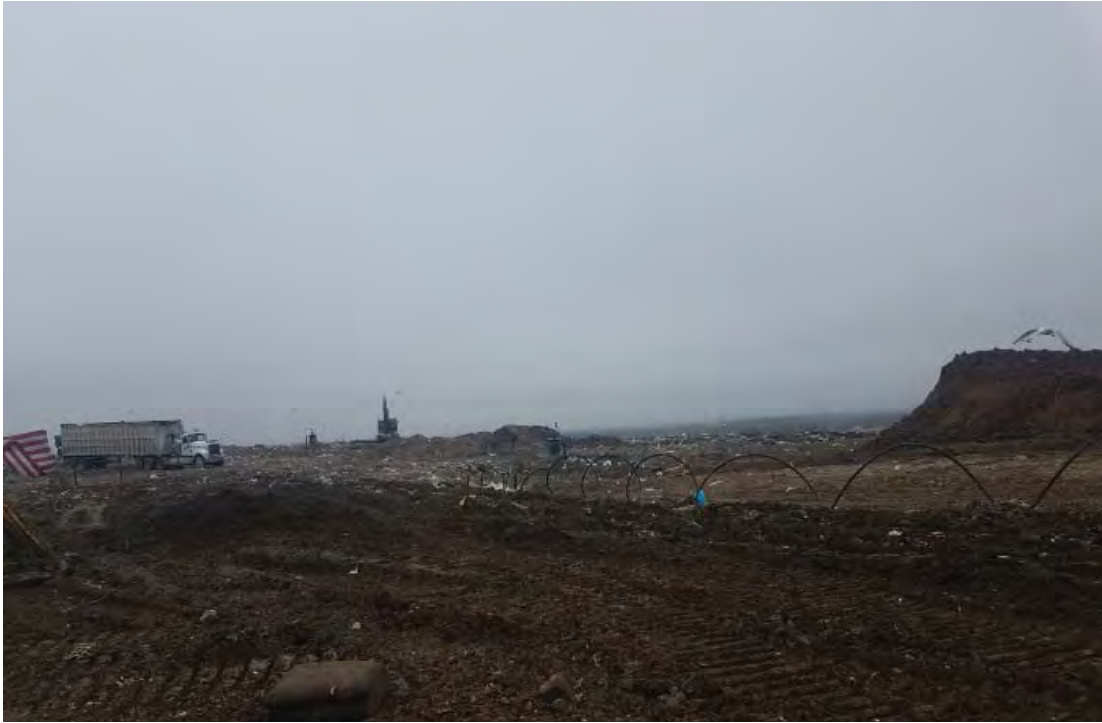
Overview of Phase 7 South
