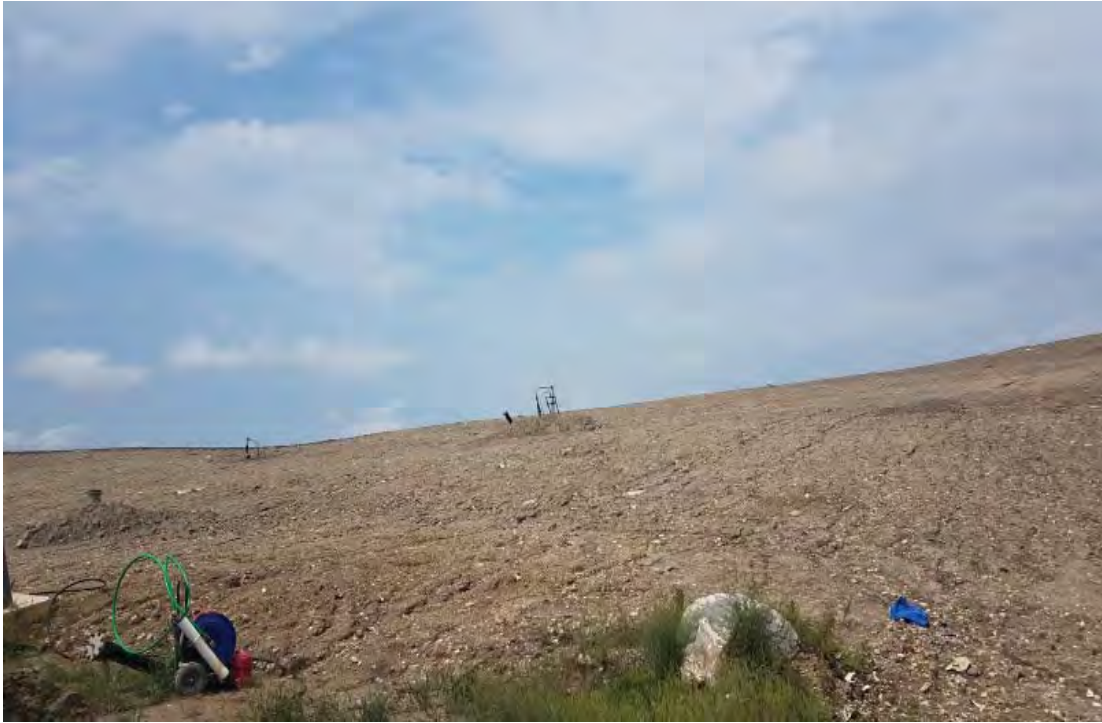
West, outboard slope, of Phase 7 South
