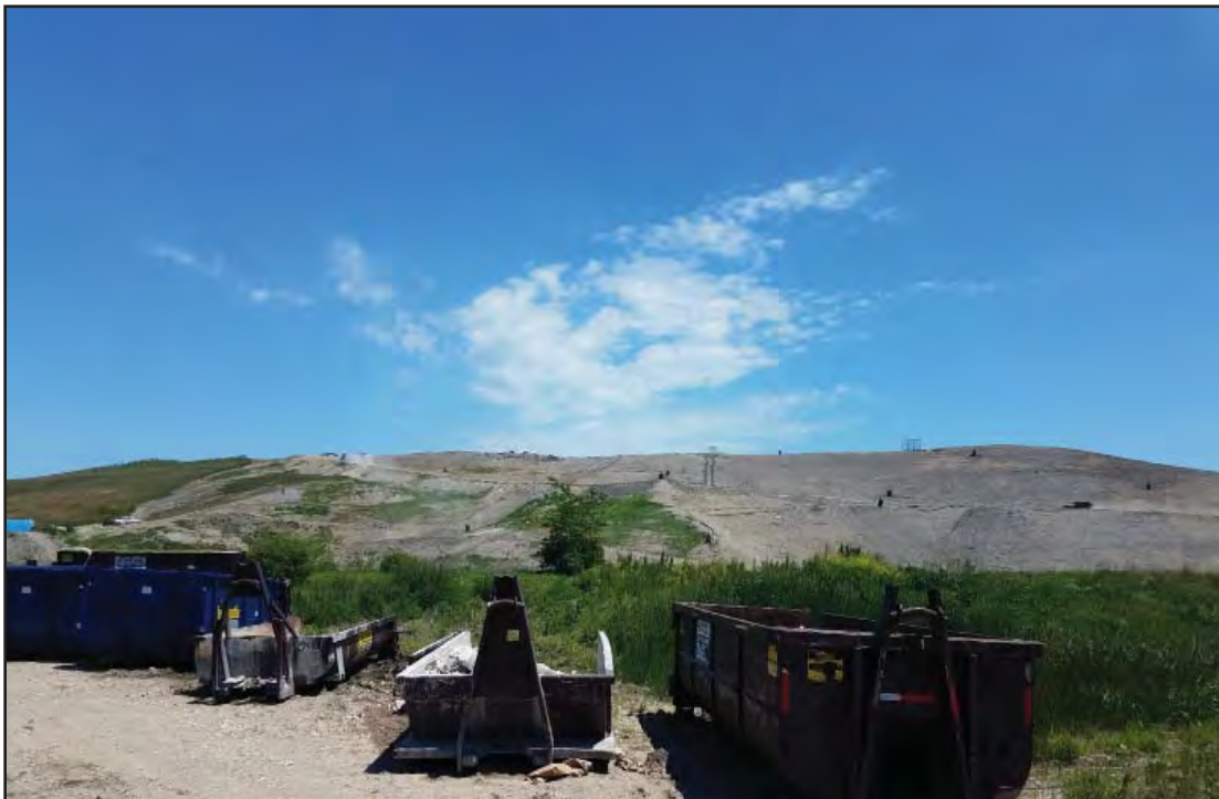
Overview of West slope of Phase 7
