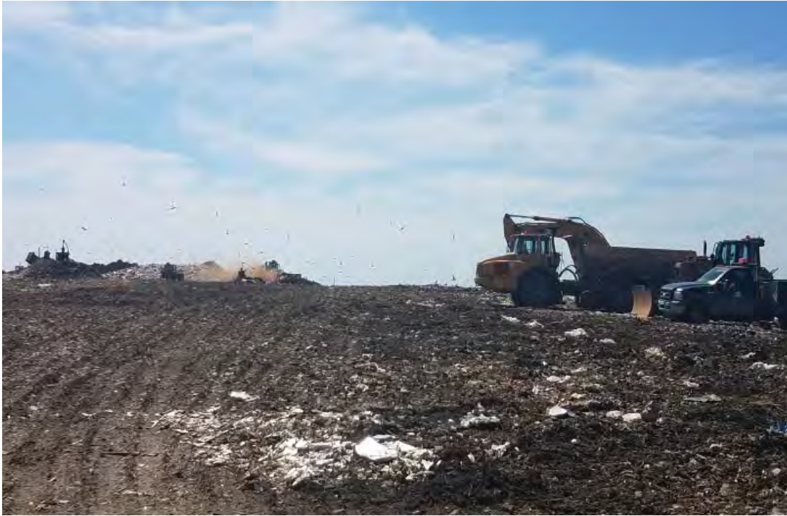
Phase 7 viewed from the North
