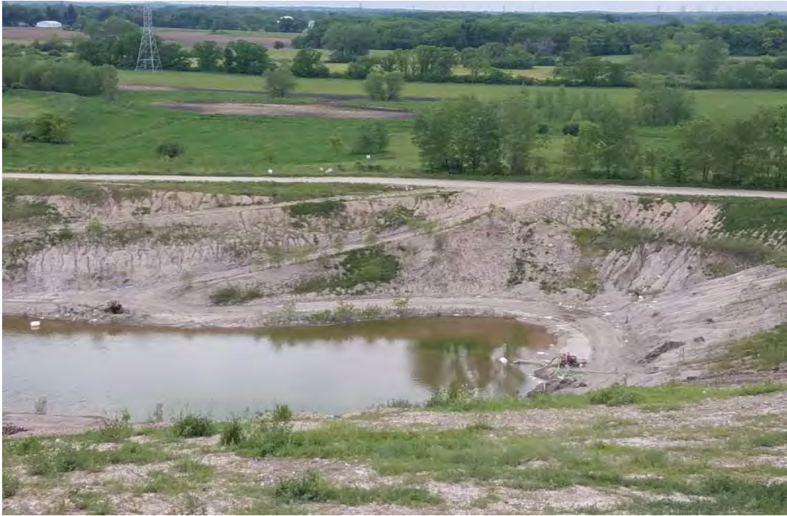
Temp sed basin, contaminated with leachate from seep in Phase 7 South
