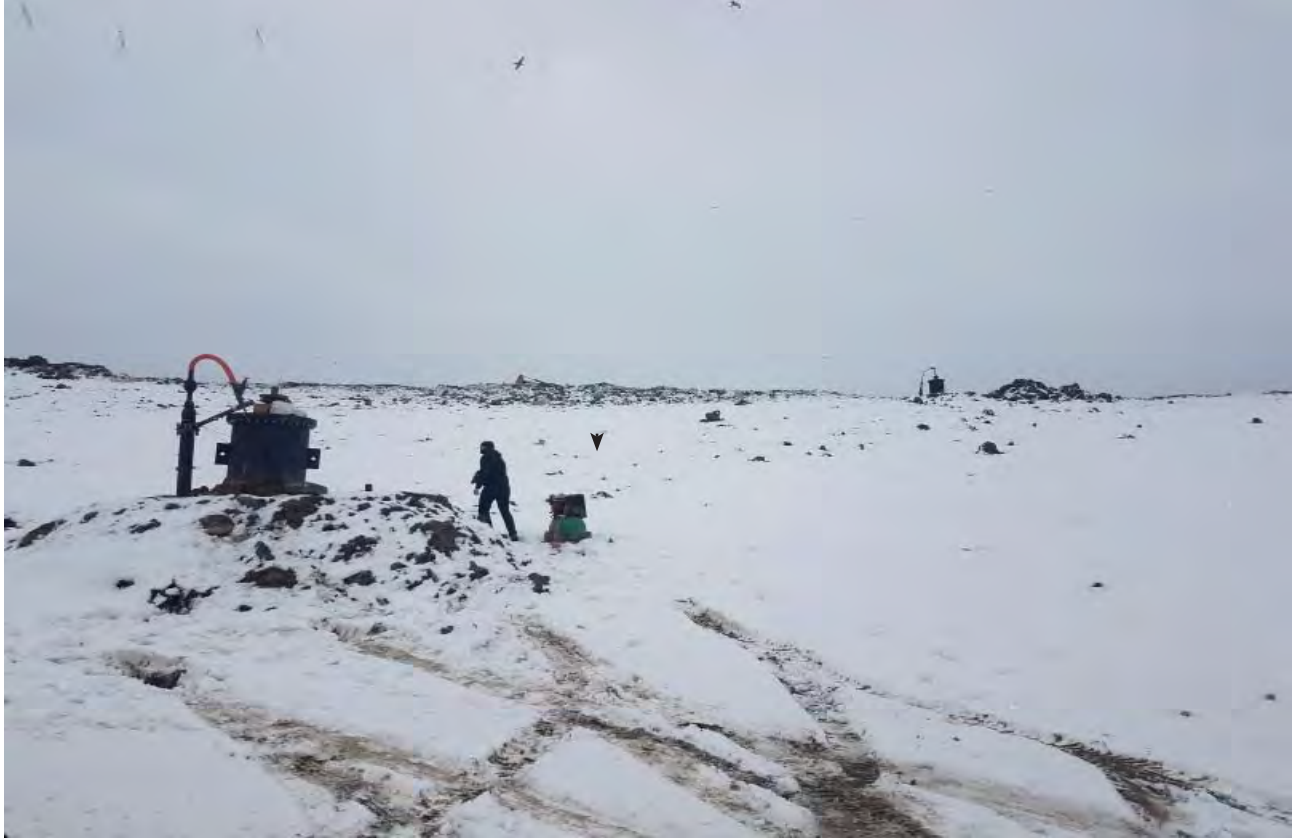
Well in West slope of Phase 7 South, well actively being pumped to remove water and allow gas collection
