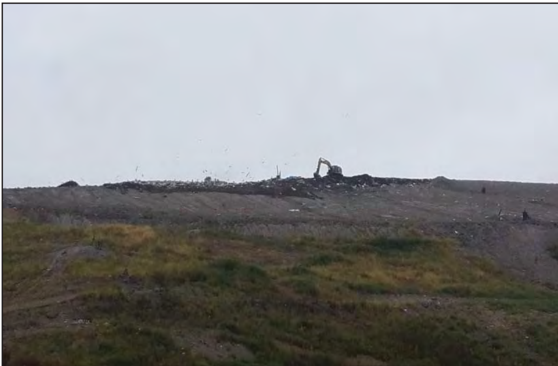
West slope of Phase 7, waste placement right along West edge at top of slope
