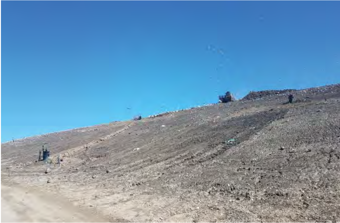
View across Phase 6
