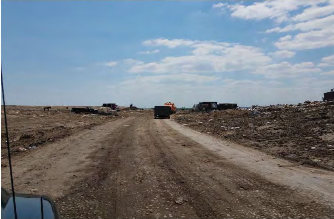
Active area of Phase 7 South, viewed from the North
