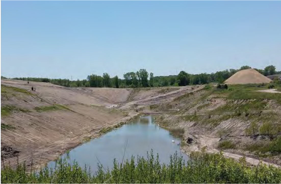
Temp Sed Basin, contaminated with leachate, pumped to tanker for removal
