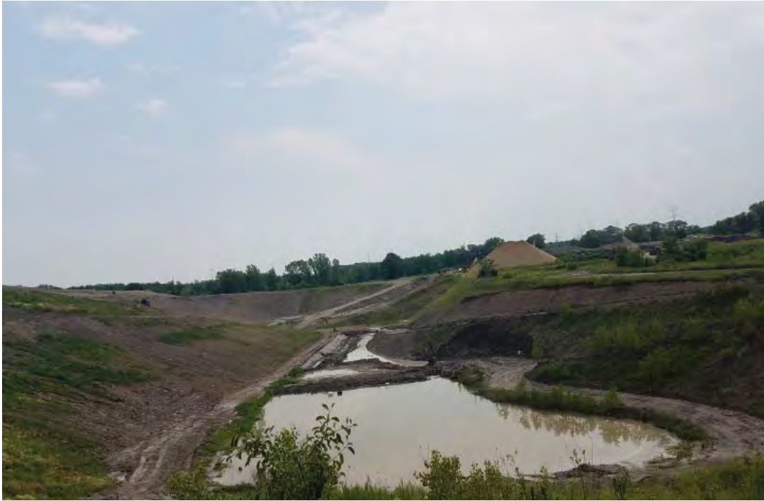
Temp sed basin, cleaning and dredging continue.
