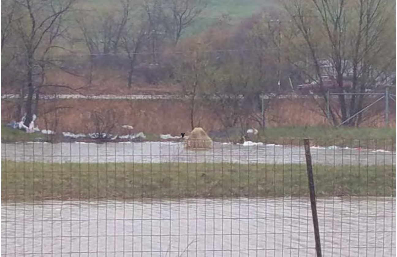
Control structure of Basin 3, litter greatly reduced. Tree growing from control structure
