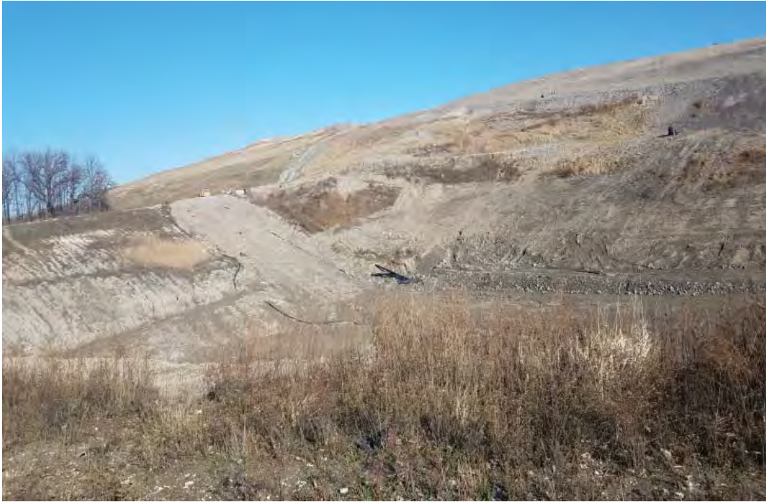
West slope of Phase 7 North
