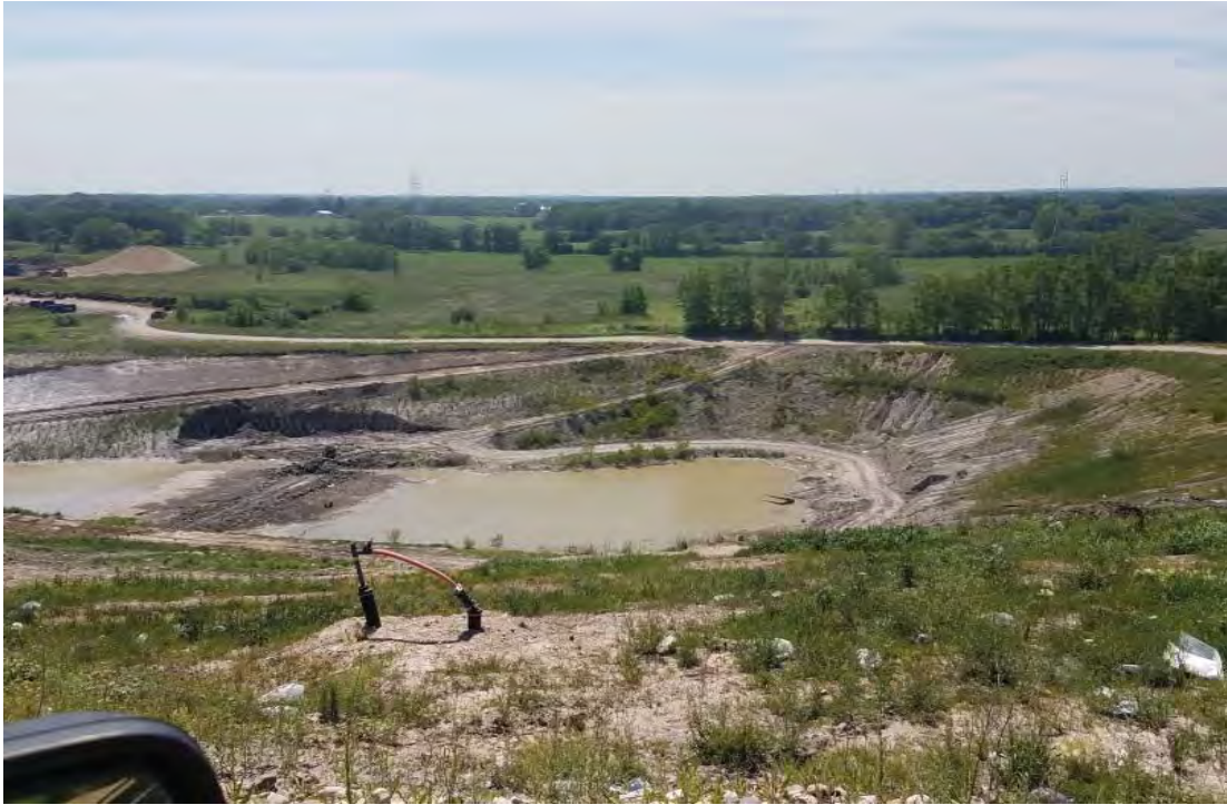
Temp sed basin split to manage leachate contamination
