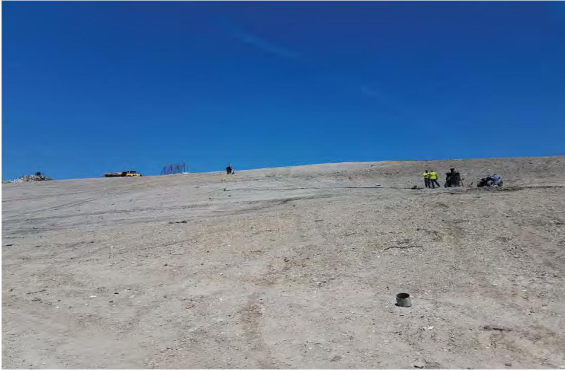
West slope of Phase 7 above access road
