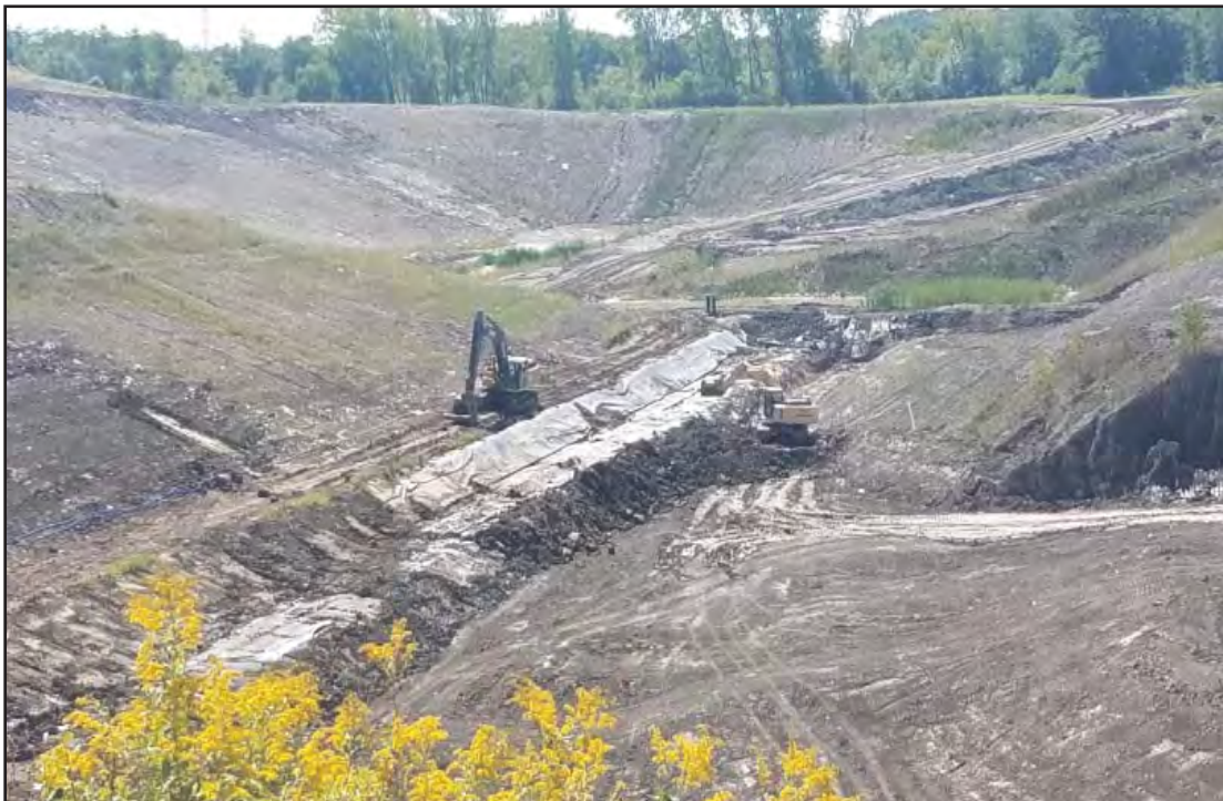
Seep repair to rainflap ongoing, there was a large volume of trapped leachate
