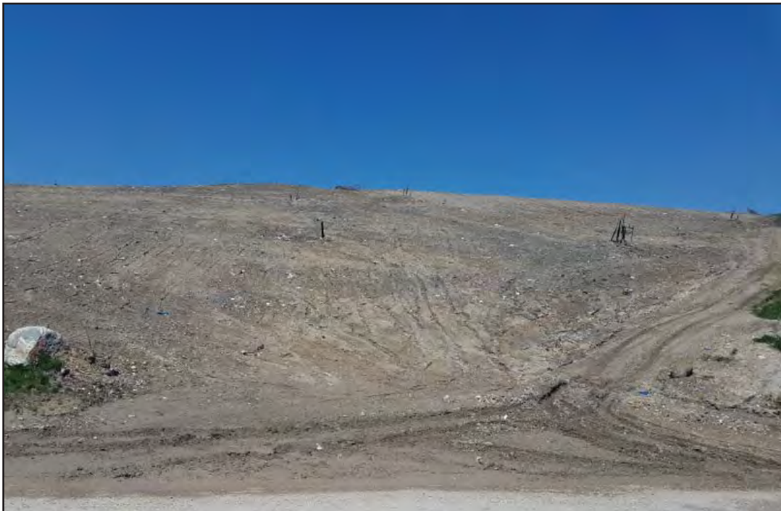
South slope with some erosion after two days of storms
