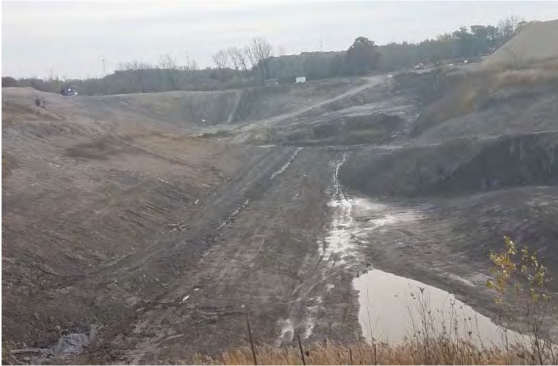
Temp sed basin reformed, access road about toe of Phase 7 slope complete
