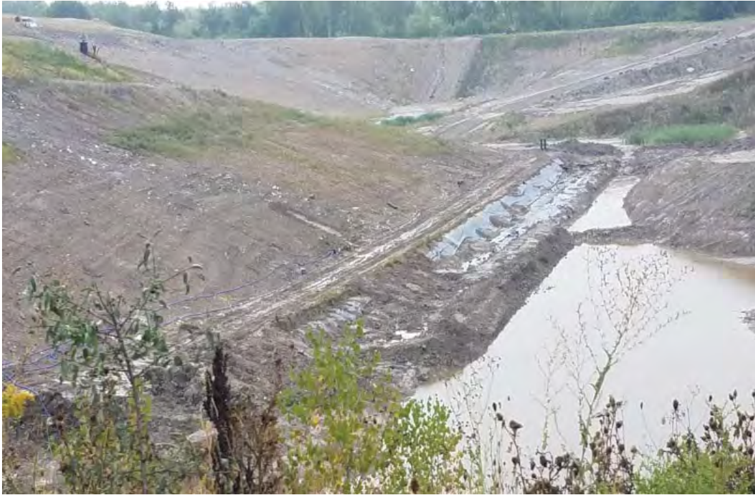
Temp sed basin viewed from the North, earth berm to separate leak from rain-flap and remainder of basin
