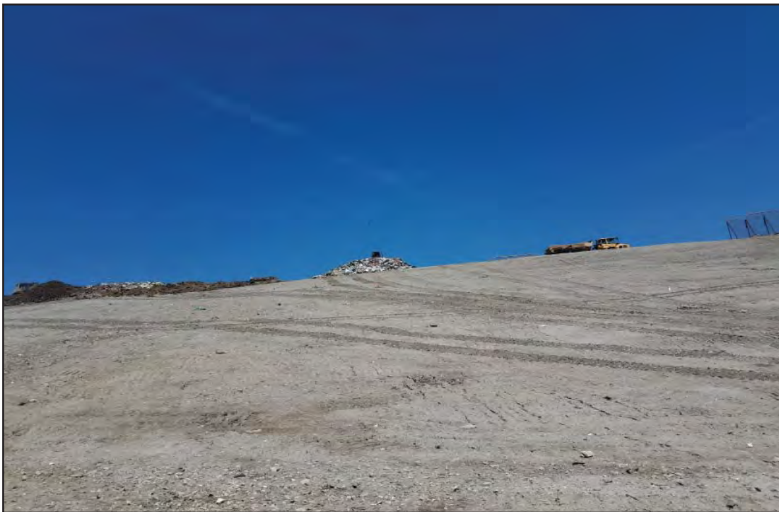
West slope of Phase 7 above access road
