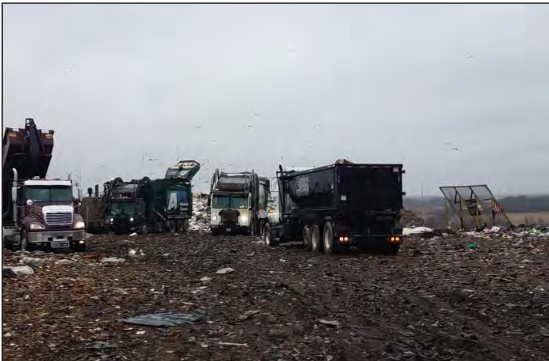
Tipping at Working face, two trucks active, one arriving and one departing
