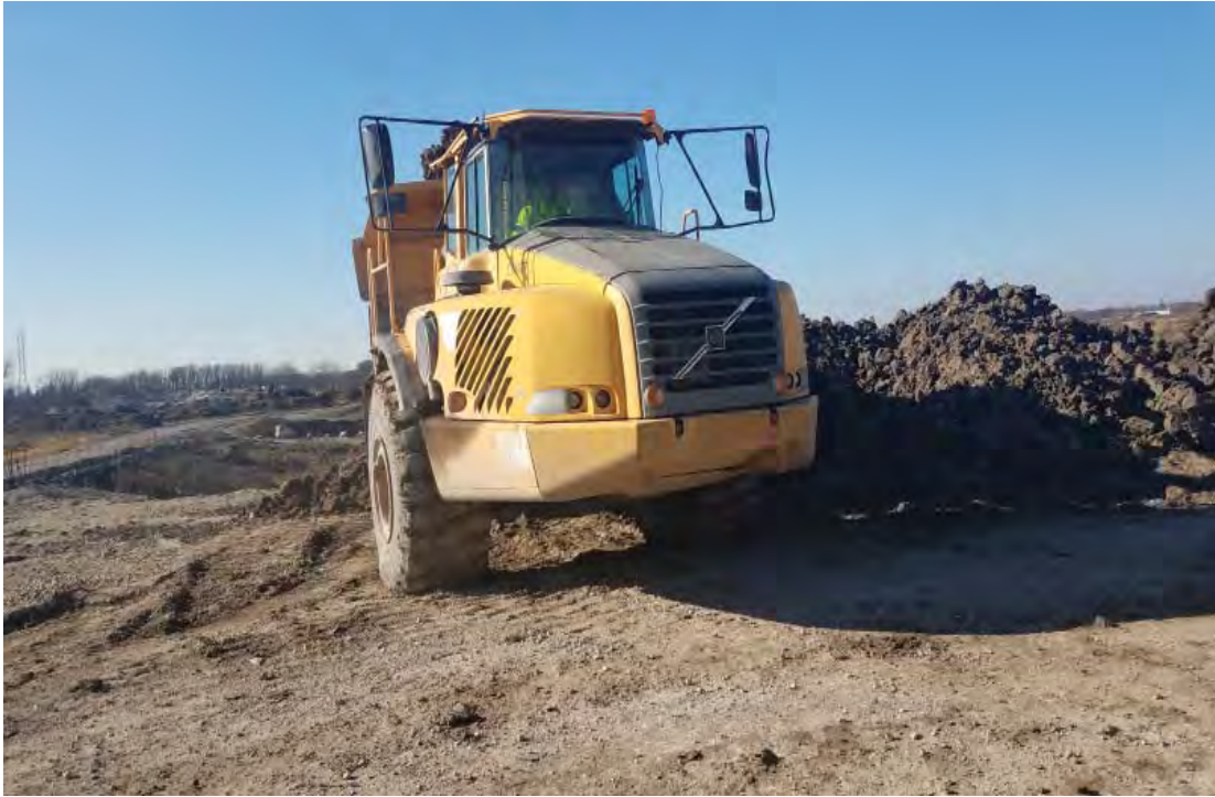
Soils being added to West slope of Phase 7 South to improve intermediate cover
