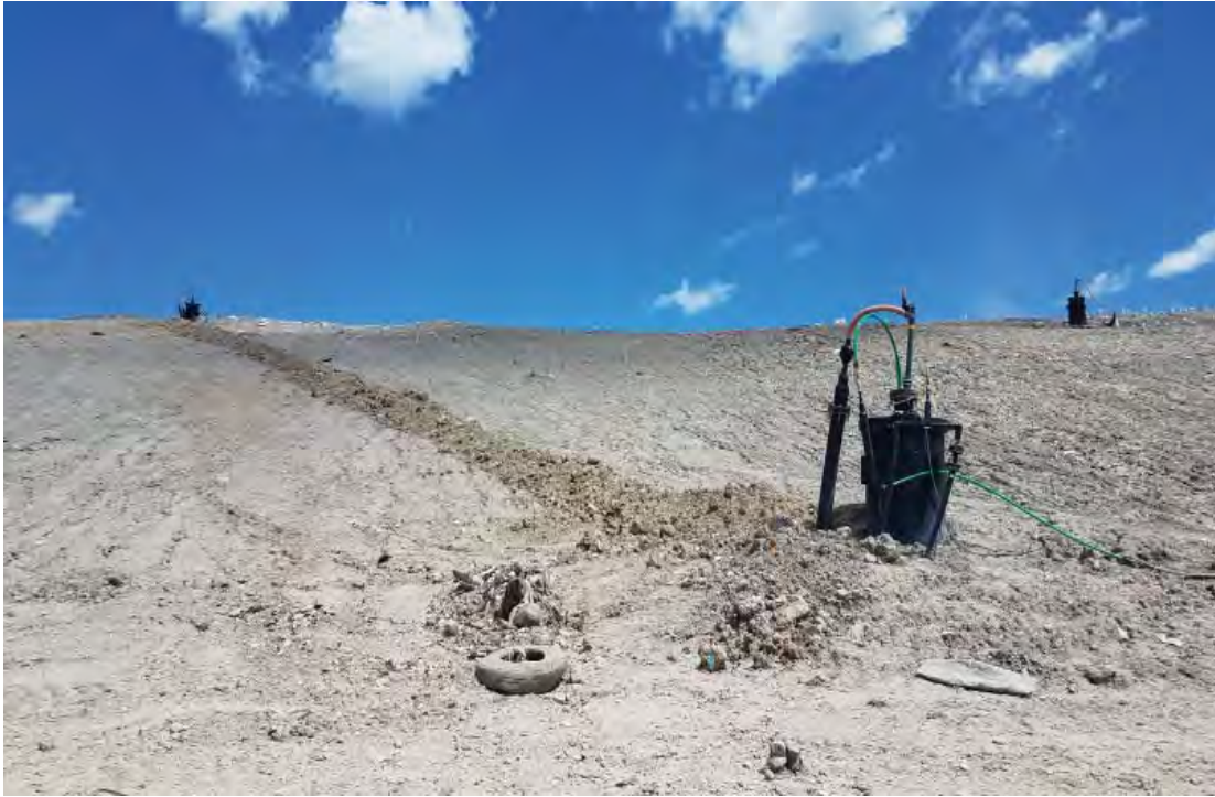
New connection between wells in Phase 7
