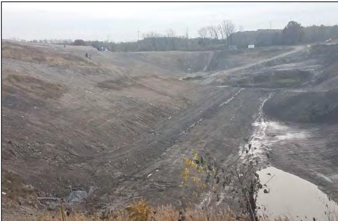
New access road about Phase 7 South toe of slope, protects rain flap
