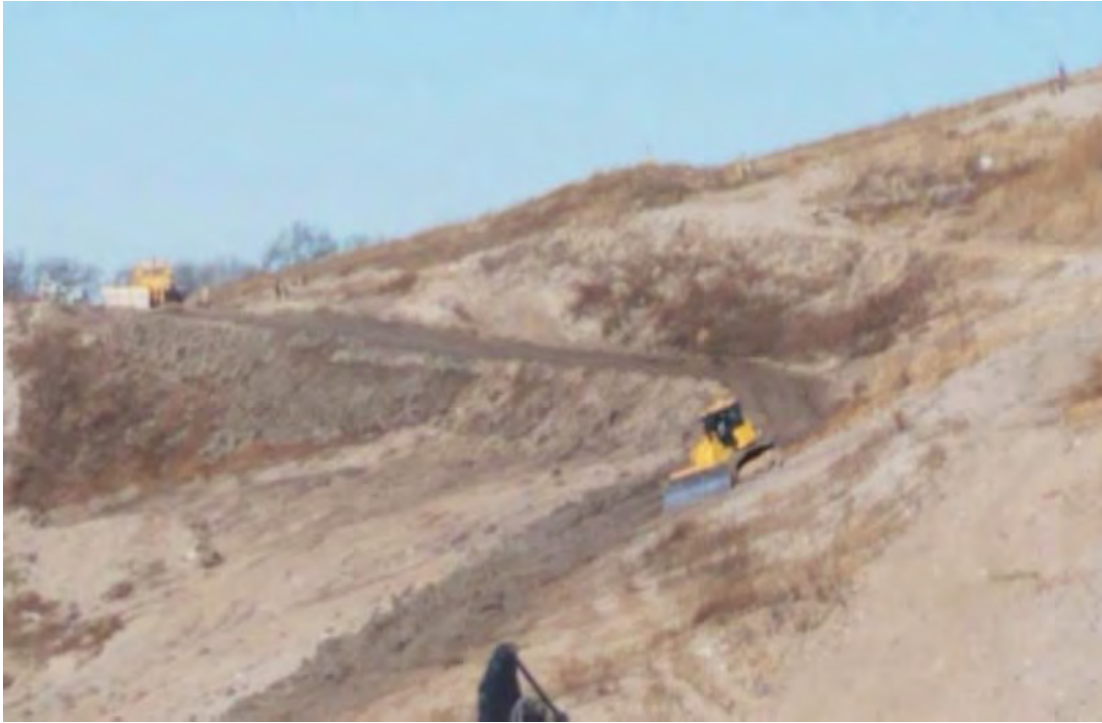
Access road built over rainflap at toe of West slope of Phase 7
