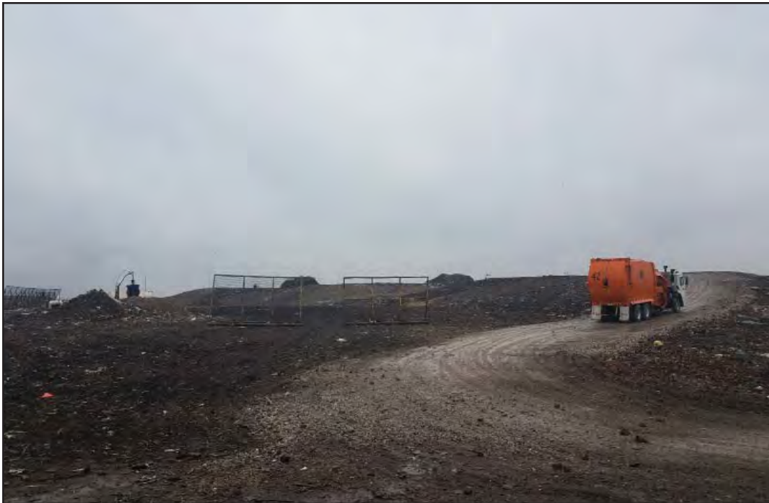
Access road to Working face, area very tight, face is small due to volume
