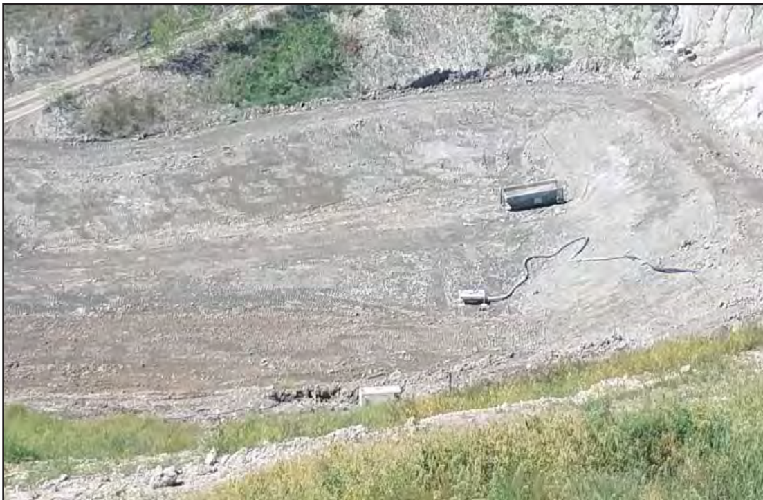
Temp Sed Basin, cleaned and drained
