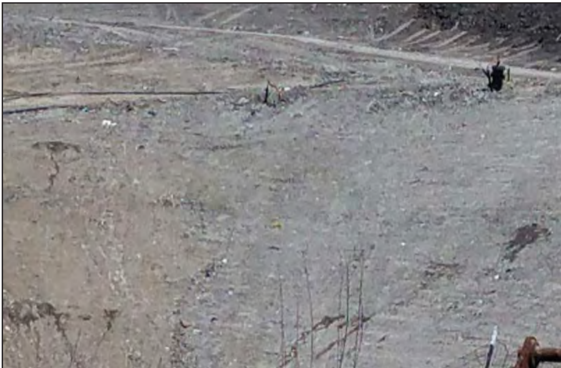
West slope of Phase 7 South, small seeps have appeared, self cured, and then reappeared
