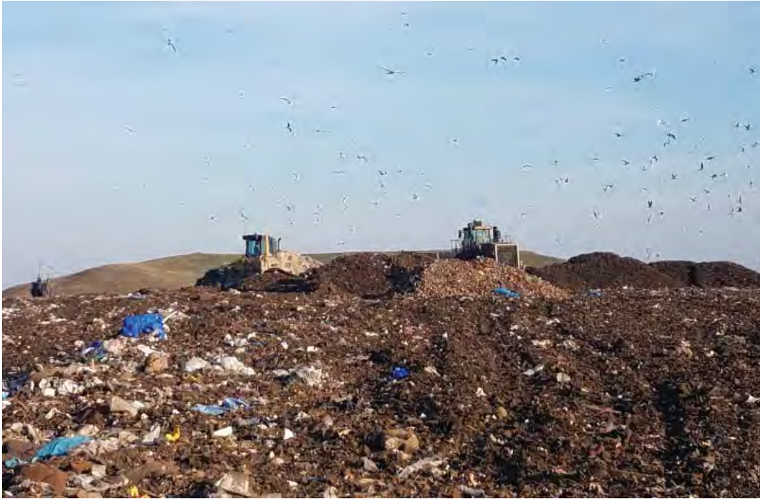
Active area in Southeast corner of Phase 7 South, abundance of autofluff for daily cover stockpiled
