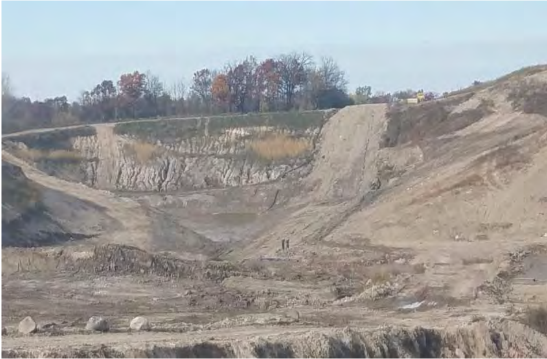
Temp sed basin viewed from the South, reshaped for better protection of rain-flap
