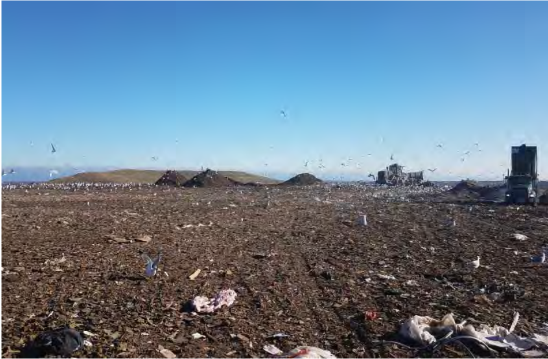
Cover materials stockpiled in active area
