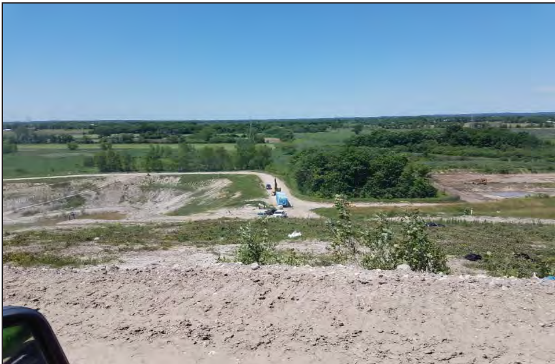
Filter trailer for removing sediment from Temp Sed Basin leachate clean up
