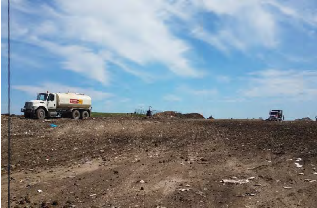
Phase 7 viewed from the North
