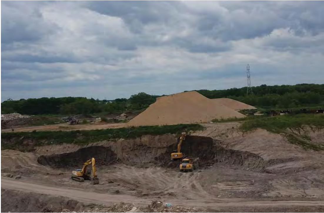
Excavation of future Phase 8
