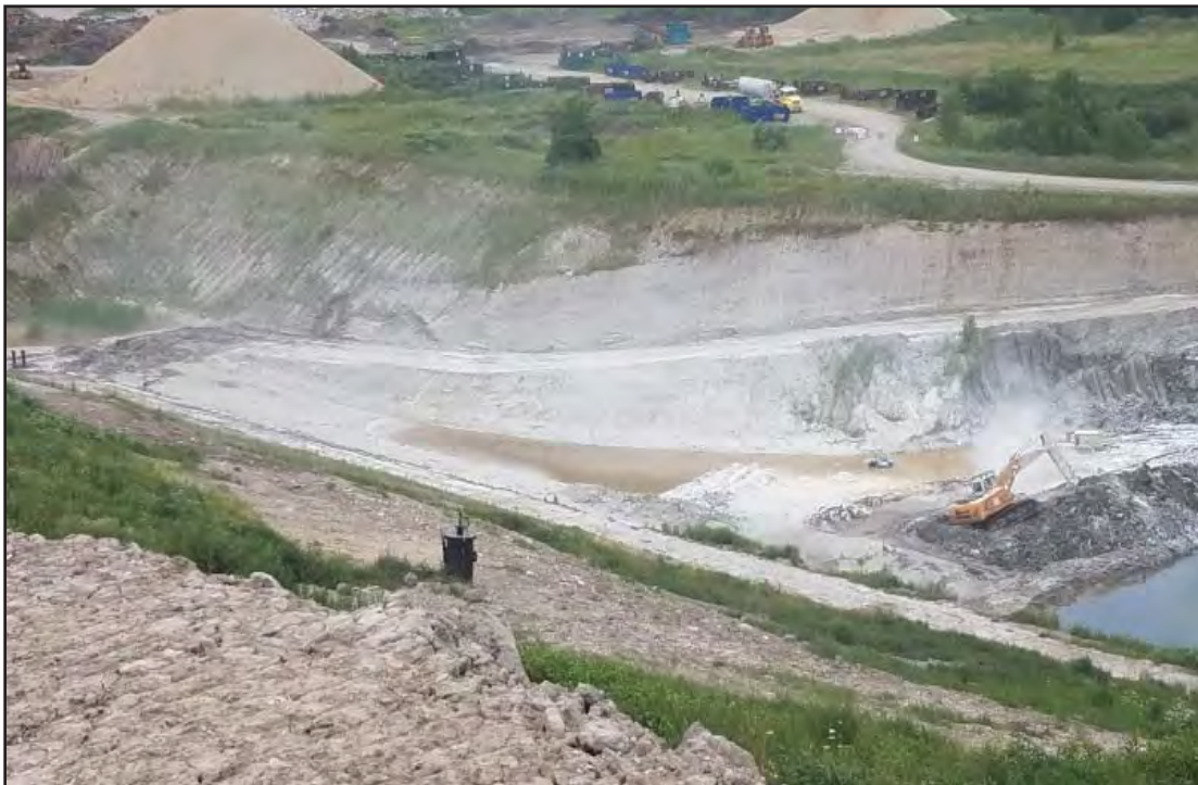
South end of temp basin, certified clean
