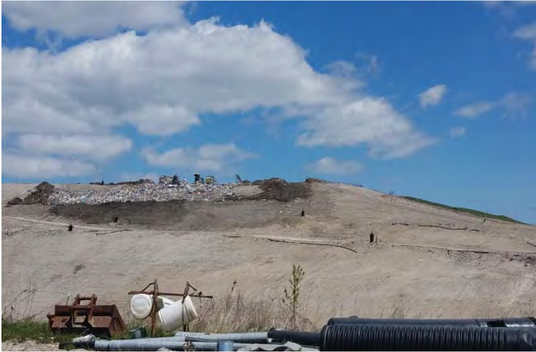
Phase 7 South, Southwest corner
