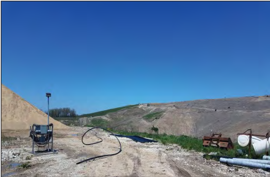
West slope of Phase 7 North
