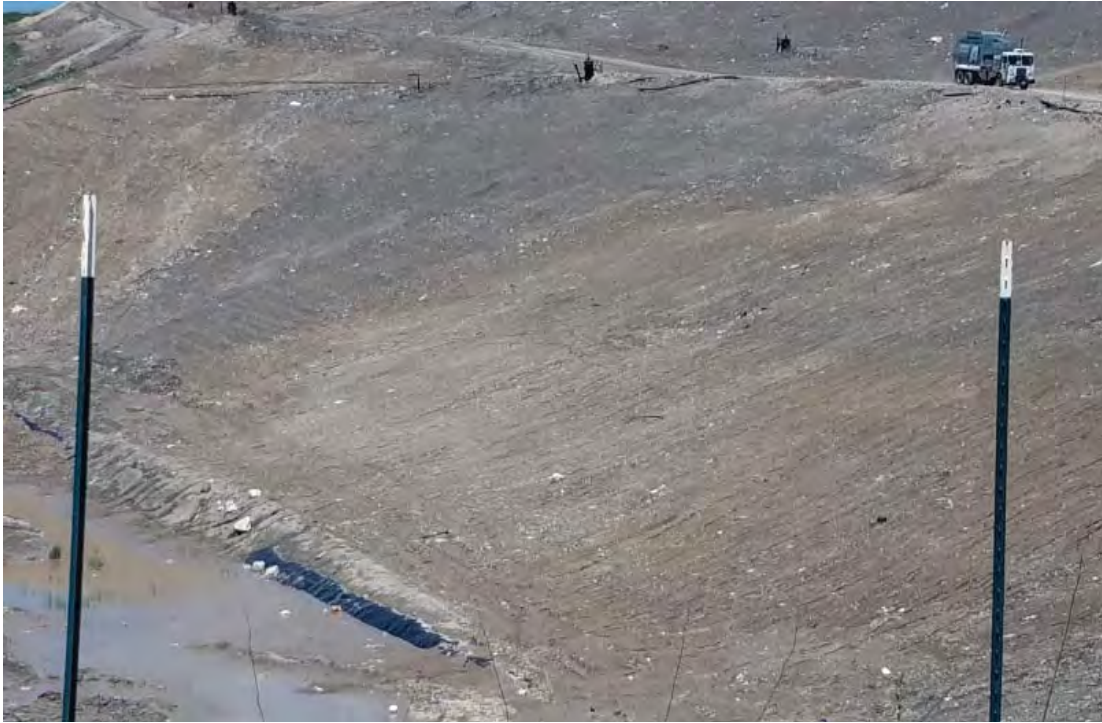
South portion of Temp Sed Basin, adjacent to Phase 7 South
