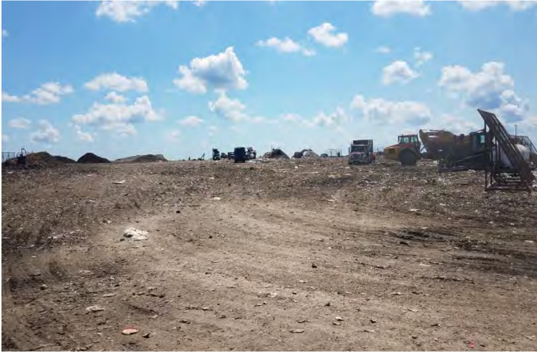
Phase 7 viewed from the North
