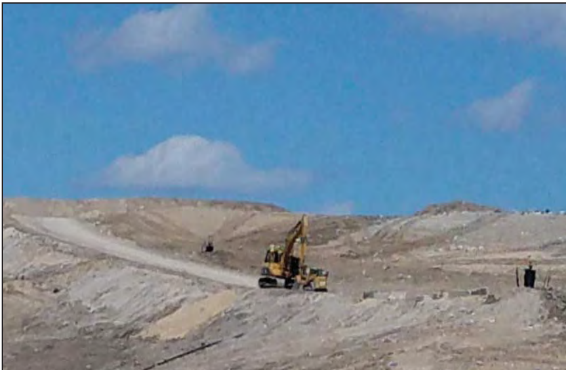
Trenching complete on West slopes and slope patched
