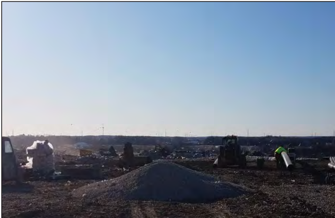
Contractor staging area on Phase 7 North
