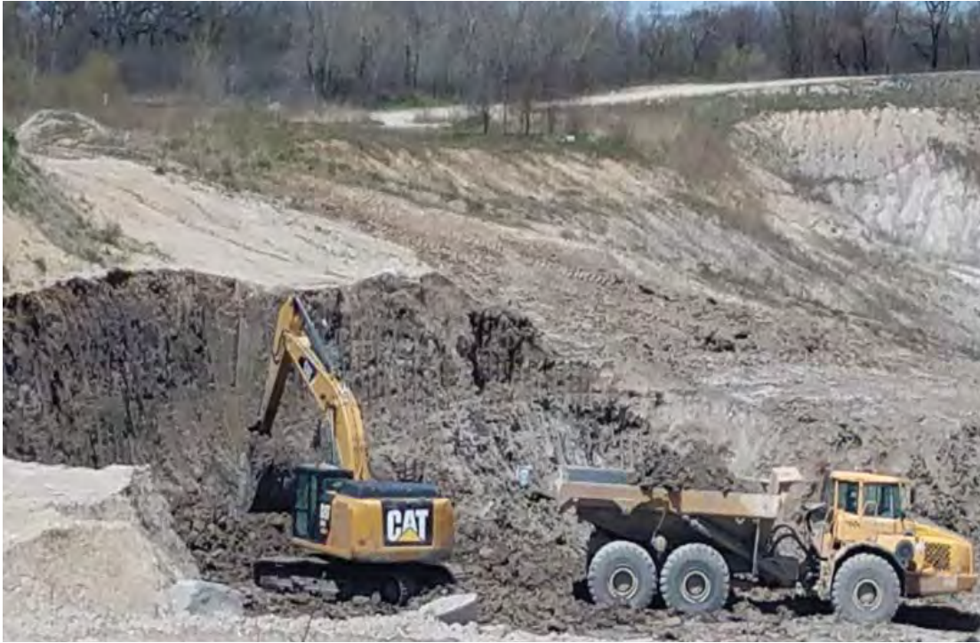
Continued excavation of future Phase 8, material being used for cover on slope
