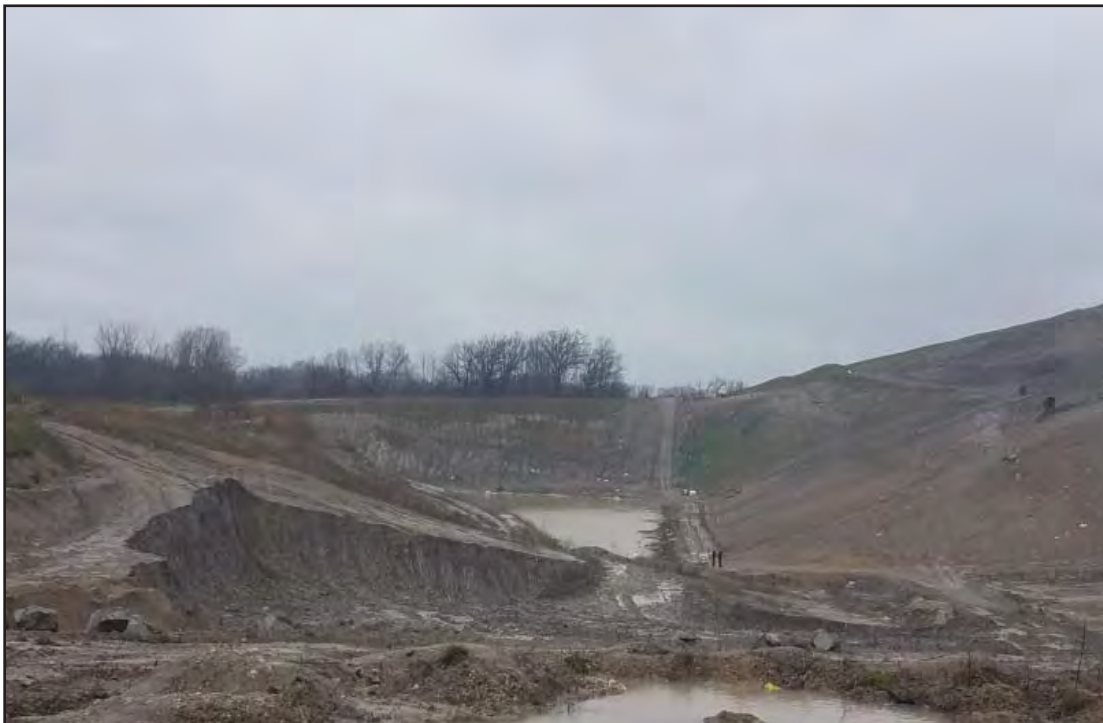
Temp. Sed Pond well pumped
