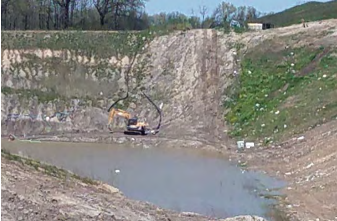
Temp sed basin, well pumped down
