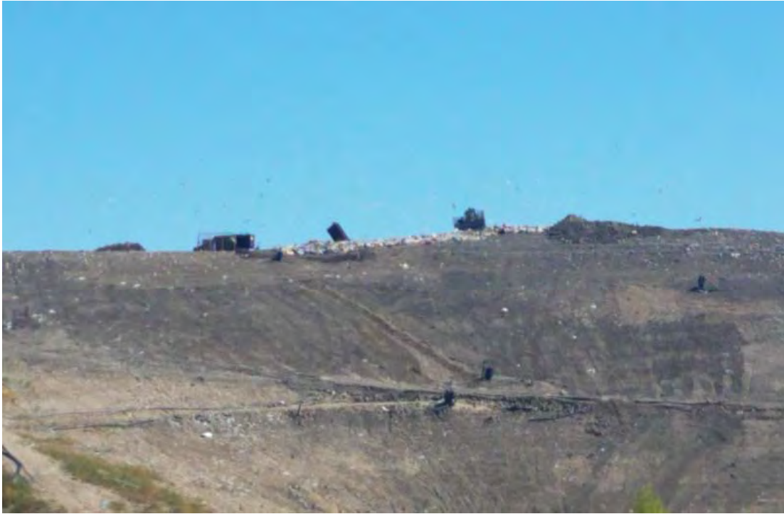
West slope of Phase 7 South, edge of working face visible
