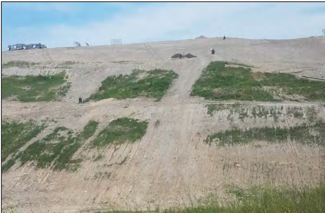
West slope of Phase 7, no evident seeps
