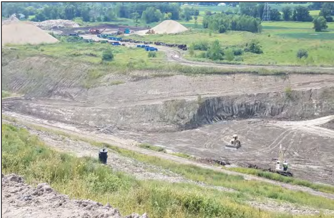
Dozer regrading "clean" area of temp sed basin
