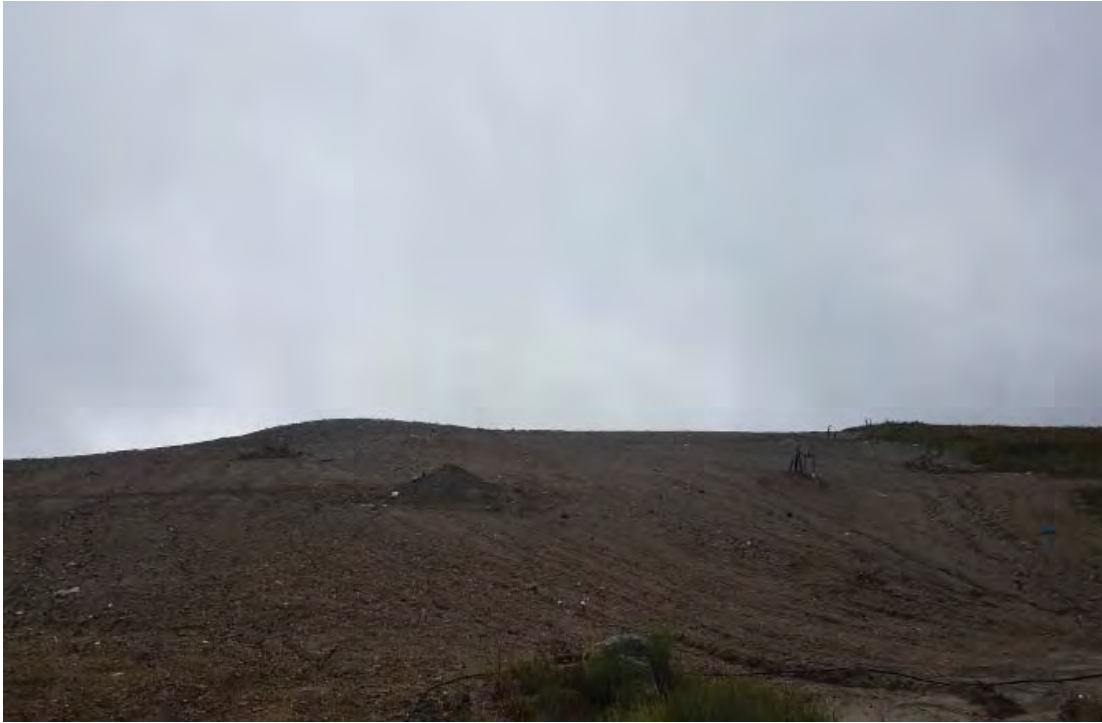
West slope of Phase 7 South, recently backdragged
