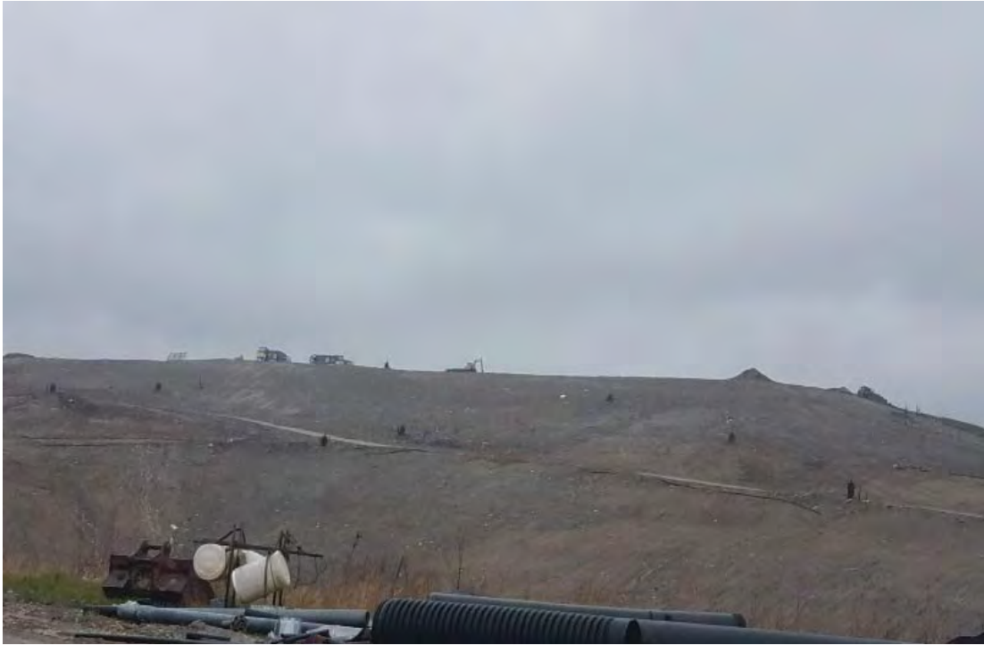
Phase 7 viewed from the West
