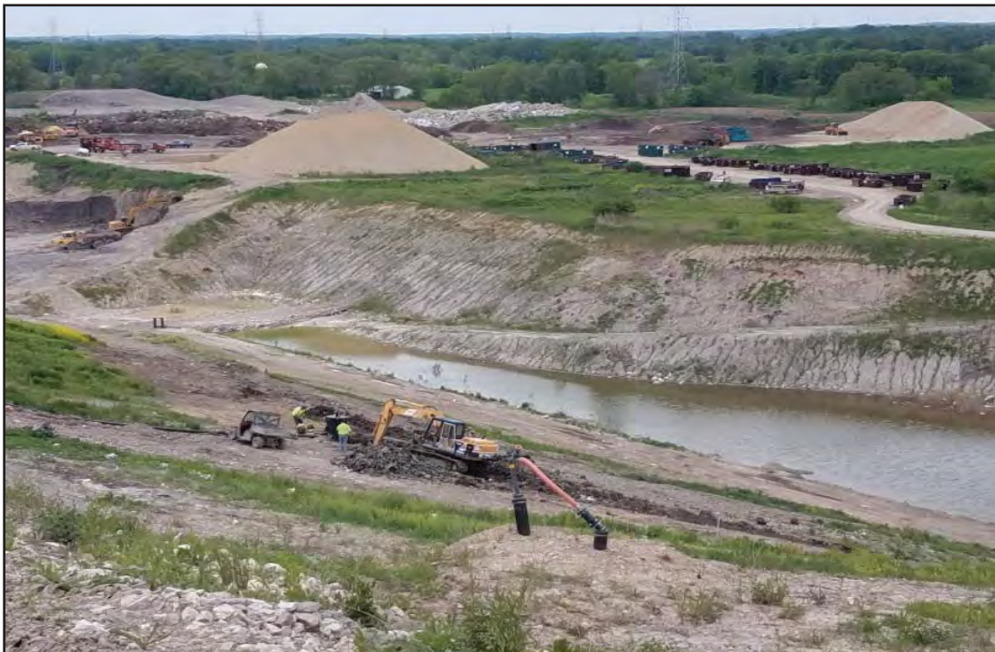
Gas system repairs on Phase 7 North, West slope
