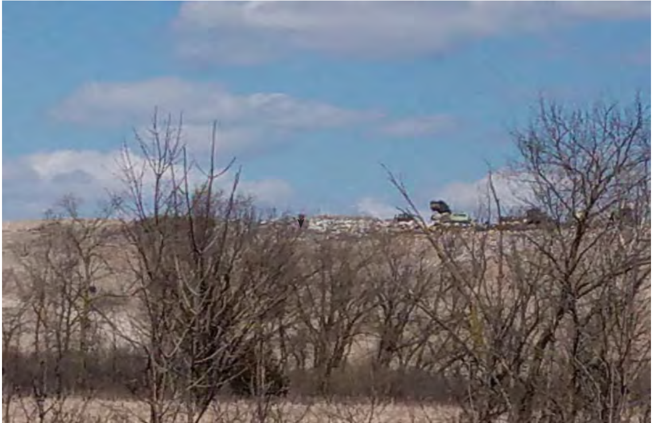
Working face viewed from Union Church Road from the South.
