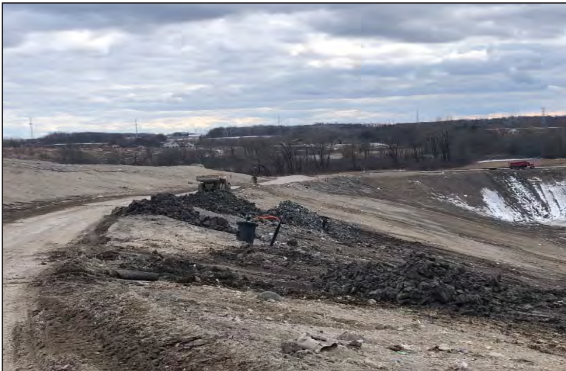
West slope of Phase 7 with completed horizontal wells and air supply
