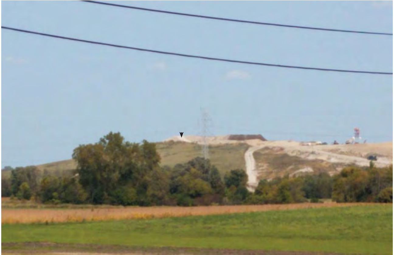
Phase 3 viewed from the West at a distance, new soils from cleaning up temp sed basin in center of photo, dark soil
