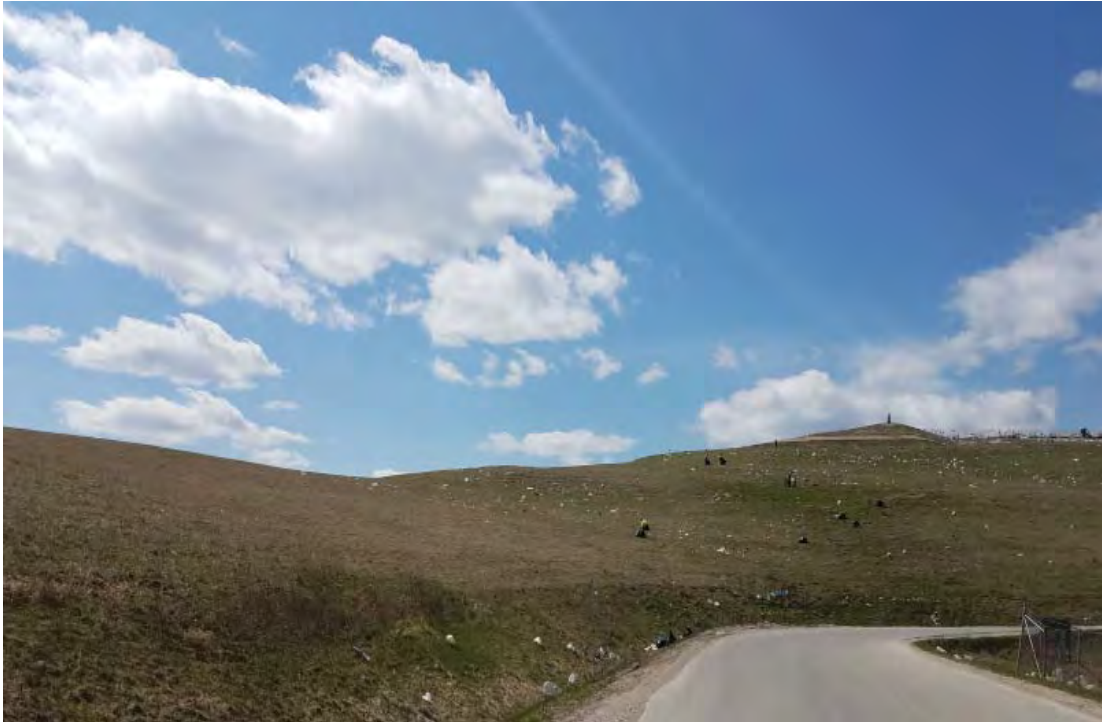
East slope of Phase 5, picker active in image
