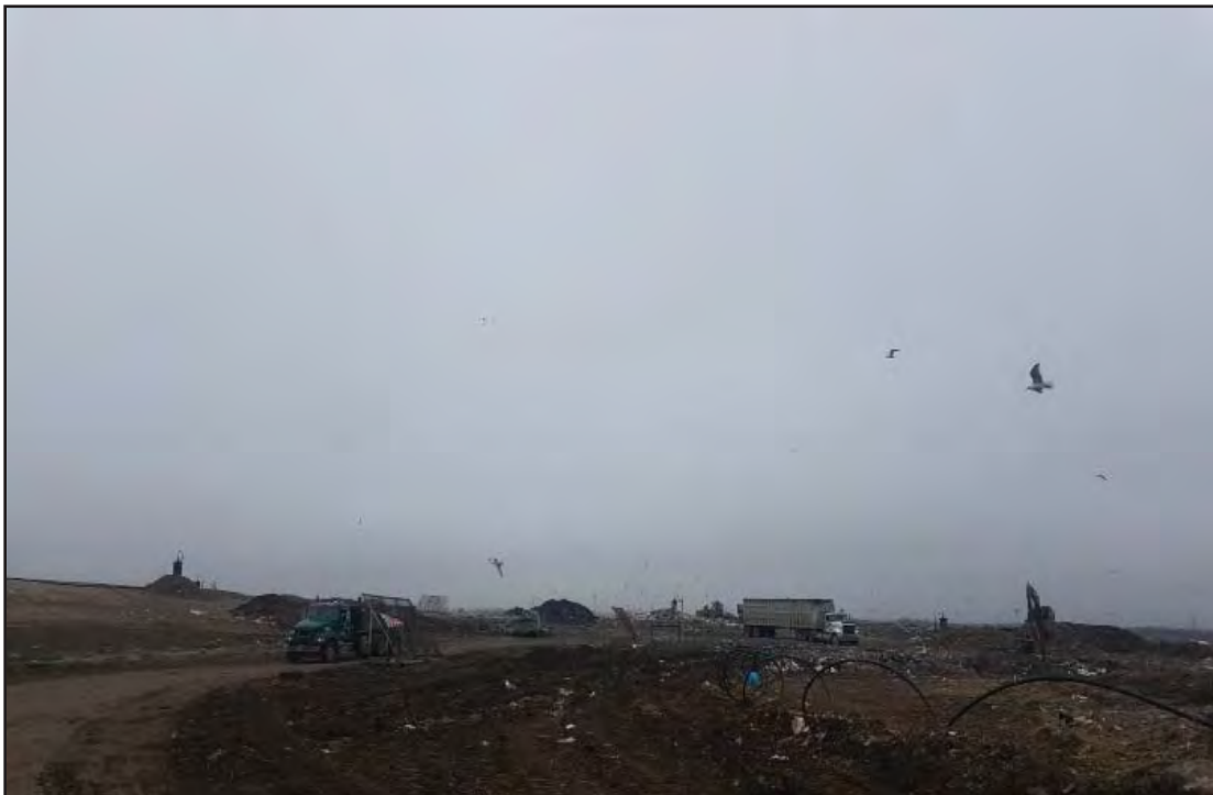
Overview of Phase 7 South
