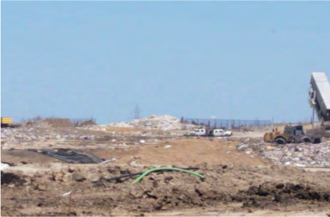
North Expansion West, (NEW), North of tipper covered with daily cover
