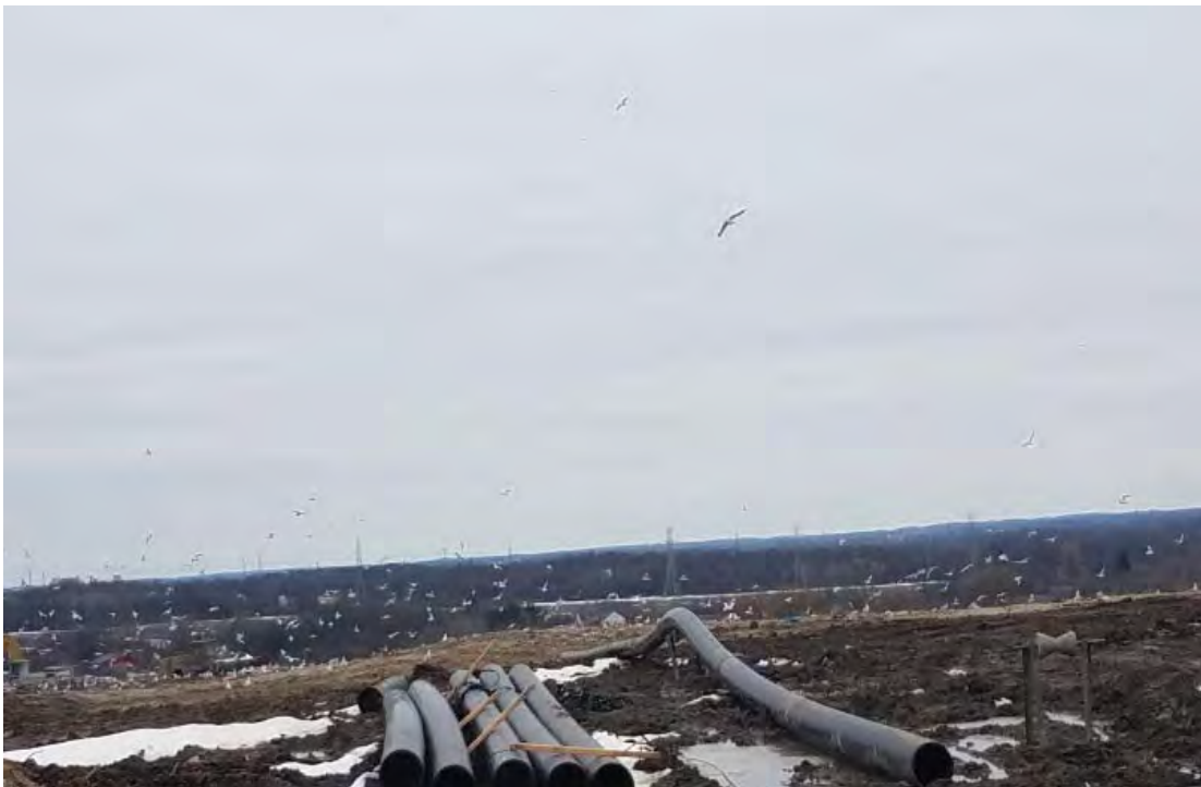
Phase 7 North, intermediate cover and pipe awaiting welding and use in gas collection system
