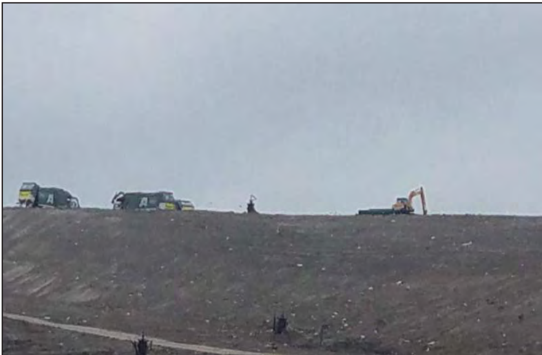
Phase 7 viewed from the West
