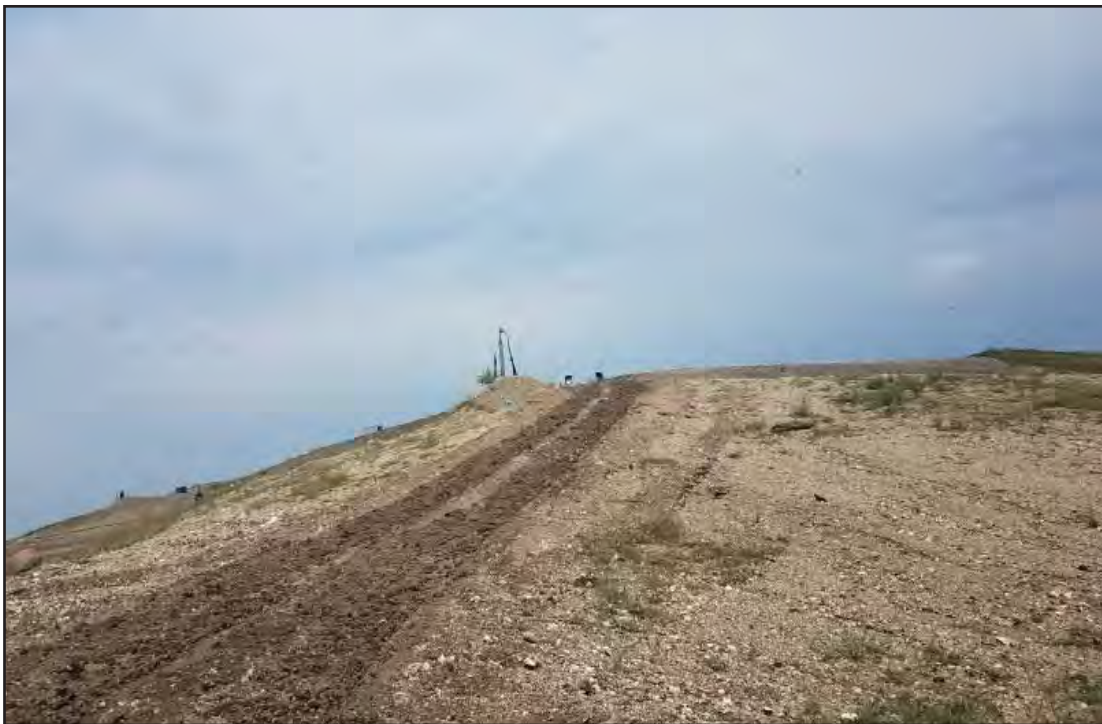
Southwest corner, South side of Phase 7 South. Heavy rutting by travel of gas techs
