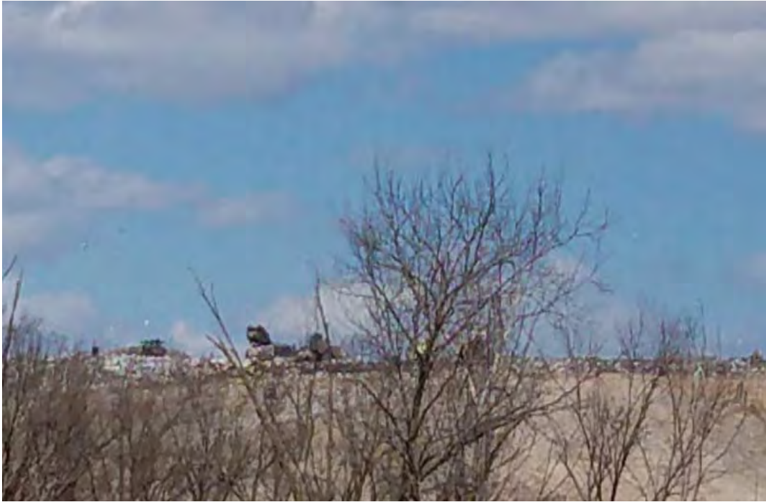
Working face on top of Phase 7 South
