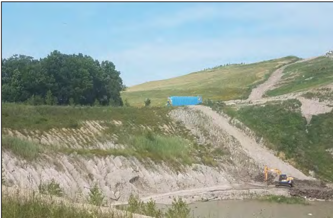
North slope out of temp sed basin, contaminated runoff pumped through filter tailer into tankers
