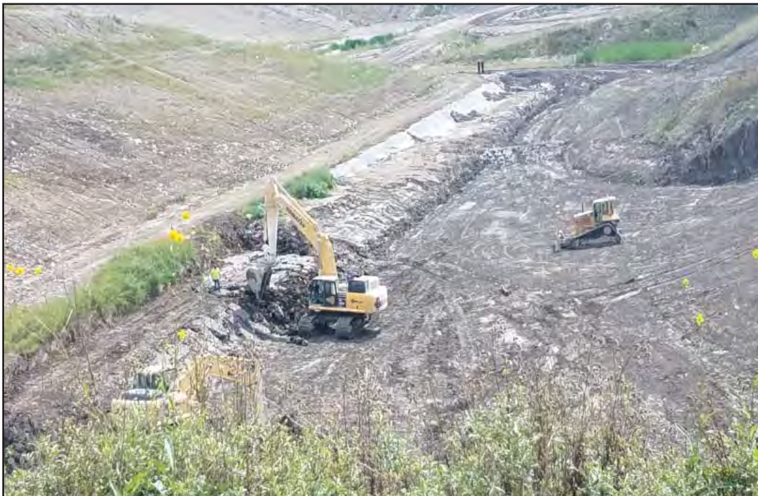
Excavator clearing rain flap to access seep
