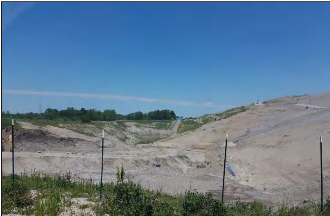
View North along West edge of Phase 7
