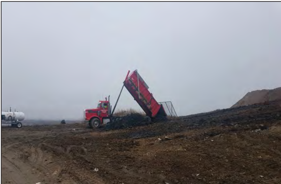
Soils tipping at North end of Phase 7
