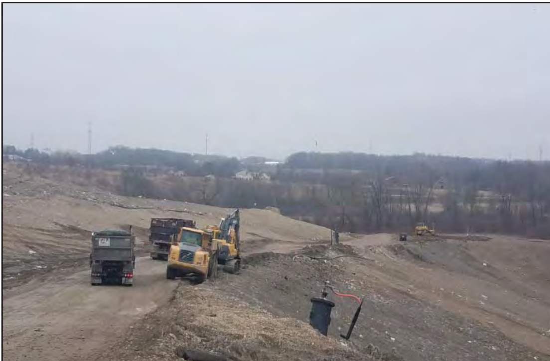
Installation of air line and force main by trenching and backfilling
