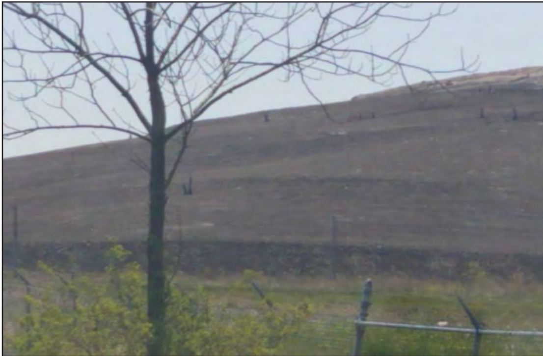
Cap development for Clearwater Pond Expansion
