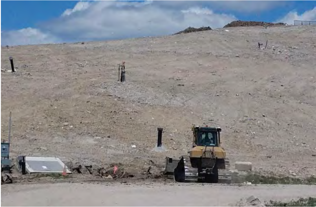
South toe of Phase 7 slope, pipe repair to left of dozer
