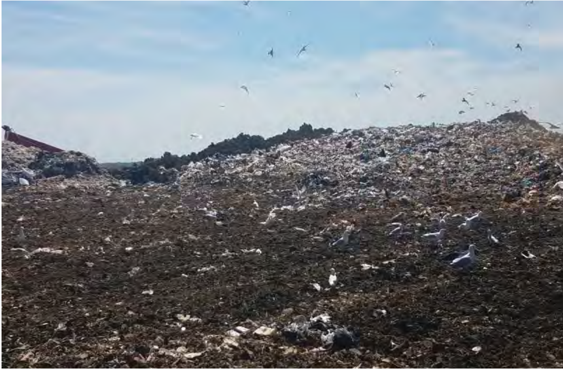
Working face, new lift starting at South end of Phase 7 South
