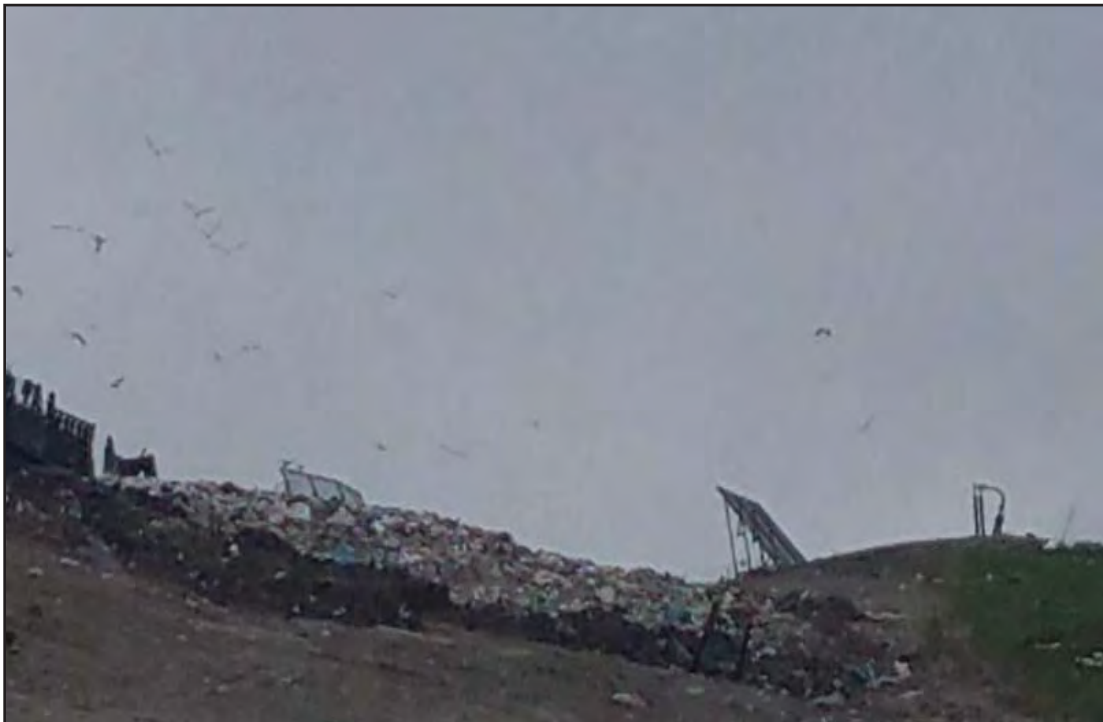
Working face at top of South slope at junction of Phase 6 & 7 South
