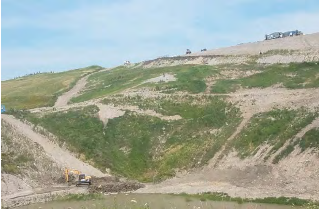
West slope above temp sed basin, excavator making repairs and access improvements
