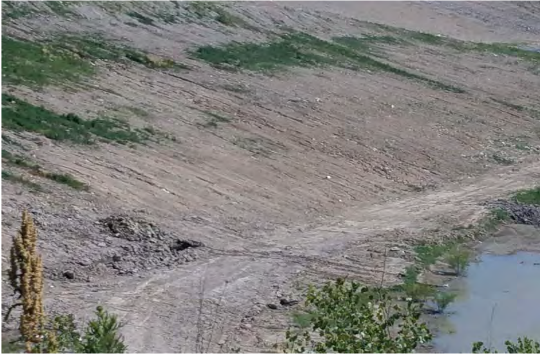
Seep in West slope, just above Temp sed basin. This is a re-accuring seep
