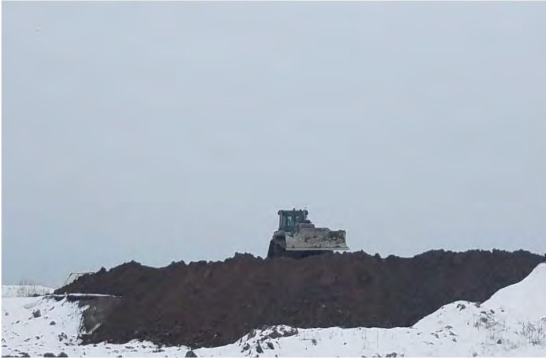
Tipped soil being stockpiled on Phase 3 for future use
