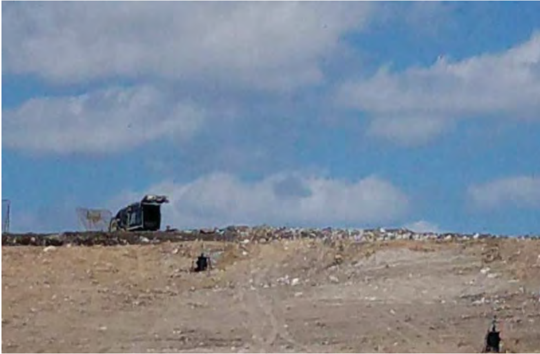
Previously placed waste, compacted and awaiting cover
