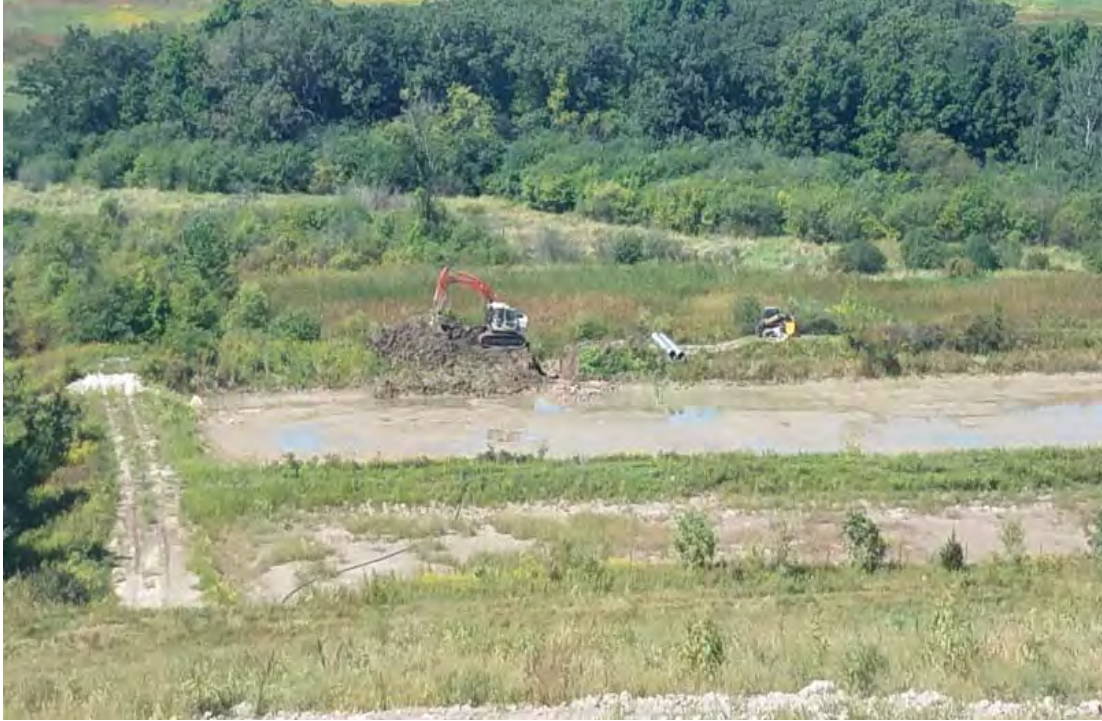
Construction of new outfall for Basin #1
