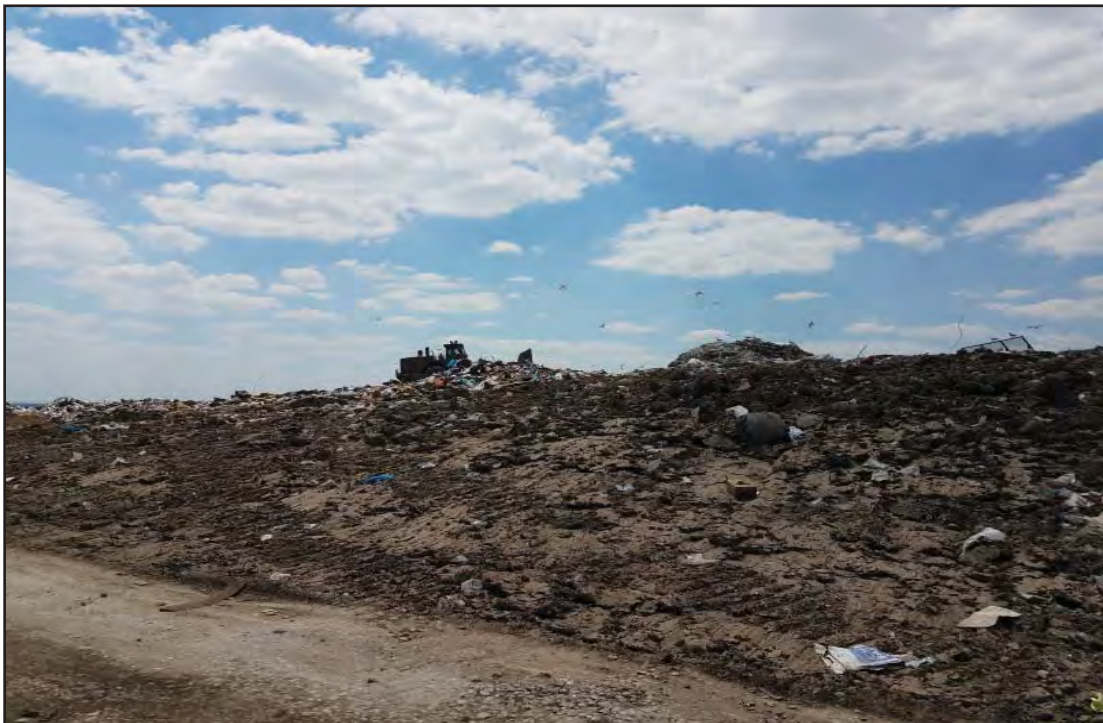
Working face between access road and top of slope, Phase 7 South
