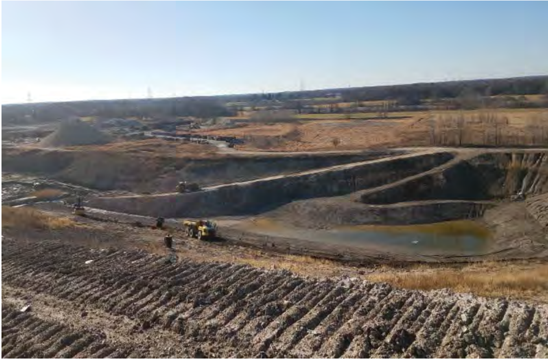
Temp sed basin restored
