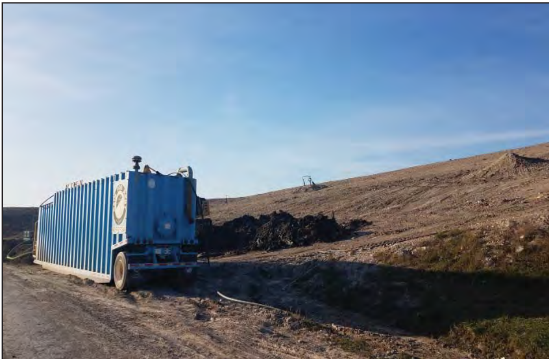
Drip leg work at North end of Phase 7 South, tanker not in use
