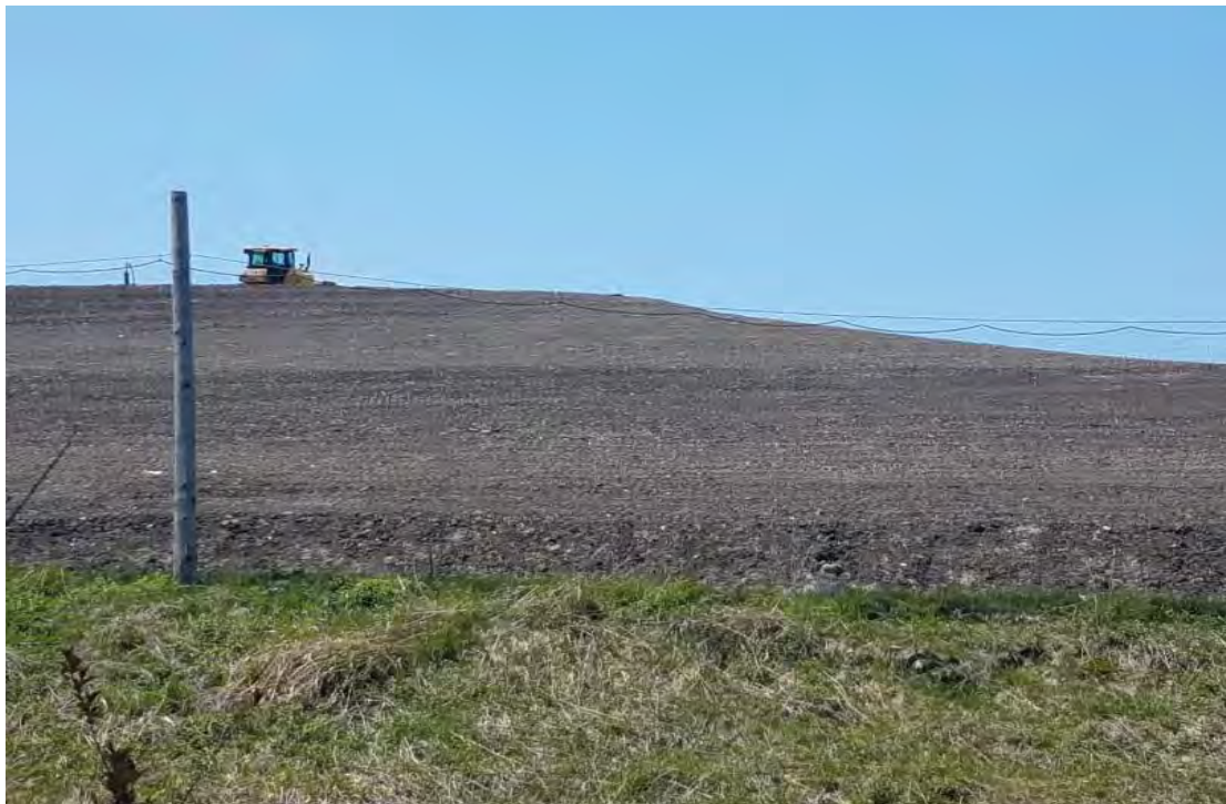
Cap development for Clearwater Pond Expansion
