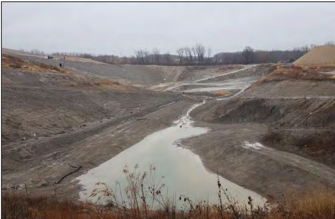
Temp sed basin viewed from the South, currently not pumping
