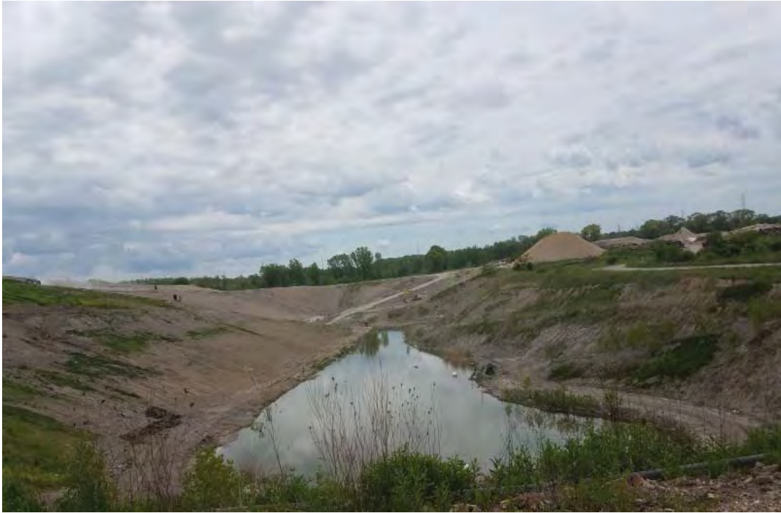
Temp sed basin viewed from the North, closed off at the South end until cleaned and graded
