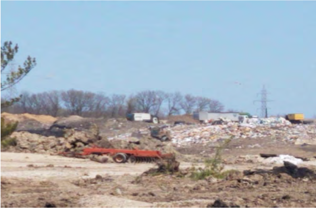
Tipped waste being pushed down into Phase 2
