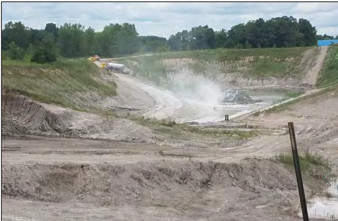
Temp Sed Basin receiving Lye to solidify basin for cleaning
