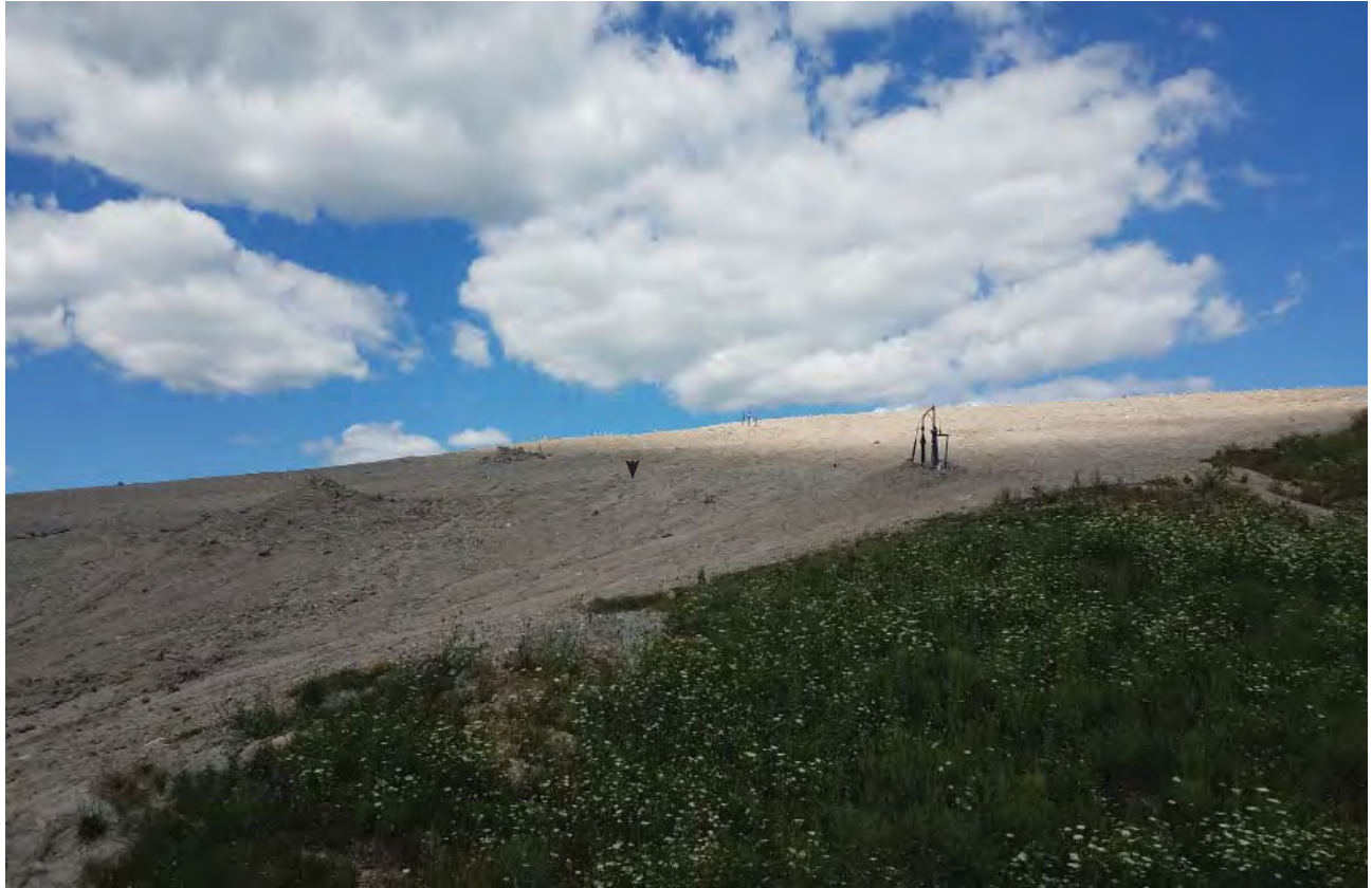
South slope Phase 7 South
