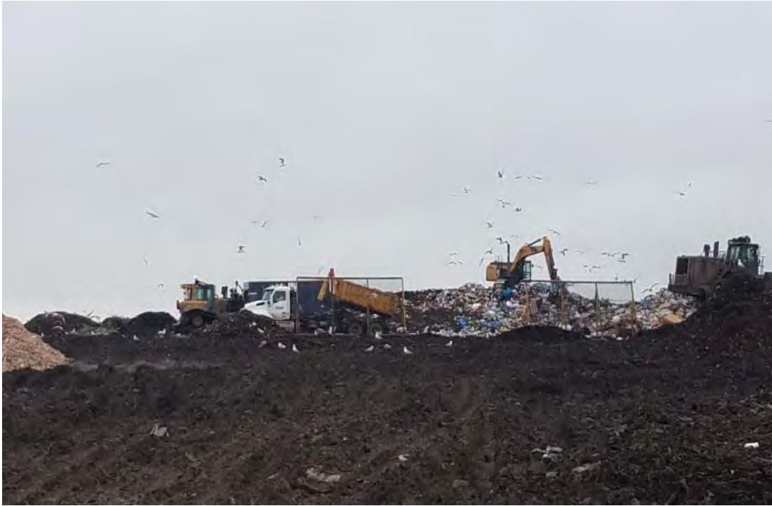
Working face, lift developing on West edge of Phase 7 South
