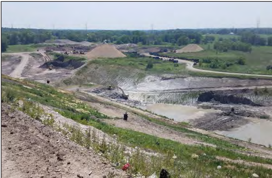
Temp sed basin being separated to manage leachate contamination
