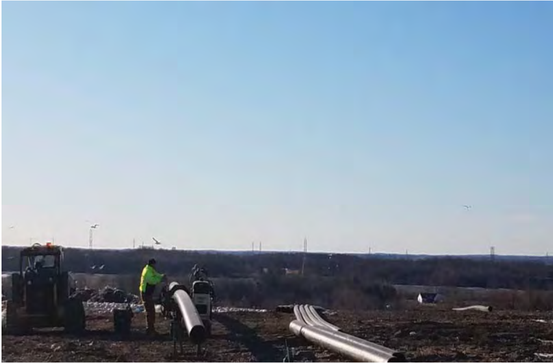
12" HDPE pipe welding, ongoing, to connect gas system to wells
