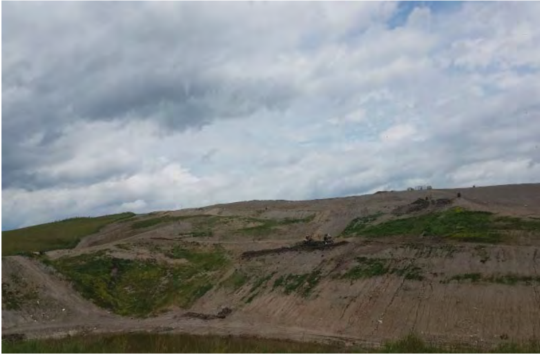
West slope of Phase 7 North, some seep repairs evident
