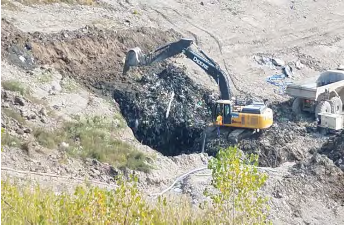
Sump at Northwest Corner of Phase 7 South, being investigated for issues. Excavation to bottom of cell will be a potential odor source
