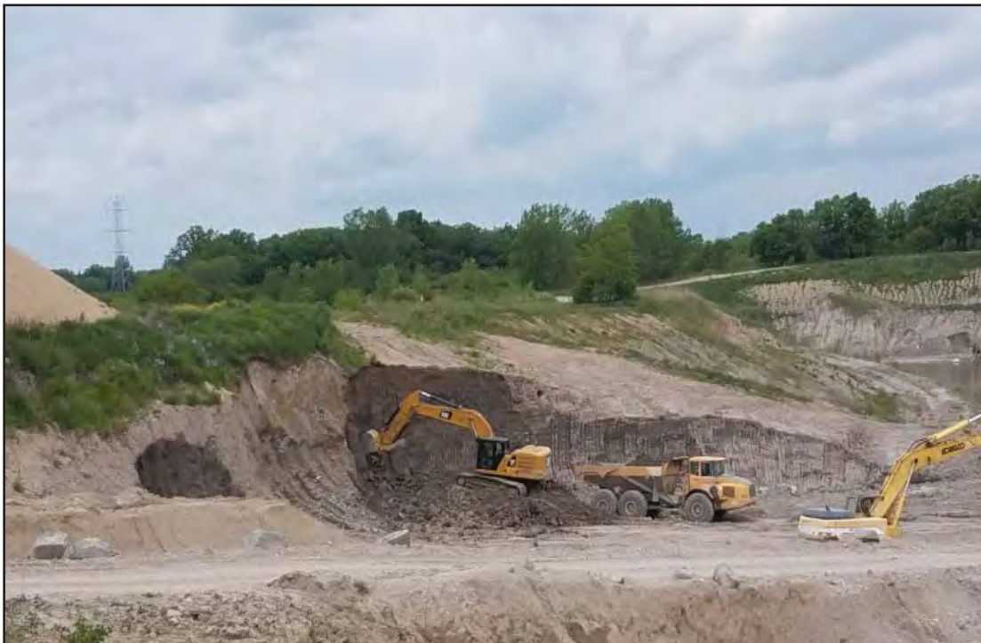
Excavation of future Phase 8, soil being used in seep repairs
