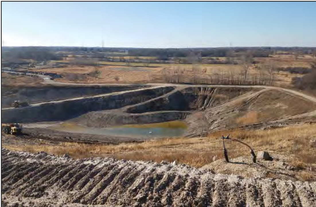
Temp sed basin pumping to clear water to basin #1
