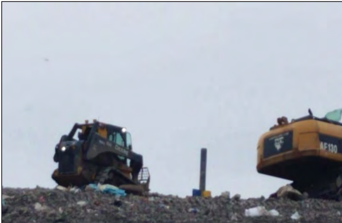
New well, last well to drill, being installed near Southwest corner of Phase 7 South
