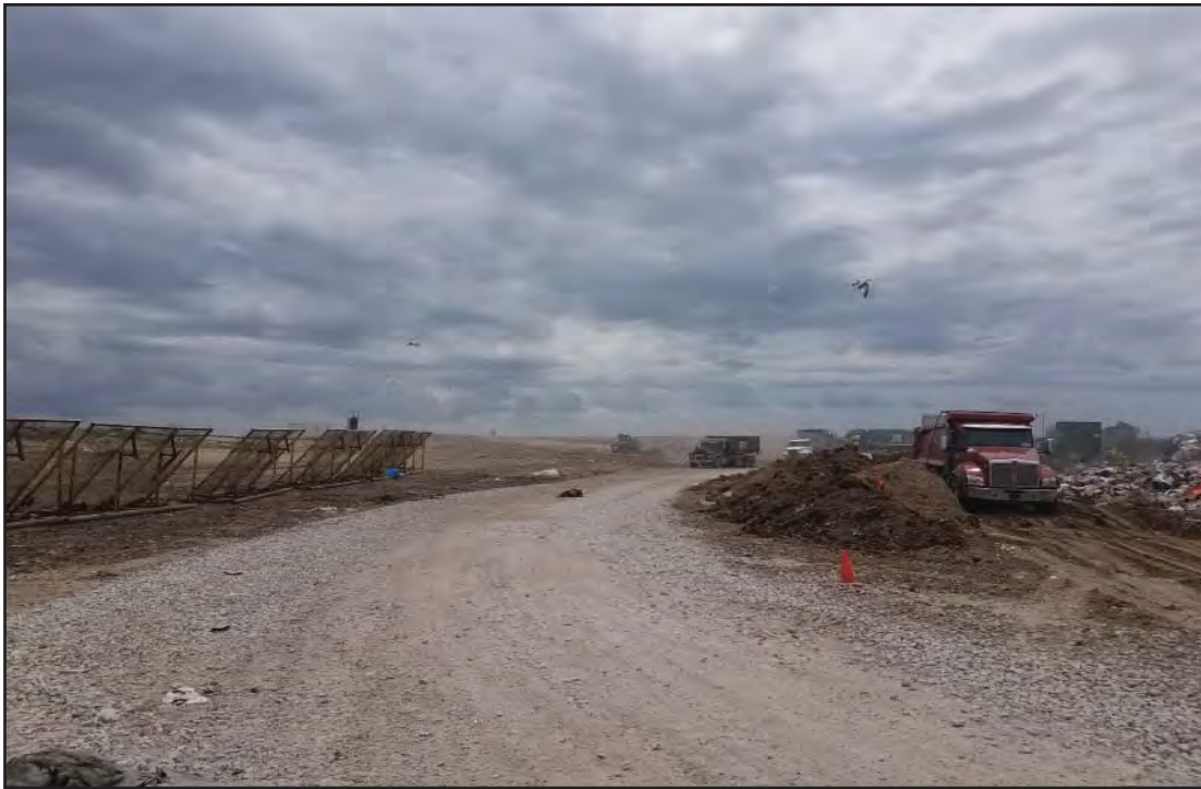
Working face and access to previous faces
