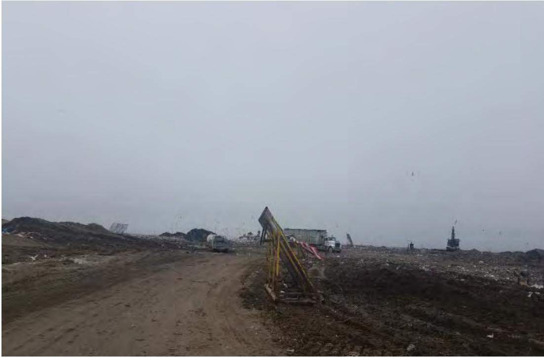
Working face and approach in Phase 7 South
