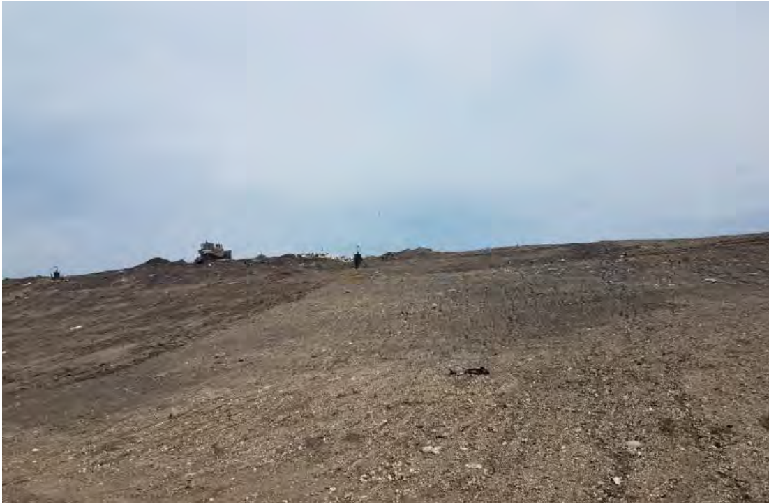
Temp sed basin being solidified and material removed
