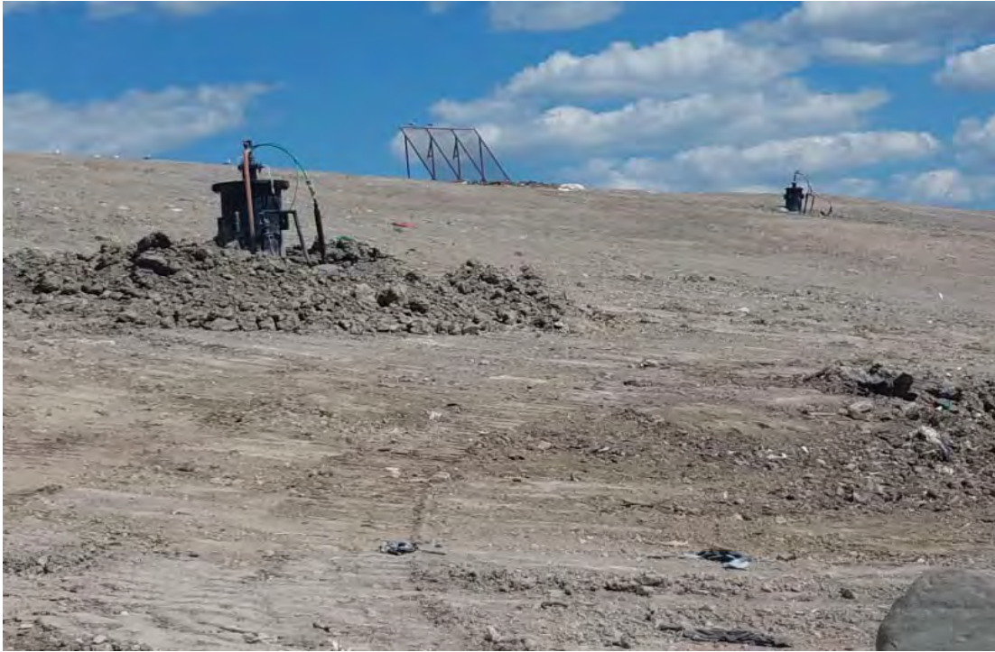
Bentonite and clay sealing about well heads
