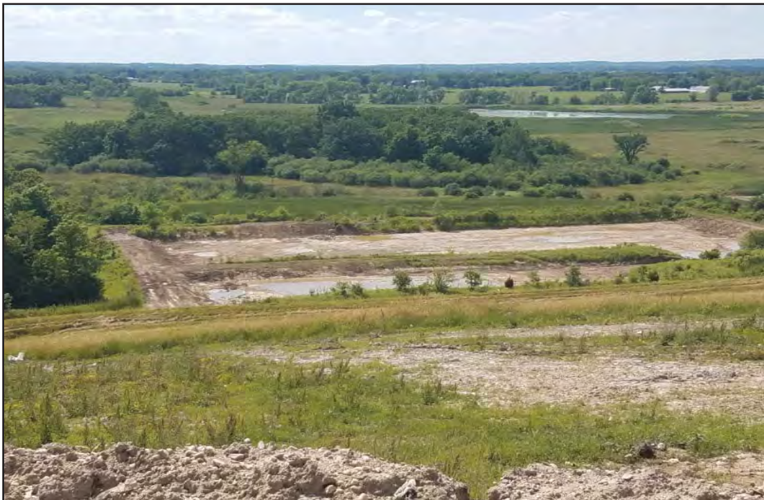
Work in cleaning and restoring basin #1 complete
