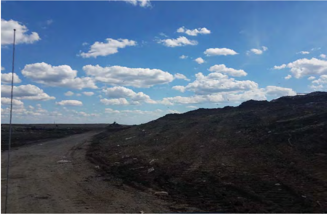
Access road up to Phase 7, area of recurring odors
