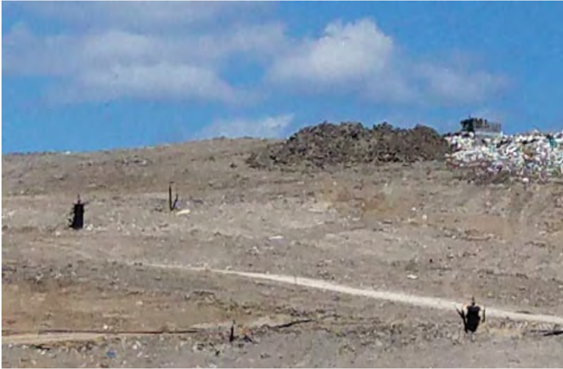
Stockpiled cover soils
