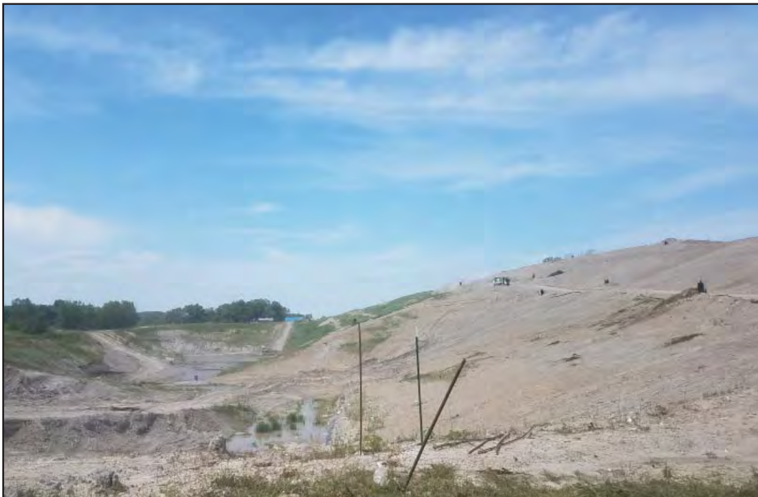
West slope of Phase 7 viewed from the South
