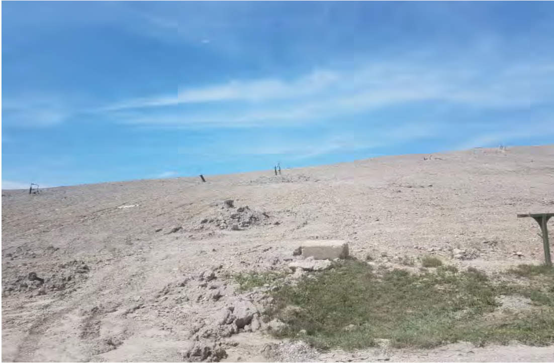
West edge of South slope of Phase 7 South
