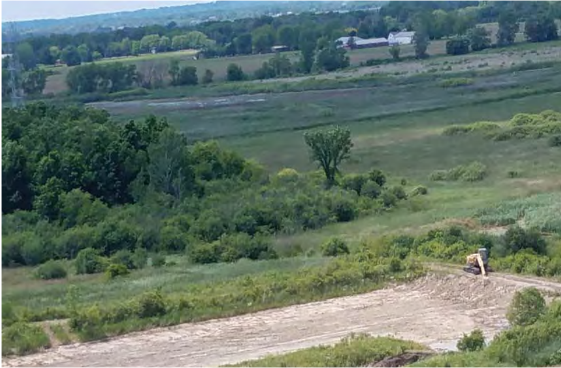
Basin #1 cleaned and restored
