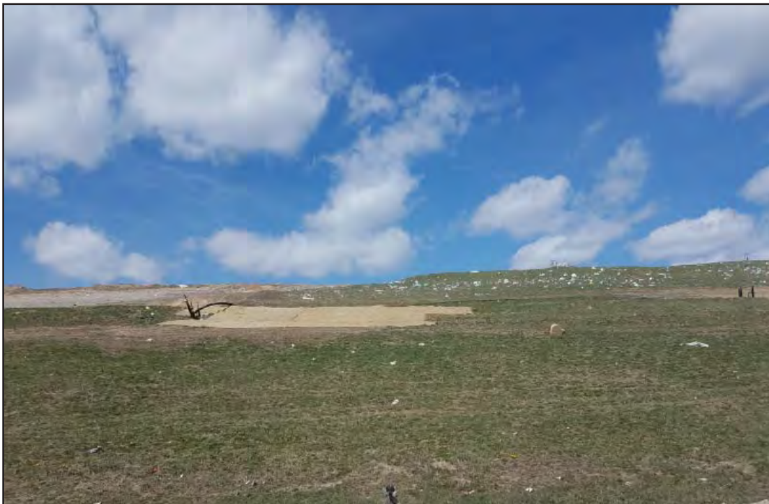
Upper slope of Phase 5/6 South slope
