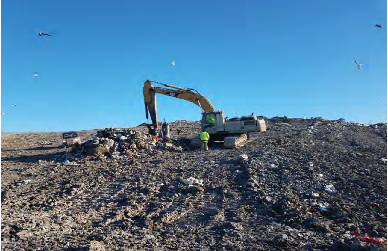
Site employees investigating location of possible oxygen intrusion to gas collection system
