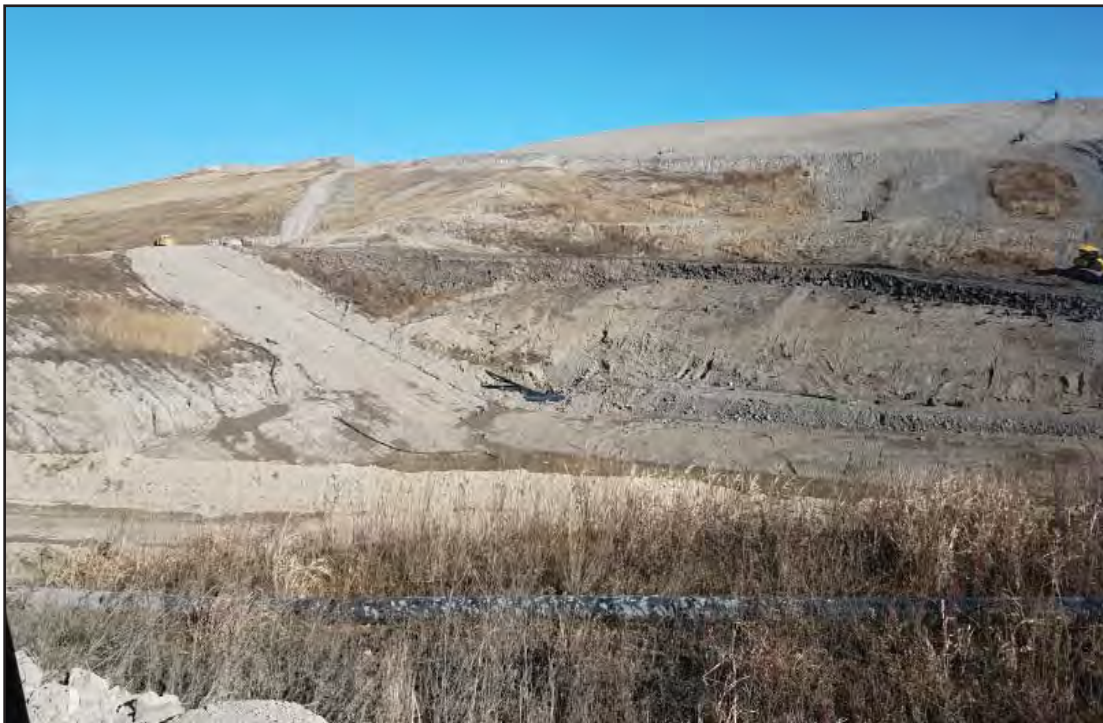
West slope of Phase 7, note new berm construction to move runoff from North to South
