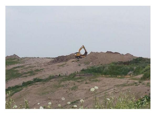
Excavator actively removing cover soils to allow placement of waste in Phase 6&7. Cover depth is excessive making excavation lengthy.
