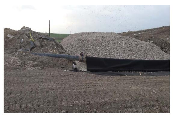
East end of overlay construction. Drainage layer will be approximately 18' at this end to adequately drain and collect leachate.
