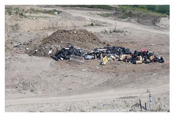
Abestos tipped in Phase 6, materials should be carefully handled, barrels should be set on end, not on their sides. Asbestos was covered before the end of the audit.
