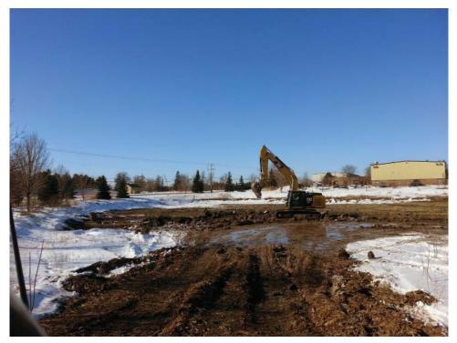
Excavator cleaning bottom of sedimentation basin
