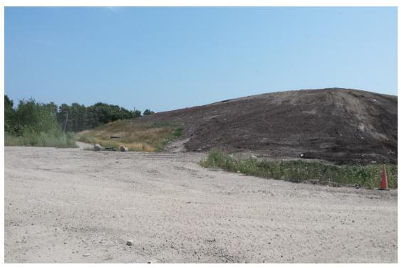
North slope of Phase 8, intermediate cover with topsoil and now seeded
