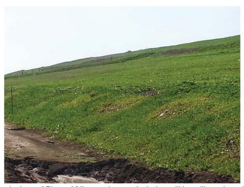
South slope of Phase 6&7, greening up nicely, but still has rill repairs to be done.
