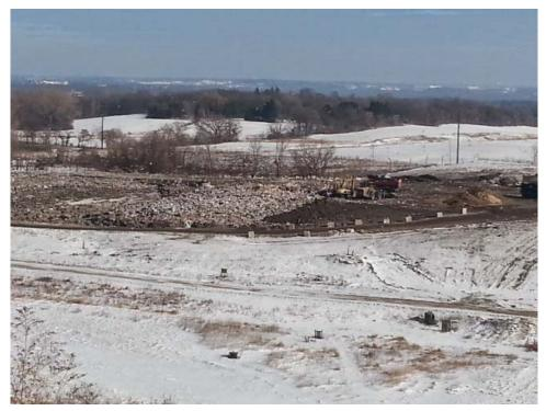
Working face, previous days cover on right in good condition, previous cover on left in poor condition
