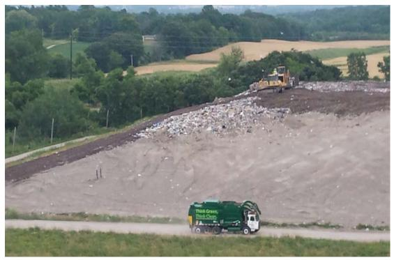
Working face on Northwest corner of Phase 9, receiving cover soils. Previously covered by tarps
