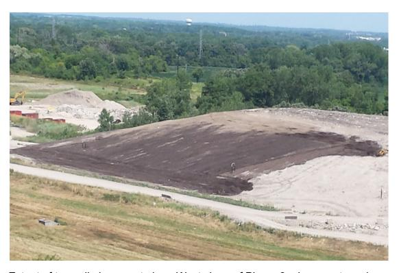
Extent of top soil placement along West slope of Phase 9, placement moving from North to South
