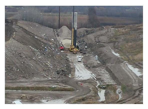
Additional stone in place for sideslope rise placement. Piping system being installed in and around man hole
