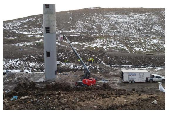
Liner material being spray appllied to manhole
