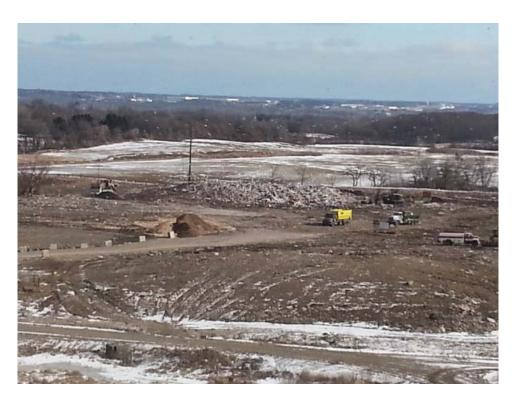
Working face in Northeast corner, waste being pushed up to create new lift
