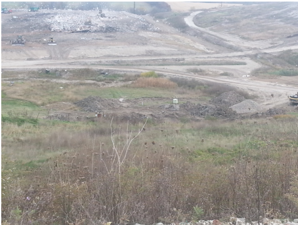
Location on East slope of old hill that the Oxygen leak was discovered and repaired.
