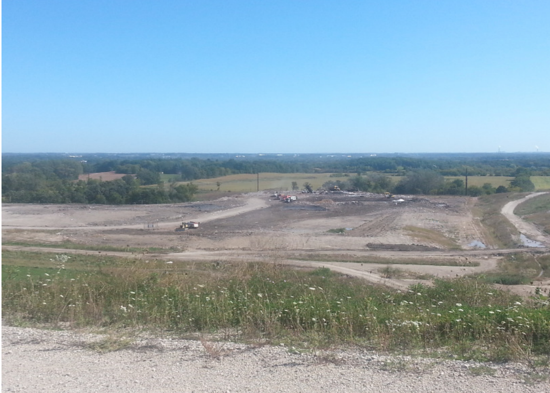
Phase 9 viewed from the West
