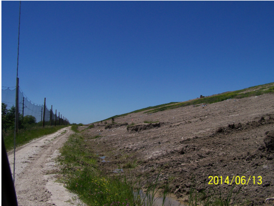
Cleaned ditch line along South slope of Phase 6 & 7
