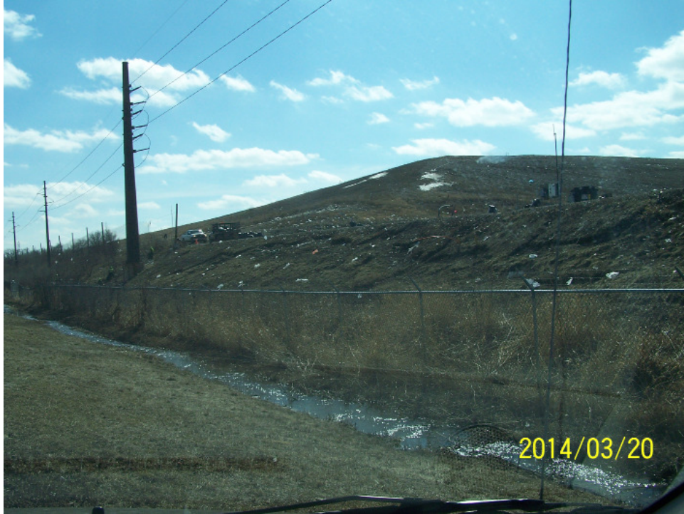
East slope of Phase 9, severe erosion and some litter
