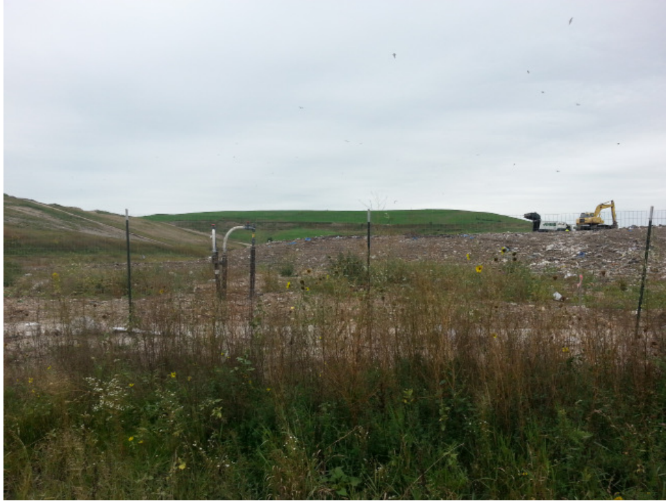
Active area viewed from the East, Phase 9
