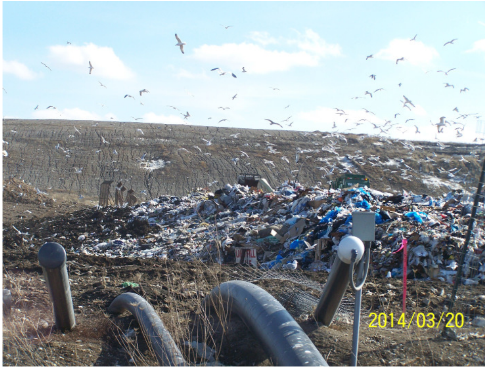
Leading edge of working face
