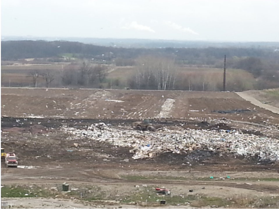
Daily cover well placed East of Working face
