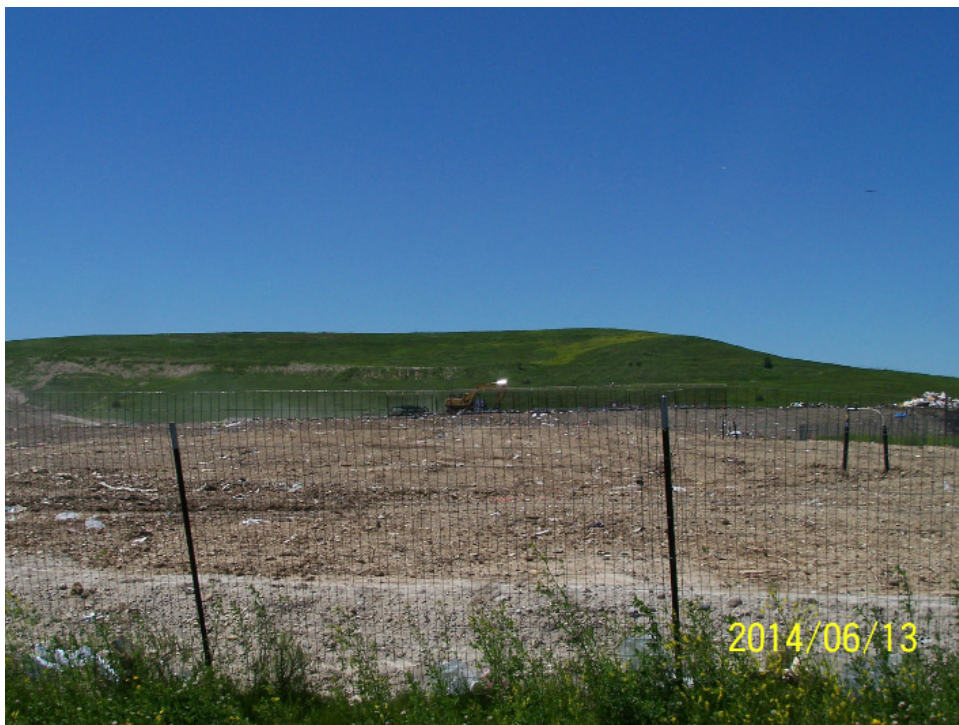
Active area viewed from the East
