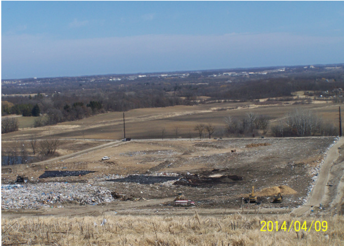
Phase 9, East slope, eroded from last year.
