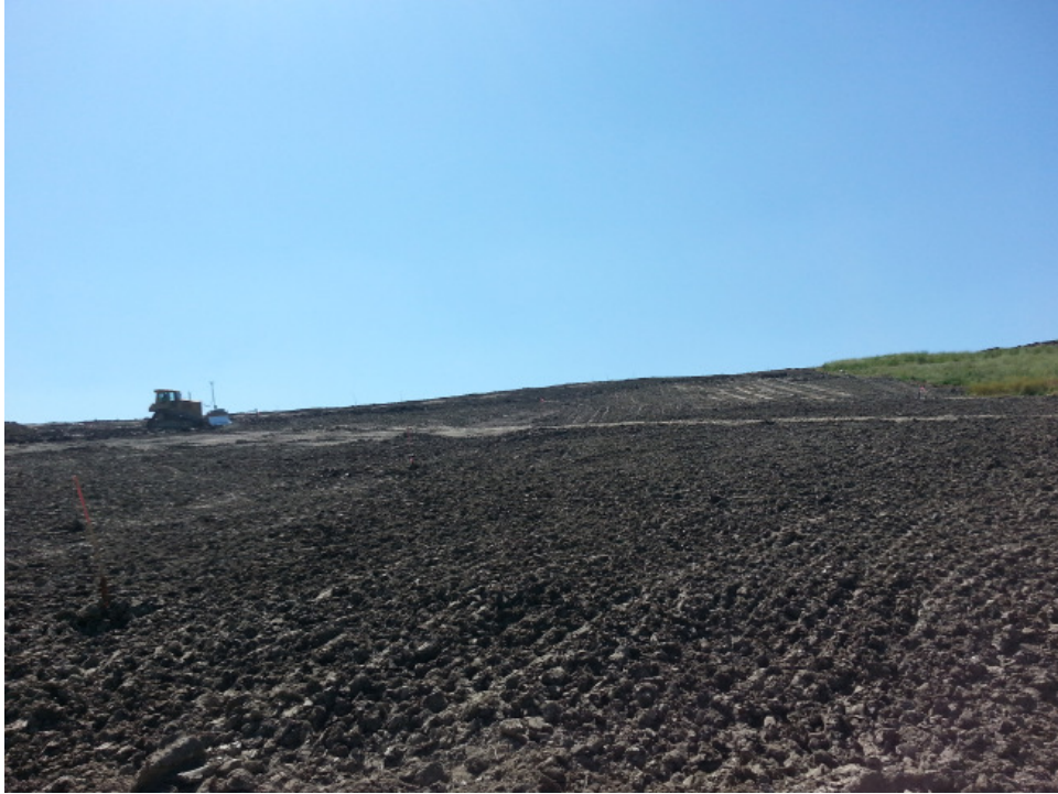
East slope of Phase 7, nearly finished with clay placement. Next stage is gas well sampling
