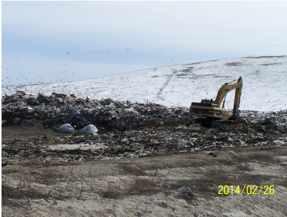
Working face in Phase 9
