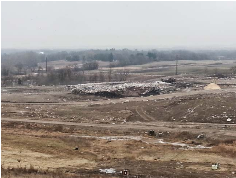
Working face in Northeast corner of Active area, Phase 9
