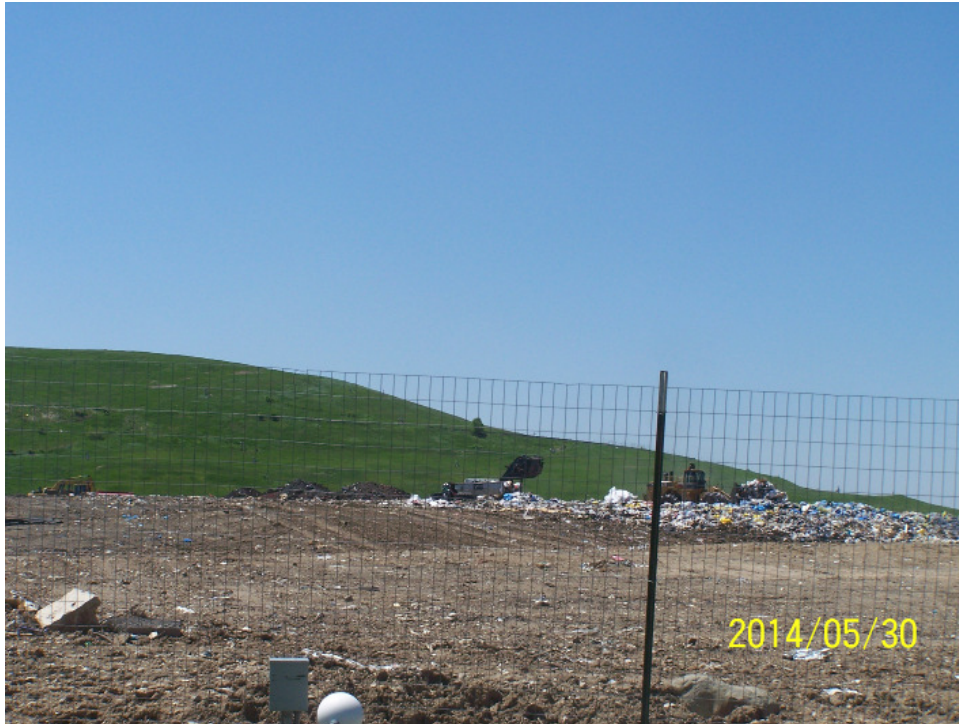
Working face in Phase 9, along North boundary
