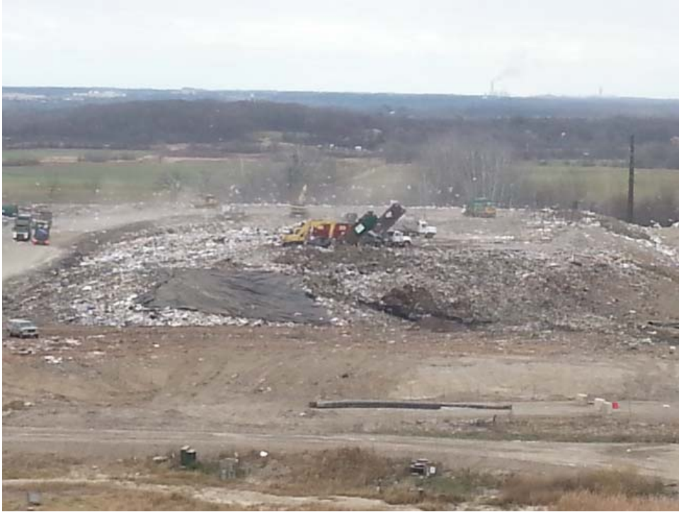
Working face with previous day's faces open about it, with poor tarp coverage
