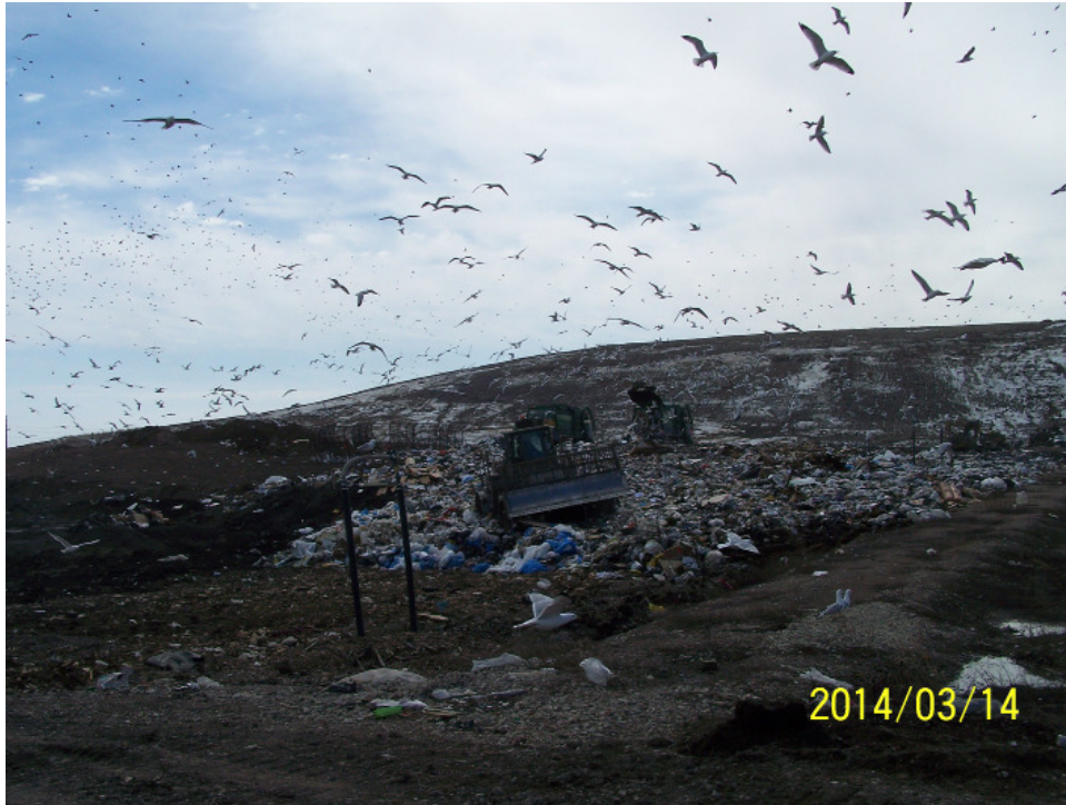
Working face in Phase 9
