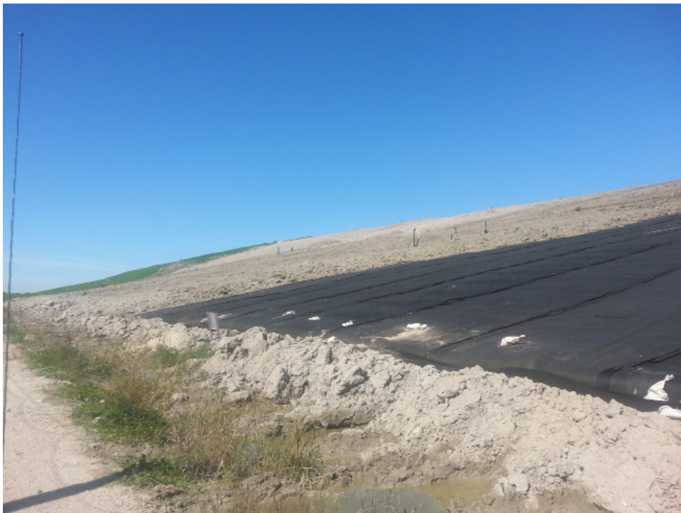
South slope of Phase 6, very little work done on soil placement for the cap since last audit
