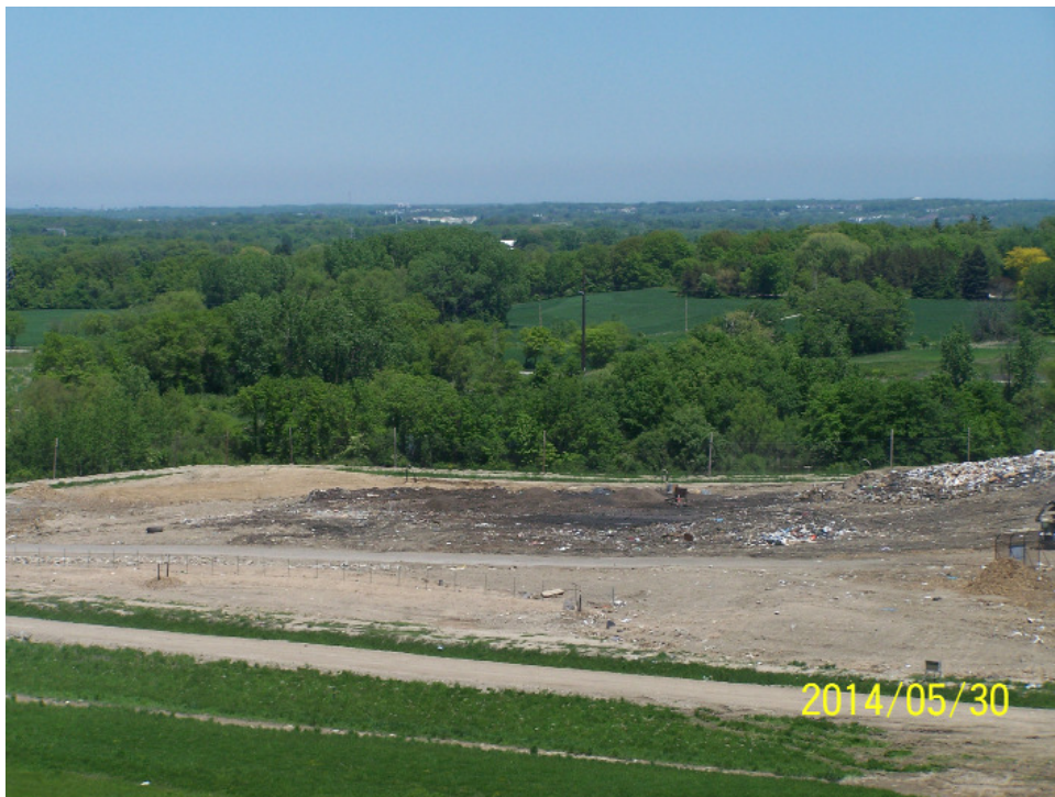
North end of Phase 9
