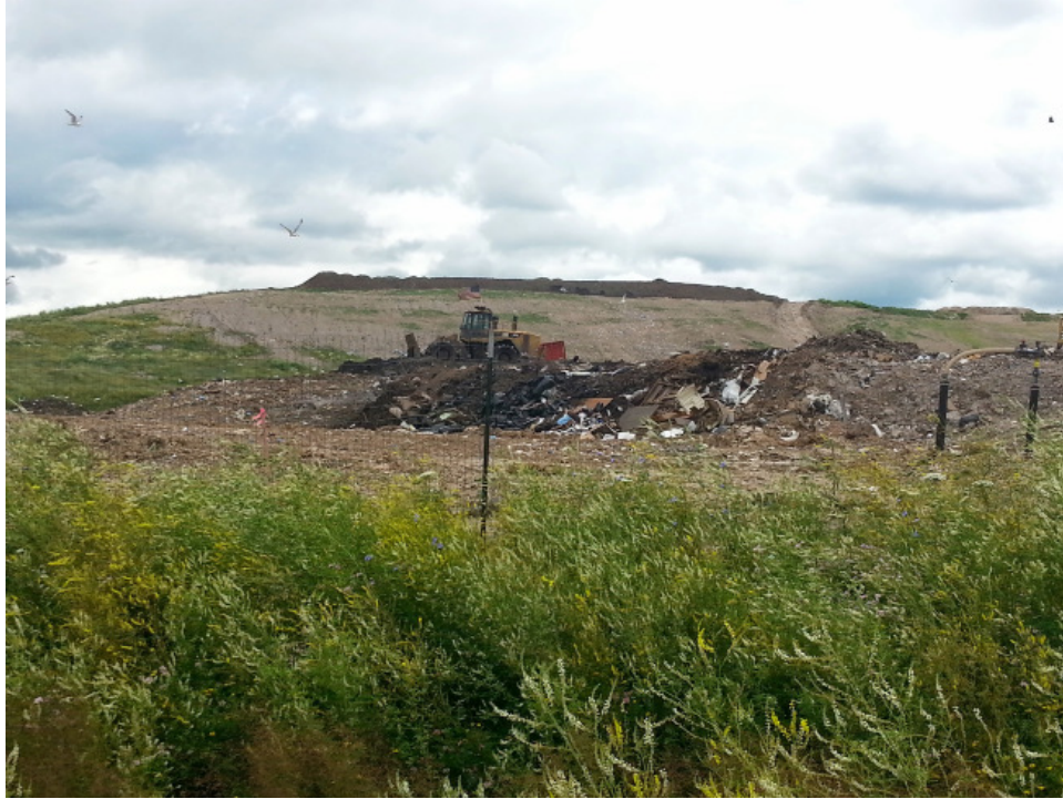
Active area viewed from the North
