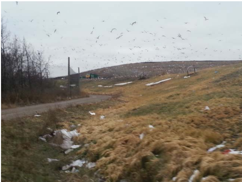
Phase 9 seeded side slope
