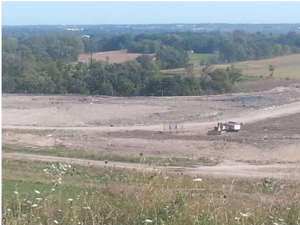
Intermediate cover placed on Northern half of Phase 9
