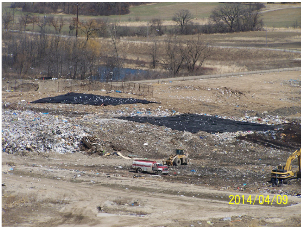
Tarps prepared for placement over working face
