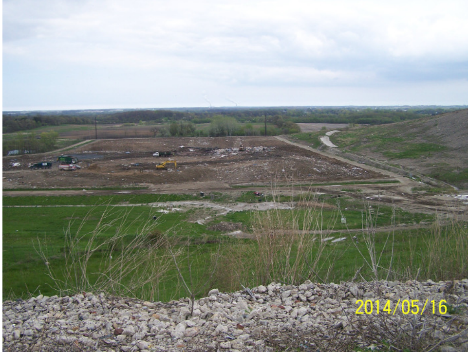
Daily cover well placed
