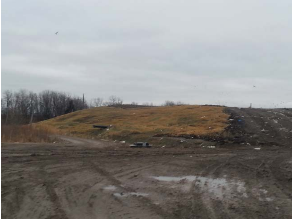
Phase 9 seeded side slope
