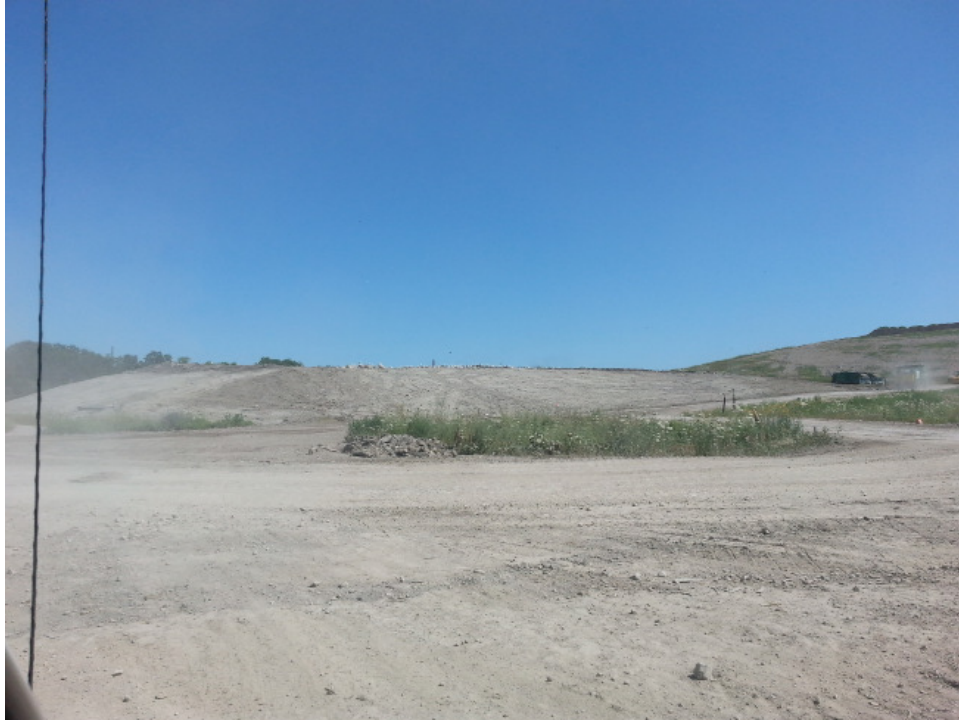
North end of Phase 9
