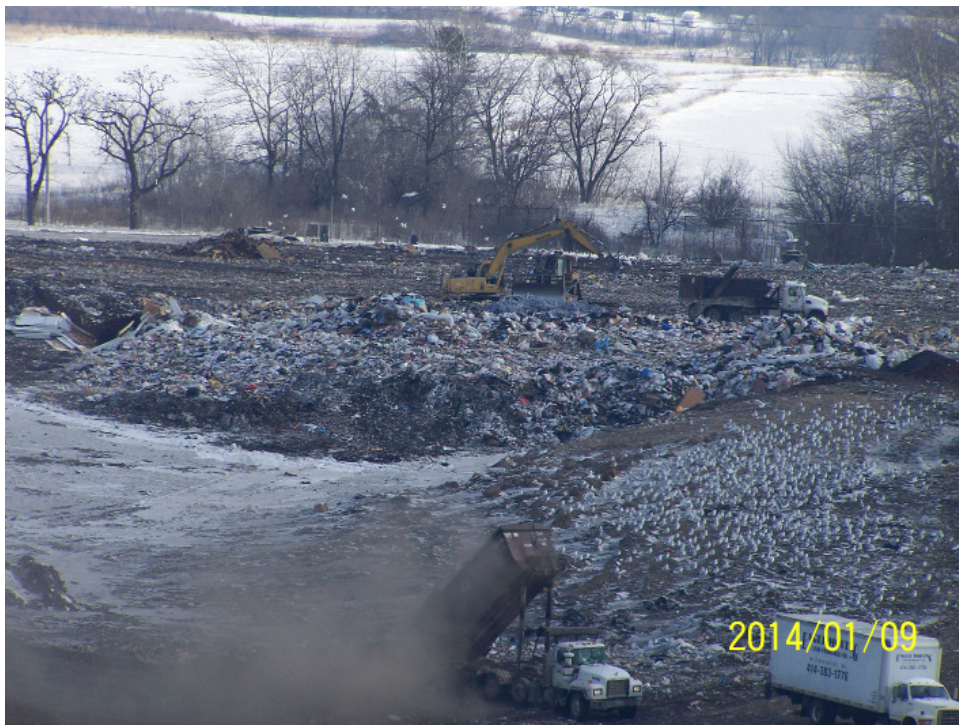
Working face, midpoint of Eastern edge of cell
