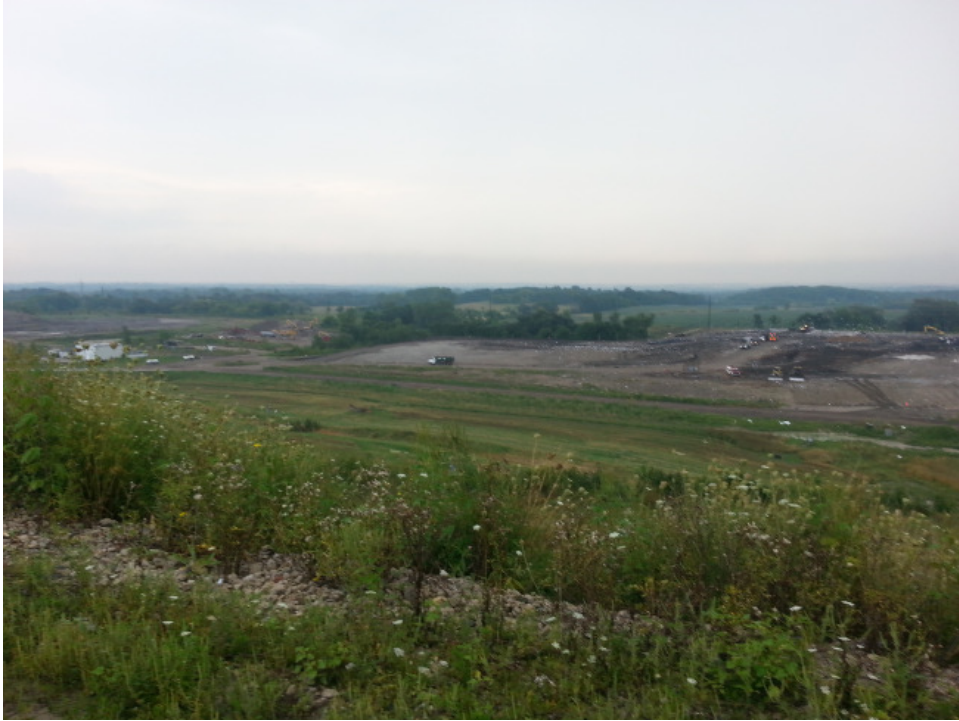
Daily cover in good condition on North end of Phase 9
