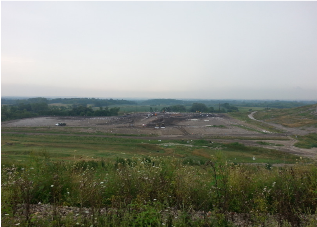
Phase 9 viewed from the West
