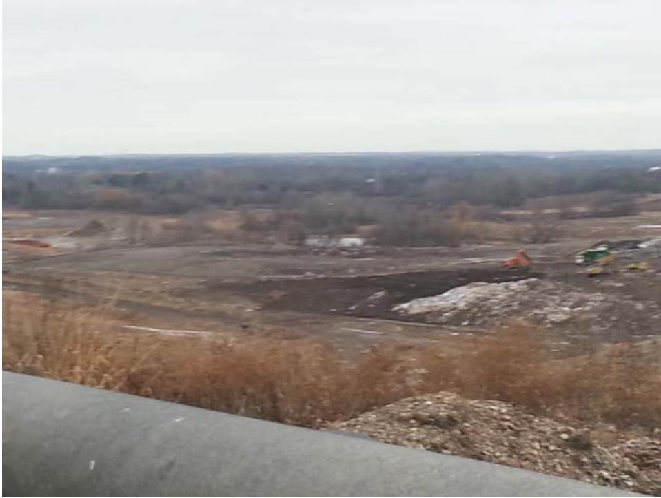
Soil being placed over previous days cover
