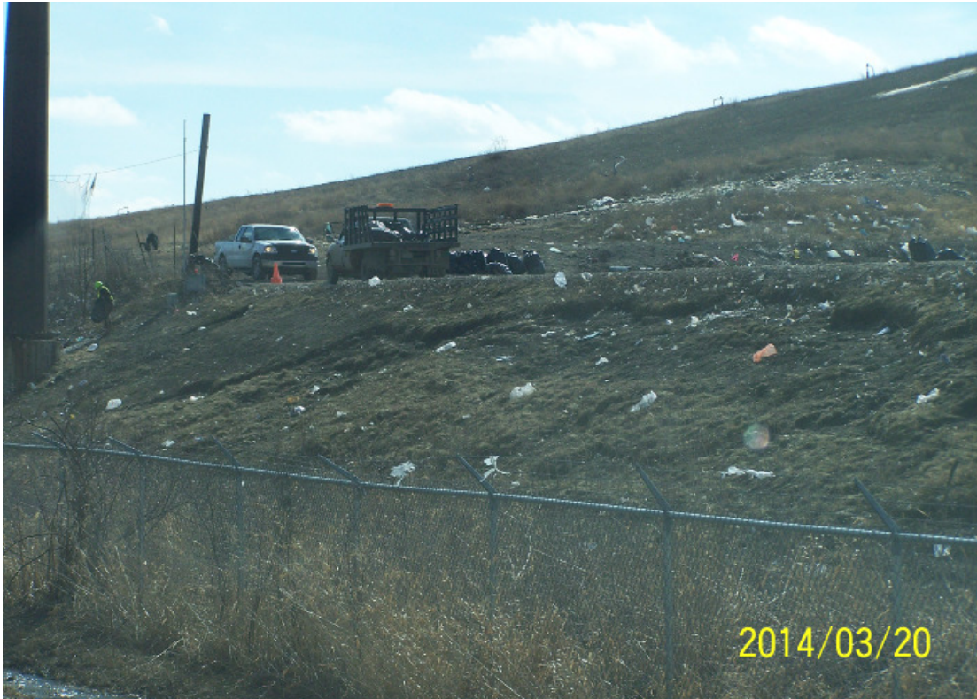
Phase 9, East slope, eroded from last year.
