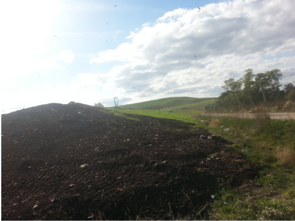
Top soil placed on Phase 9 Northeast corner expected to be seeded this week.
