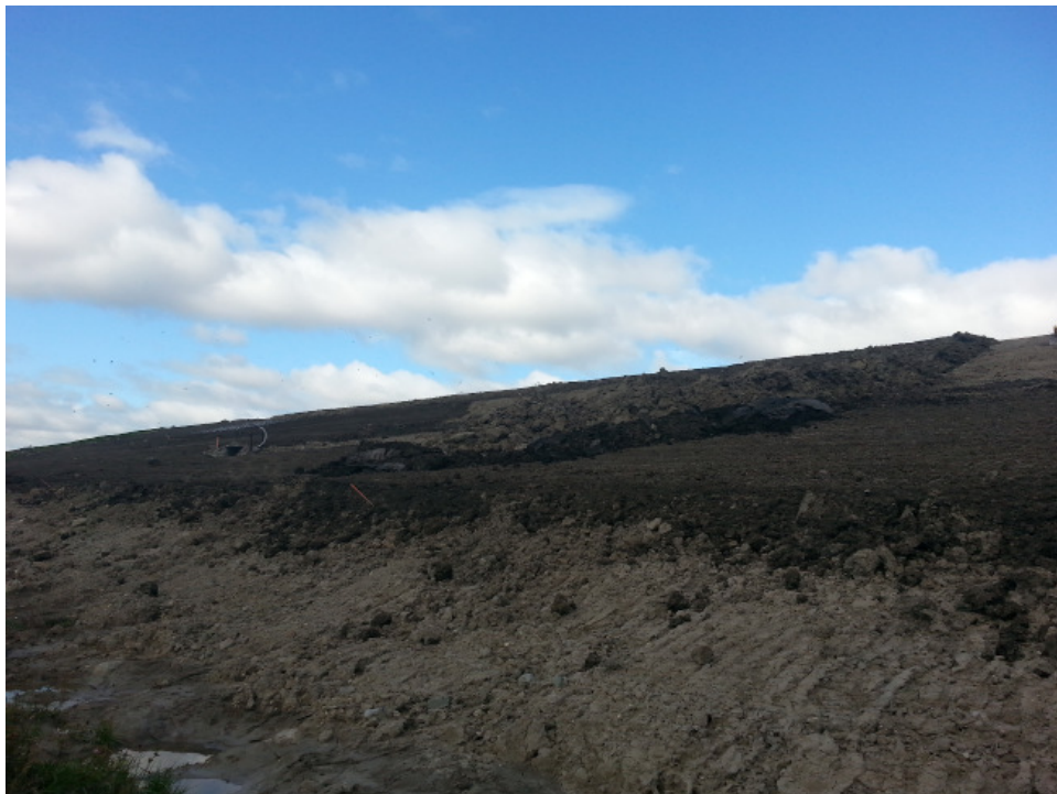
Top soil placed on cap around diversion berm, topsoil will be spread on berm when construction completed
