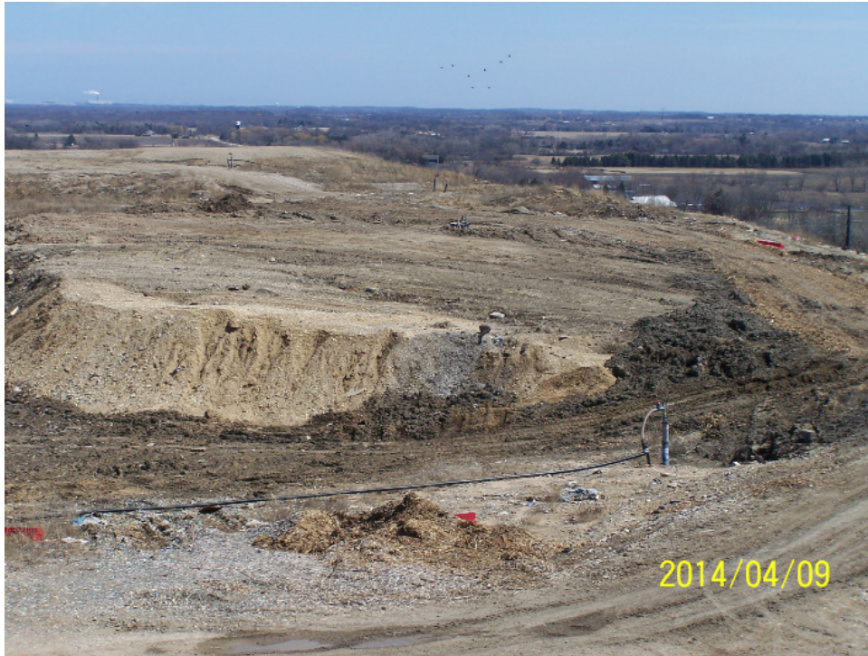
Gas header installation
