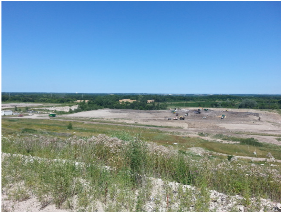
Phase 9 viewed from West
