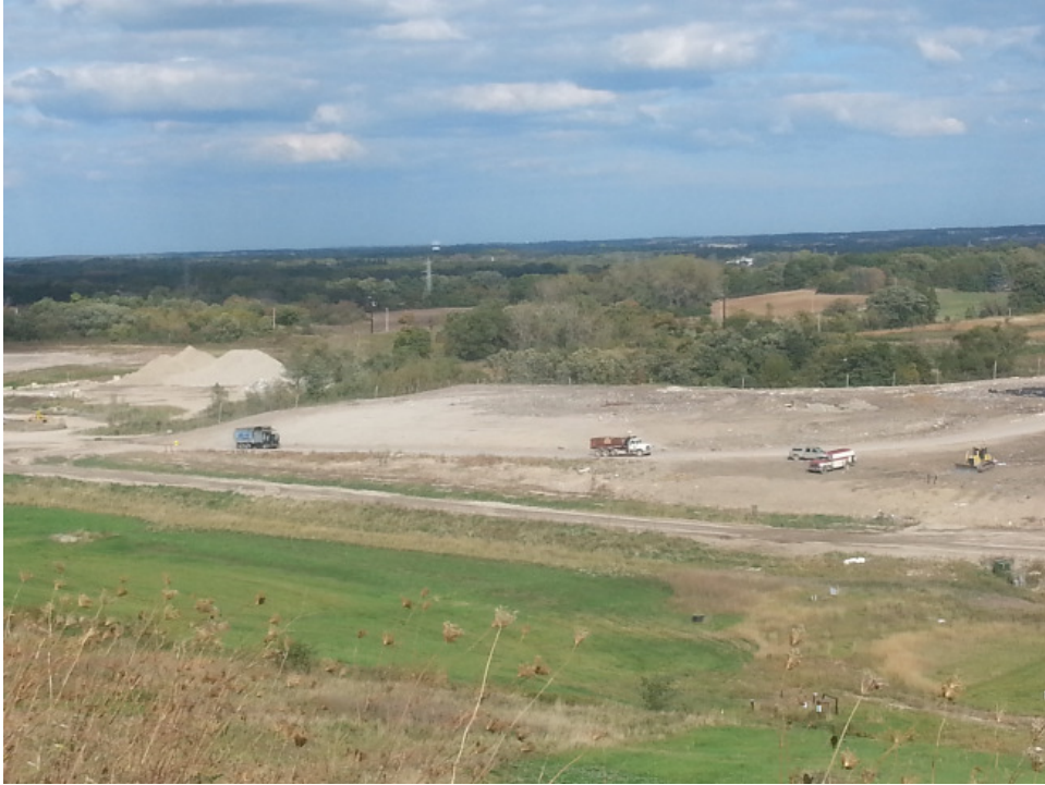
North half of Phase 9, covered with intermediate cover
