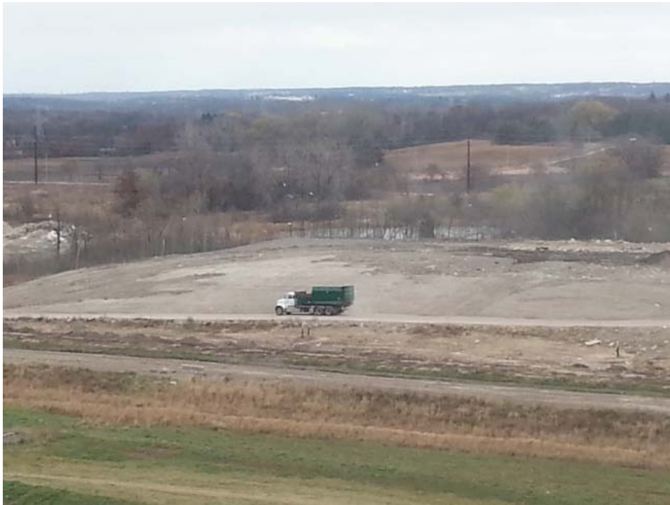
North end of Phase 9, intermediate cover in good shape
