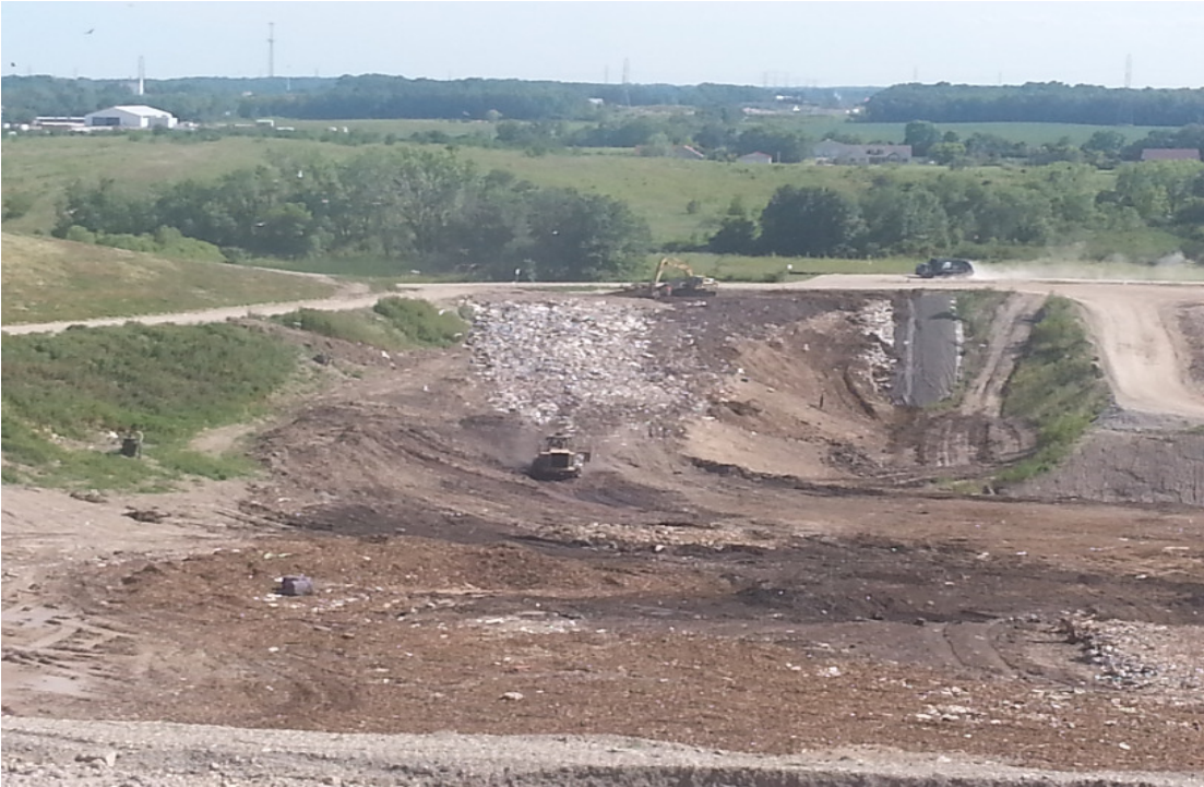
Working face along Phase 6, West Slope
