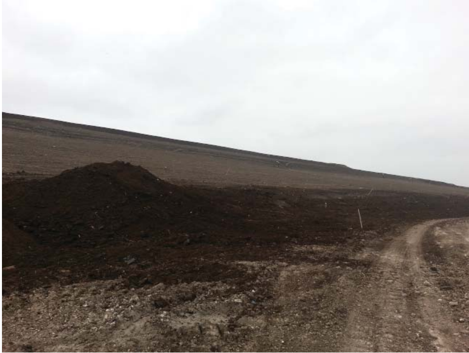
Final cover placement in Phase 6 & 7 South Slope
