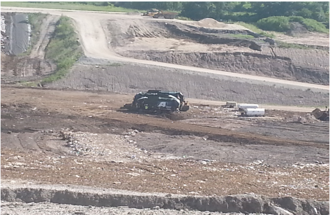
Active Area in Phase 7B West, select fluff waste only.
