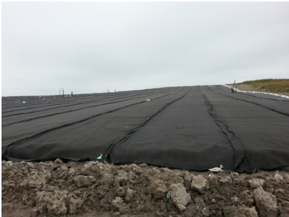
West Slope of Phase 7, capped with geomembrane and geocomposite
