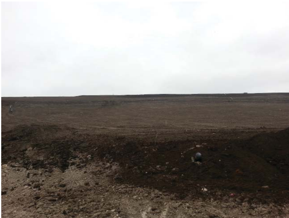
Final cover placement in Phase 6 & 7 South Slope
