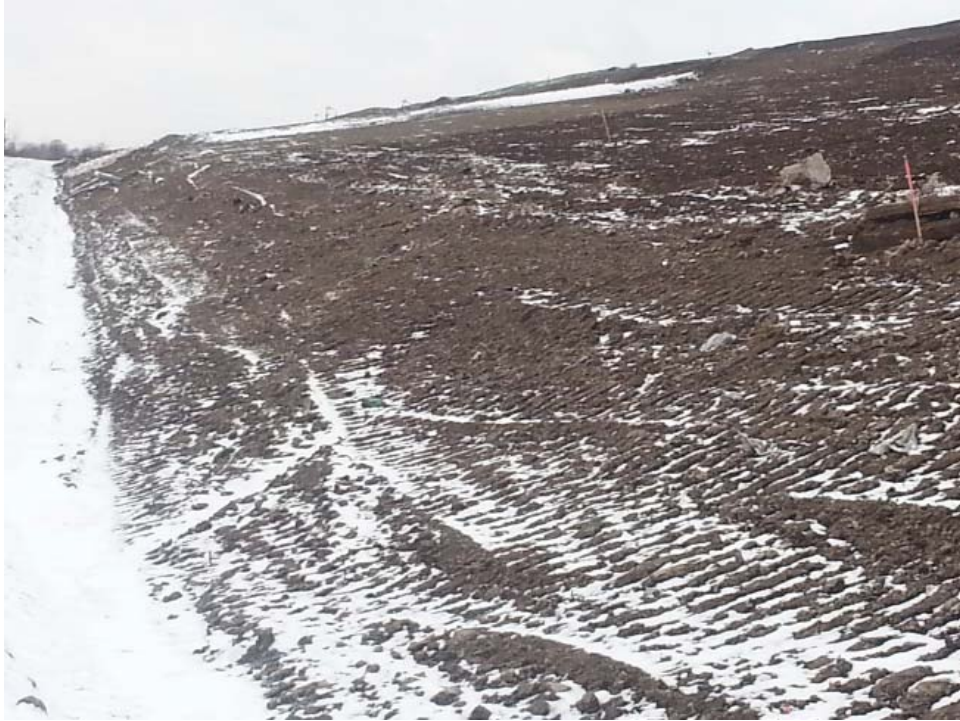
Final cover/cap system, East slope
