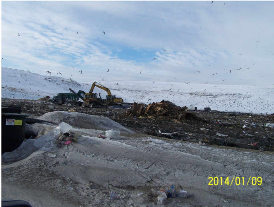
Excavator managing frozen load
