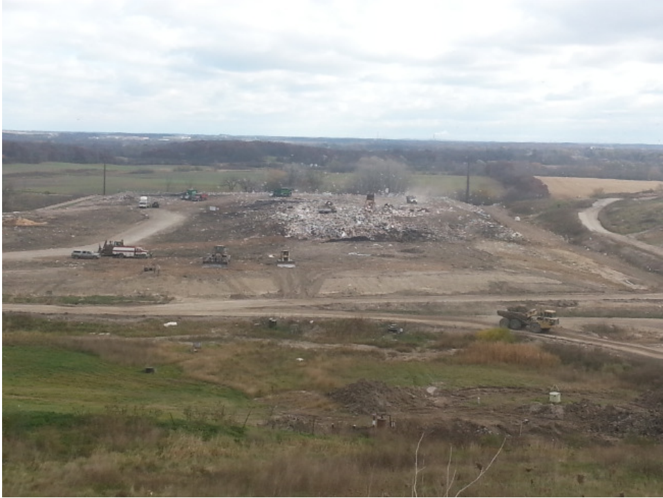
Working face in active area of Phase 9
