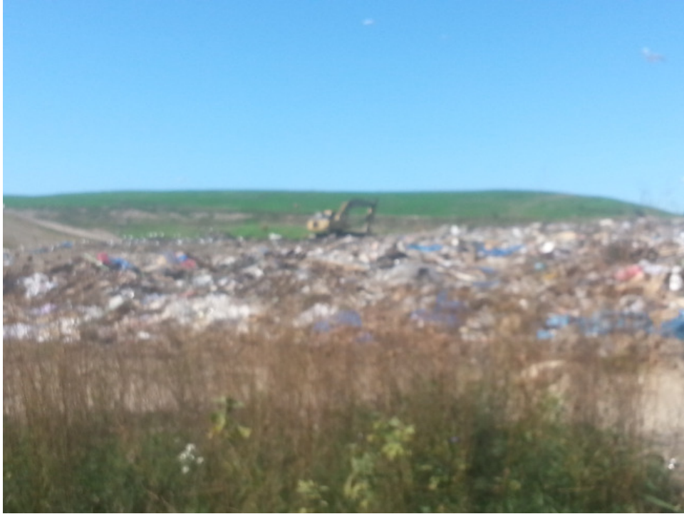
Active area viewed from the East
