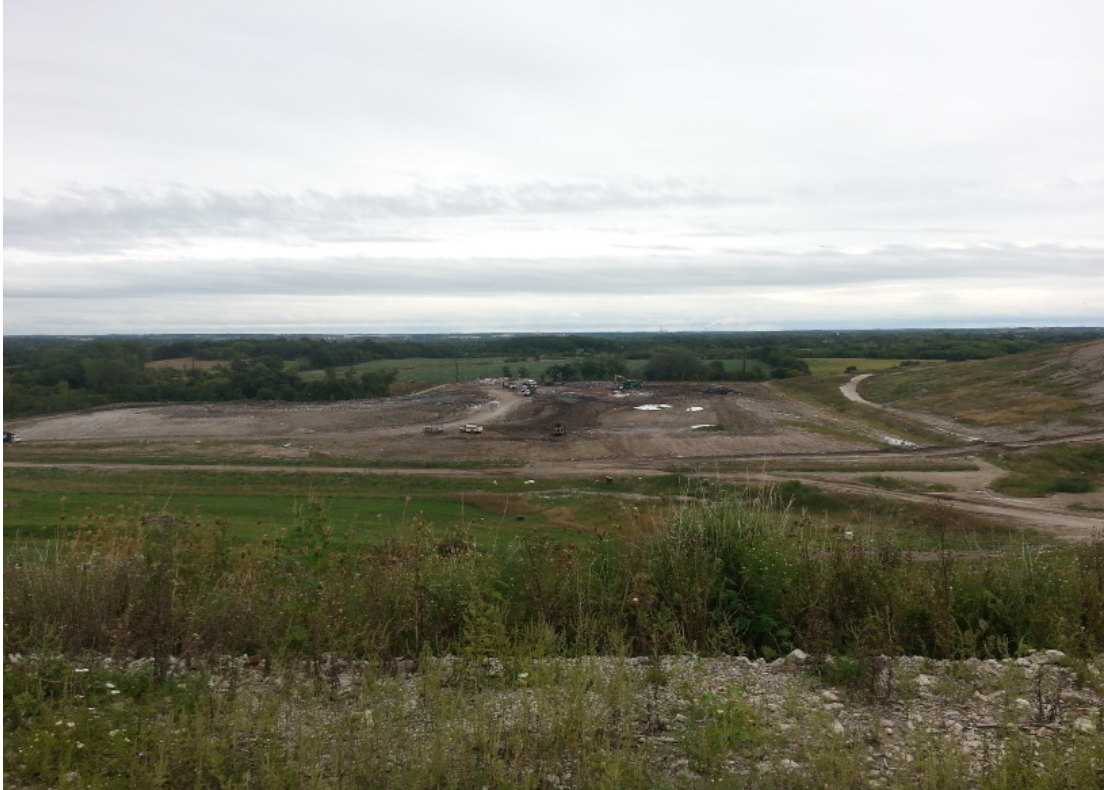
Phase 9 viewed from the West
