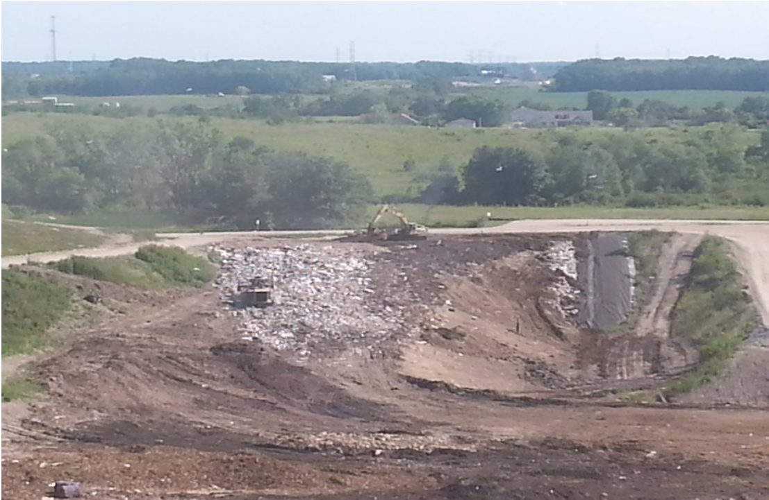
Working face on West slope of Phase 6, all wastes not suitable for fluff layer
