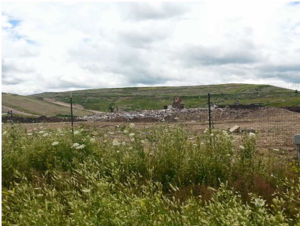
Active area viewed from the East
