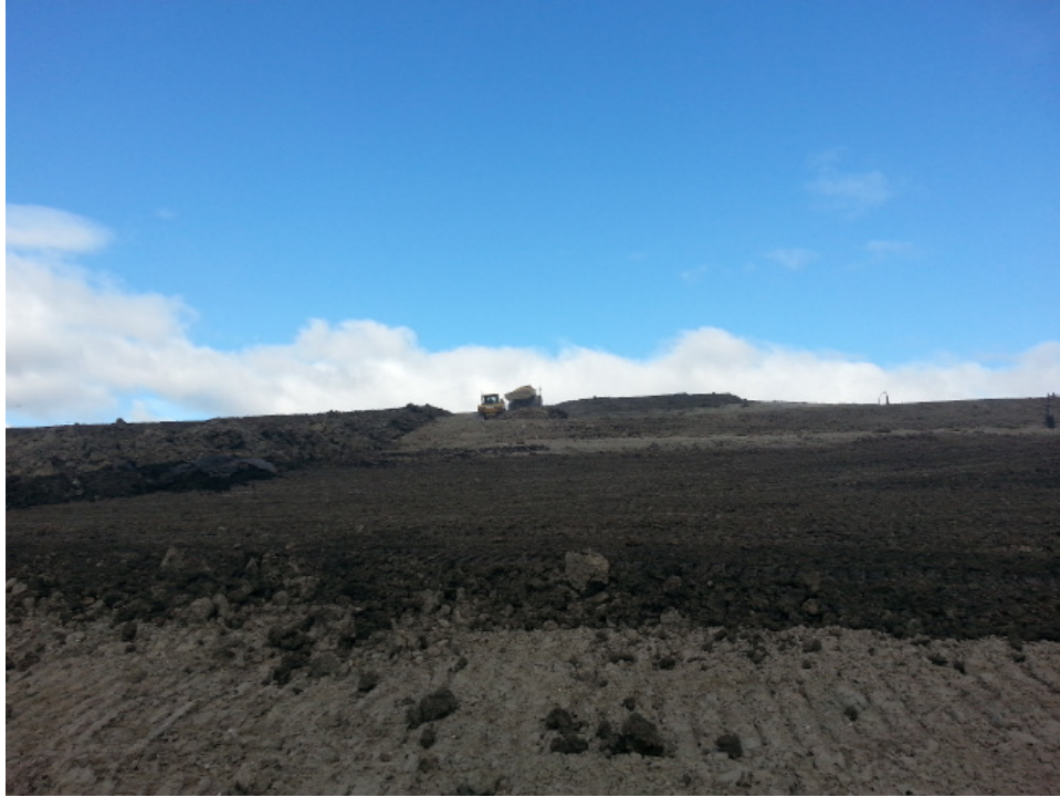
Diversion berm constructed of clay at top and mid-point of the slope.
