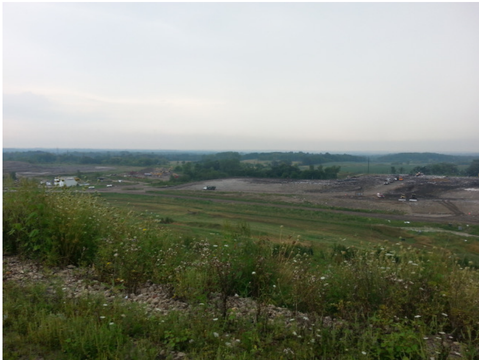
Phase 9 North end
