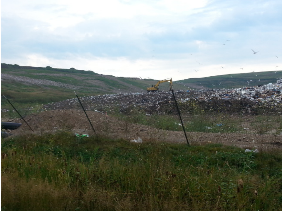
Active area viewed from Northeast
