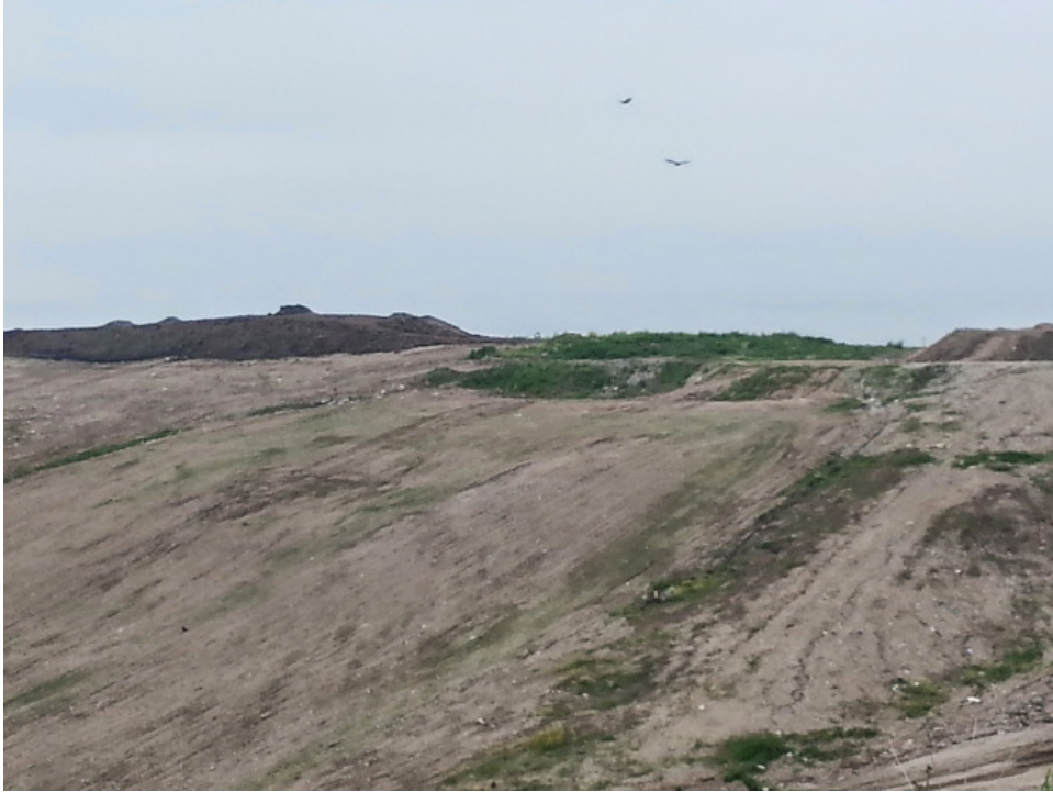
Phases 6 & 7, soil to be used on final cover.
