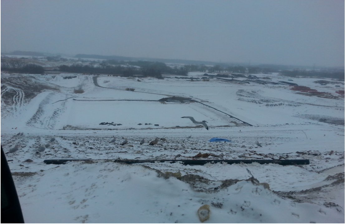
Phase 8 being prepared for berm construction
