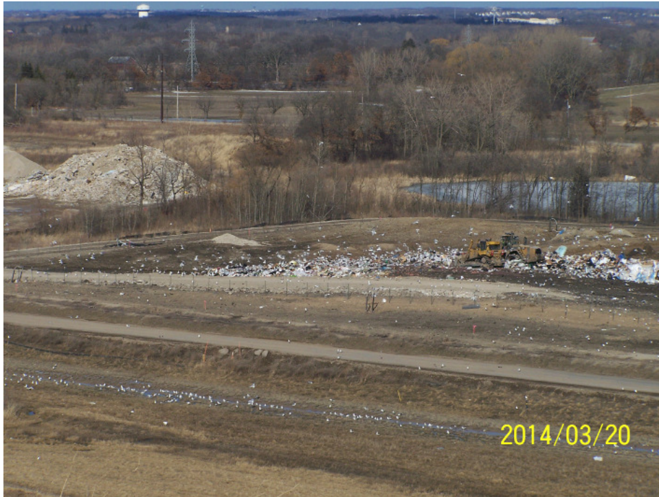
North end of Phase 9, and working face.
