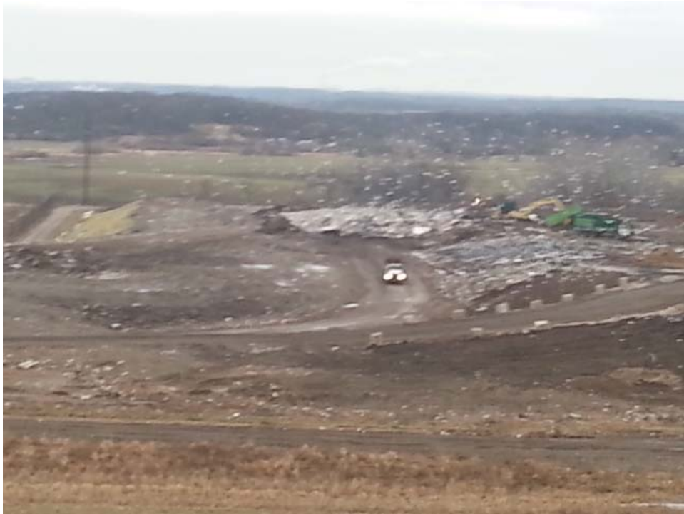
Working face in Northwest corner of Phase 9
