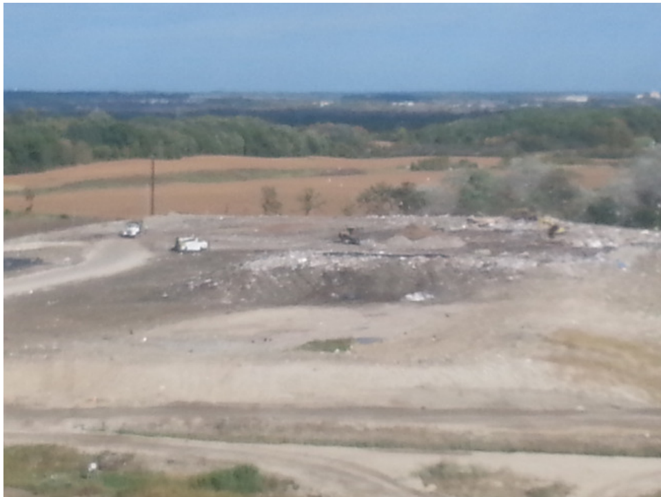
Phase 9, with working face in Southeast corner
