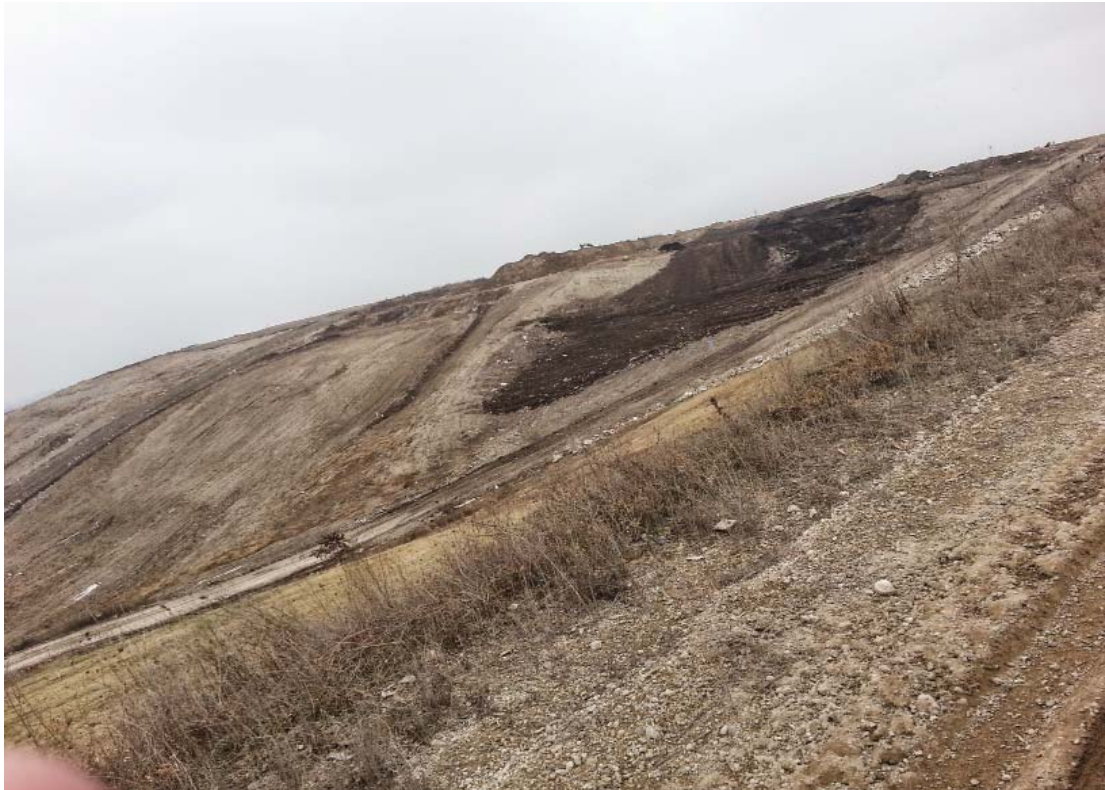
Seep repair on North slope of Phase 6
