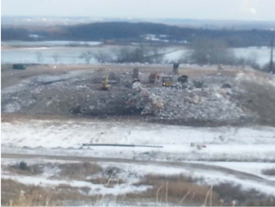
Working face, previous days cover in good condition
