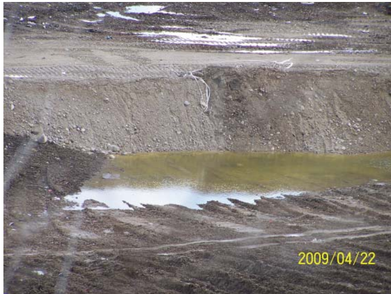
Ponding water noted on 4/22
