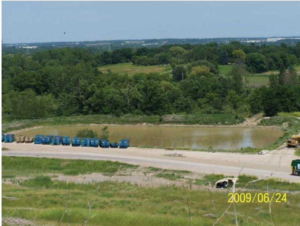
Drainage basin, now discharging around clear water pond.
