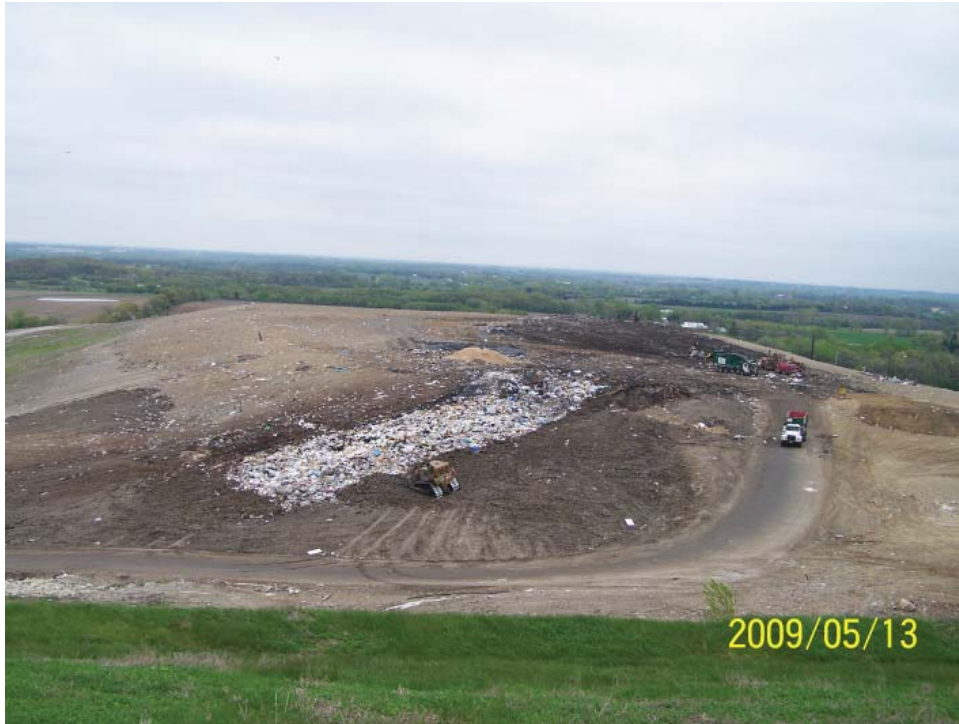
Active area. Waste from previous week well covered
