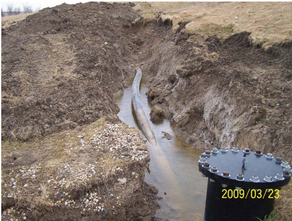
Pipe freed from settling soils, awaiting stone back fill.
