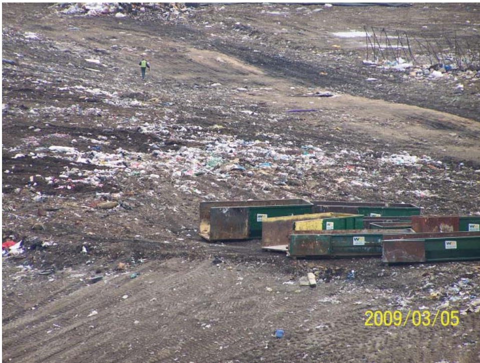
Severe flagging on active area
