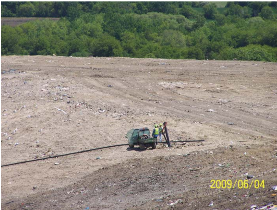
Intermediate cover on North side of Active area
