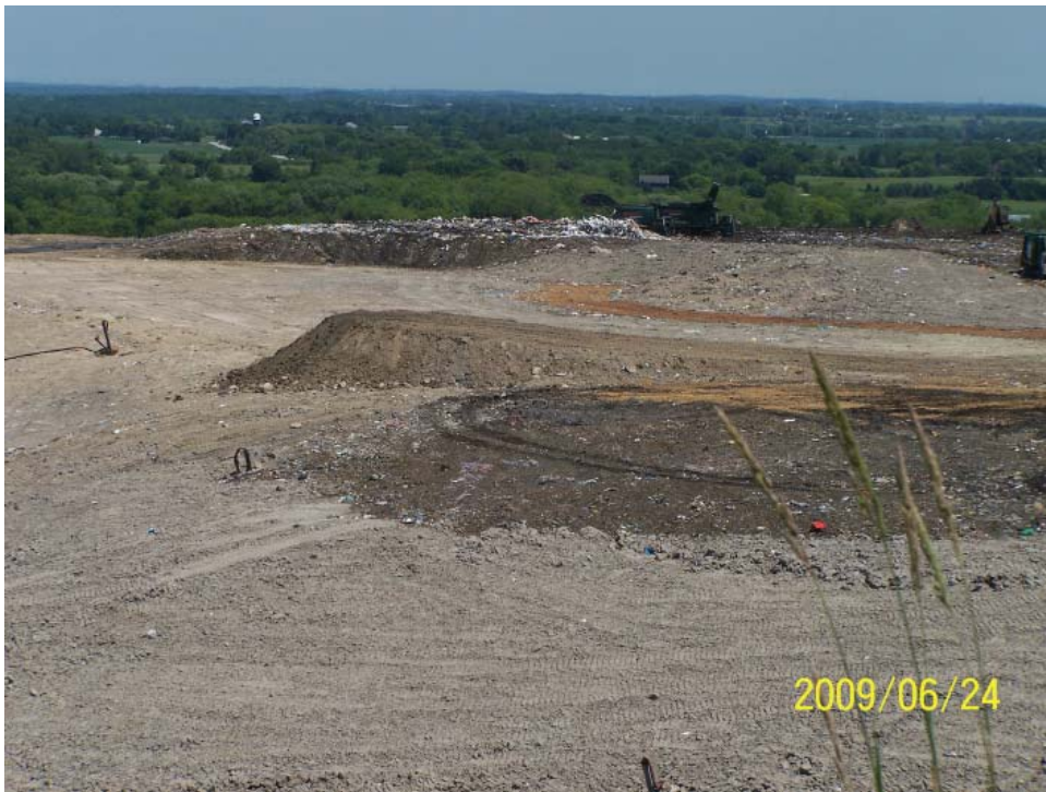
Stock piles of soil for cover
