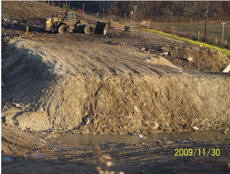
Ponding on cover at toe of bio soil pile
