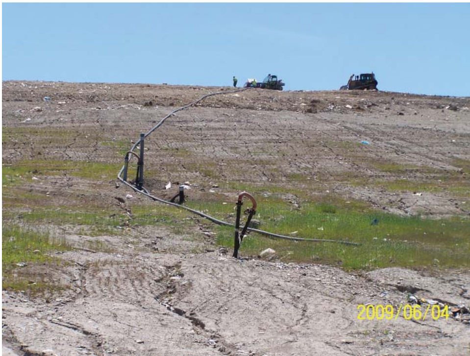
Eroded side slope and temporary gas header under installation.
