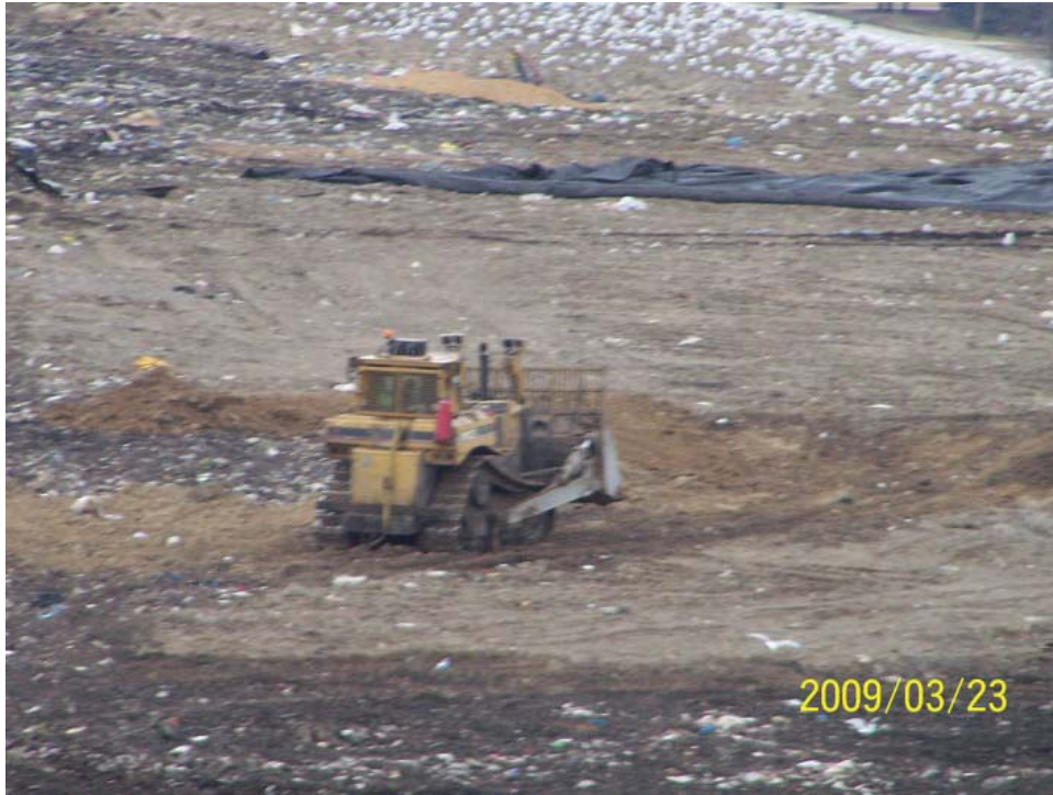
Dozer backdragging intermediated cover
