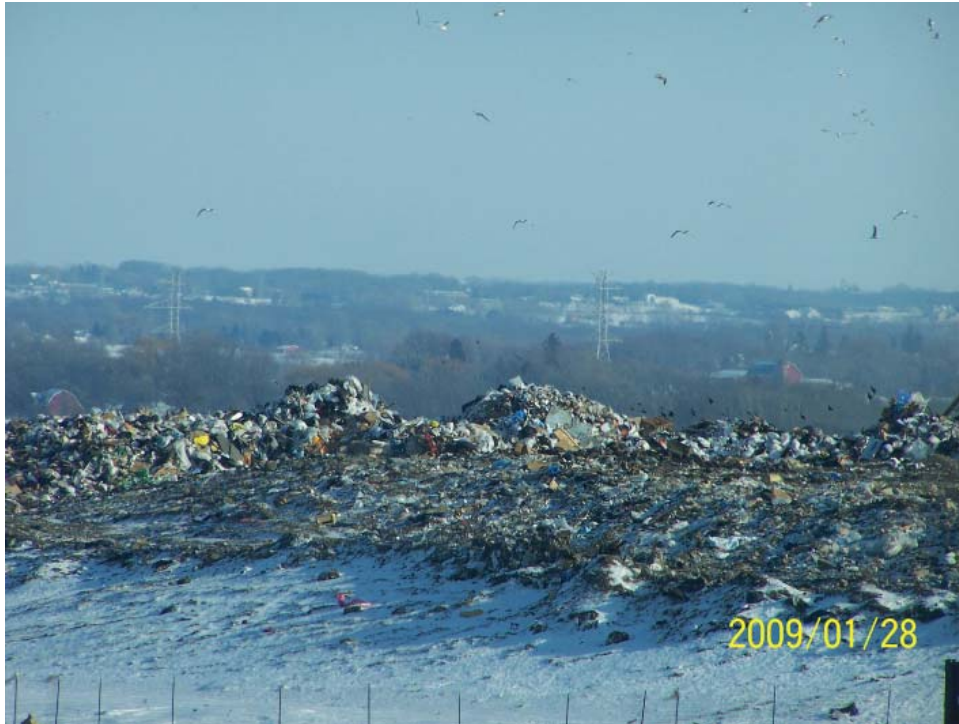
Working face, waste being pushed into place by dozer and not yet rolled by compactor.
