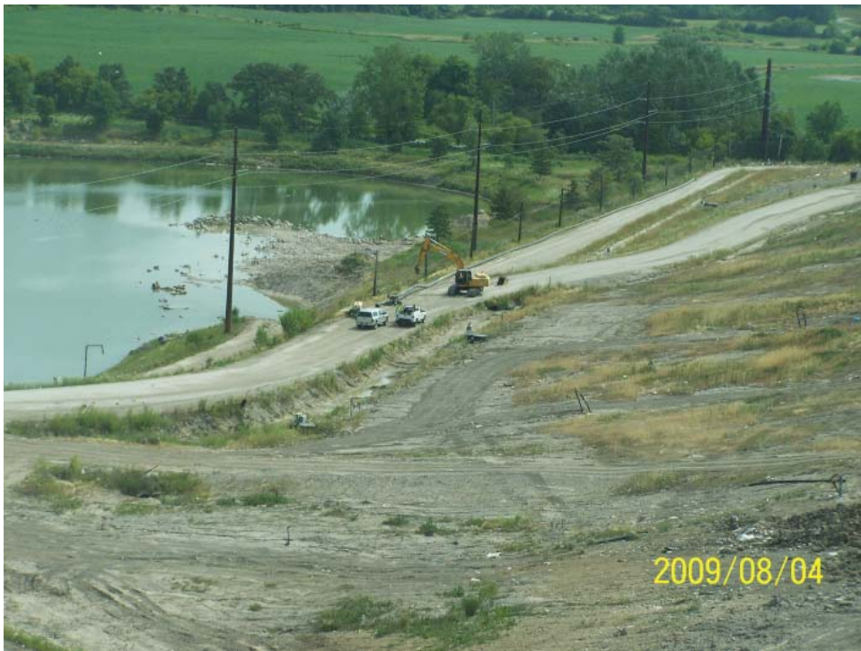
Terra preparing HDPE well pipe
