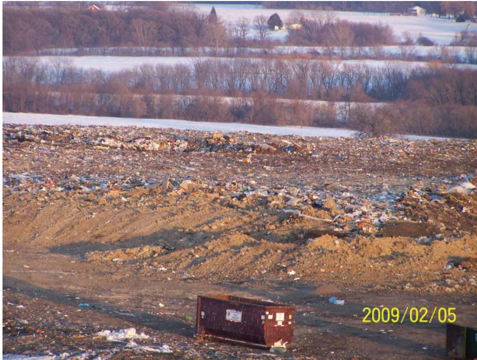
Heavy flagging on covered areas. Cover level through lift.
