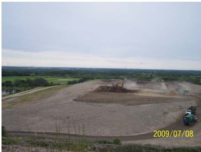
Intermediate cover well placed across active area and soils stockpiled for daily cover.
