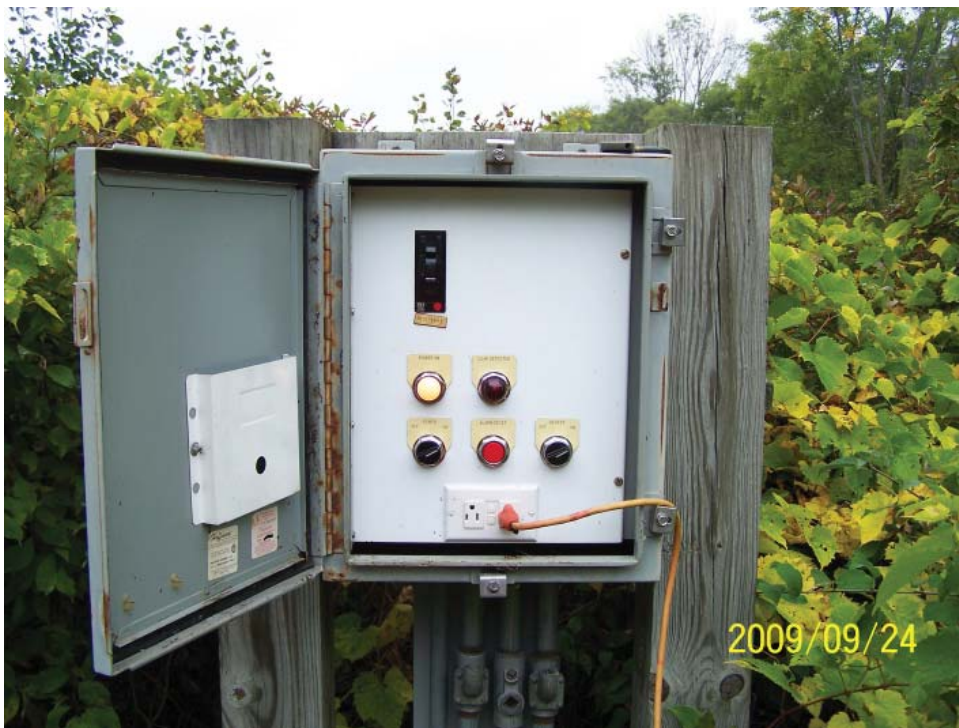
Unsecured panel for Manhole 4.
