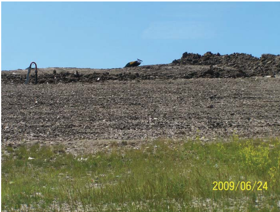
Eastern slope backdragged above grass line and new cover added
