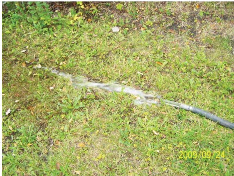
Discharge from forcemain, secondary containment, water only.
