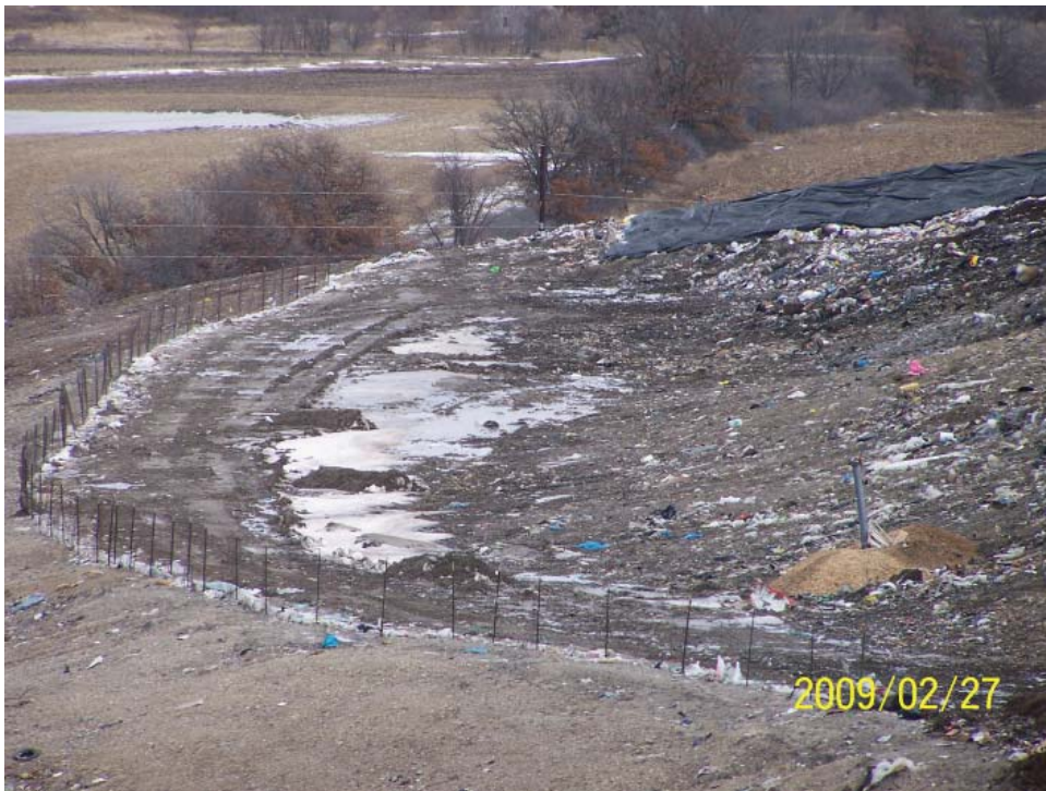
Tarp ADC cover and pooled water on daily cover
