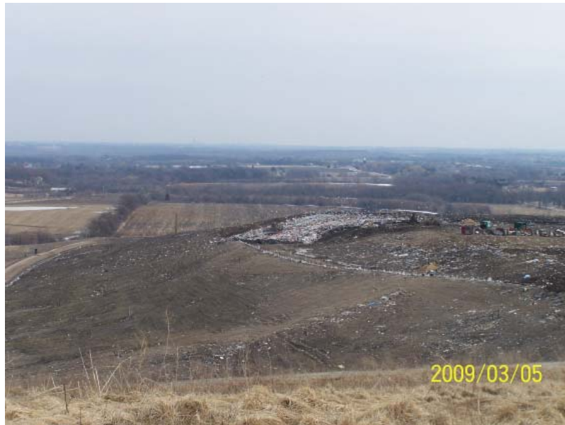
Current working face adjacent to area of exposed waste in last audit. Cover at corner more than adequate
