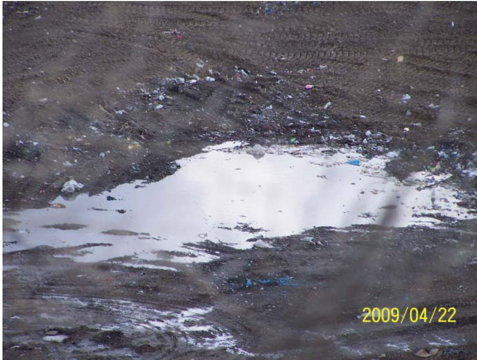
Ponding water in old solidification tank location noted on 4/22
