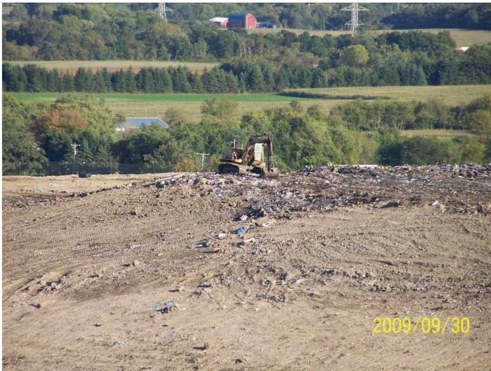
Intermediate cover in Northwest corner of Active area
