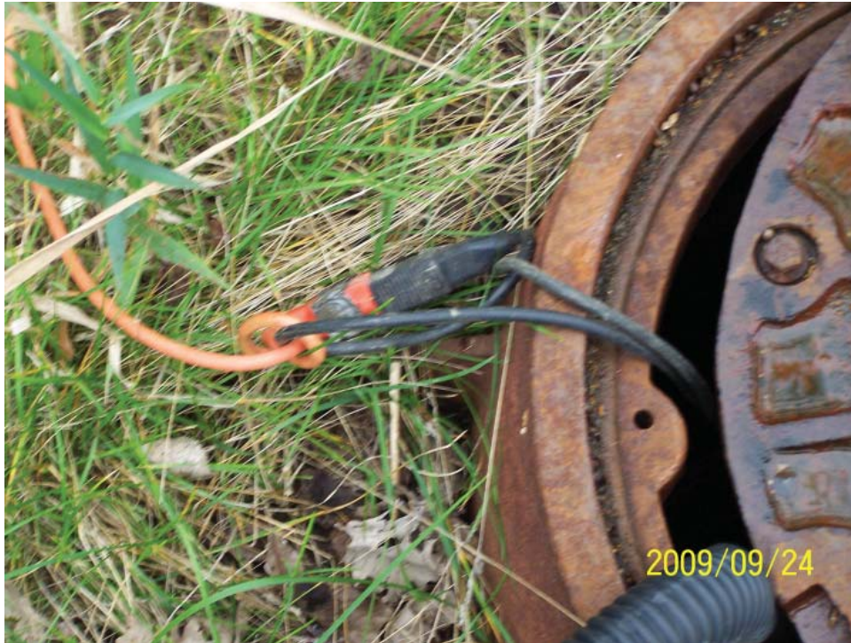
Extention cord to power pump
