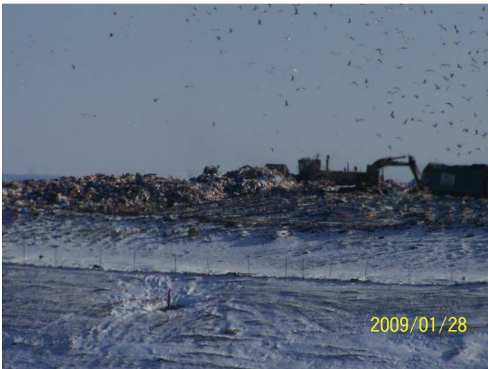
Compactor entering working face
