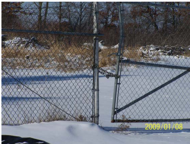
Rear gate damage or in disrepair.
