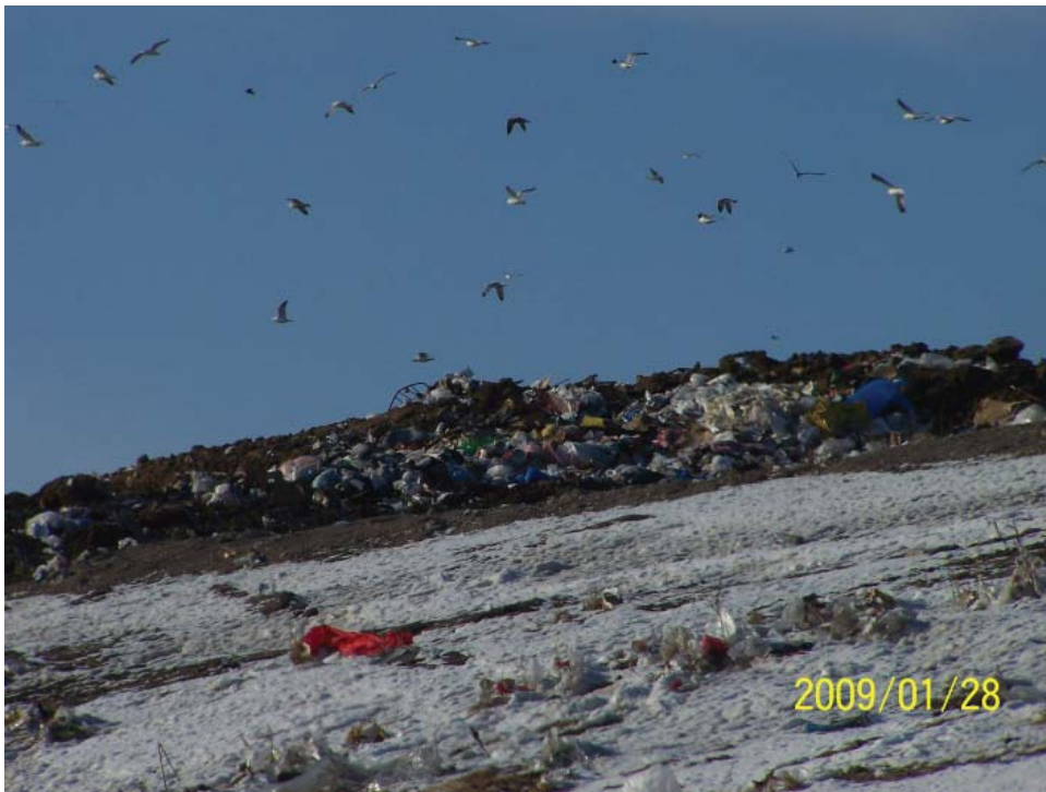
Exposed waste to be covered at end of day on South top of slope, previous days tarp cover location
