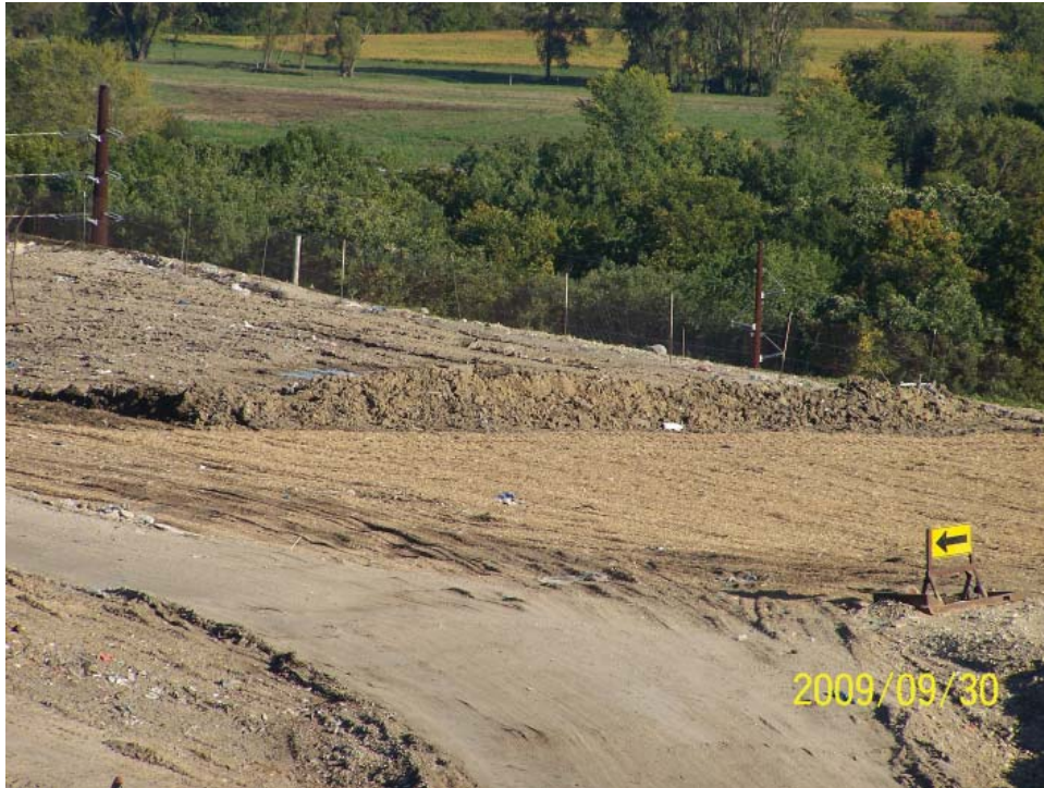
Intermediate Cover on South side of Active area
