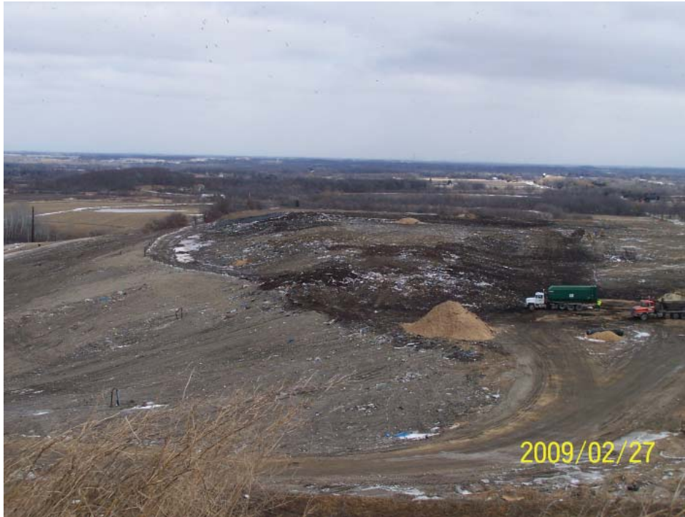
North half of active area, flagging and tarp still from yesterday as cover.
