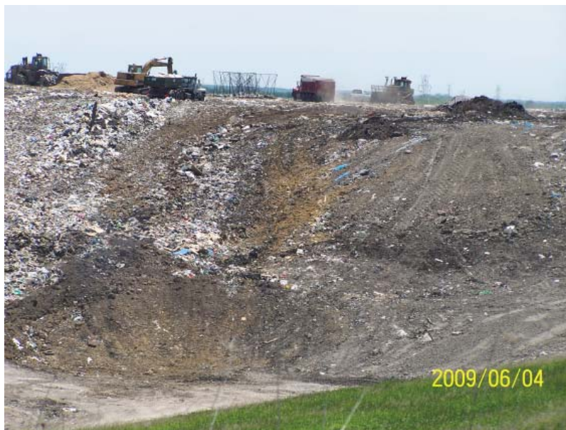
Working face on slope to recovery area lost to solidification tank
