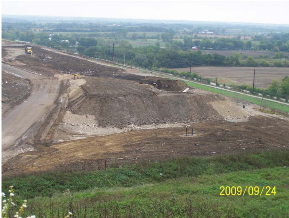
Bio soils stockpiled for treatment
