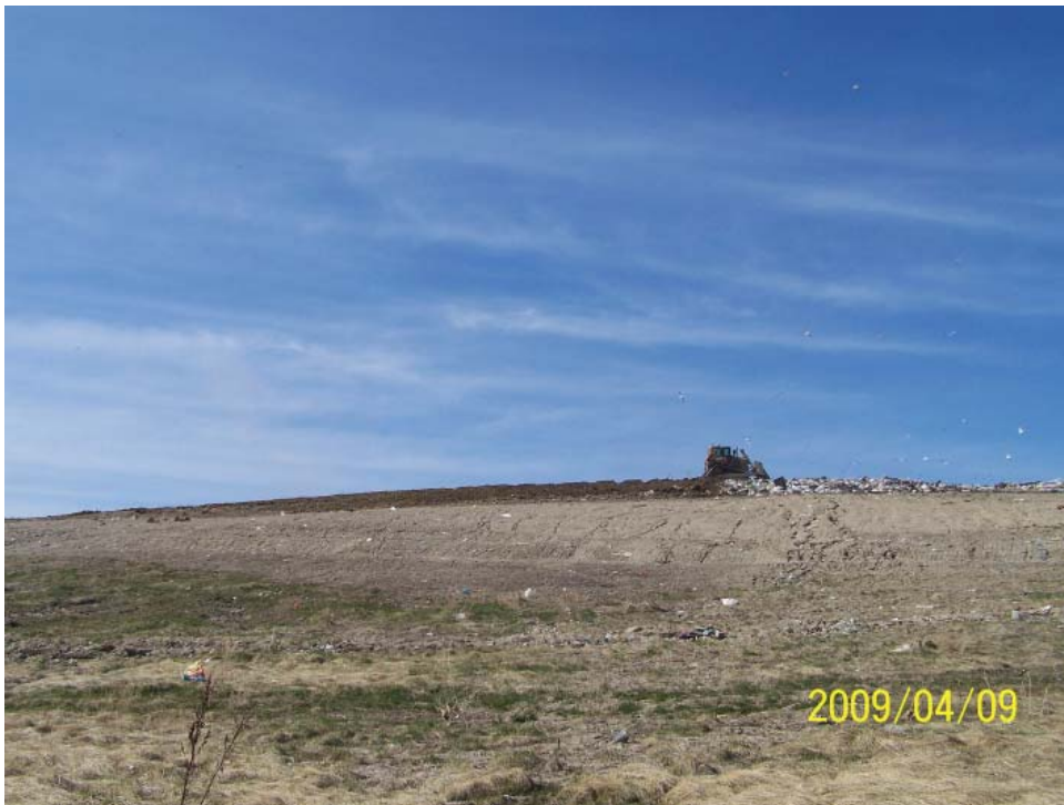
Intermediate cover placed over waste
