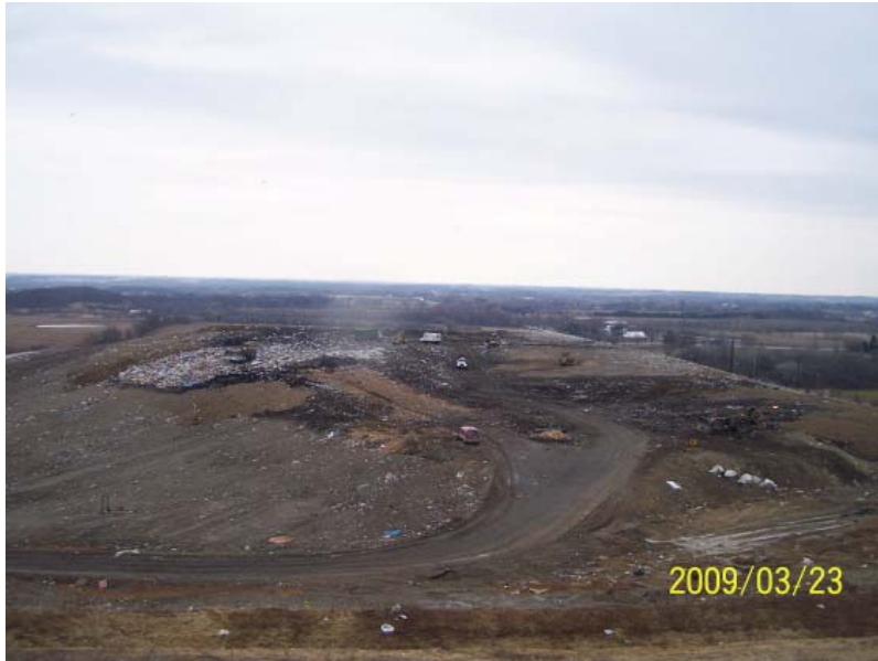
Active area viewed from the West, cover conditions greatly improved
