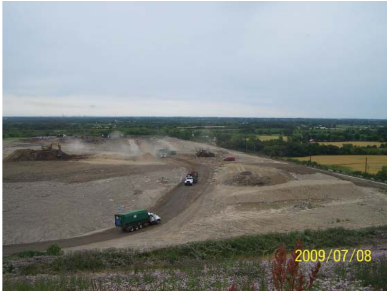
Active area, good cover though dusty conditions. Not access road recently wetted
