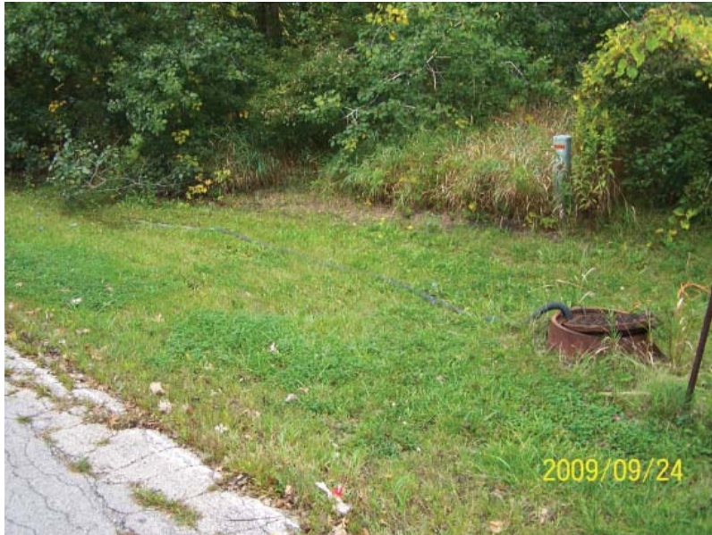
Manhole #4 of the forcemain system.
