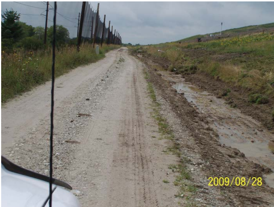
Perimeter ditches have been cleaned of silt and reshaped.
