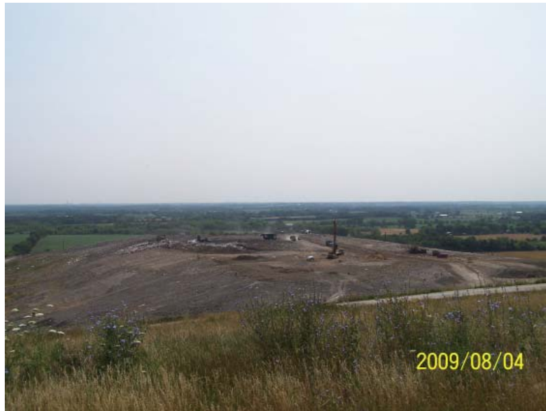
Active area, with drill rig in center
