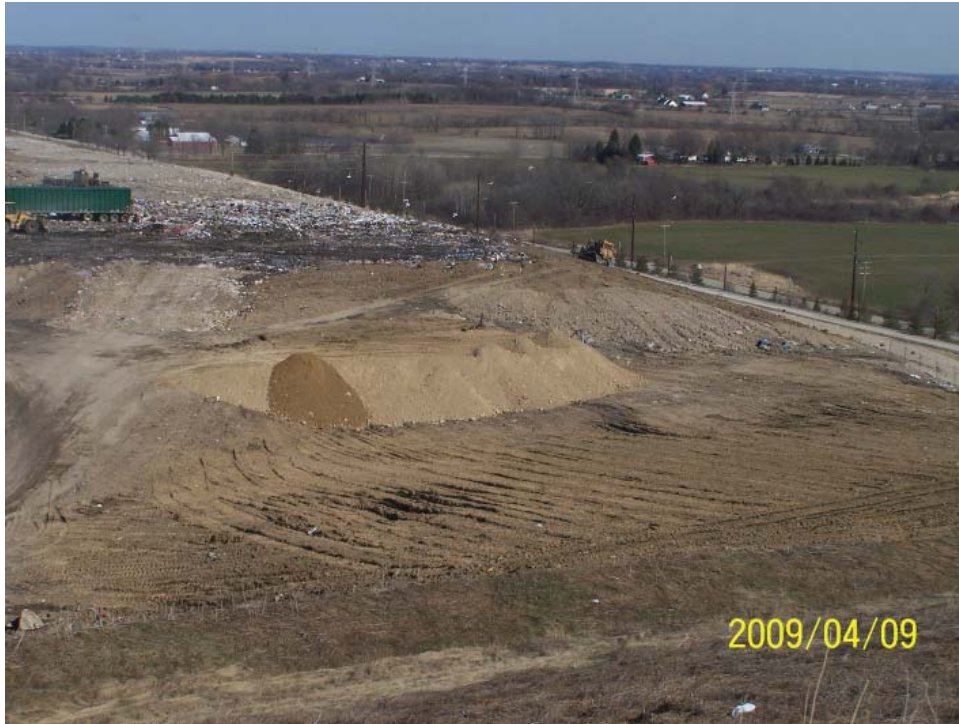
New bio soil pile East of existing bio soils
