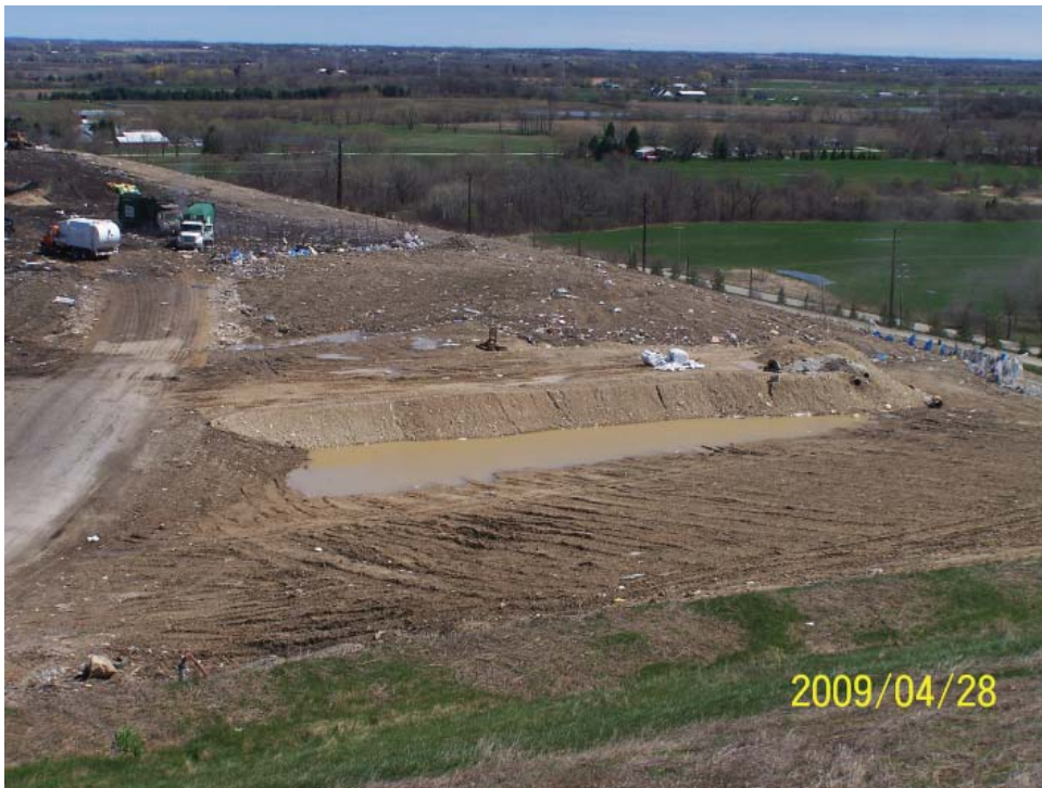
Cover and remaining ponding.
