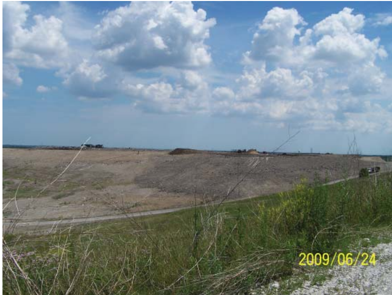
Intermediate cover placed over area previous audits working face
