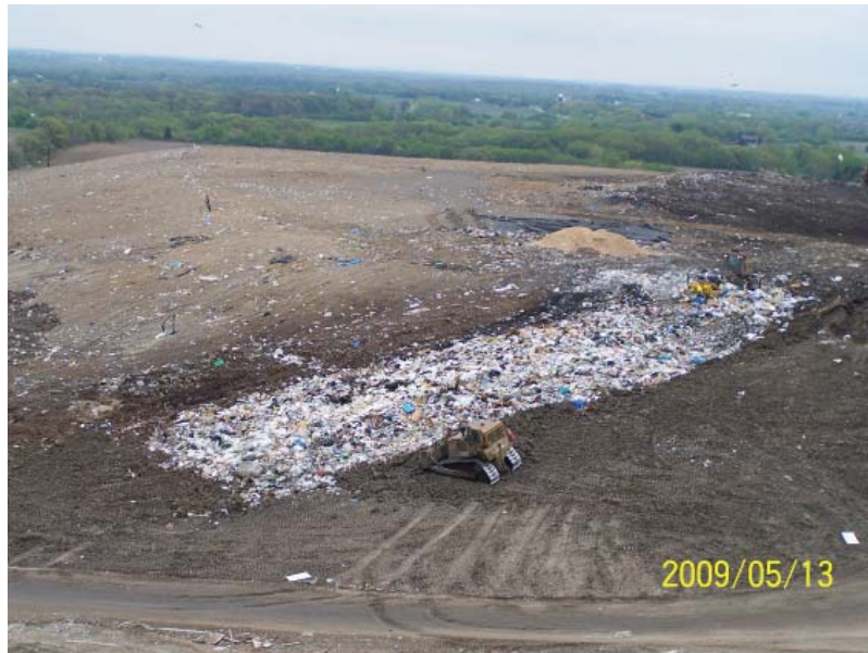
Working face placed to fill in area around previous solidification tank
