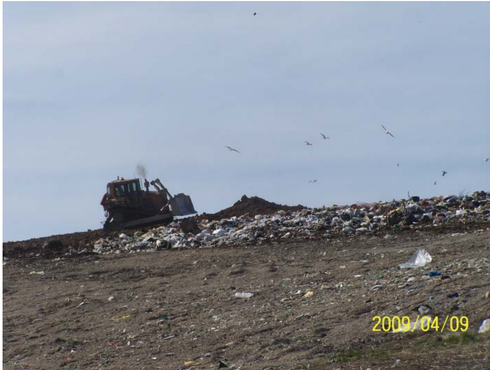
Intermediate cover being placed across South slope
