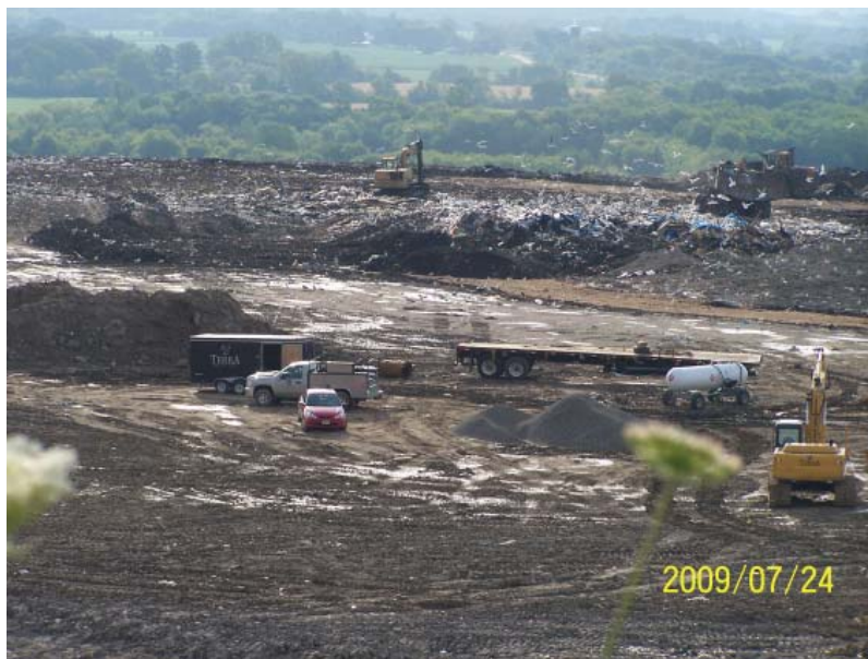
Staging area for gas well construction
