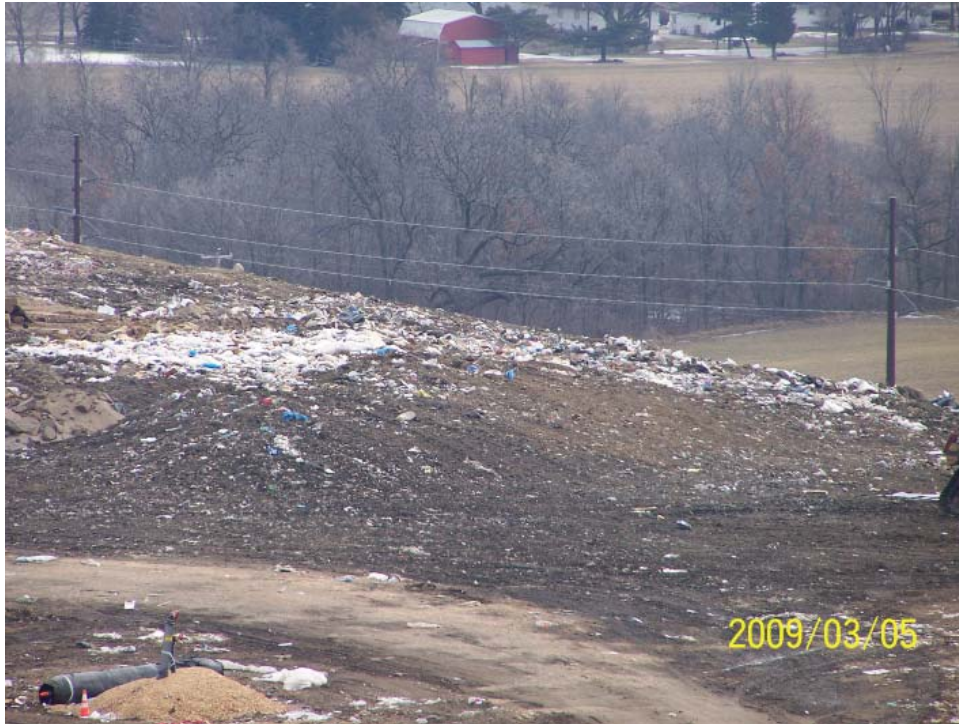
Location of working face at last audit. Cover is poor, flagging or exposed waster present
