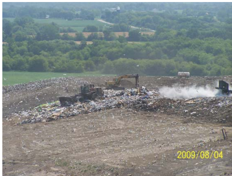
Working face on North Slope
