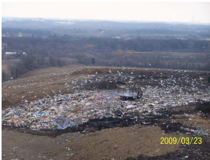
Working face in Northwest corner above solidification tank
