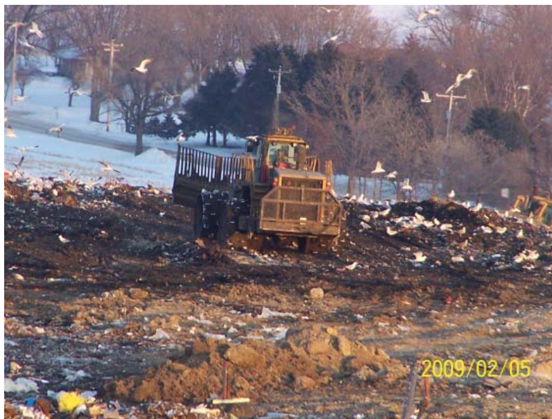
Compactor spreading cover on top of lift
