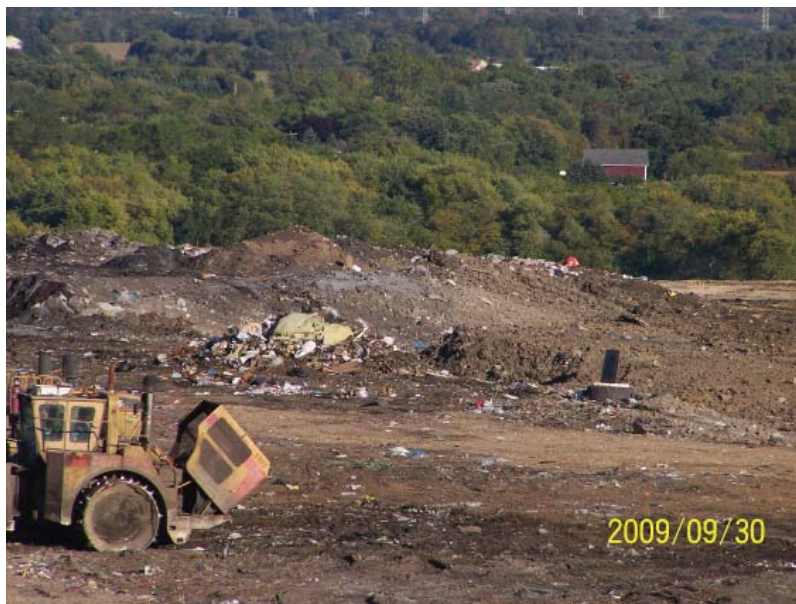
Foundry Sands and Soils stockpiled for cover
