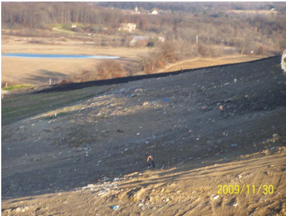
North slope of active area, topsoil placed at Northeast corner
