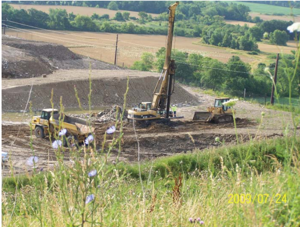
Terra drilling gas well
