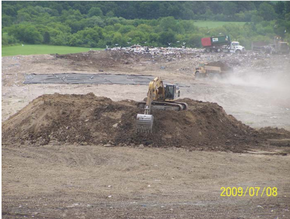
Stockpile soils being harvested for daily cover
