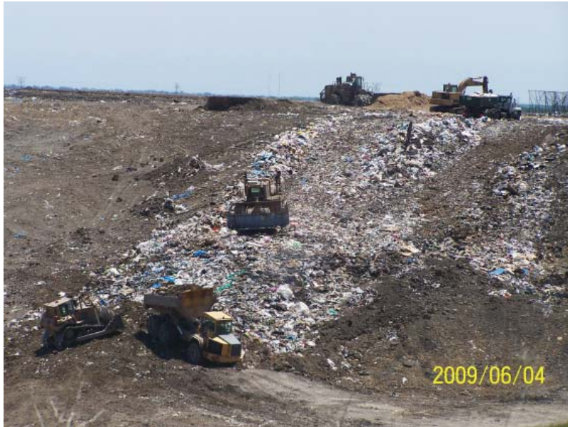
Working face, soil being stockpile for cover at base of face
