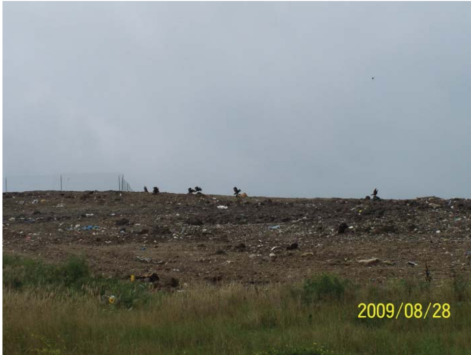
East out board slope, awaiting top soil coverage
