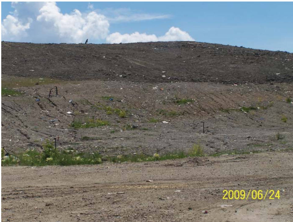
Upper portion of Northwest corner covered with new clay
