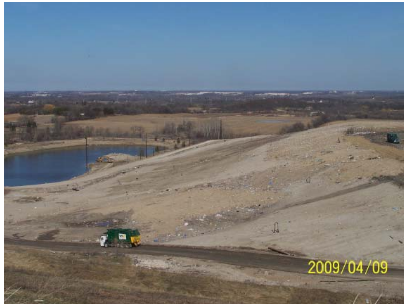
North side of active area, solidification tank has been removed and filled
