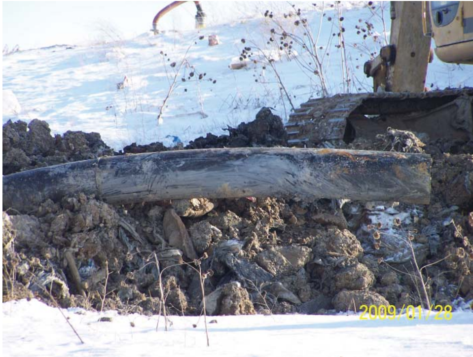
Damaged pipe removed while new pipe is being connected
