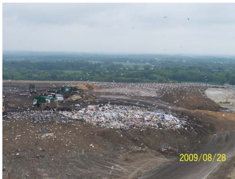
Working face at top of West access road
