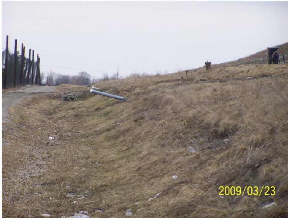
Sediment in ditch reduces capacity
