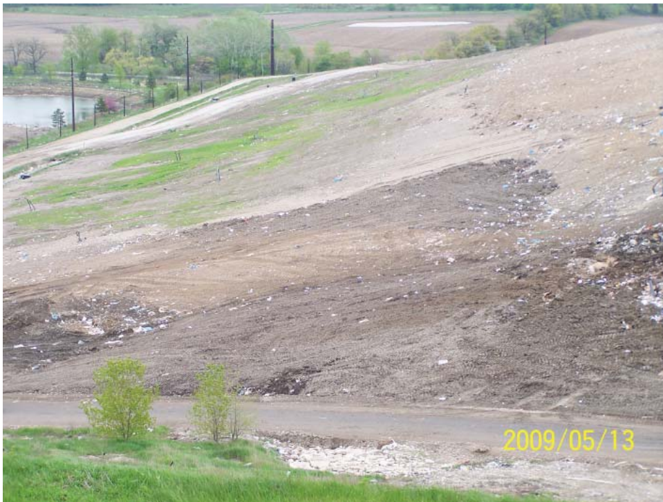
Areas of repaired and newly placed intermediate cover
